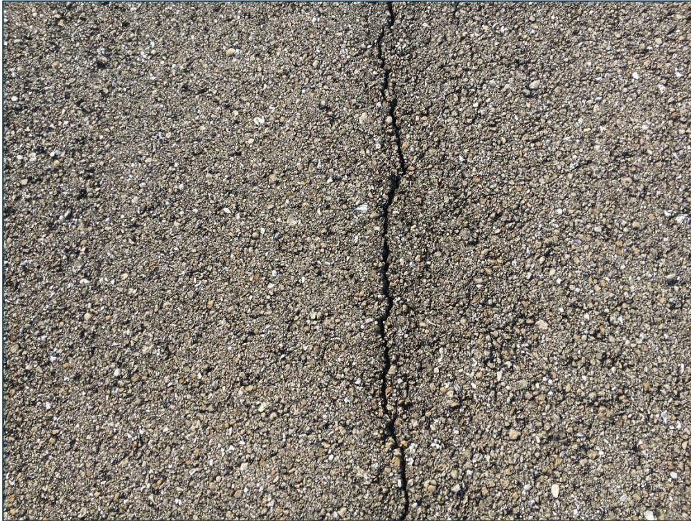
Runway 14-32, Section 6205, Sample Unit 101 – Low Severity (48) Longitudinal and Transverse Cracking, Low Severity (57) Weathering
