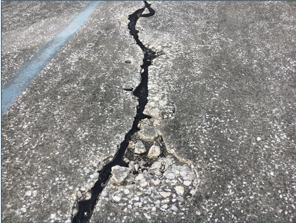
Apron, Section 4105, Sample Unit 429 – High Severity (63) Longitudinal, Transverse, and Diagonal Cracking
