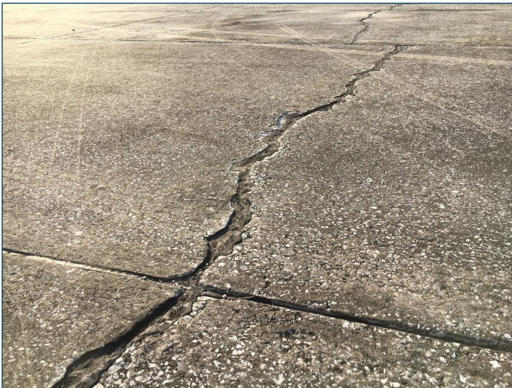
Apron, Section 4105, Sample Unit 301 – Medium Severity (63) Longitudinal, Transverse, and Diagonal Cracking, Medium Severity (65) Joint Seal Damage
