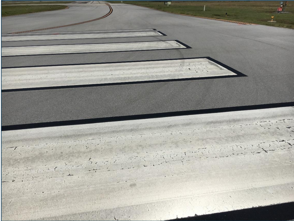
Runway 01-19, Section 6105, Sample Unit 204 – Low Severity (57) Weathering
