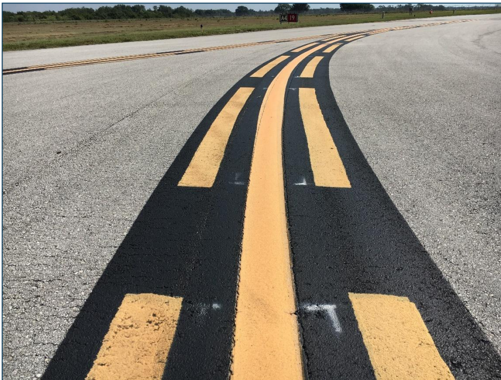
Taxiway A, Section 420, Sample Unit 254 – Low Severity (48) Longitudinal and Transverse Cracking, Low Severity (52) Raveling, Low Severity (57) Weathering
