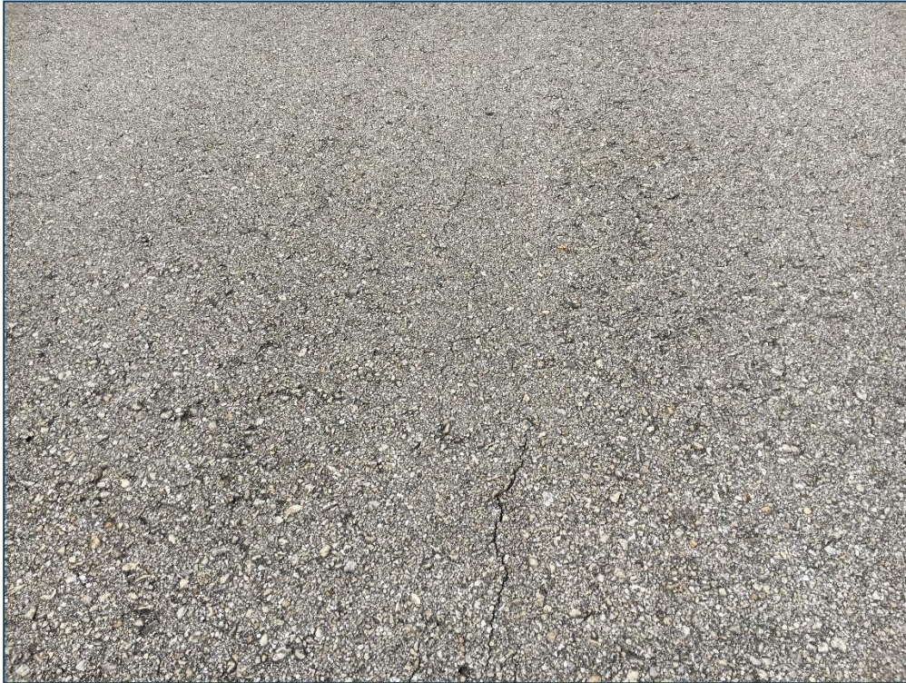
Taxiway A, Section 405, Sample Unit 233 – Low Severity (48) Longitudinal and Transverse Cracking, Low Severity (57) Weathering
