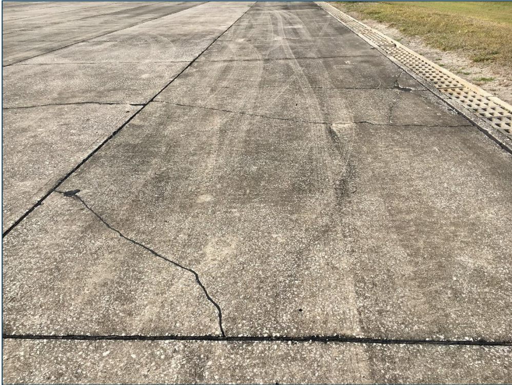
Apron, Section 4105, Sample Unit 114 – Medium Severity (72) Shattered Slab
