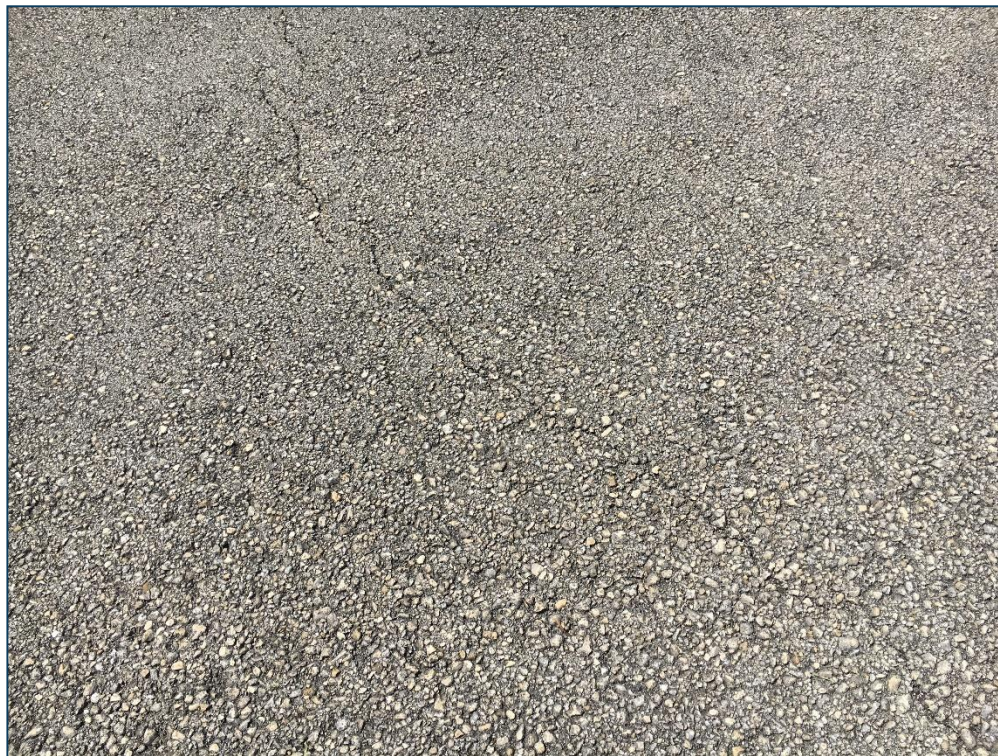
Taxiway A, Section 405, Sample Unit 207 – Low Severity (48) Longitudinal and Transverse Cracking, Low Severity (52) Raveling, Low Severity (57) Weathering
