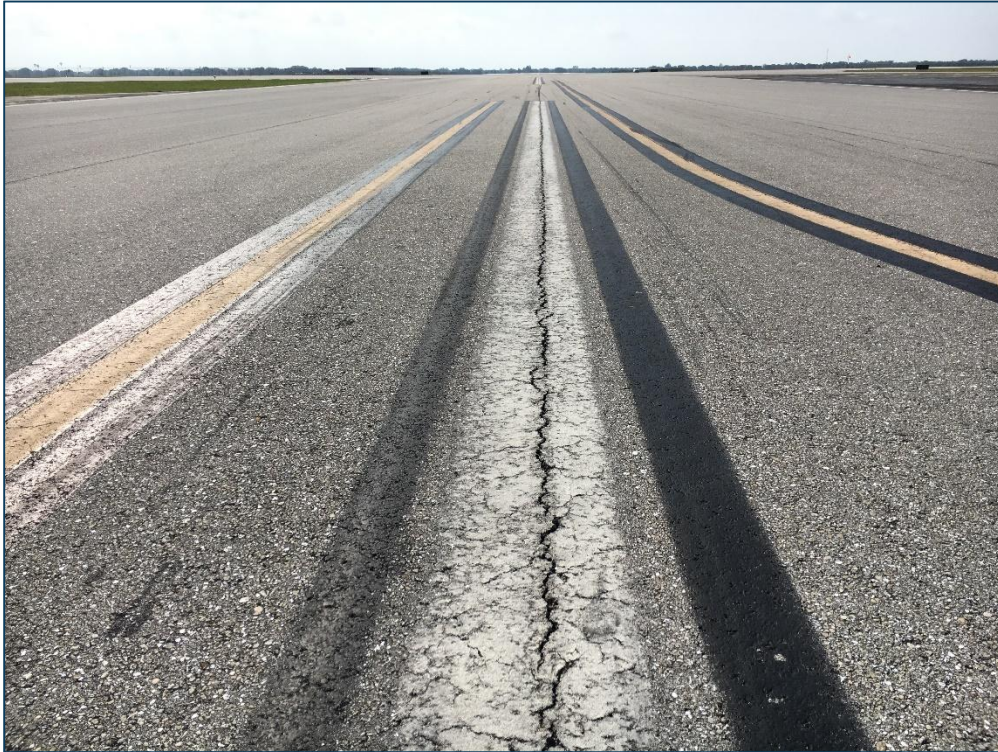
Runway 14-32, Section 6205, Sample Unit 170 – Low Severity (48) Longitudinal and Transverse Cracking, Low Severity (57) Weathering
