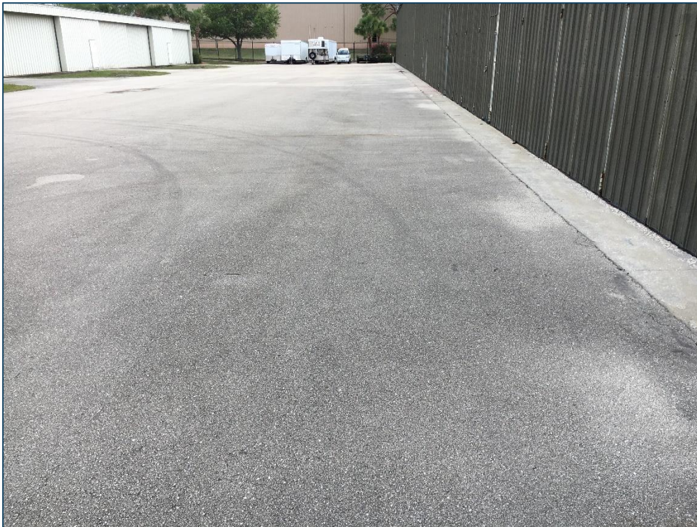
T-Hangar Apron, Section 4125, Sample Unit 102 – Low Severity (52) Raveling, Low Severity (57) Weathering
