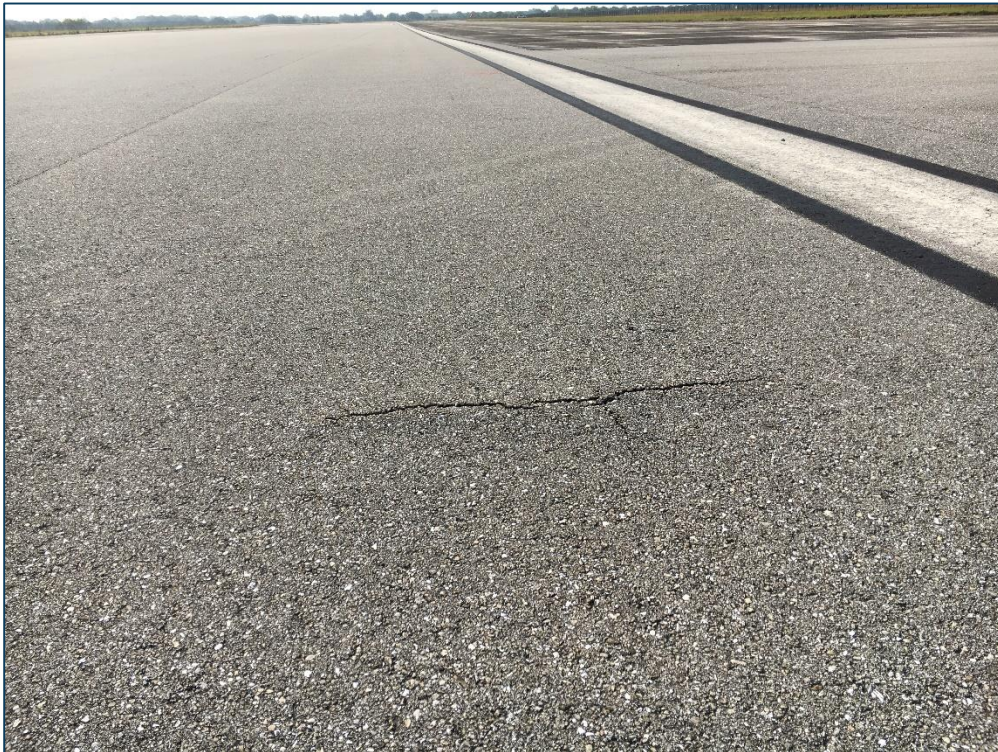
Runway 14-32, Section 6205, Sample Unit 133 – Low Severity (48) Longitudinal and Transverse Cracking, Low Severity (56) Swelling, Low Severity (57) Weathering
