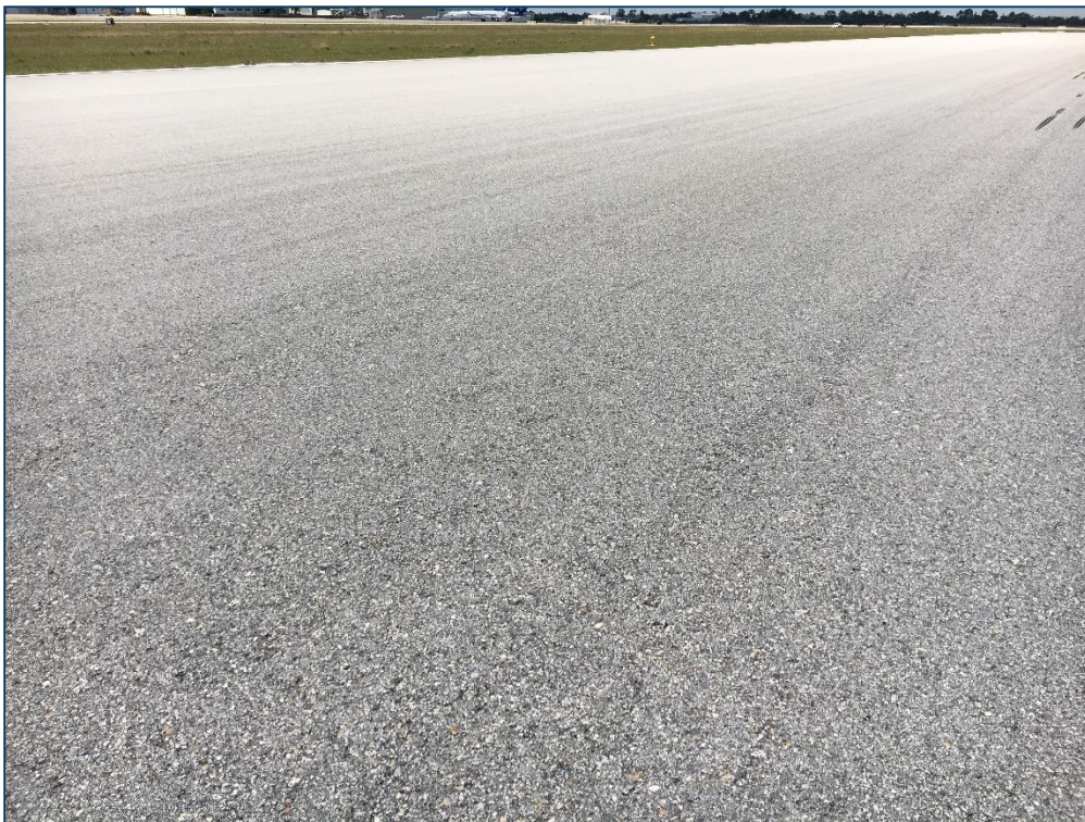
Runway 01-19, Section 6105, Sample Unit 157 – Low Severity (57) Weathering
