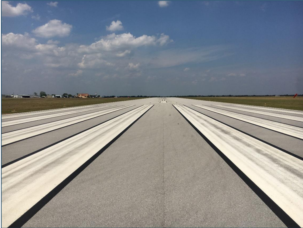
Runway 01-19, Section 6105, Sample Unit 100 – Low Severity (57) Weathering
