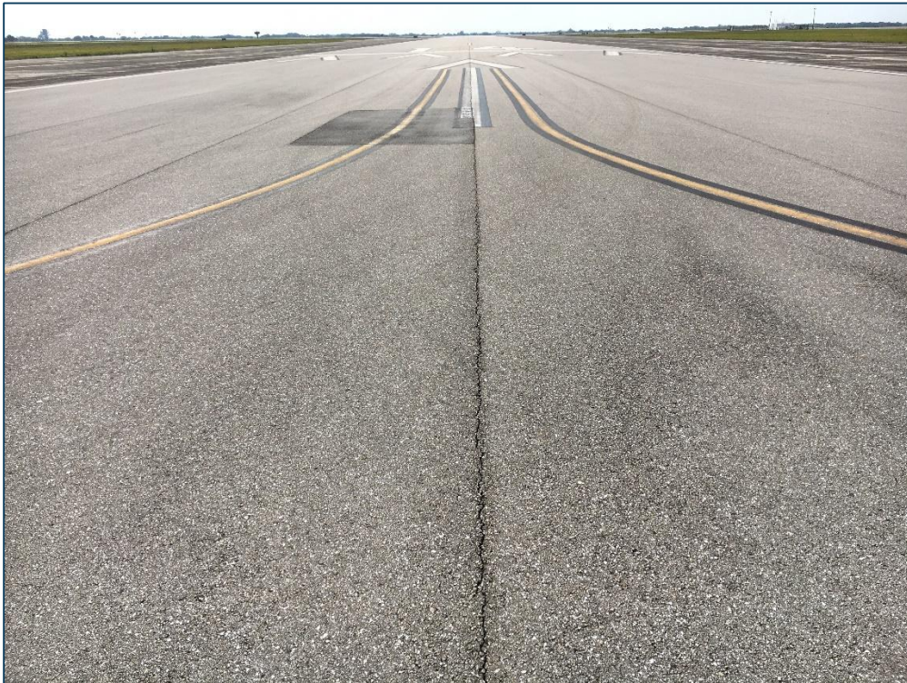
Runway 14-32, Section 6205, Sample Unit 198 – Low Severity (48) Longitudinal and Transverse Cracking, Low Severity (50) Patching, Low Severity (57) Weathering
