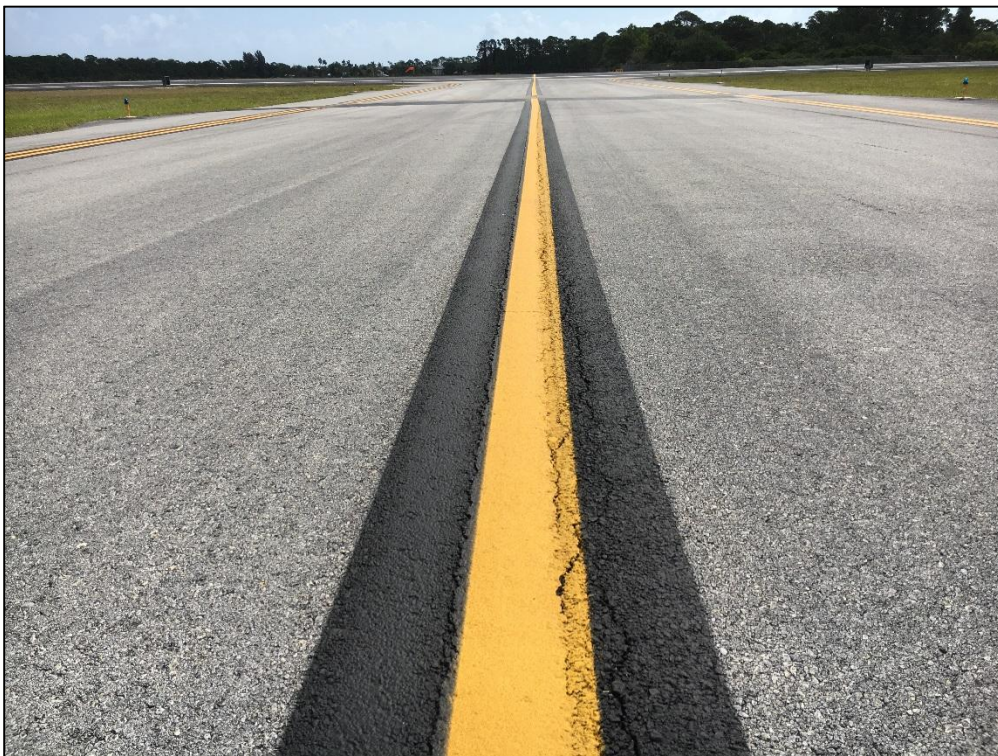
Taxiway C, Section 305, Sample Unit 420 - Low Severity (48) Longitudinal and Transverse Cracking, Low Severity (57) Weathering
