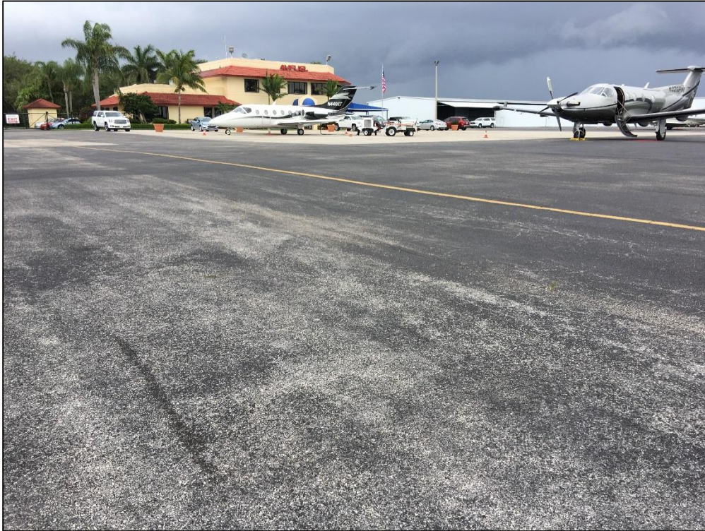
East Apron, Section 4205, Sample Unit 208 - Low Severity (52) Raveling, Low Severity (57) Weathering
