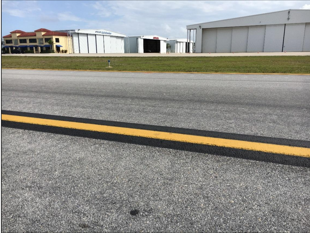
Taxiway A, Section 110, Sample Unit 225 - Low Severity (48) Longitudinal and Transverse Cracking, Low Severity (53) Rutting, Low Severity (57) Weathering
