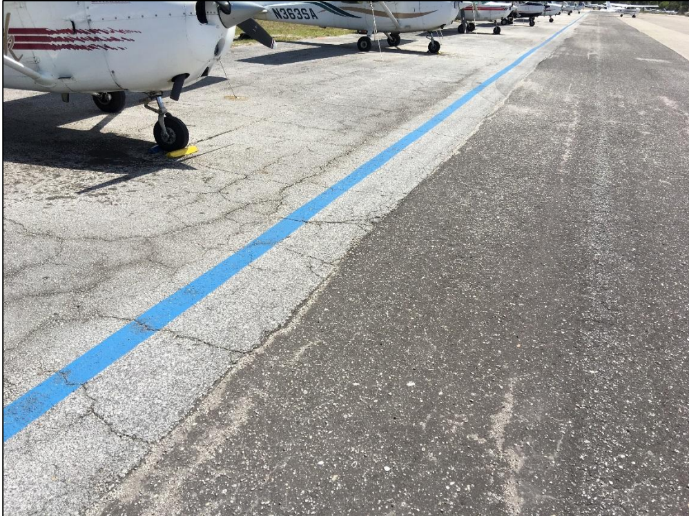
East Apron, Section 4235, Sample Unit 54 - Low Severity (43) Block Cracking, Medium Severity (52) Raveling
