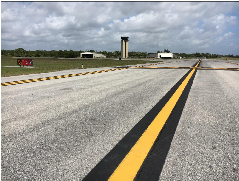
Taxiway D, Section 405, Sample Unit 320 - Low Severity (48) Longitudinal and Transverse Cracking, Low Severity (57) Weathering
