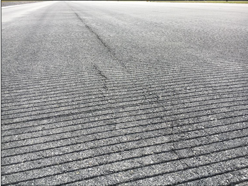
Runway 7-25, Section 6205, Sample Unit 389 - Low Severity (48) Longitudinal and Transverse Cracking, Low Severity (56) Swelling, Low Severity (57) Weathering
