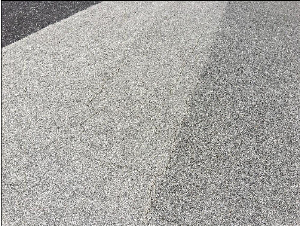
Taxiway C, Section 330, Sample Unit 902 - Low Severity (43) Block Cracking, Medium Severity (52) Raveling
