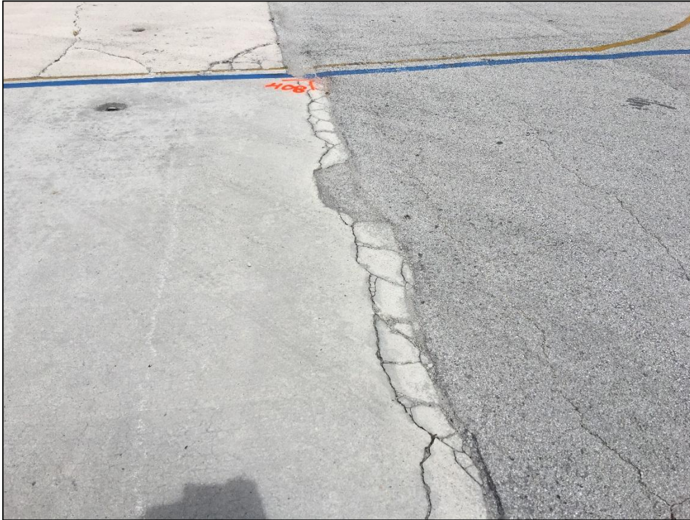
West Apron, Section 4110, Sample Unit 408 - High Severity (65) Joint Seal Damage, High Severity (74) Joint Spall, Medium Severity (75) Corner Spall
