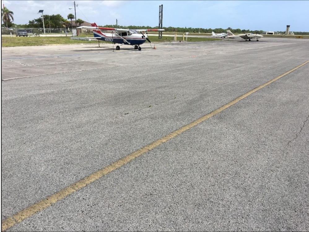
Taxiway B, Section 205, Sample Unit 207 - Medium Severity (52) Raveling, Low Severity (53) Rutting
