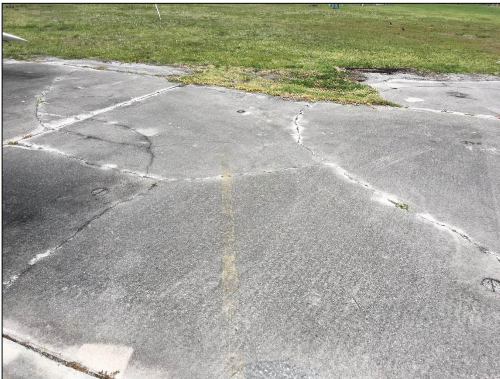
West Apron, Section 4110, Sample Unit 404 – Medium Severity (72) Shattered Slab
