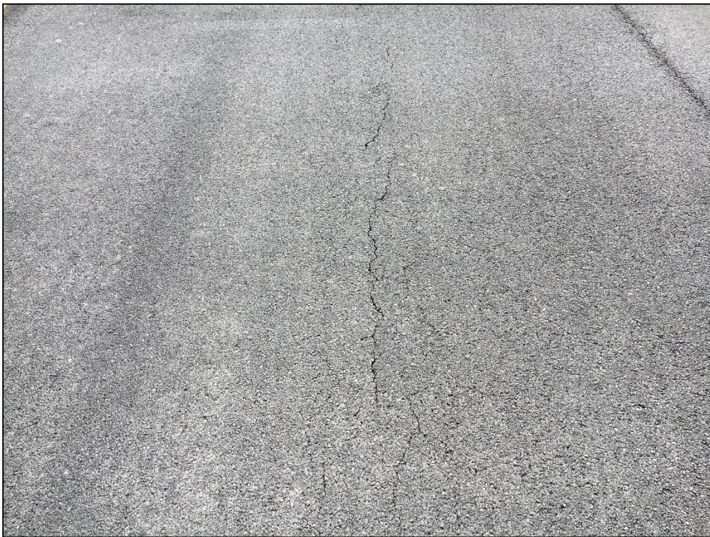
Taxiway A, Section 110, Sample Unit 204 - Low Severity (48) Longitudinal and Transverse Cracking, Low Severity (57) Weathering
