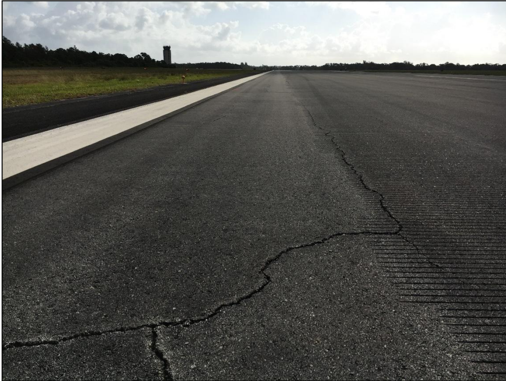
Runway 7-25, Section 6205, Sample Unit 315 - Low Severity (48) Longitudinal and Transverse Cracking, Low Severity (56) Swelling, Low Severity (57) Weathering
