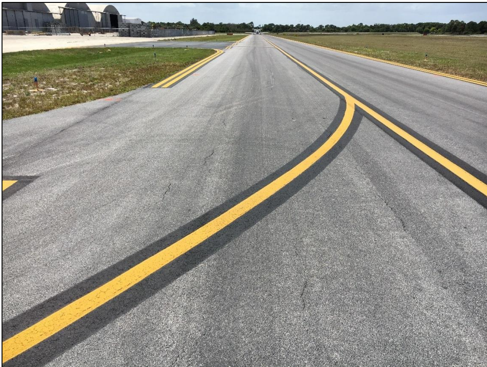
Taxiway A, Section 105, Sample Unit 112 - Low Severity (48) Longitudinal and Transverse Cracking, Low Severity (52) Raveling, Low Severity (56) Swelling, Low Severity (57) Weathering
