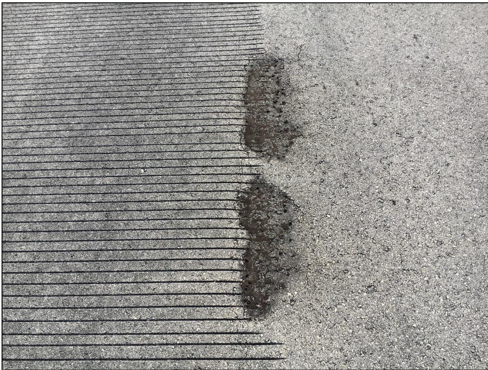
Runway 7-25, Section 6205, Sample Unit 319 - (42) Bleeding, Low Severity (48) Longitudinal and Transverse Cracking, Low Severity (57) Weathering
