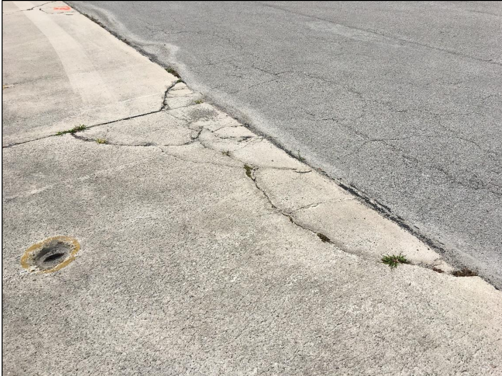
West Apron, Section 4107, Sample Unit 202 - High Severity (62) Corner Break, High Severity (65) Joint Seal Damage, (73) Shrinkage Cracking
