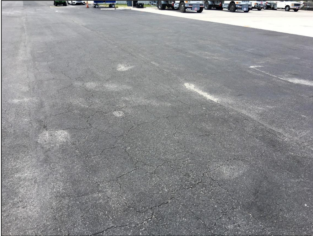
West Apron, Section 4120, Sample Unit 810 - Low Severity (43) Block Cracking, Low Severity (48) Longitudinal and Transverse Cracking, Low Severity (52) Raveling, Low Severity (57) Weathering
