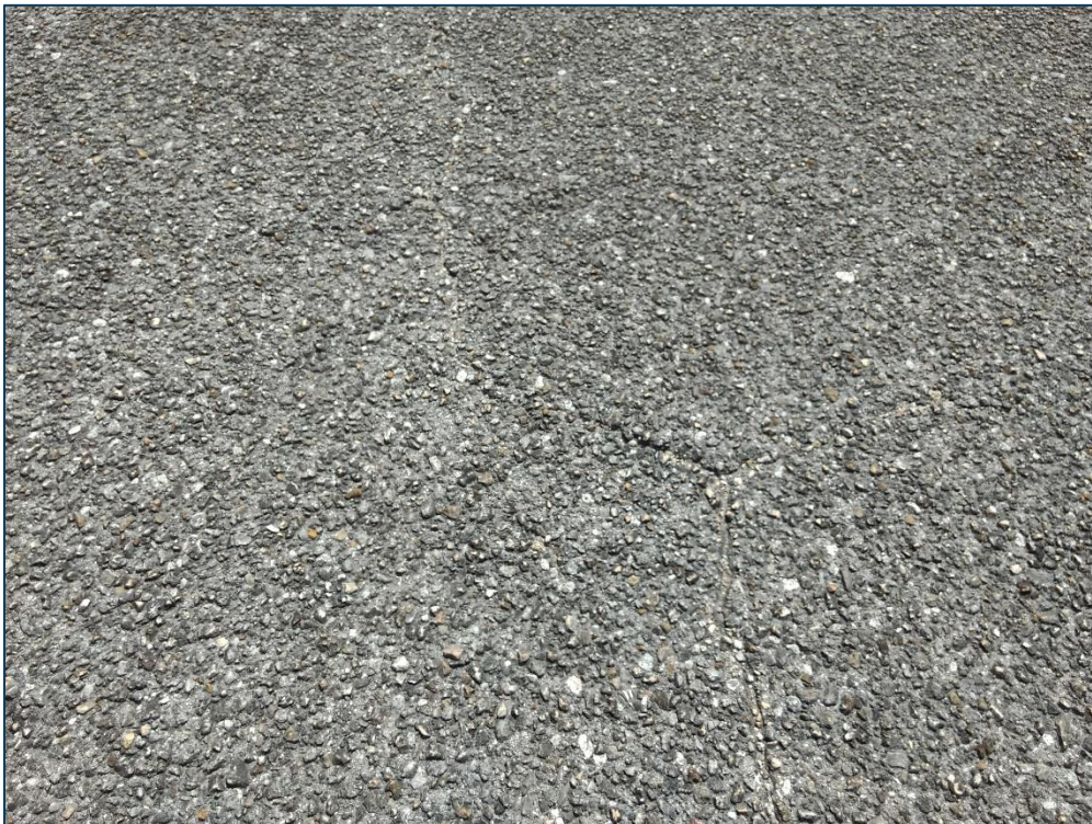
Taxiway A1, Section 120, Sample Unit 106 – Low Severity (48) Longitudinal and Transverse Cracking, Medium Severity (52) Raveling
