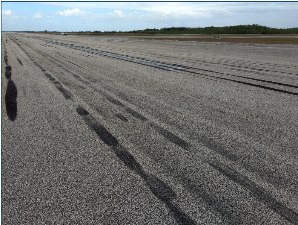
Runway 9-27, Section 6105, Sample Unit 385 – Low Severity (48) Longitudinal and Transverse Cracking, Low Severity (52) Raveling, Medium Severity (52) Raveling
