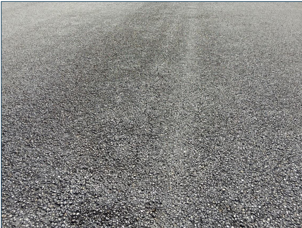
Taxiway B, Section 215, Sample Unit 105 – Low Severity (48) Longitudinal and Transverse Cracking, Low Severity (52) Raveling, Medium Severity (52) Raveling, Low Severity (56) Swelling
