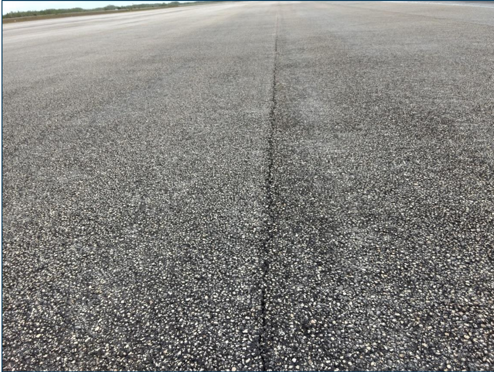
Runway 9-27, Section 6110, Sample Unit 580 – Low Severity (48) Longitudinal and Transverse Cracking, Low Severity (52) Raveling, Medium Severity (52) Raveling, Low Severity (56) Swelling
