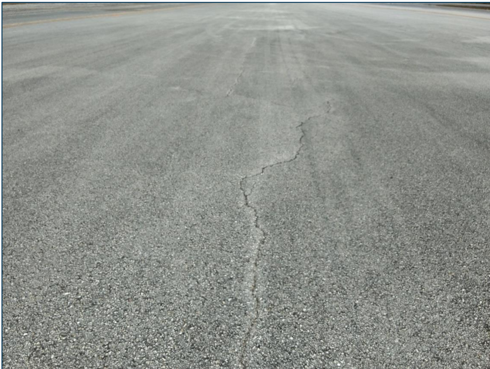
Taxiway A, Section 110, Sample Unit 106 – Low Severity (48) Longitudinal and Transverse Cracking, Low Severity (52) Raveling, Low Severity (56) Swelling
