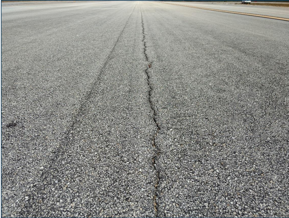
Taxiway A, Section 105, Sample Unit 123 – Low Severity (48) Longitudinal and Transverse Cracking, Low Severity (52) Raveling, Low Severity (56) Swelling
