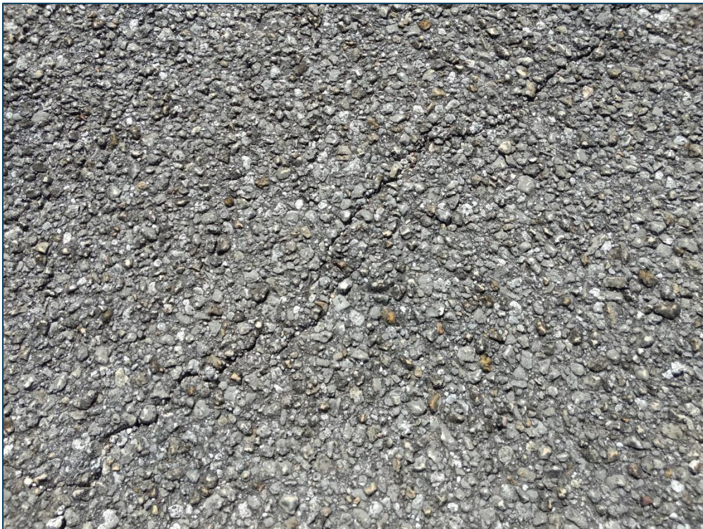
Apron North, Section 4105, Sample Unit 121 – Low Severity (48) Longitudinal and Transverse Cracking, Low Severity (52) Raveling, Medium Severity (52) Raveling
