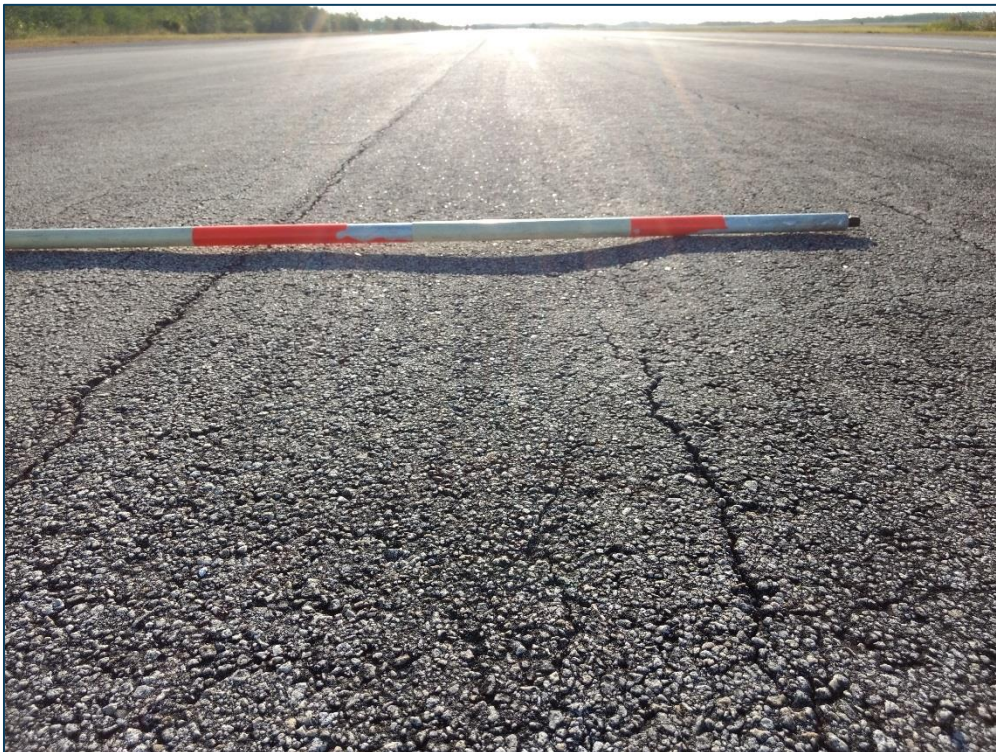
Taxiway A, Section 105, Sample Unit 237 – Low Severity (48) Longitudinal and Transverse Cracking, Low Severity (52) Raveling, Medium Severity (53) Rutting, Low Severity (56) Swelling, Low Severity (57) Weathering
