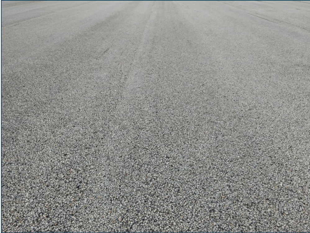
Runway 9-27, Section 6105, Sample Unit 344 – Low Severity (48) Longitudinal and Transverse Cracking, Low Severity (52) Raveling, Medium Severity (52) Raveling
