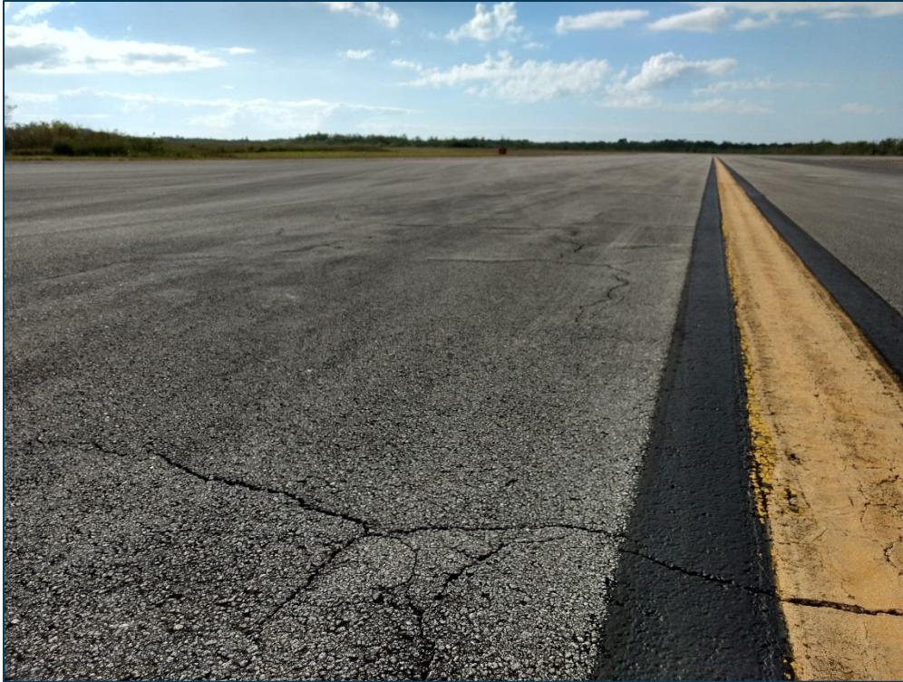
Taxiway A, Section 180, Sample Unit 111 – Low Severity (48) Longitudinal and Transverse Cracking, Low Severity (43) Block Cracking, Low Severity (52) Raveling, Low Severity (56) Swelling, Low Severity (57) Weathering
