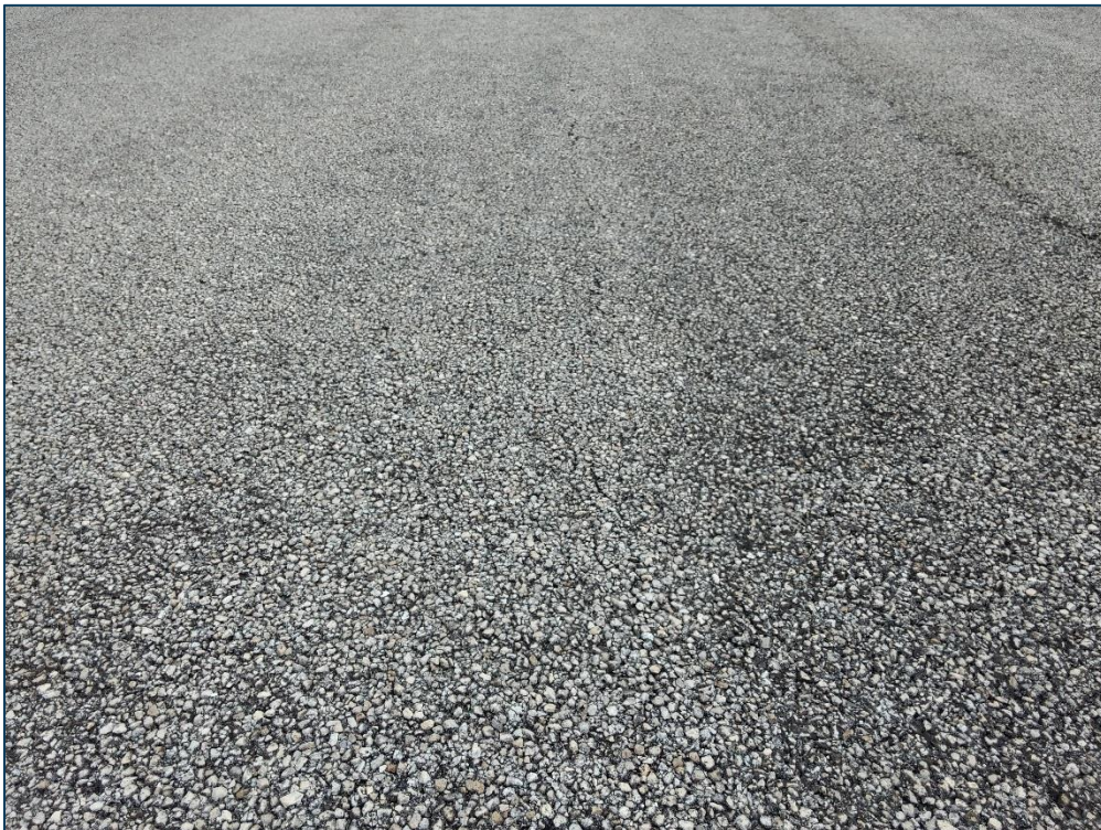
Runway 9-27, Section 6110, Sample Unit 126 – Low Severity (48) Longitudinal and Transverse Cracking, Low Severity (52) Raveling, Medium Severity (52) Raveling, Low Severity (56) Swelling
