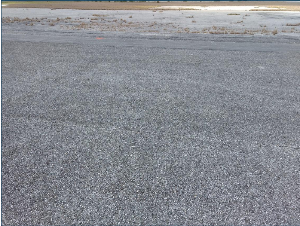
Apron North, Section 4105, Sample Unit 114 – Low Severity (48) Longitudinal and Transverse Cracking, Low Severity (52) Raveling, Medium Severity (52) Raveling
