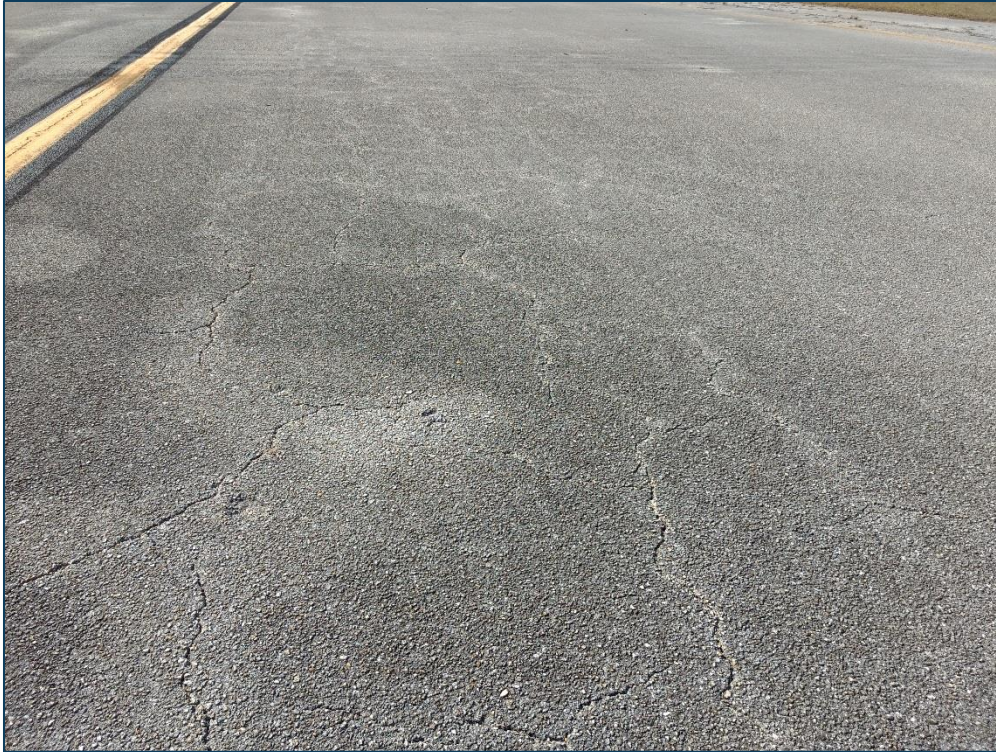
Taxiway A6, Section 170, Sample Unit 608 – Low Severity (43) Block Cracking, Low Severity (52) Raveling, Medium Severity (52) Raveling, Low Severity (56) Swelling
