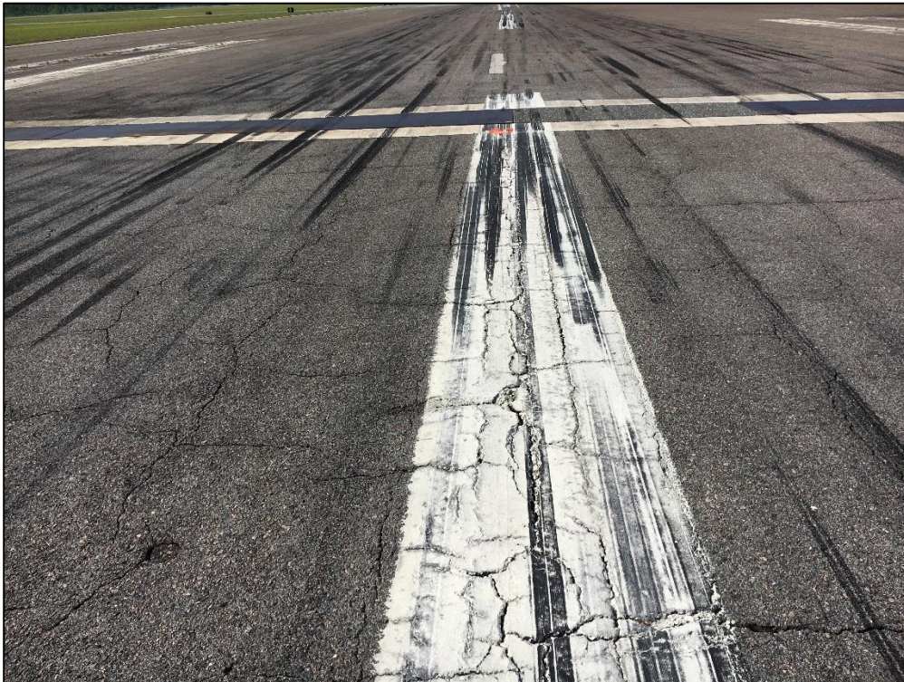
Runway 18R-36L, Section 6115, Sample Unit 216 - Low Severity (41) Alligator Cracking, Medium Severity (43) Block Cracking, Medium Severity (52) Raveling, Low Severity (56) Swelling
