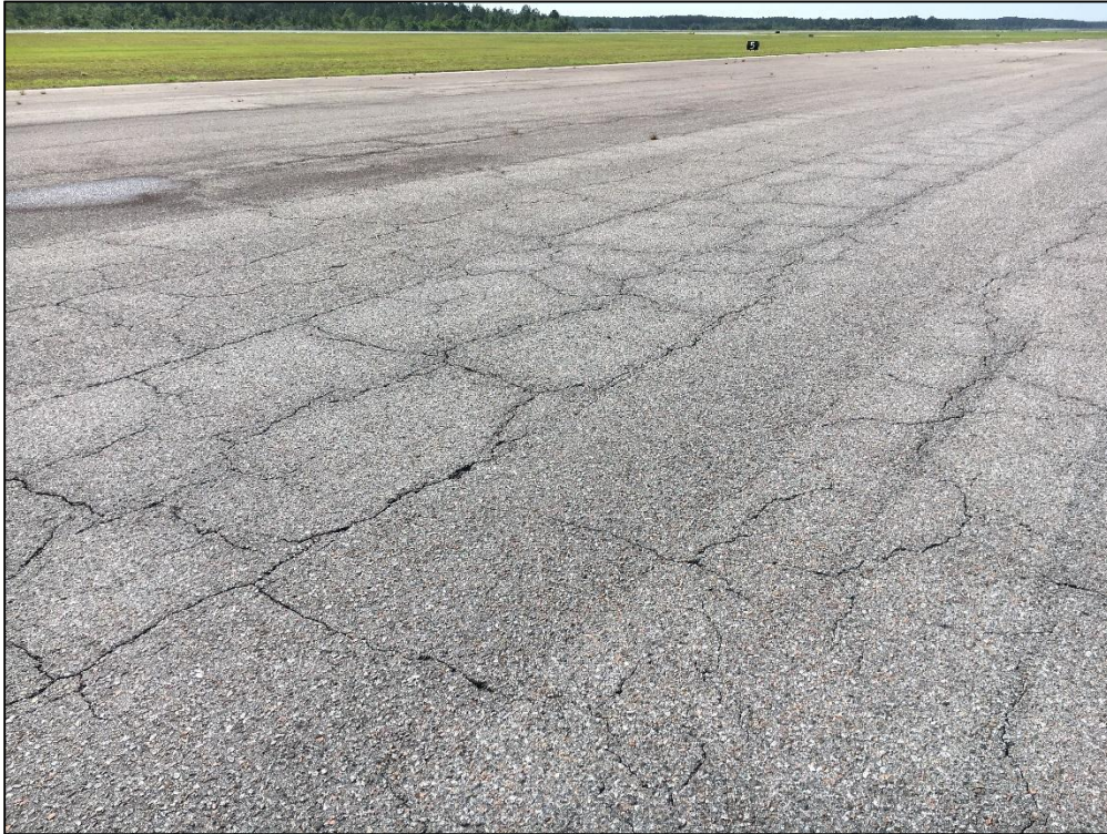
Runway 18R-36L, Section 6115, Sample Unit 229 - Medium Severity (43) Block Cracking, Low Severity (45) Depression, Medium Severity (52) Raveling, Low Severity (53) Rutting, Low Severity (56) Swelling
