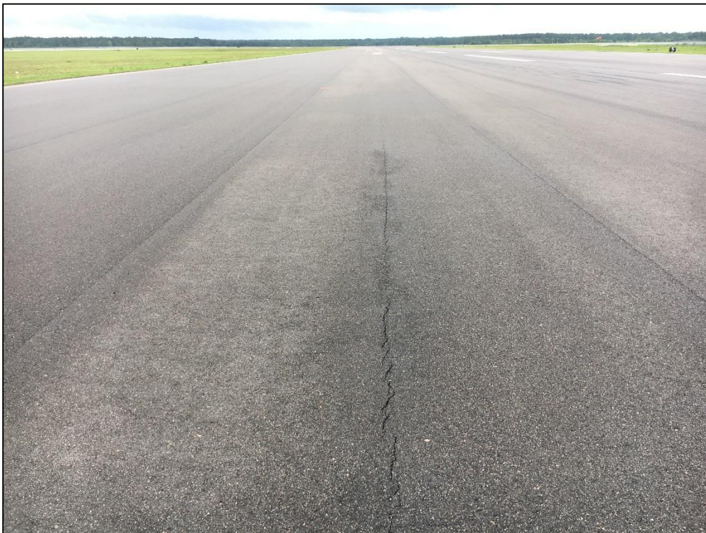
Runway 9R-27L, Section 6315, Sample Unit 328 - Low Severity (48) Longitudinal and Transverse Cracking, Low Severity (57) Weathering
