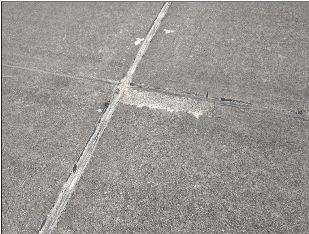
Runway 9L-27R, Section 6410, Sample Unit 105 - Medium Severity (65) Joint Seal Damage, Medium Severity (66) Small Patch, Low Severity (71) Faulting
