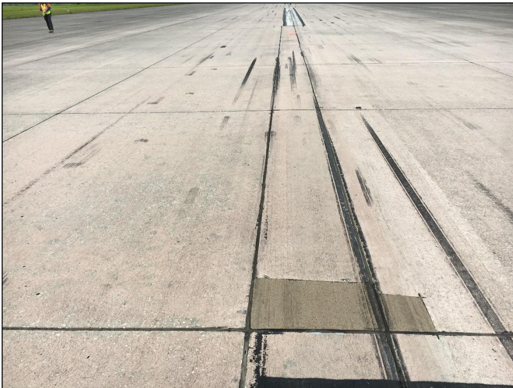
Runway 18L-36R, Section 6235, Sample Unit 388 - Low Severity (66) Small Patch
