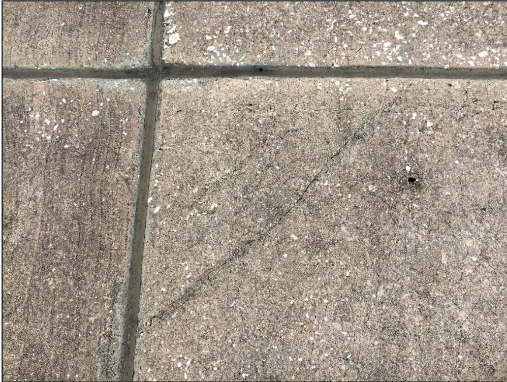
Runway 18L-36R, Section 6235, Sample Unit 425 - Low Severity (62) Corner Break, (73) Shrinkage Cracking
