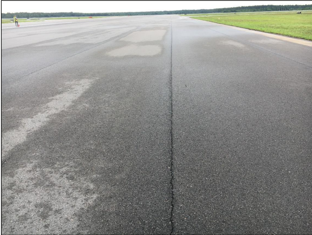
Runway 9R-27L, Section 6320, Sample Unit 741 - Low Severity (48) Longitudinal and Transverse Cracking, Low Severity (57) Weathering
