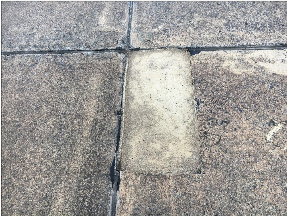
Taxiway B, Section 205, Sample Unit 148 - Low Severity (66) Small Patch, (73) Shrinkage Cracking
