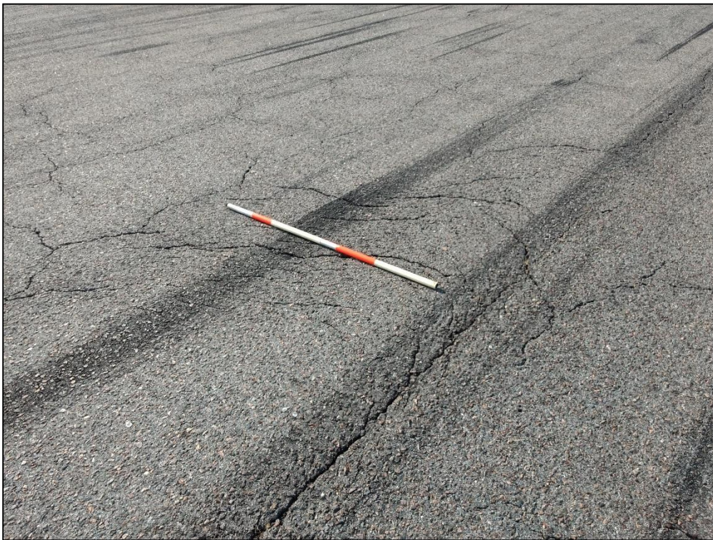
Runway 18R-36L, Section 6115, Sample Unit 313 - Medium Severity (43) Block Cracking, Medium Severity (52) Raveling, (55) Slippage Cracking
