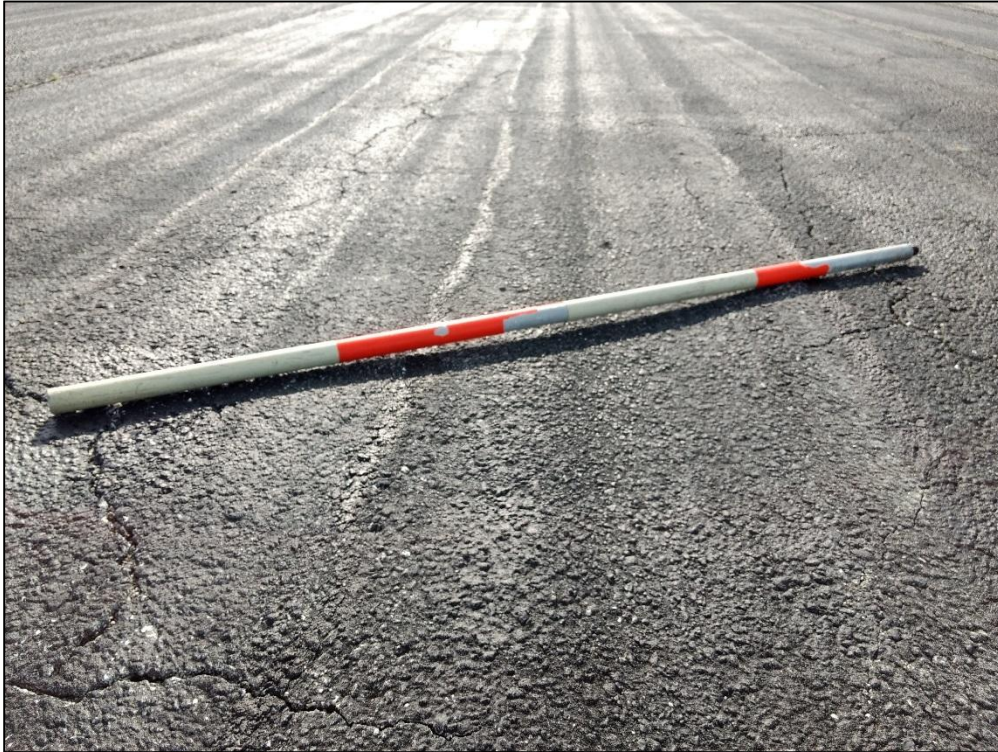
Runway 9L-27R, Section 6420, Sample Unit 709 – Low Severity (43) Block Cracking, Medium Severity (52) Raveling, Low Severity (56) Swelling
