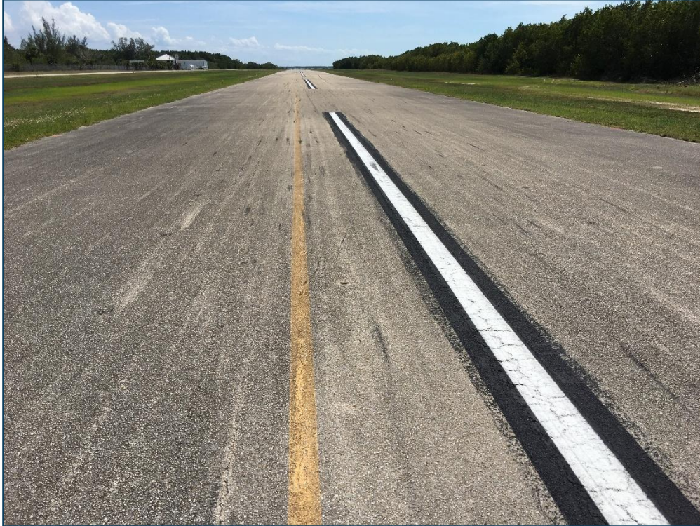
Runway 15-33, Section 6105, Sample Unit 101 – Low Severity (43) Block Cracking, Low Severity (48) Longitudinal and Transverse Cracking, Low Severity (52) Raveling, Medium Severity (52) Raveling
