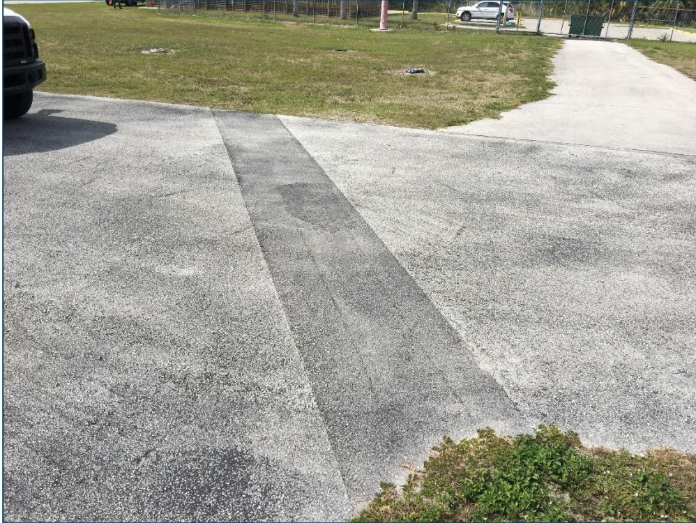
Apron, Section 4110, Sample Unit 100 – Low Severity (48) Longitudinal and Transverse Cracking, Low Severity (50) Patching, Low Severity (52) Raveling, Low Severity (57) Weathering
