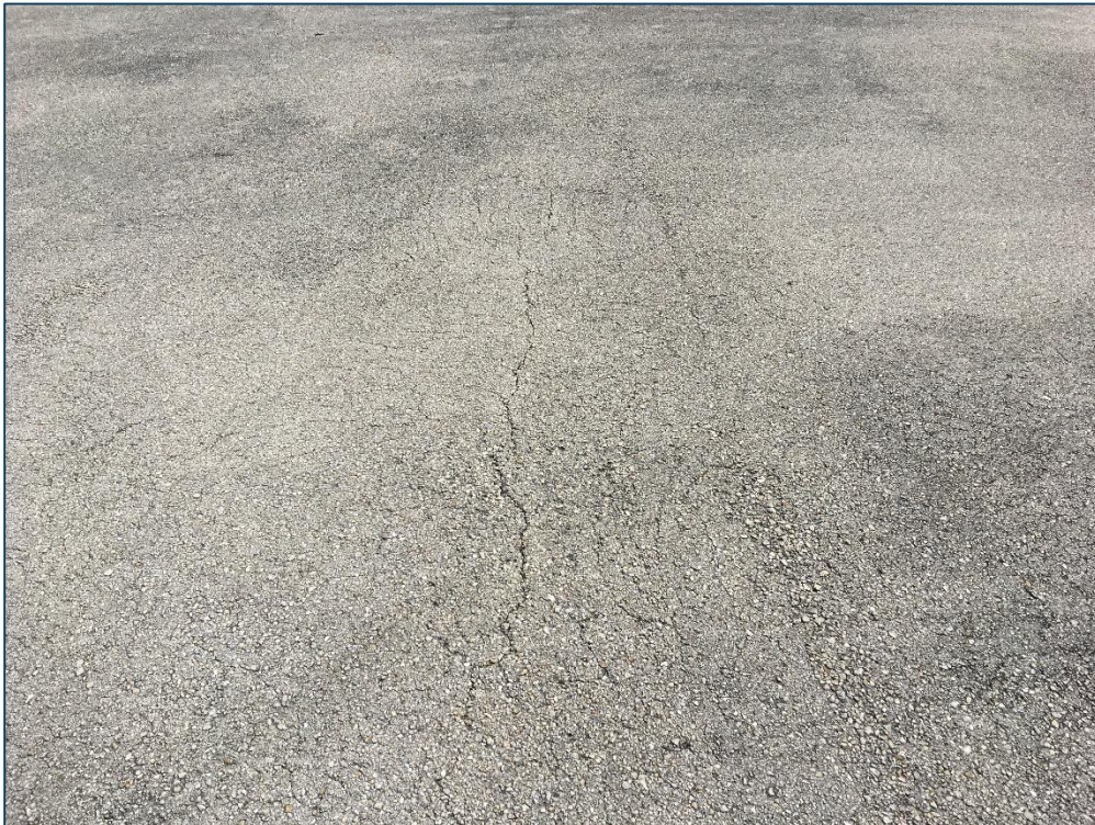
Run Up Apron RW33, Section 4120, Sample Unit 100 – Low Severity (48) Longitudinal and Transverse Cracking, Low Severity (52) Raveling, Low Severity (57) Weathering
