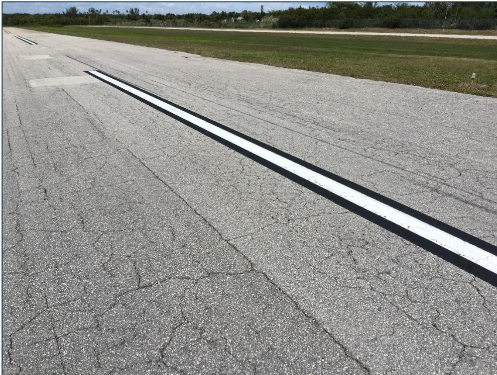
Runway 15-33, Section 6110, Sample Unit 109 – Low Severity (43) Block Cracking, Medium Severity (43) Block Cracking, Low Severity (50) Patching, Low Severity (52) Raveling, Medium Severity (52) Raveling
