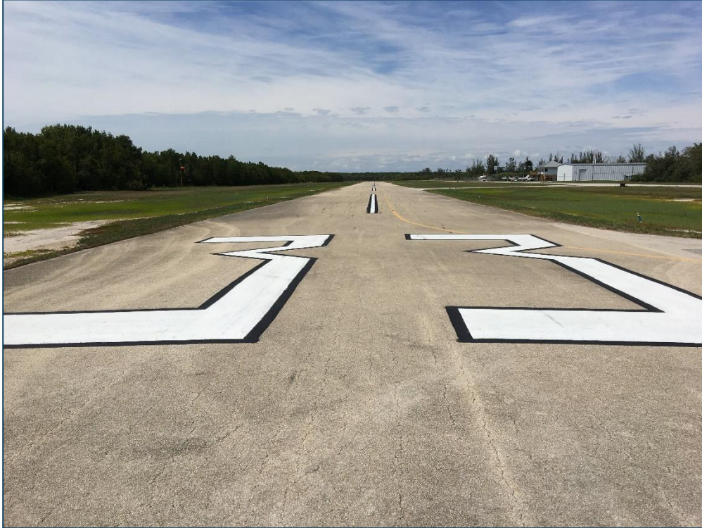
Runway 15-33, Section 6115, Sample Unit 122 – Low Severity (43) Block Cracking, Low Severity (48) Longitudinal and Transverse Cracking, Low Severity (52) Raveling, Medium Severity (52) Raveling
