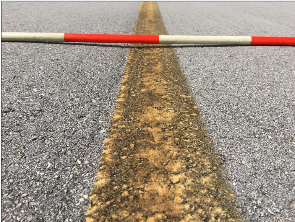
Taxiway A, Section 130, Sample Unit 103 – Low Severity (45) Depression, Low Severity (57) Weathering
