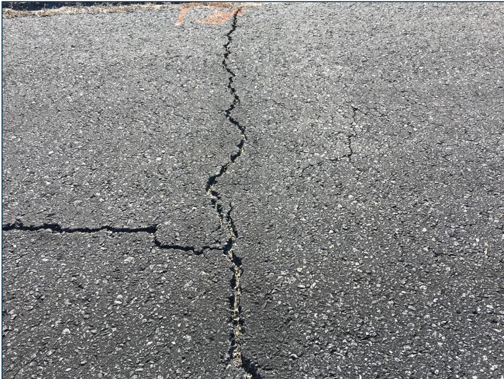
Runway 6-24, Section 6105, Sample Unit 106 – Low and Medium Severity (48) Longitudinal and Transverse Cracking, Low Severity (57) Weathering, Low Severity (52) Raveling
