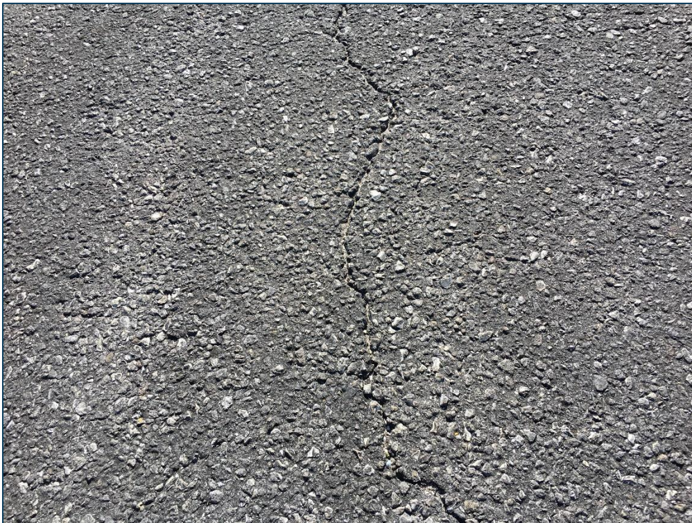
Apron, Section 4105, Sample Unit 100 – Low Severity (48) Longitudinal and Transverse Cracking, Low Severity (52) Raveling, Low Severity (57) Weathering
