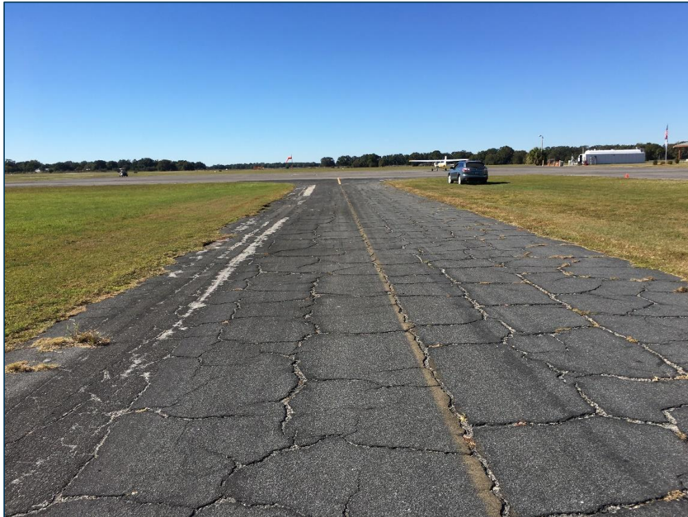
Hangar Taxiway, Section 210, Sample Unit 101 – Medium Severity (43) Block Cracking, High Severity (43) Block Cracking, Low Severity (52) Raveling, Medium Severity (52) Raveling
