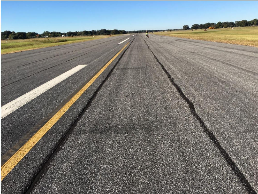
Runway 6-24, Section 6105, Sample Unit 134 – Low Severity (48) Longitudinal and Transverse Cracking, Low Severity (52) Raveling, Low Severity (57) Weathering
