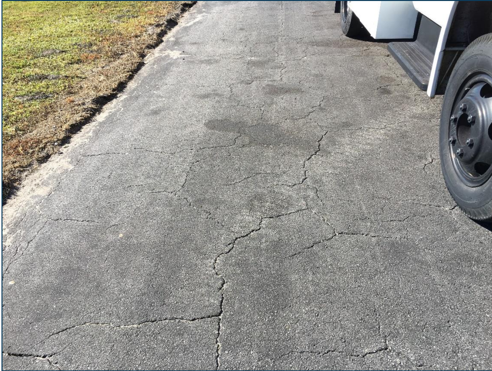
Apron, Section 4110, Sample Unit 401 – Low Severity (43) Block Cracking, Low Severity (57) Weathering
