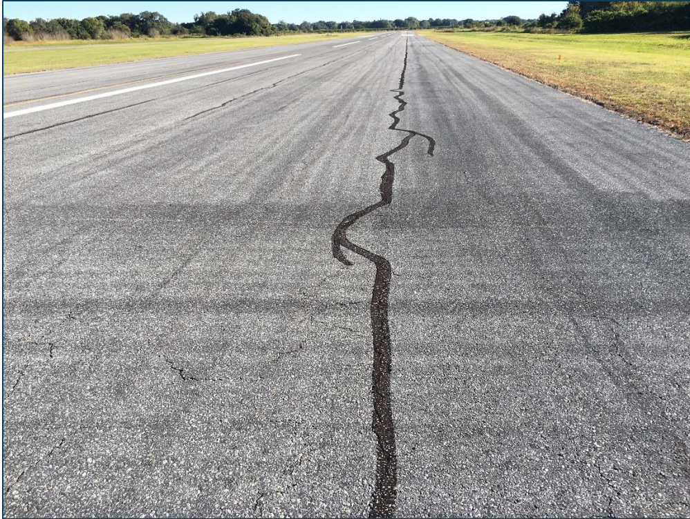
Runway 6-24, Section 6105, Sample Unit 137 – Low Severity (48) Longitudinal and Transverse Cracking, Low Severity (52) Raveling, Low Severity (57) Weathering
