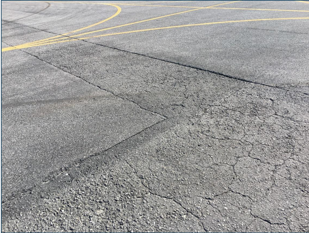
Taxiway, Section 115, Sample Unit 300 – Low Severity (48) Longitudinal and Transverse Cracking, Medium Severity (50) Patching, Low Severity (52) Raveling, Low Severity (57) Weathering
