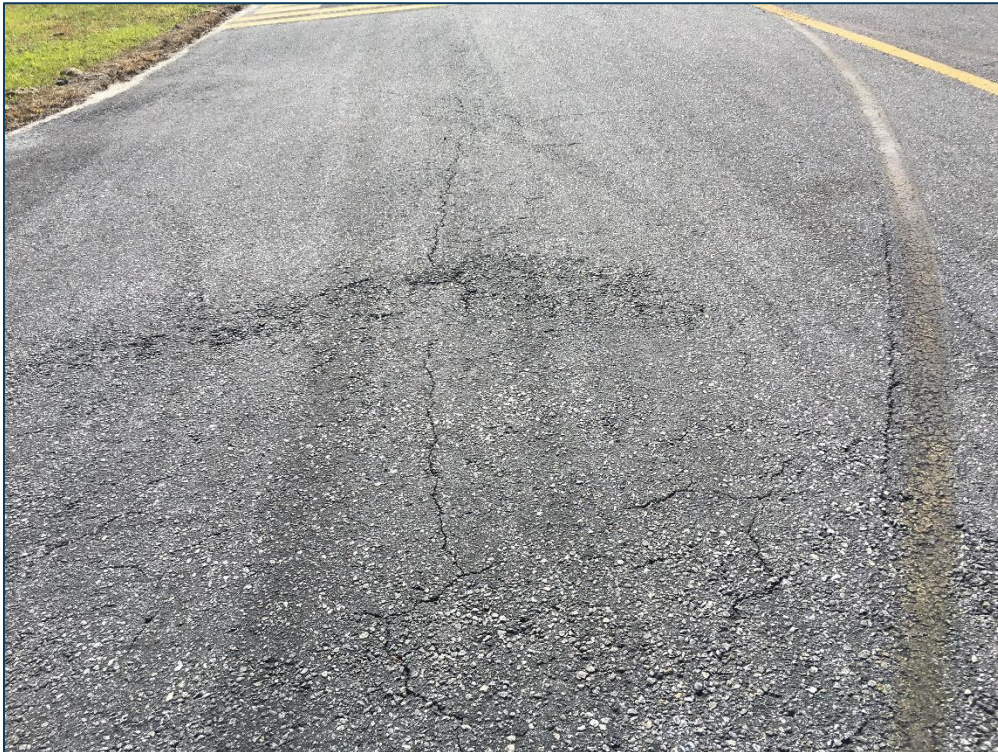
Taxiway, Section 110, Sample Unit 201 – Low Severity (48) Longitudinal and Transverse Cracking, Low Severity (52) Raveling, Low Severity (57) Weathering
