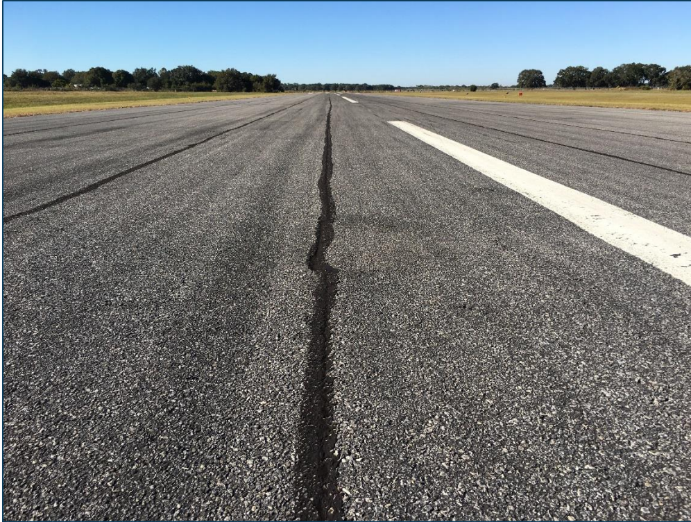
Runway 6-24, Section 6105, Sample Unit 118 – Low Severity (45) Depression, Low Severity (48) Longitudinal and Transverse Cracking, Low Severity (52) Raveling, Low Severity (57) Weathering
