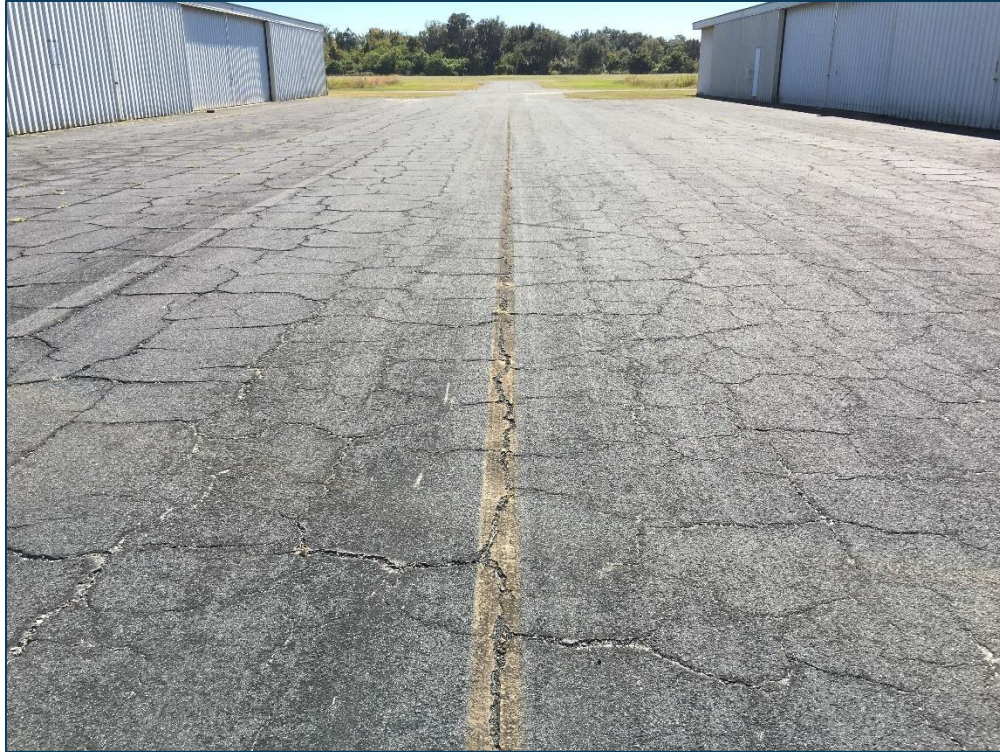
Hangar Taxiway, Section 230, Sample Unit 101 – Medium Severity (43) Block Cracking, High Severity (43) Block Cracking, Low Severity (52) Raveling, Medium Severity (52) Raveling
