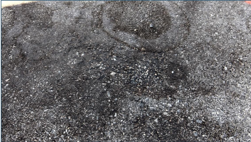
Apron, Section 4205, Sample Unit 602 – (49) Oil Spillage
