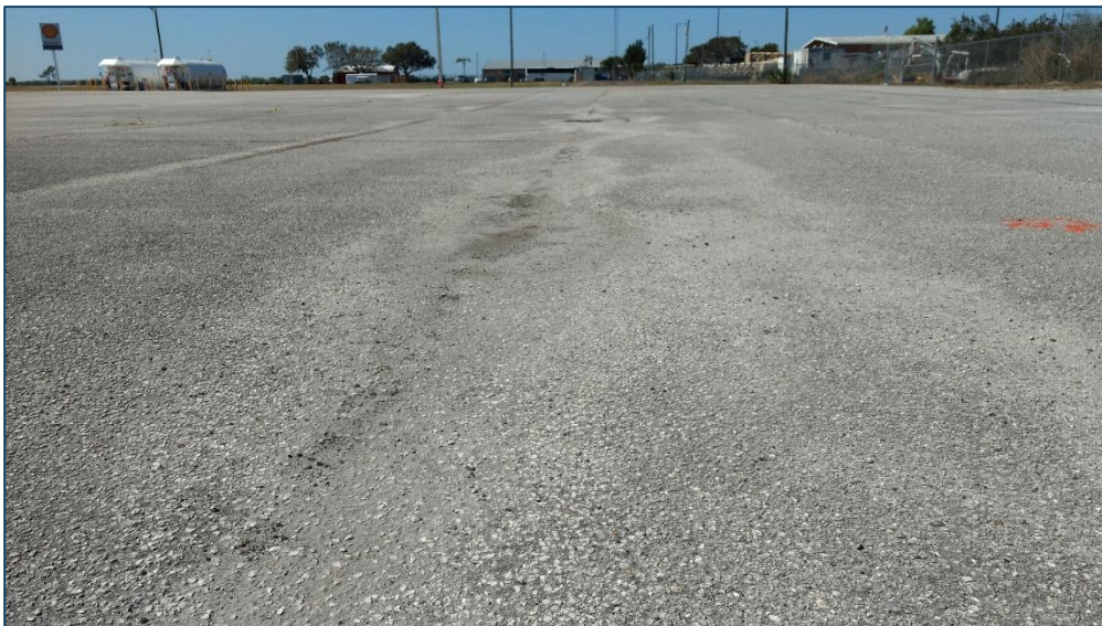
Apron, Section 4105, Sample Unit 105 – Low Severity (45) Depression, Low Severity (48) Longitudinal and Transverse Cracking, Low Severity (52) Raveling, Medium Severity (52) Raveling
