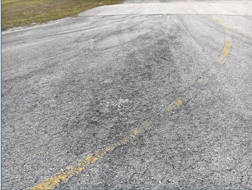
Apron, Section 4110, Sample Unit 301 – Low Severity (41) Alligator Cracking Low Severity (48) Longitudinal and Transverse Cracking, Low Severity (50) Patching, Low Severity (52) Raveling, Medium Severity (52) Raveling, High Severity (52) Raveling
