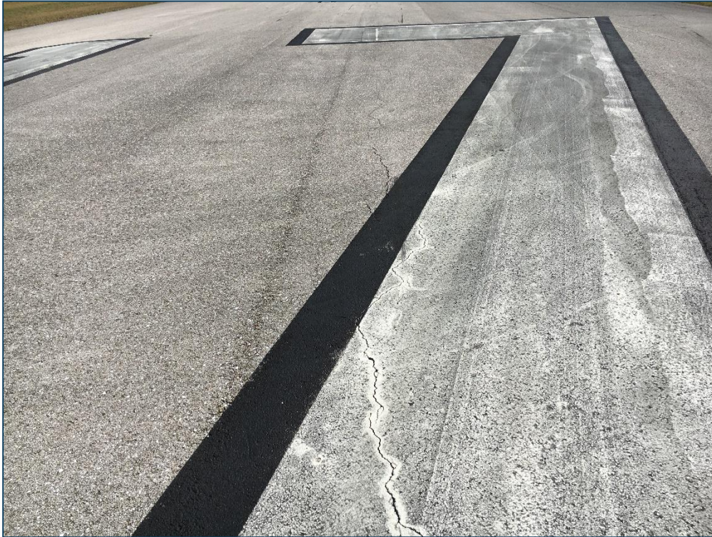
Runway 17-35, Section 6205, Sample Unit 179 – Low and Medium Severity (48) Longitudinal and Transverse Cracking, Low Severity (52) Raveling, Medium Severity (52) Raveling
