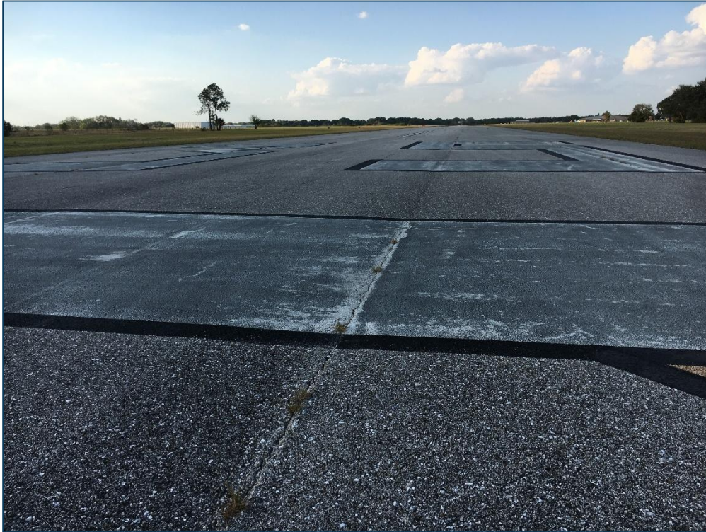
Runway 17-35, Section 6205, Sample Unit 103 – Low and Medium Severity (48) Longitudinal and Transverse Cracking, Low Severity (52) Raveling
