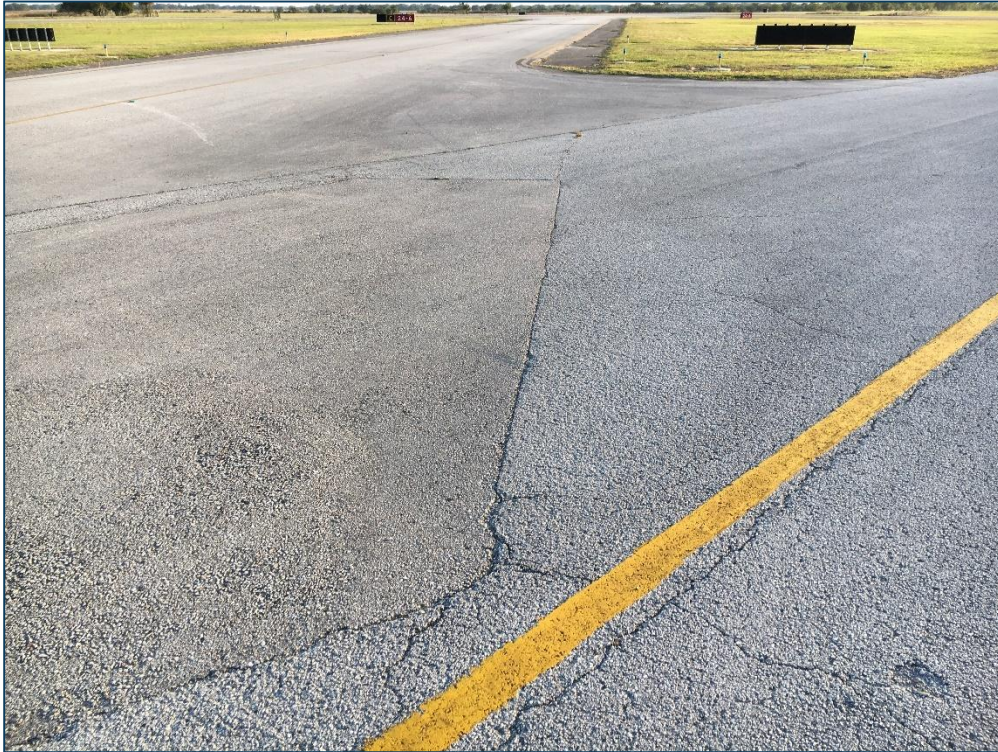
Taxiway A, Section 105, Sample Unit 118 – Low Severity (43) Block Cracking, Low Severity (48) Longitudinal and Transverse Cracking, Low Severity (50) Patching, Low Severity (52) Raveling, Medium Severity (52) Raveling
