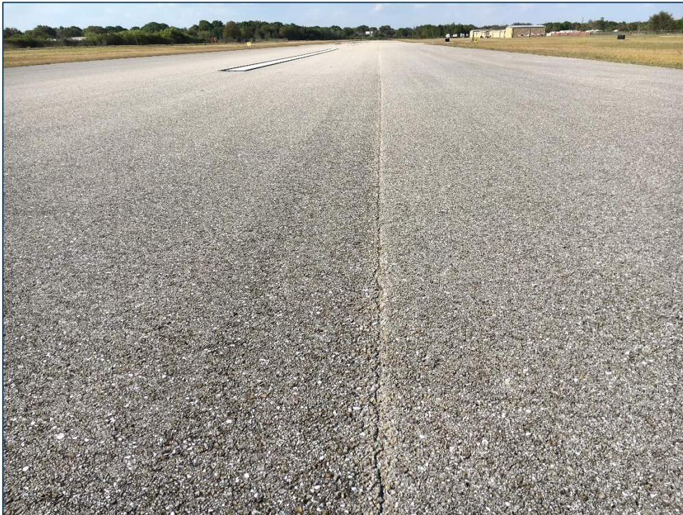
Runway 17-35, Section 6205, Sample Unit 142 – Low and Medium Severity (48) Longitudinal and Transverse Cracking, Low Severity (52) Raveling, Medium Severity (52) Raveling
