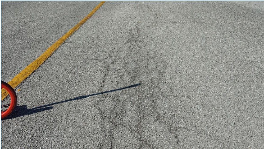
Taxiway A, Section 105, Sample Unit 104 – Low Severity (41) Alligator Cracking, Low and Medium Severity (48) Longitudinal and Transverse Cracking, Low Severity (52) Raveling, Medium Severity (52) Raveling
