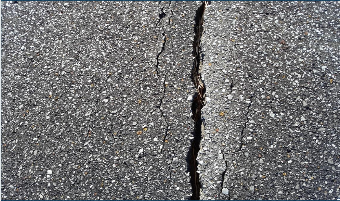
Runway 5-23, Section 6105, Sample Unit 115 – Low and Medium Severity (48) Longitudinal and Transverse Cracking, Low Severity (56) Swelling, Low Severity (52) Raveling
