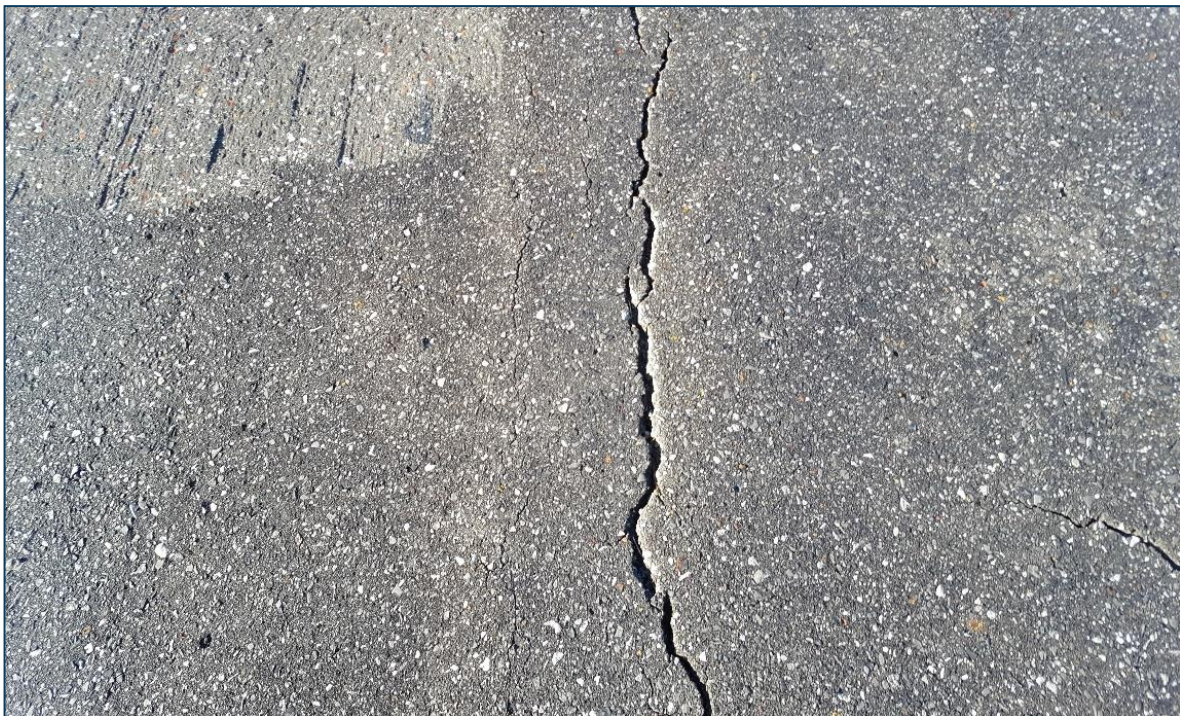
Runway 5-23, Section 6105, Sample Unit 100 – Low and Medium Severity (48) Longitudinal and Transverse Cracking, Low Severity (52) Raveling, Medium Severity (52) Raveling, Low Severity (56) Swelling
