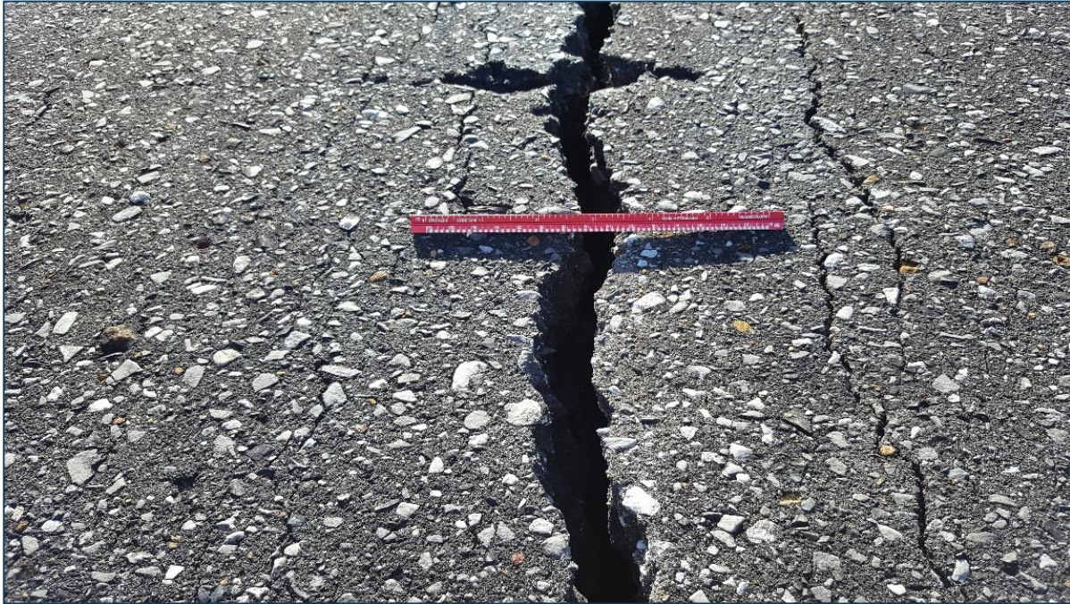
Runway 5-23, Section 6105, Sample Unit 105 – Low and Medium Severity (48) Longitudinal and Transverse Cracking, Low Severity (52) Raveling
