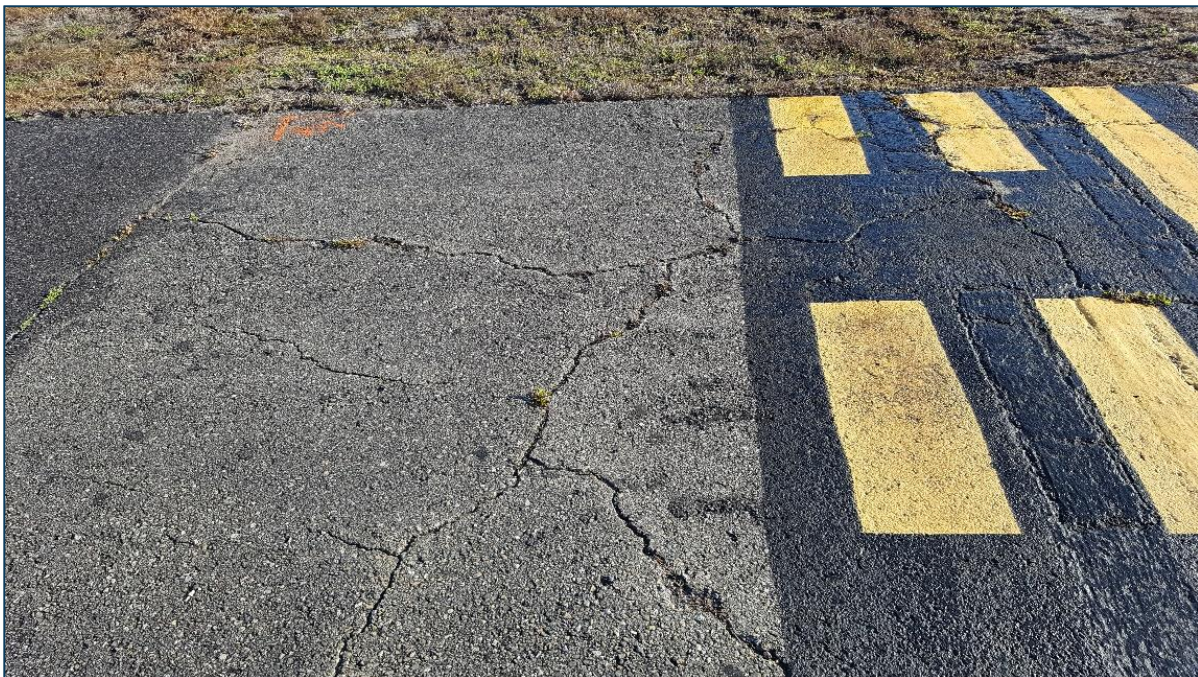
Taxiway A, Section 105, Sample Unit 101 – Low Severity (43) Block Cracking, Low and Medium Severity (48) Longitudinal and Transverse Cracking, Low Severity (52) Raveling, Low Severity (57) Weathering
