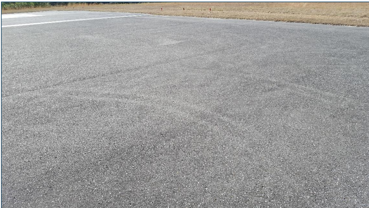
Apron AP RU, Section 5105, Sample Unit 100 – Low Severity (45) Depression, Low Severity (48) Longitudinal and Transverse Cracking, Low Severity (52) Raveling, Medium Severity (52) Raveling
