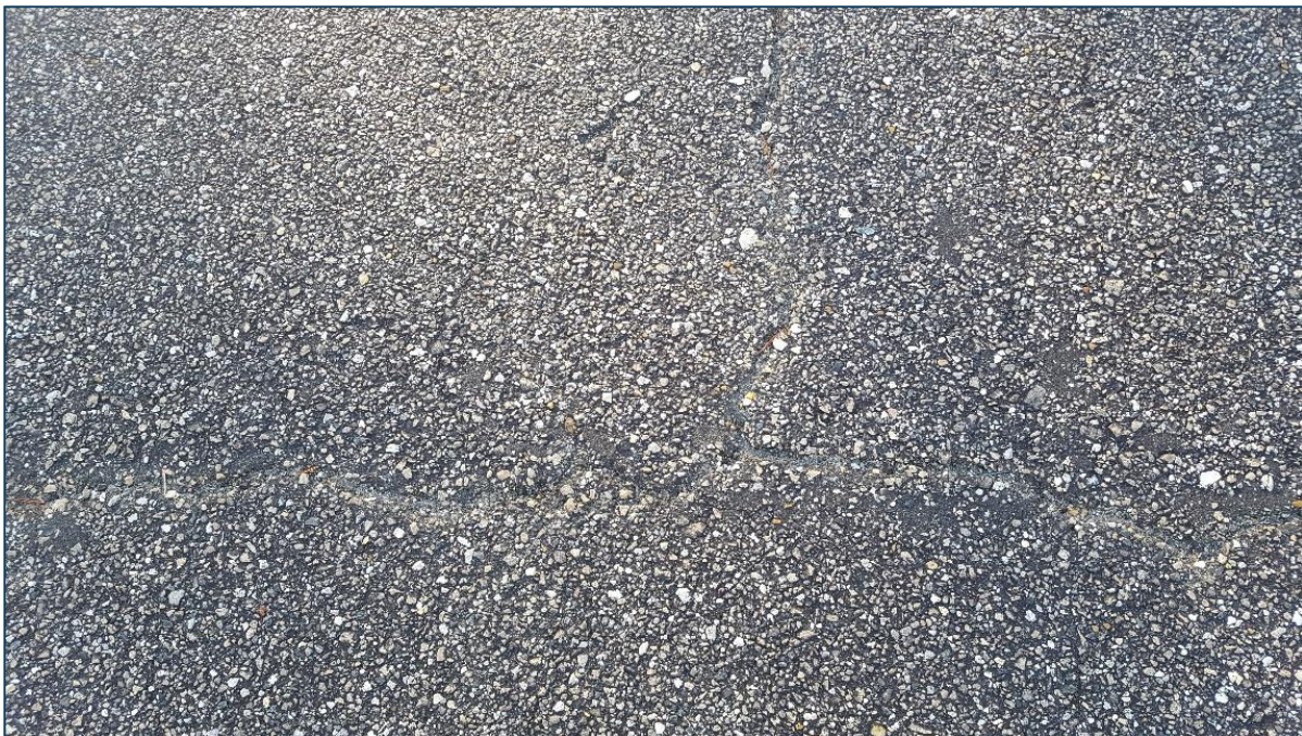
Apron AP, Section 4120, Sample Unit 501 – Low and Medium Severity (48) Longitudinal and Transverse Cracking, Low Severity (52) Raveling, Medium Severity (52) Raveling
