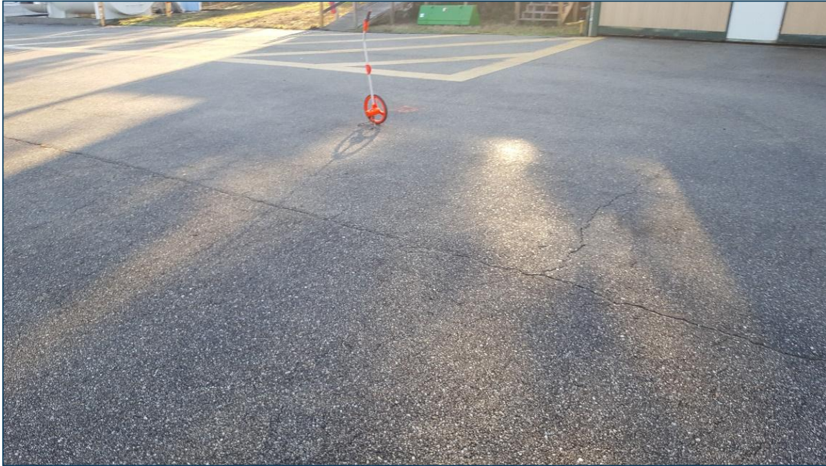
Apron AP, Section 4120, Sample Unit 501 – Low and Medium Severity (48) Longitudinal and Transverse Cracking, Low Severity (52) Raveling
