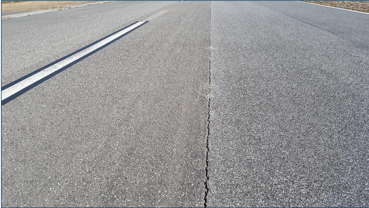
Runway 5-23, Section 6105, Sample Unit 145 – Low and Medium Severity (48) Longitudinal and Transverse Cracking, Low Severity (52) Raveling, Medium Severity (52) Raveling
