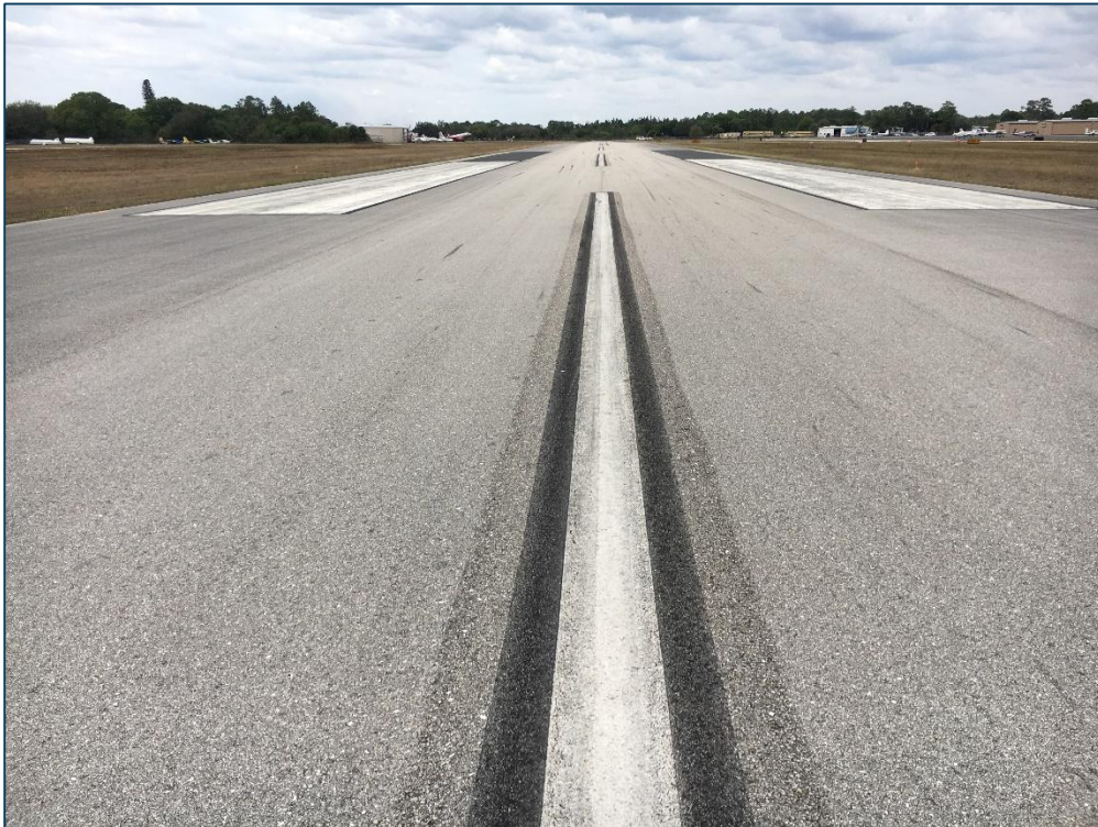
Runway 14-32, Section 6105, Sample Unit 124 – Low Severity (48) Longitudinal and Transverse Cracking, Low Severity (52) Raveling, Low Severity (57) Weathering
