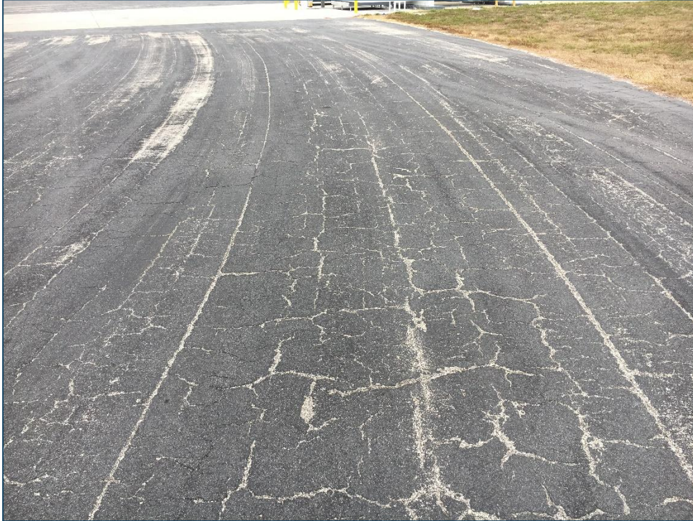
Taxiway SE to NR, Section 705, Sample Unit 202 – Medium Severity (43) Block Cracking, Low Severity (57) Weathering
