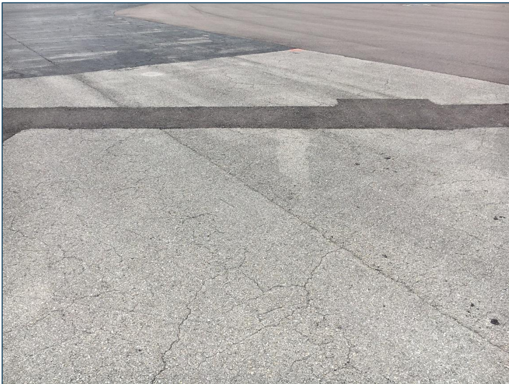
North Apron, Section 4135, Sample Unit 600 - Low Severity (43) Block Cracking, Low Severity (45) Depression, Low Severity (50) Patching, Medium Severity (52) Raveling
