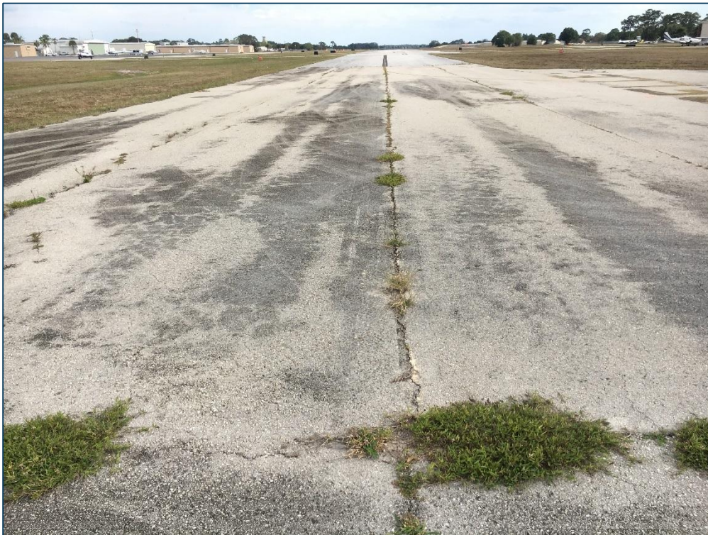
Taxiway to Runway, Section 905, Sample Unit 100 - Medium Severity (48) Longitudinal and Transverse Cracking, Low Severity (52) Raveling, Medium Severity (52) Raveling
