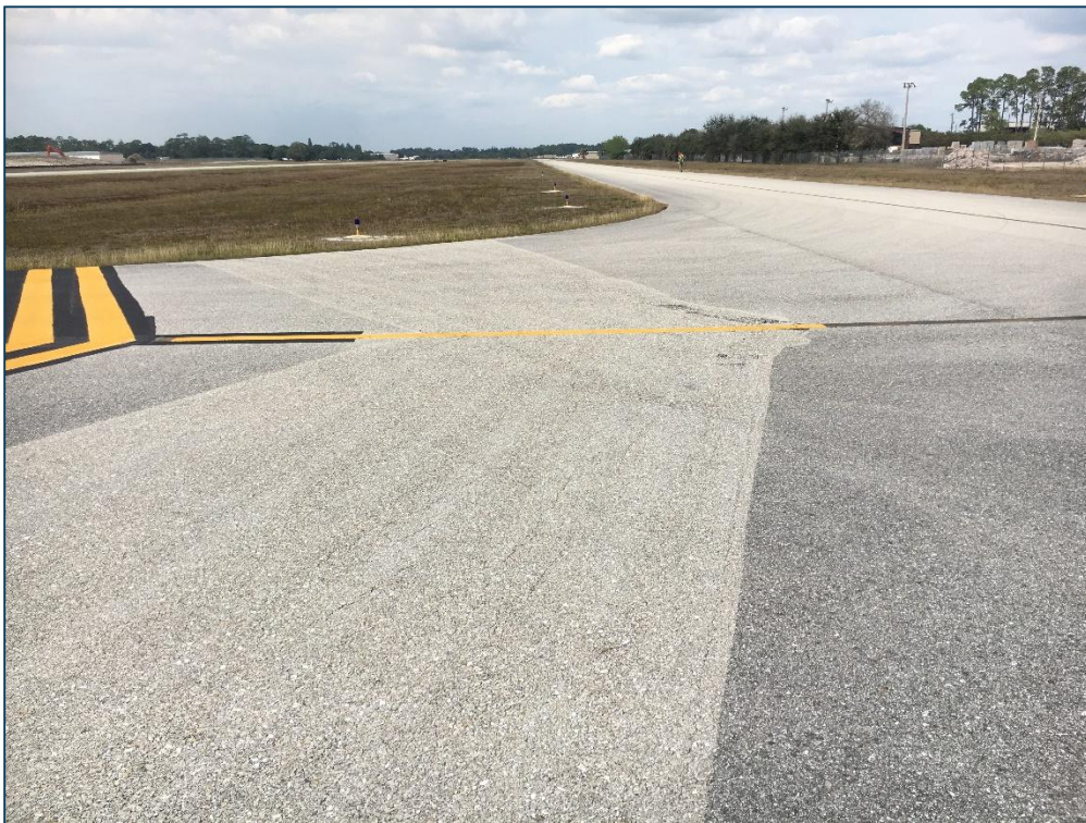
Taxiway A4, Section 115, Sample Unit 101 – Low Severity (48) Longitudinal and Transverse Cracking, Low Severity (52) Raveling, Low Severity (57) Weathering.
