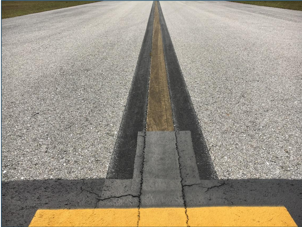
Taxiway A2, Section 205, Sample Unit 101 – Low Severity (48) Longitudinal and Transverse Cracking, Low Severity (52) Raveling, Low Severity (57) Weathering
