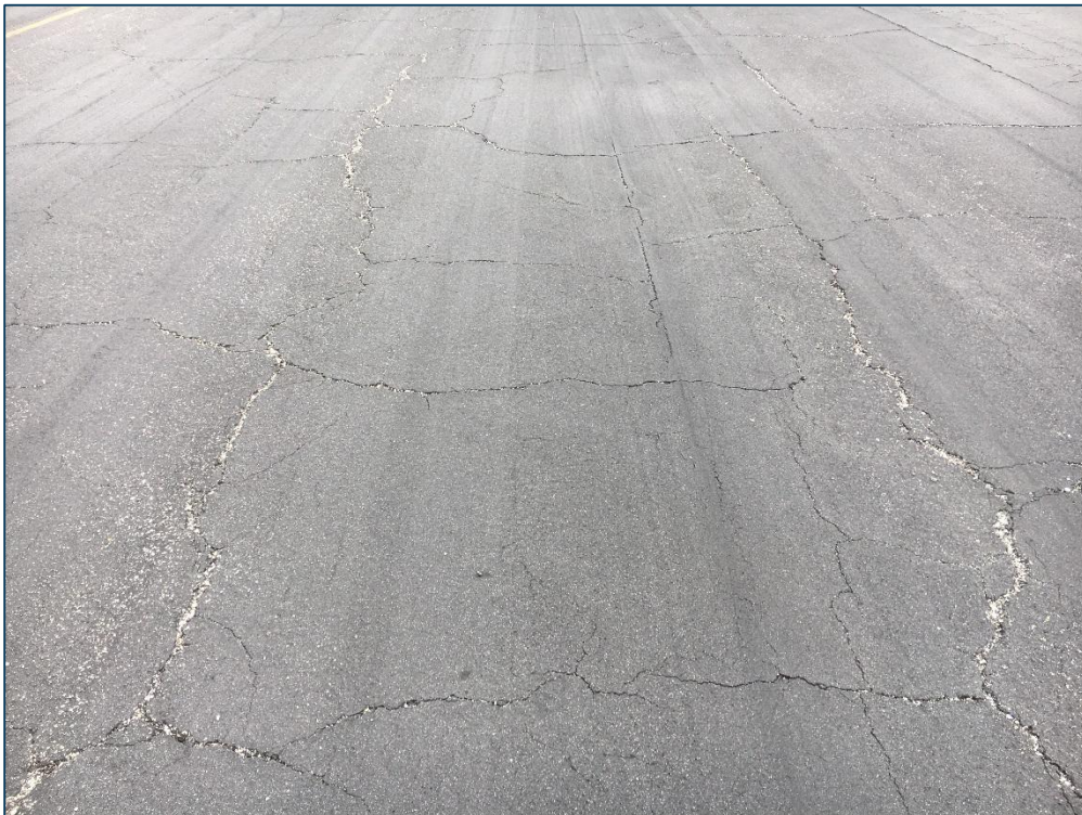
North Apron, Section 4110, Sample Unit 503 - Low Severity (43) Block Cracking, Medium Severity (43) Block Cracking, Low Severity (52) Raveling
