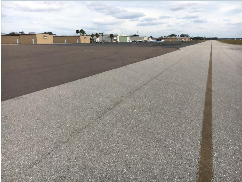
Taxiway A, Section 405, Sample Unit 101 – Low Severity (48) Longitudinal and Transverse Cracking, Low Severity (57) Weathering
