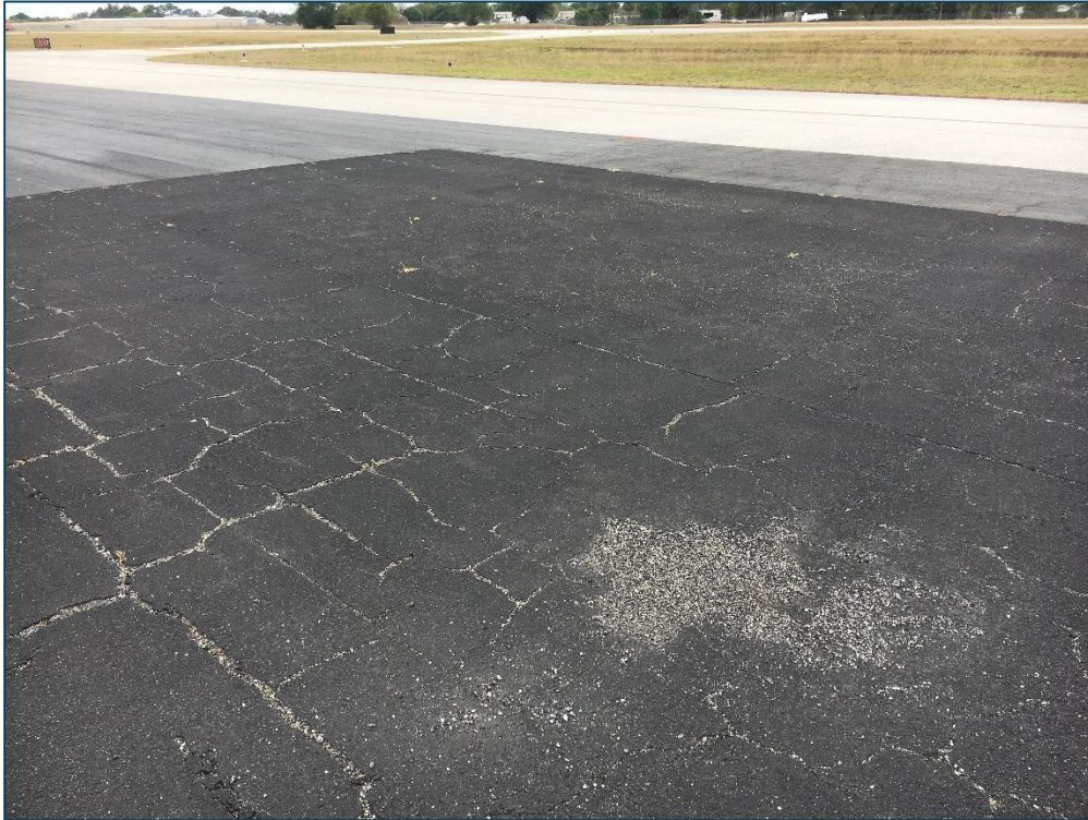
North Apron, Section 4110, Sample Unit 202 - Low Severity (43) Block Cracking, Medium Severity (43) Block Cracking, Low Severity (45) Depression, Low Severity (52) Raveling
