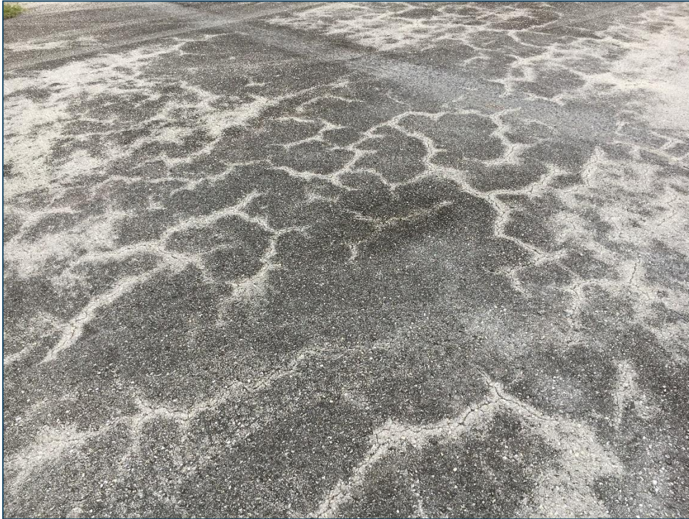
Taxiway to Runway, Section 905, Sample Unit 100 - Low Severity (43) Block Cracking, Low Severity (52) Raveling, Medium Severity (52) Raveling
