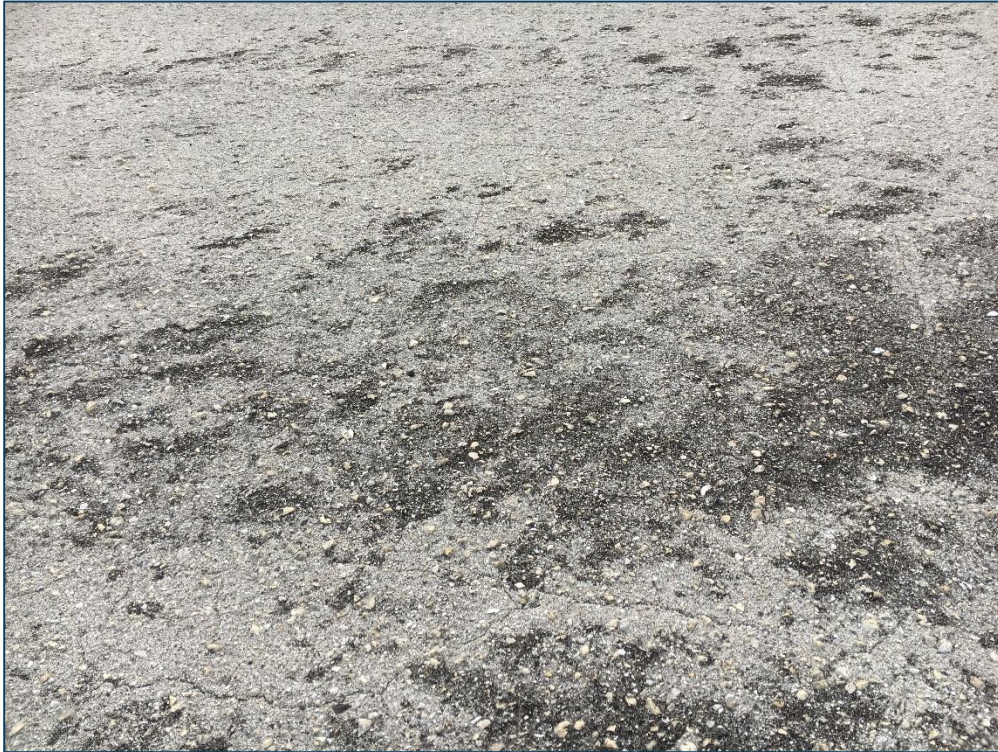
Northwest Apron, Section 4160, Sample Unit 105 - Medium Severity (52) Raveling
