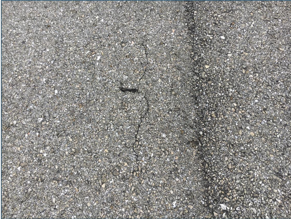
Runway 14-32, Section 6105, Sample Unit 114 – Low Severity (48) Longitudinal and Transverse Cracking, Low Severity (52) Raveling, Low Severity (57) Weathering
