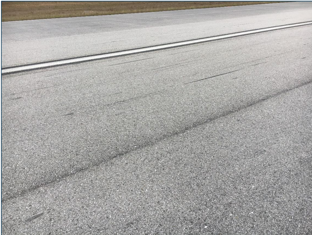
Runway 14-32, Section 6105, Sample Unit 119 – Low Severity (48) Longitudinal and Transverse Cracking, Low Severity (52) Raveling, Low Severity (57) Weathering
