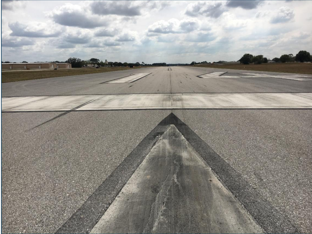
Runway 14-32, Section 6105, Sample Unit 108 – Low Severity (48) Longitudinal and Transverse Cracking Low Severity (57) Weathering
