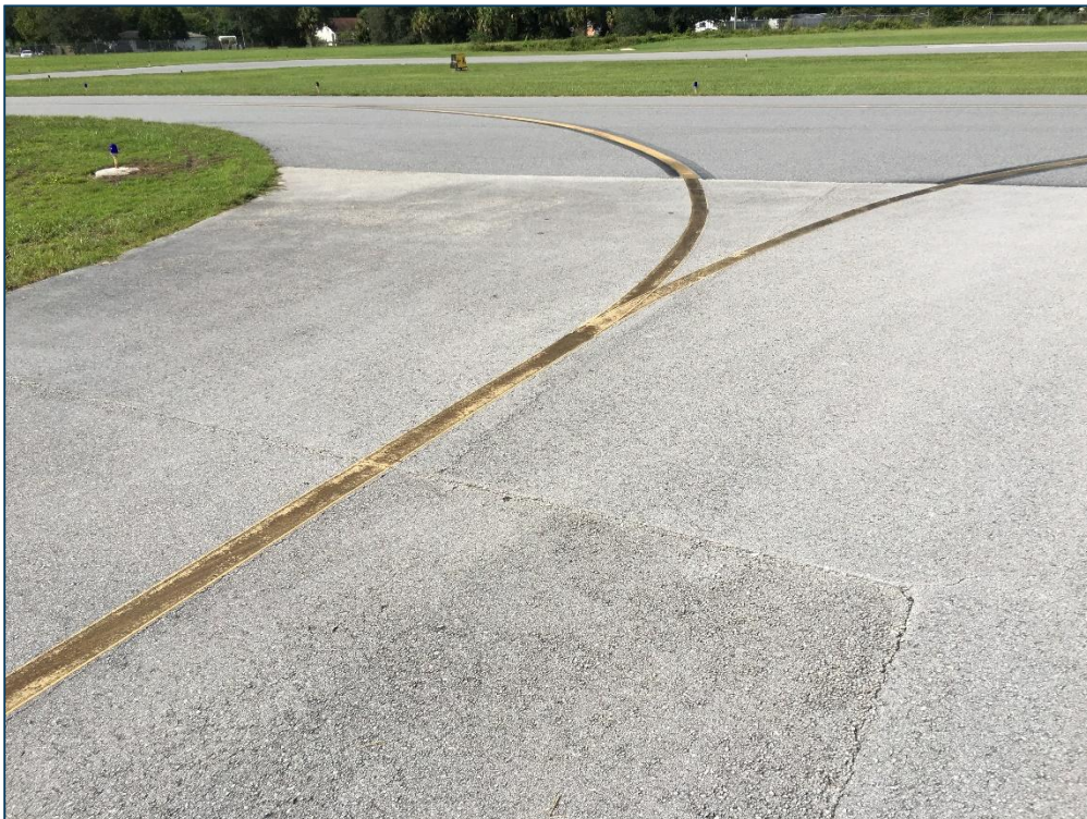
Taxiway AP, Section 115, Sample Unit 115 – Low Severity (48) Longitudinal and Transverse Cracking, Low Severity (57) Weathering, Medium Severity (57) Weathering
