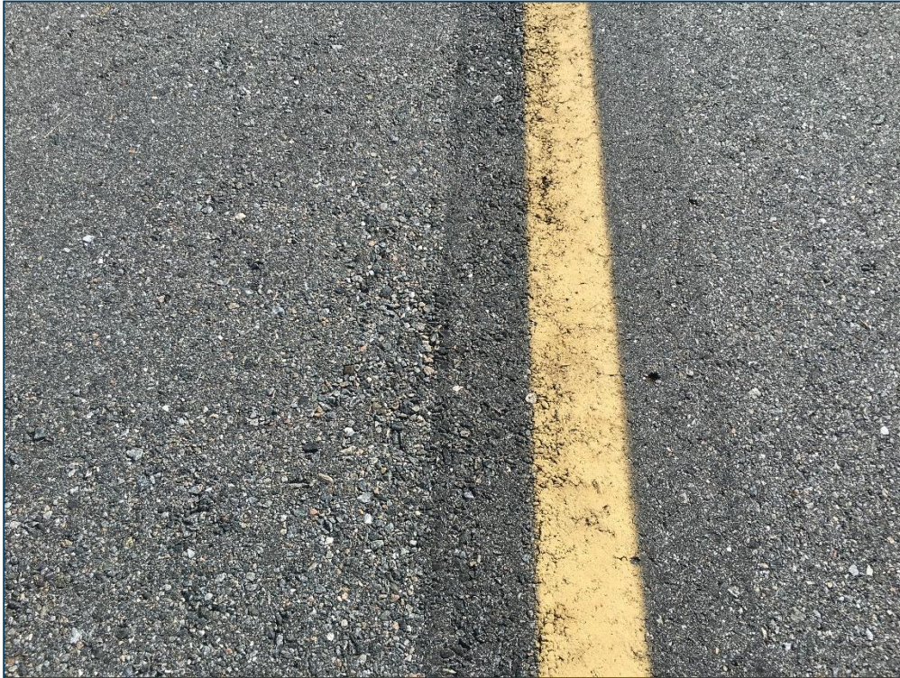
Taxiway D, Section 405, Sample Unit 100 – Low Severity (57) Weathering, Low Severity (52) Raveling, Low Severity (48) Longitudinal and Transverse Cracking
