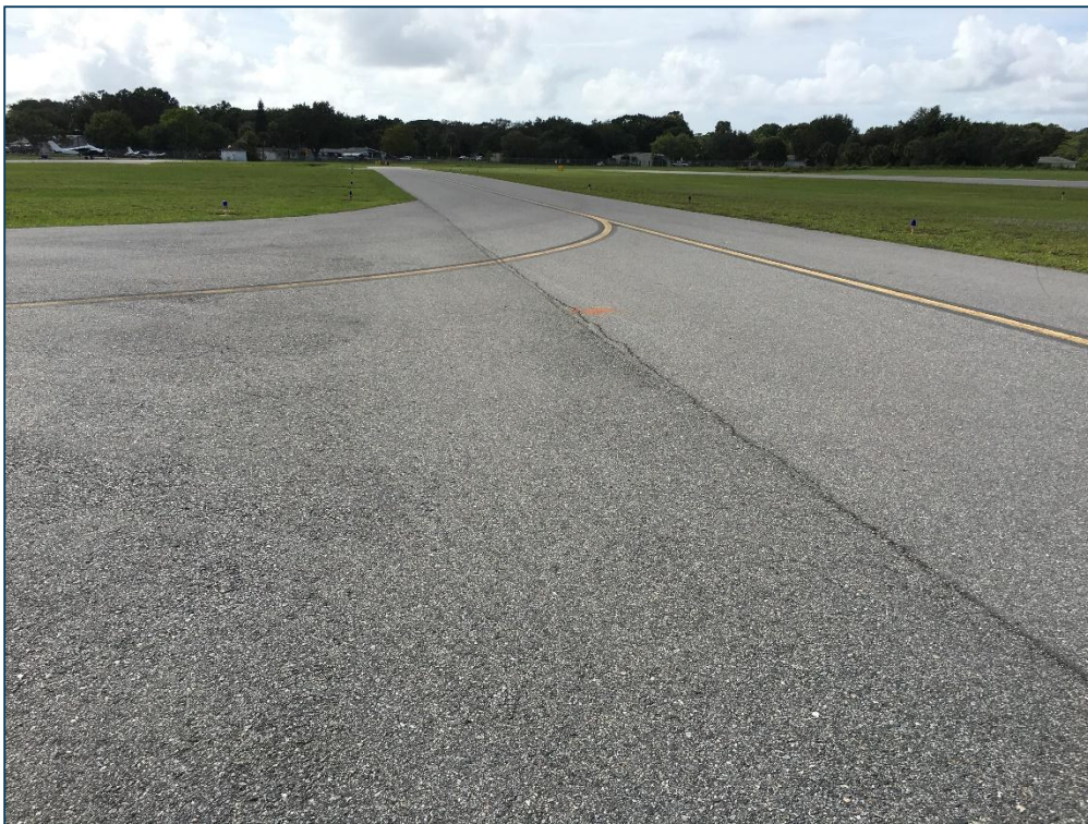
Taxiway B, Section 210, Sample Unit 100 – Low Severity (48) Longitudinal and Transverse Cracking, Low Severity (57) Weathering, Low Severity (52) Raveling
