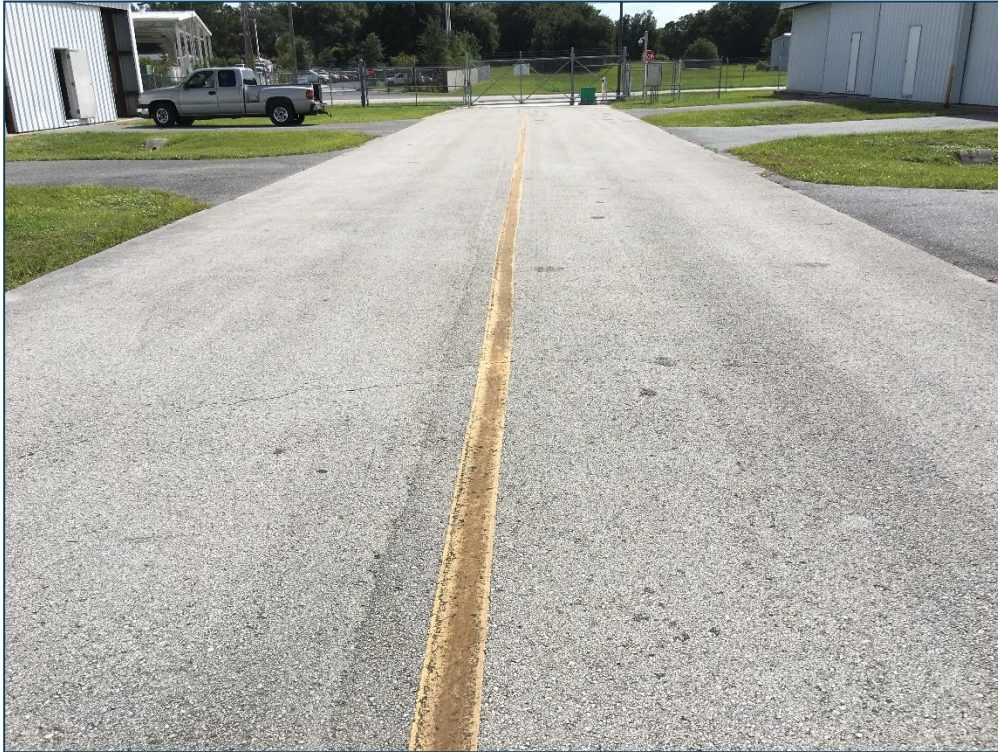
Taxiway C, Section 320, Sample Unit 104 – Low Severity (48) Longitudinal and Transverse Cracking, Low Severity (57) Weathering, Low Severity (52) Raveling
