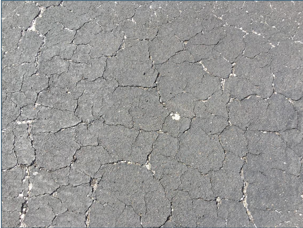
Apron AP, Section 4107, Sample Unit 203 – Low Severity (43) Block Cracking, Low Severity (52) Raveling
