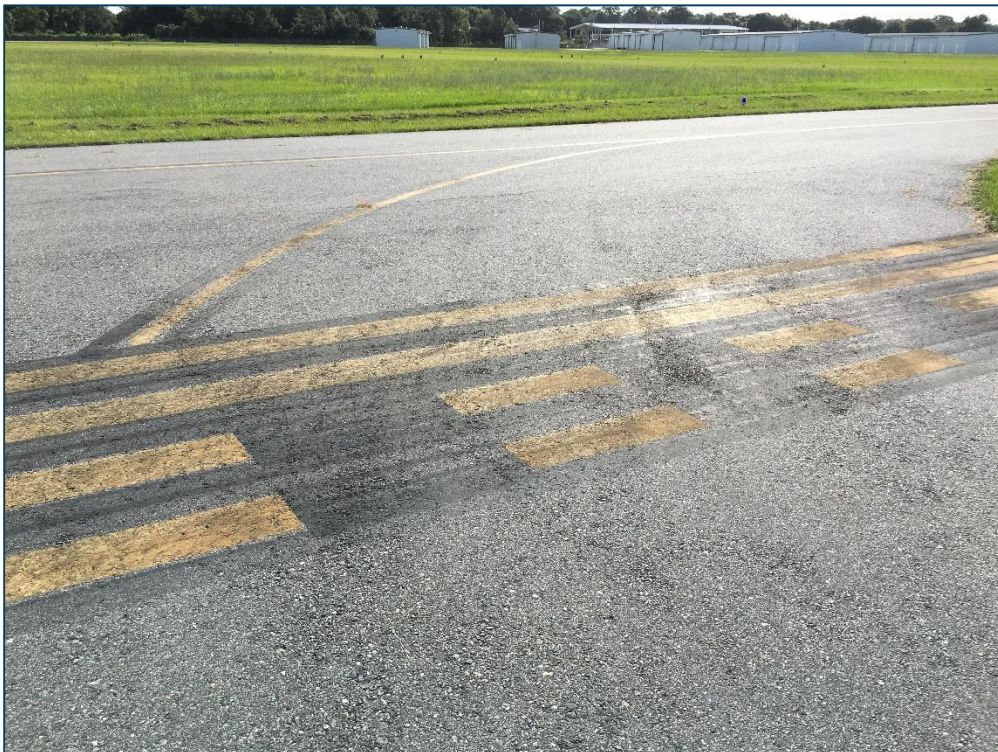
Taxiway D, Section 405, Sample Unit 100 – Low Severity (57) Weathering, Low Severity (52) Raveling
