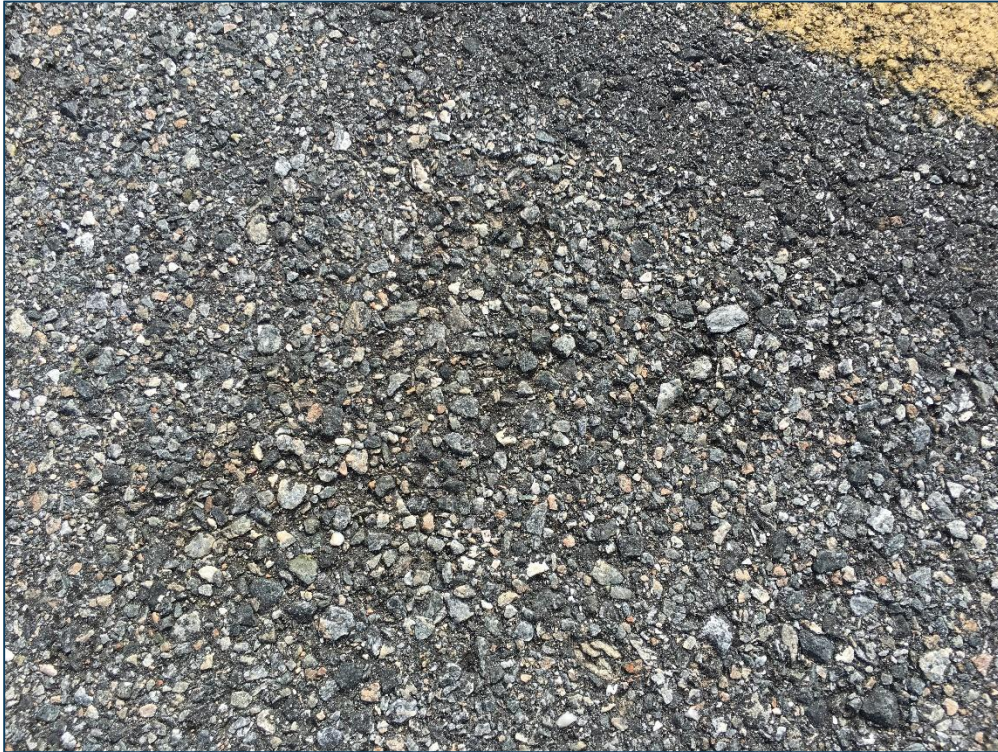
Taxiway B, Section 210, Sample Unit 100 – Low Severity (52) Raveling
