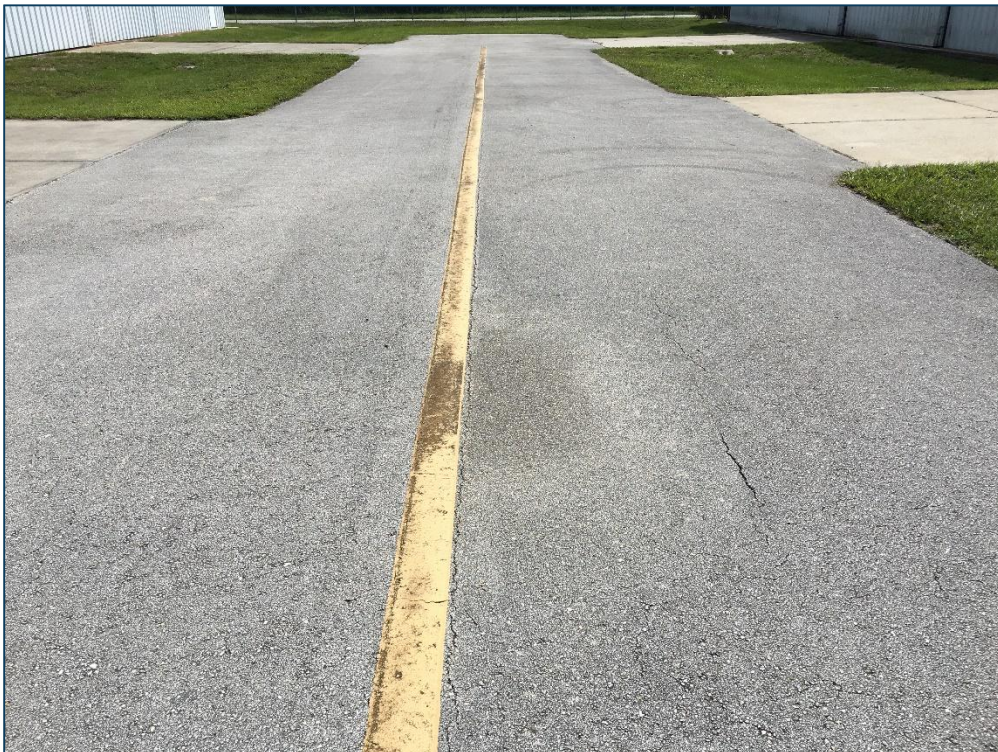
Apron AP T-HANG, Section 4205, Sample Unit 300 – Low Severity (52) Raveling, Low Severity (48) Longitudinal and Transverse Cracking, Low Severity (57) Weathering
