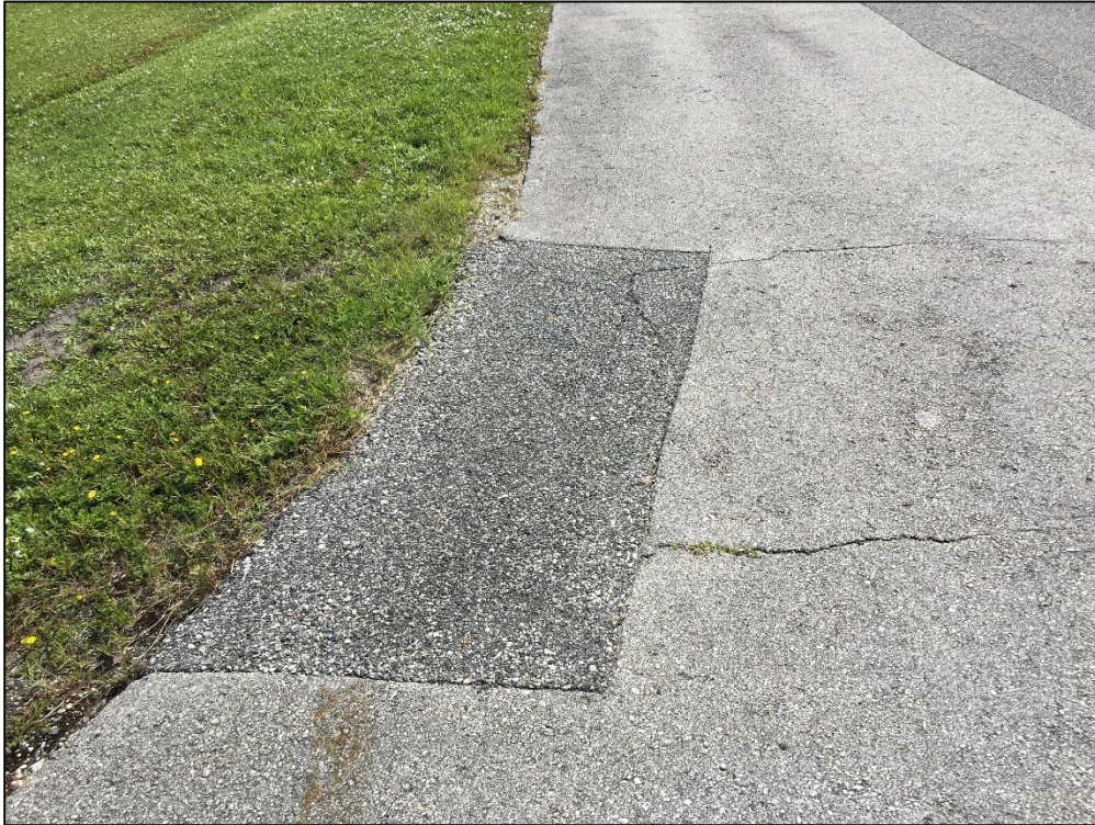
Apron AP T-HANG, Section 4205, Sample Unit 600 – Low Severity (52) Raveling, Low Severity (48) Longitudinal and Transverse Cracking, Low Severity (50) Patching, Low Severity (57) Weathering
