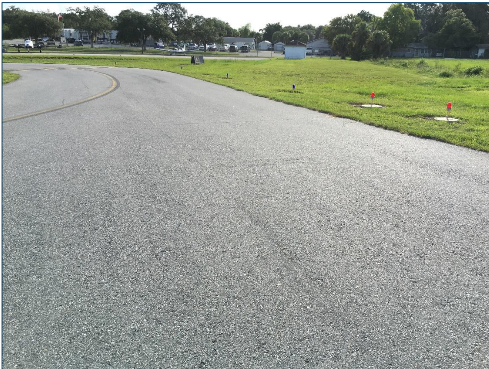
Runway 15-33, Section 6105, Sample Unit 129 – Low Severity (48) Longitudinal and Transverse Cracking, Low Severity (57) Weathering
