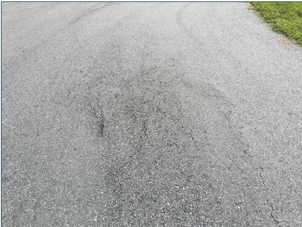
Taxiway A, Section 105, Sample Unit 100 – Low Severity (48) Longitudinal and Transverse Cracking, Low Severity (57) Weathering, Medium Severity (57) Weathering
