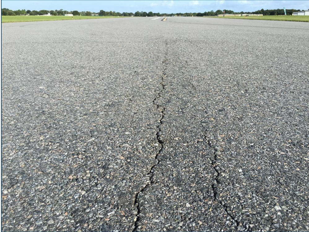
Runway 15-33, Section 6105, Sample Unit 129 – Low Severity (48) Longitudinal and Transverse Cracking Low Severity (56) Swelling, Low Severity (57) Weathering
