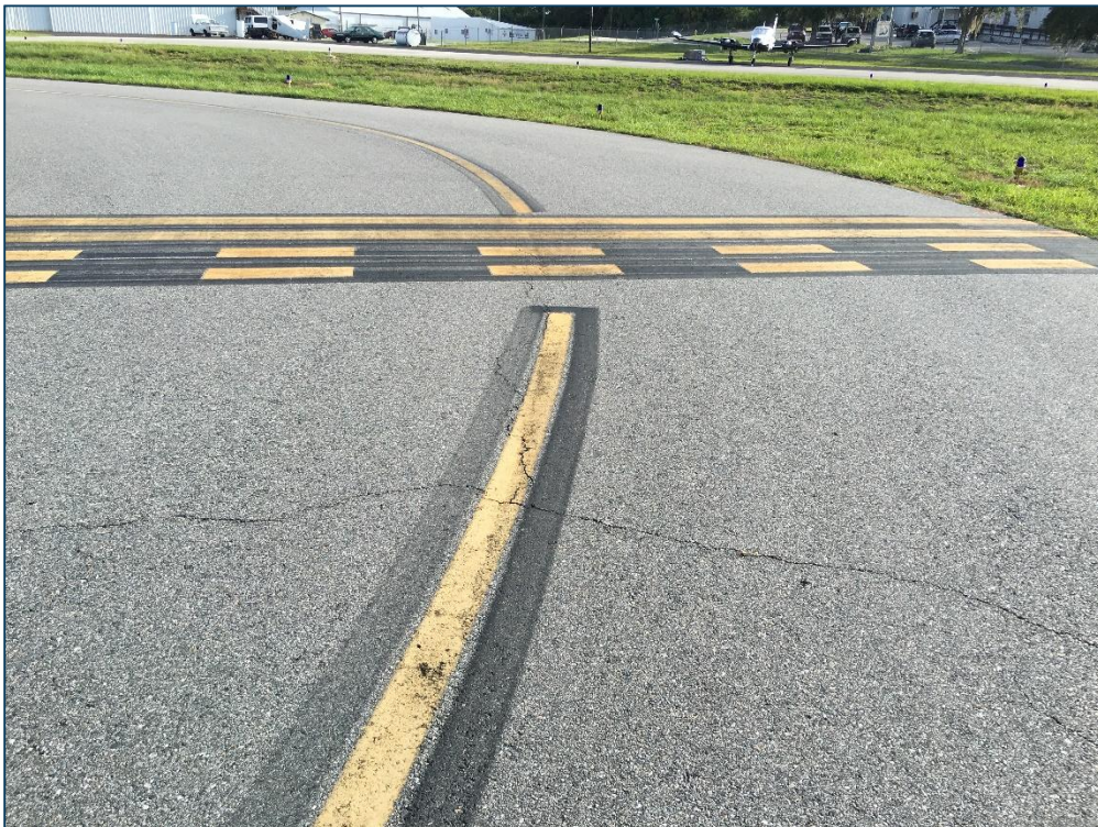
Taxiway A, Section 110, Sample Unit 100 – Low Severity (57) Weathering, Low Severity (52) Raveling, Low Severity (48) Longitudinal and Transverse Cracking
