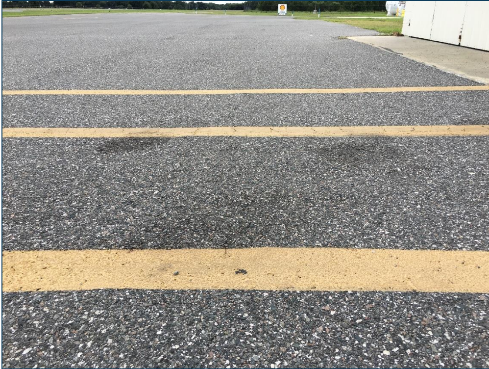
Taxiway AP, Section 110, Sample Unit 204 – Low Severity (56) Swelling, Low Severity (52) Raveling, Low Severity (57) Weathering
