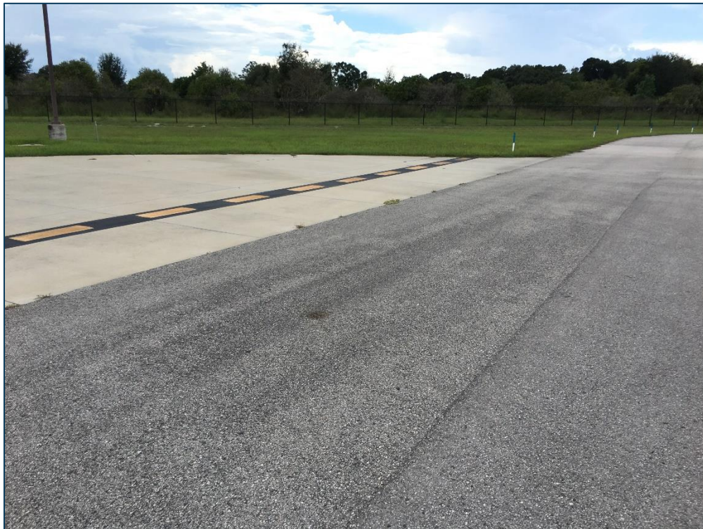
Taxilane To Hangar, Section 110, Sample Unit 301 – Low Severity (48) Longitudinal and Transverse Cracking, Low Severity (52) Raveling, Low Severity (57) Weathering
