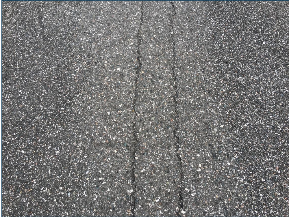
Taxiway AP, Section 110, Sample Unit 100 – Low Severity (48) Longitudinal and Transverse Cracking, Low Severity (52) Raveling, Low Severity (57) Weathering
