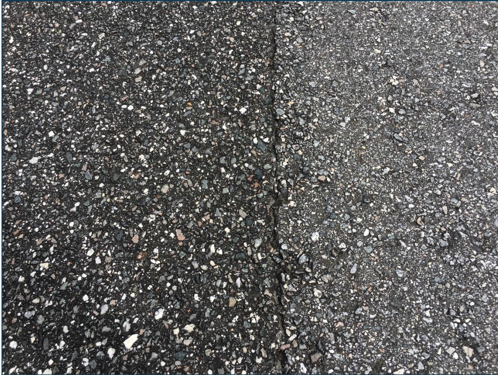
Run-Up Apron, Section 5105, Sample Unit 100 – Low Severity (57) Weathering, Low Severity (52) Raveling, Low Severity (48) Longitudinal and Transverse Cracking
