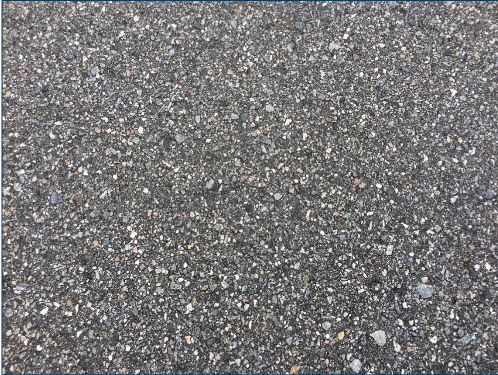
Taxilane To Hangar, Section 4115, Sample Unit 501 – Low Severity (57) Weathering, Medium Severity (57) Weathering
