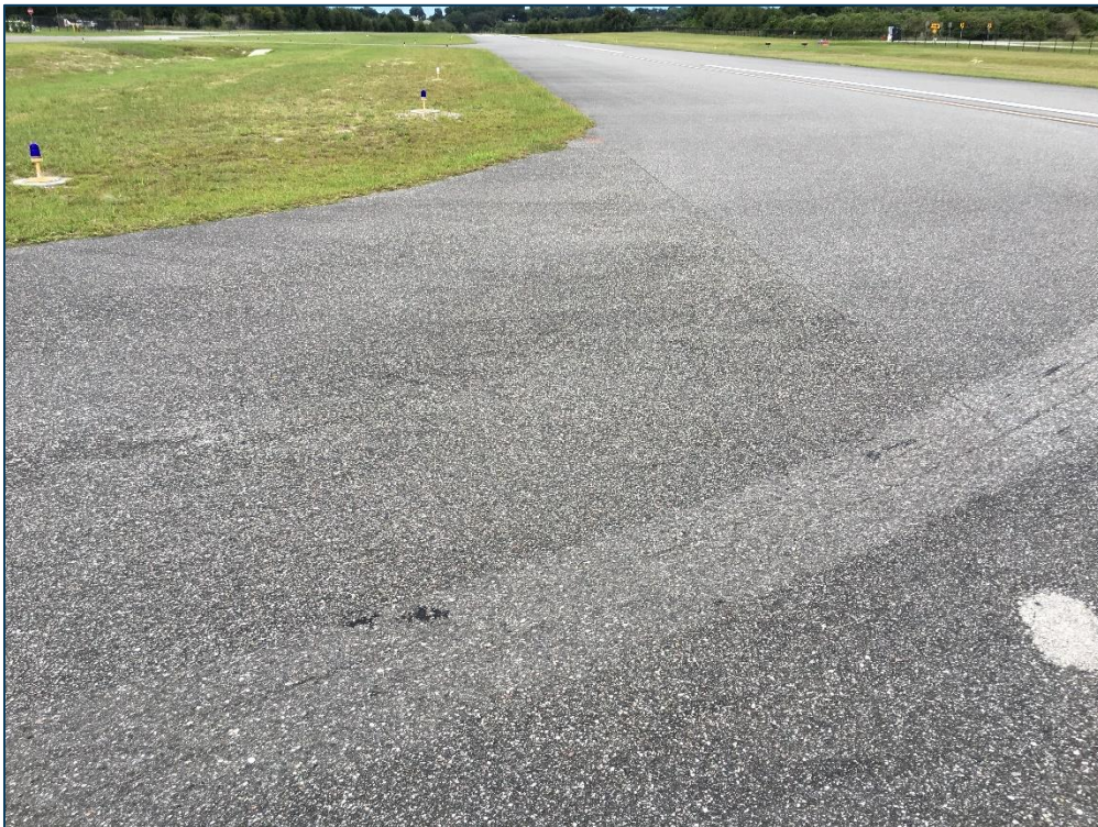
Taxiway AP, Section 110, Sample Unit 100 – Low Severity (52) Raveling, Low Severity (57) Weathering
