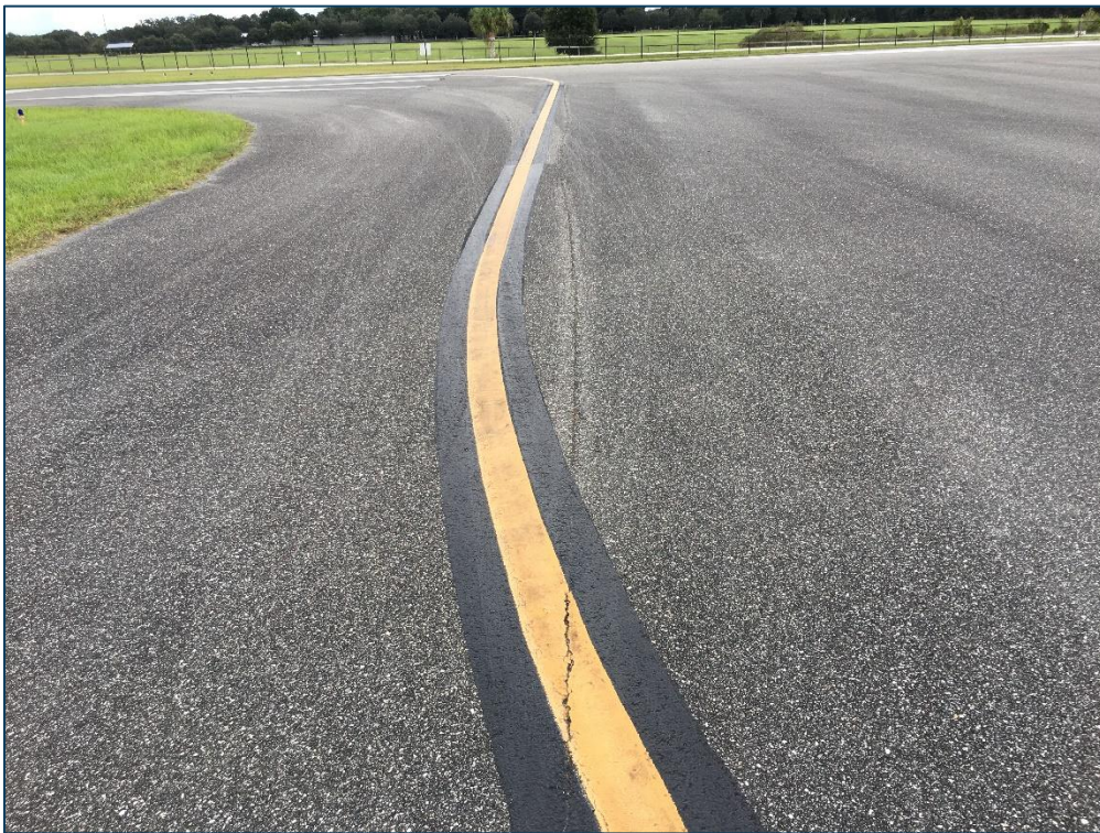
Taxilane To Hangar, Section 4205, Sample Unit 102 – Low Severity (48) Longitudinal and Transverse Cracking, Low Severity (52) Raveling, Low Severity (57) Weathering
