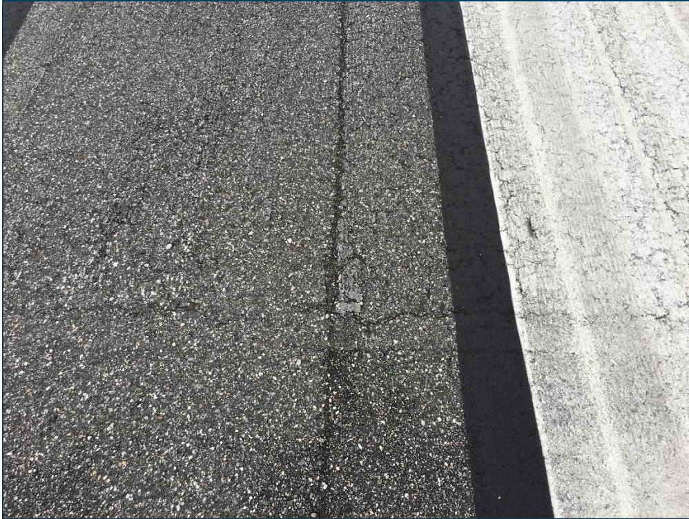
Runway 01-19, Section 6105, Sample Unit 202 – Low Severity (48) Longitudinal and Transverse Cracking, Low Severity (52) Raveling, Low Severity (57) Weathering
