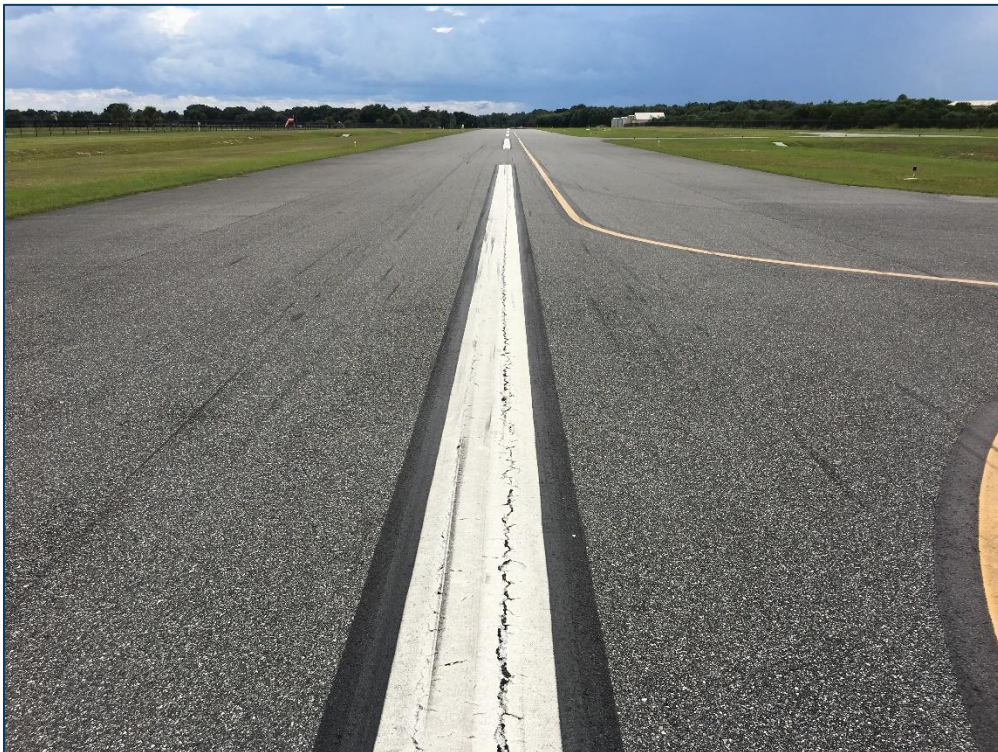
Runway 01-19, Section 6105, Sample Unit 217 – Low Severity (48) Longitudinal and Transverse Cracking, Low Severity (52) Raveling, Low Severity (57) Weathering
