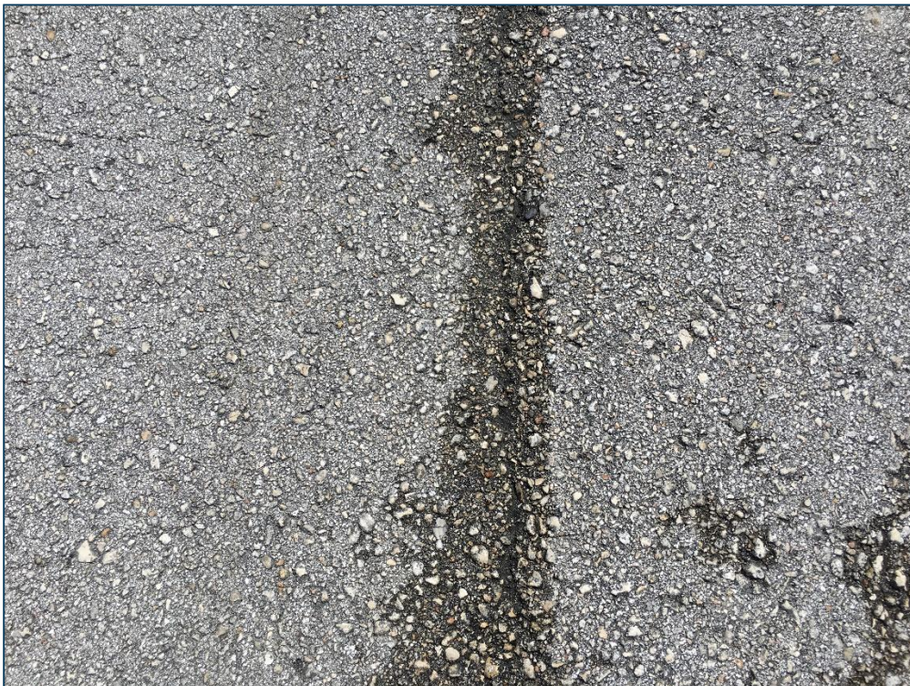
Taxiway A, Section 425, Sample Unit 99 – Low Severity (48) Longitudinal and Transverse Cracking, Low Severity (57) Weathering, Low Severity (52) Raveling
