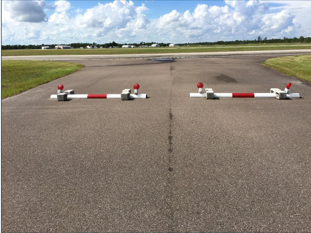
Taxiway E, Section 700, Sample Unit 101 – Low Severity (48) Longitudinal and Transverse Cracking, Low Severity (57) Weathering
