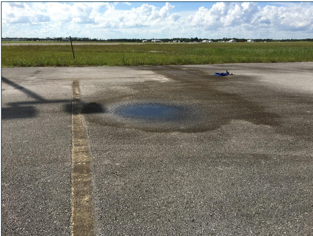
Apron Term, Section 5705, Sample Unit 101 – Low Severity (45) Depression, Low Severity (57) Weathering
