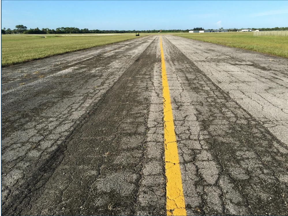
Taxiway C, Section 305, Sample Unit 305 – Medium Severity (43) Block Cracking, Medium Severity (41) Alligator Cracking, Low Severity (53) Rutting, Low Severity (52) Raveling
