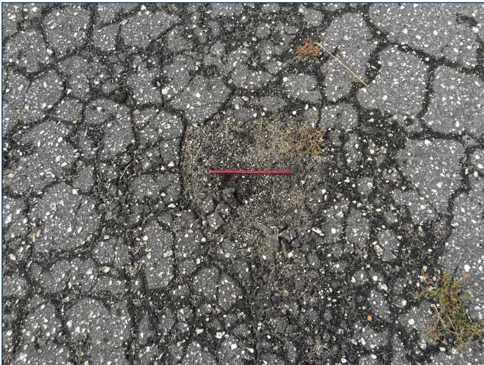
Apron SE, Section 5605, Sample Unit 101 – Low Severity (52) Raveling and Medium Severity (41) Alligator Cracking
