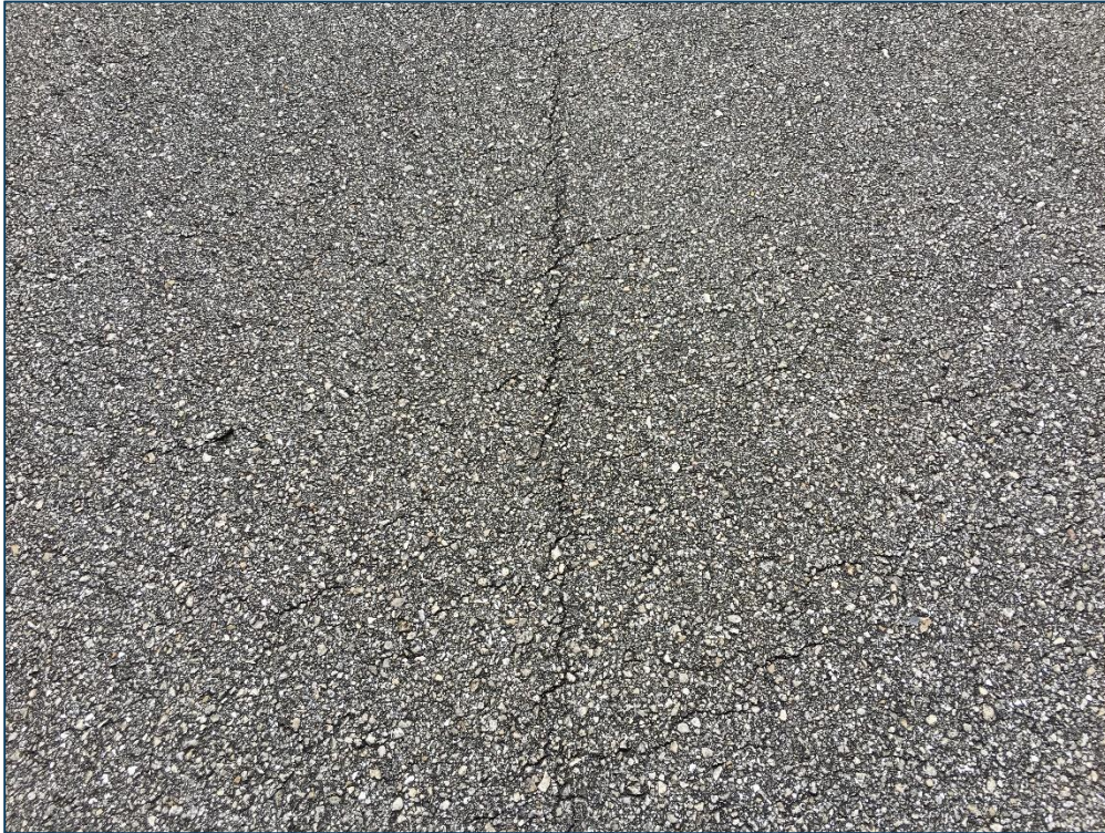
Apron RU SW, Section 5405, Sample Unit 301 – Low Severity (48) Longitudinal and Transverse Cracking, Low Severity (57) Weathering
