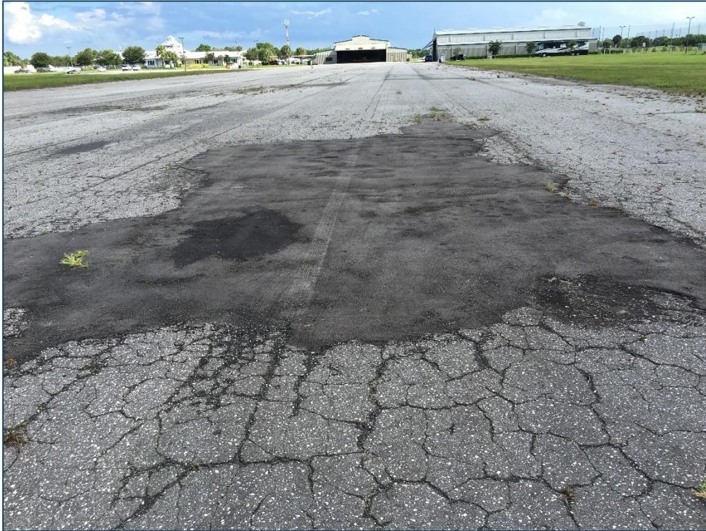
Apron SE, Section 5605, Sample Unit 101 – Low Severity (43) Block Cracking, Medium Severity (50) Patching, Medium Severity (41) Alligator Cracking, Low Severity (52) Raveling
