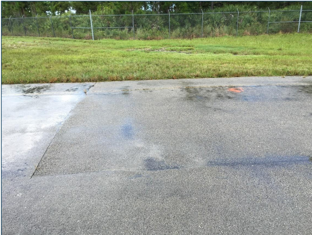
Apron RU E, Section 5510, Sample Unit 302 – Low Severity (50) Patching and Low Severity (57) Weathering
