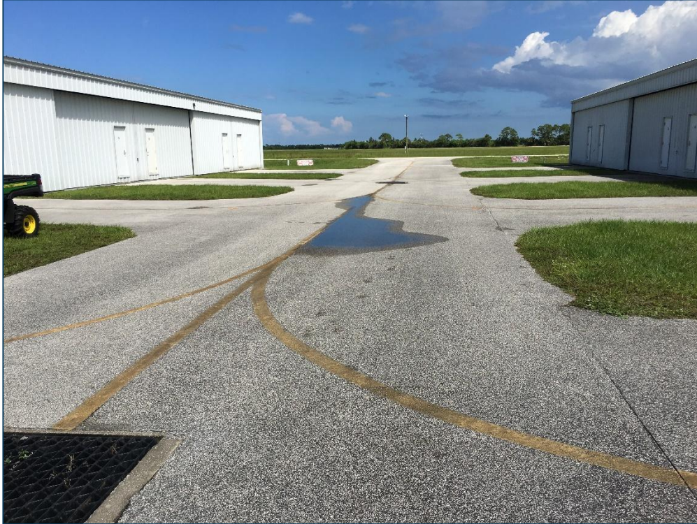
Apron T-Hang, Section 5305, Sample Unit 301 – Low Severity (48) Longitudinal and Transverse Cracking, Low Severity (45) Depression, Low Severity (57) Weathering
