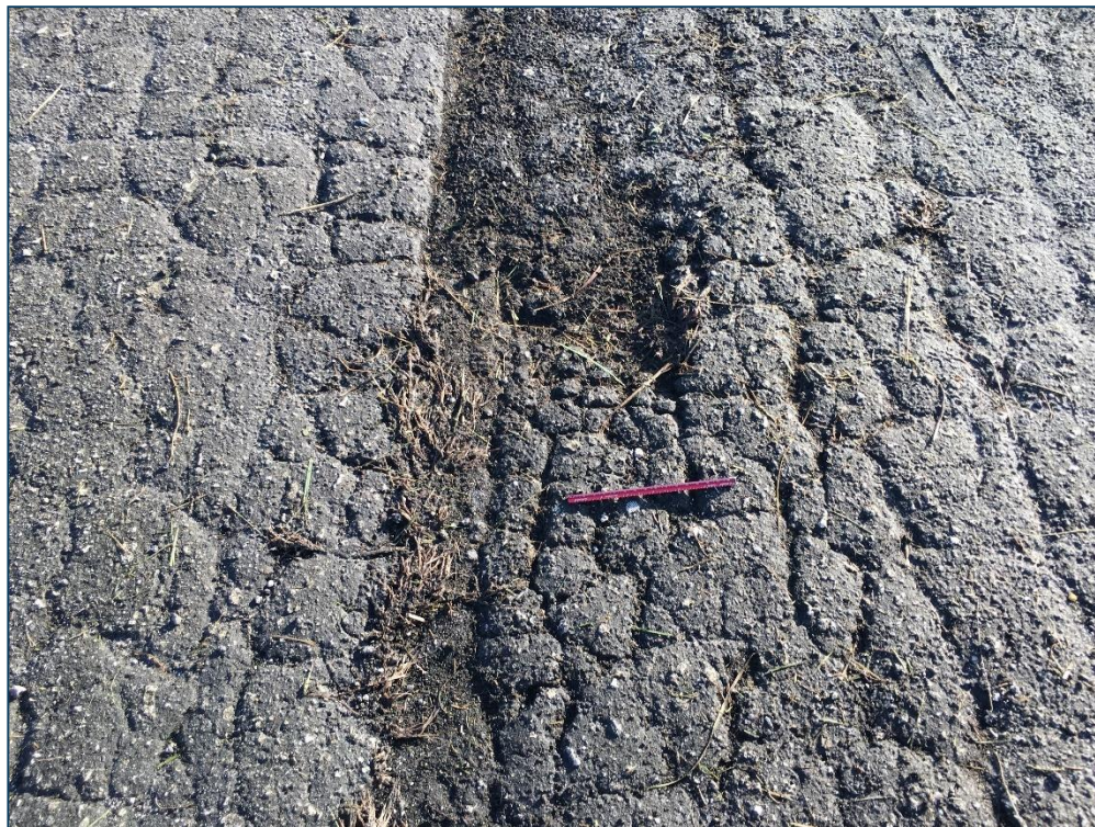
Taxiway C, Section 305, Sample Unit 300 – Medium Severity (41) Alligator Cracking, Medium Severity (52) Raveling
