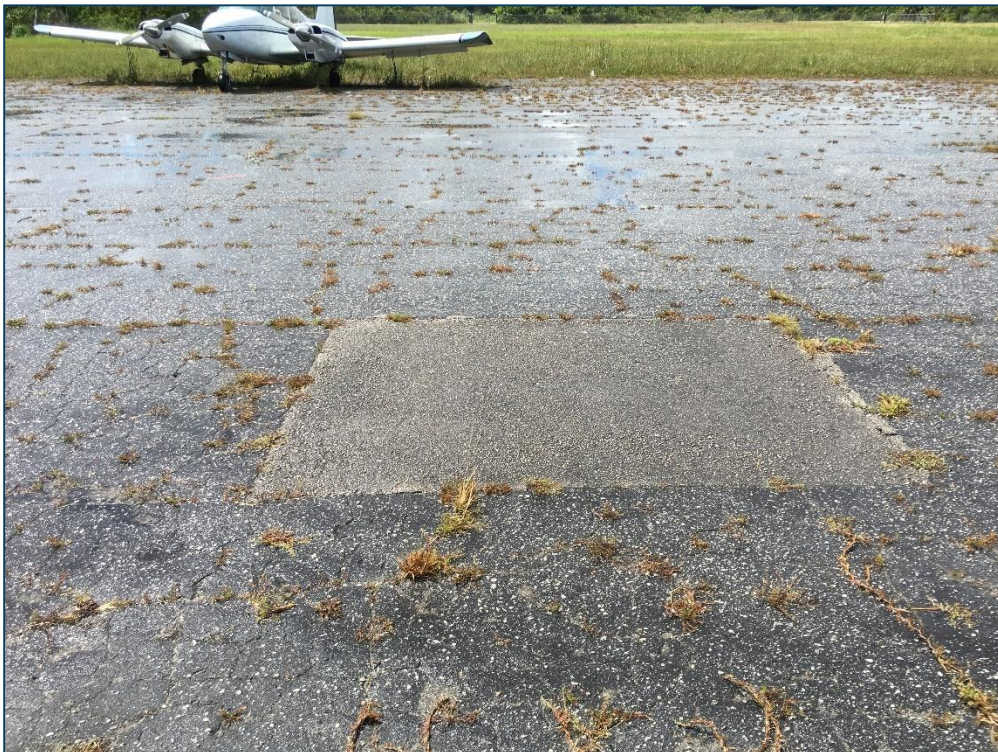
Apron W, Section 5115, Sample Unit 435 – Medium Severity (43) Block Cracking, Low Severity (50) Patching, Low Severity (52) Raveling
