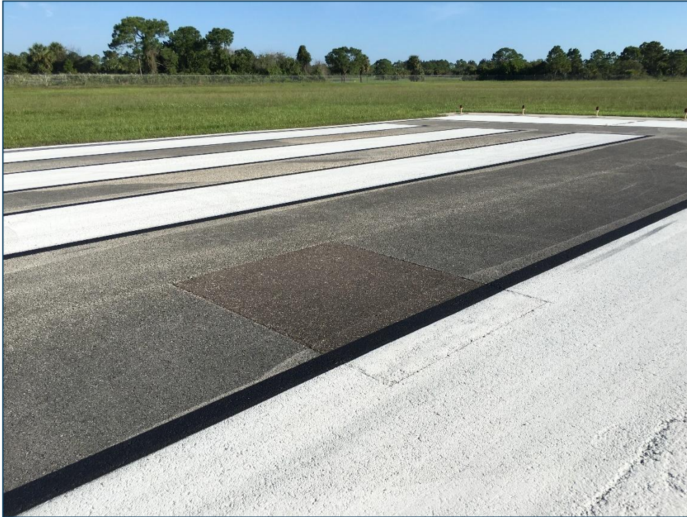
Runway 5-23, Section 6205, Sample Unit 379 – Low Severity (48) Longitudinal and Transverse Cracking, Low Severity (50) Patching, Low Severity (57) Weathering
