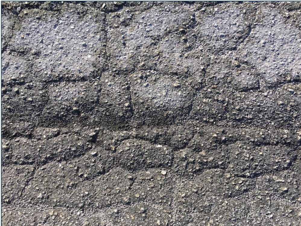
Taxiway C, Section 305, Sample Unit 305 – Medium Severity (41) Alligator Cracking, Low Severity (53) Rutting, Low Severity (52) Raveling
