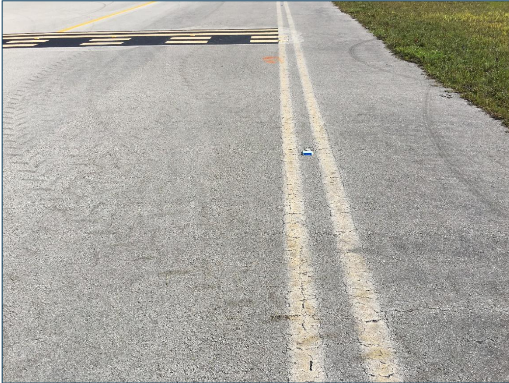
Taxiway CONN, Section 515, Sample Unit 100 – Low Severity (48) Longitudinal and Transverse Cracking, Low Severity (57) Weathering, Low Severity (52) Raveling
