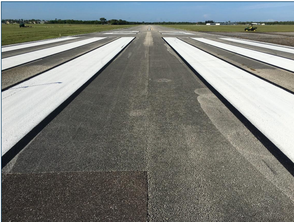
Runway 5-23, Section 6205, Sample Unit 379 – Low Severity (48) Longitudinal and Transverse Cracking, Low Severity (50) Patching, Low Severity (57) Weathering, Low Severity (52) Raveling
