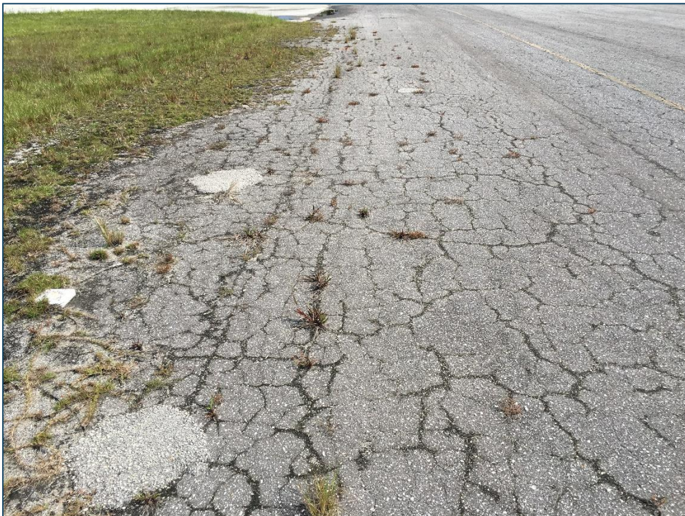
Apron SE, Section 5605, Sample Unit 305 – Low Severity (41) Alligator Cracking and Low Severity (50) Patching, Low Severity (52) Raveling
