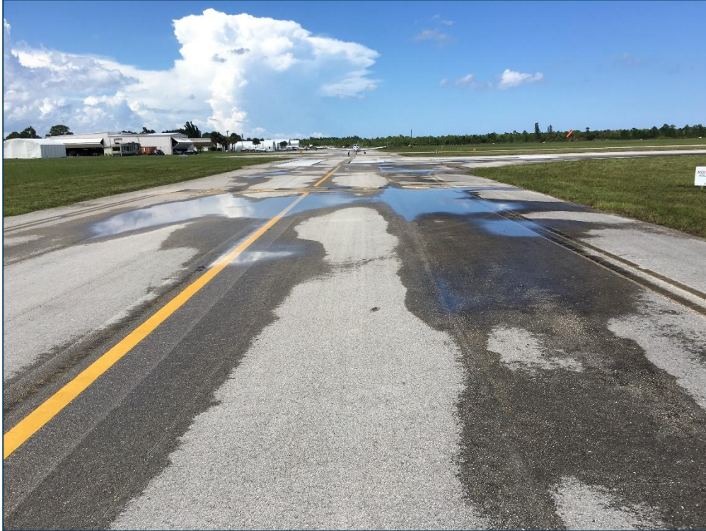
Taxiway A, Section 425, Sample Unit 99 – Low Severity (45) Depression, Low Severity (52) Raveling, Low Severity (48) Longitudinal and Transverse Cracking, Low Severity (57) Weathering
