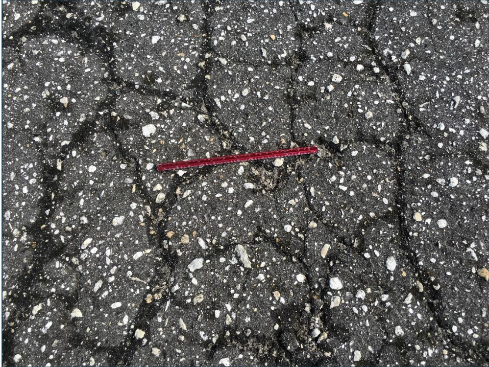
Apron SE, Section 5605, Sample Unit 203 – Low Severity (41) Alligator Cracking, Low Severity (43) Block Cracking, Low Severity (52) Raveling
