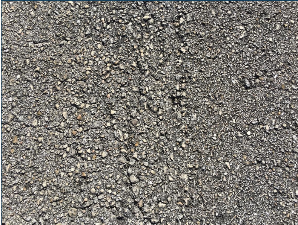
Runway 10-28, Section 6305, Sample Unit 514 – Low Severity (52) Raveling
