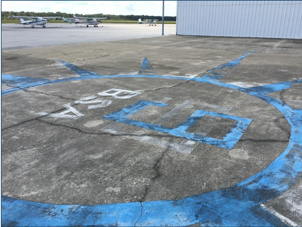
Hangar Apron, Section 4230, Sample Unit 401 – Low Severity (65) Joint Seal Damage, (73) Shrinkage Cracks, Low Severity (72) Shattered Slab
