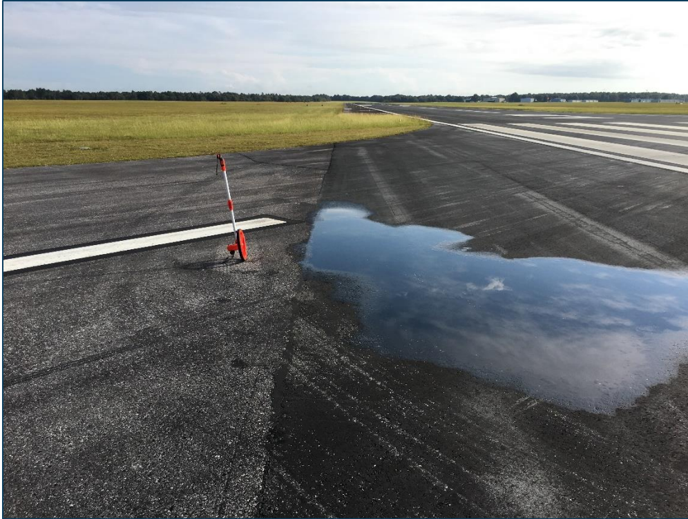
Runway 10-28, Section 6105, Sample Unit 177 – Low Severity (48) Longitudinal and Transverse Cracking, Low Severity (52) Raveling, Low Severity (57) Weathering
