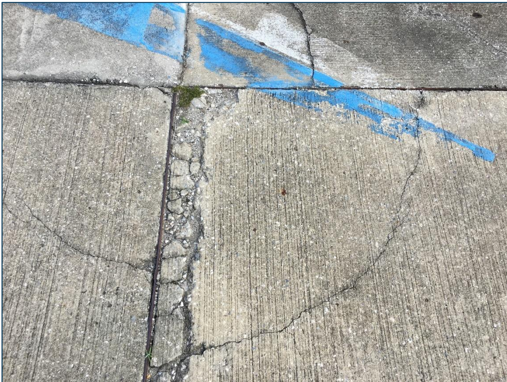
Hangar Apron, Section 4230, Sample Unit 401 – Low Severity (65) Joint Seal Damage, (73) Shrinkage Cracks, Medium Severity (74) Joint Spalling, Low Severity (62) Corner Break
