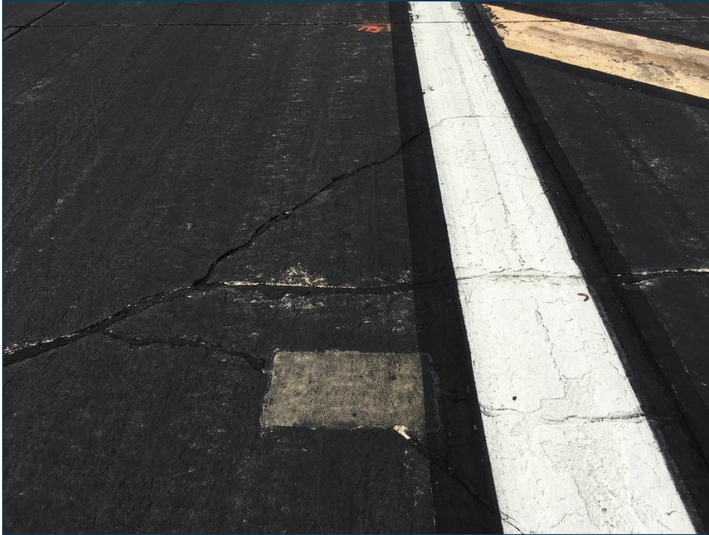
Runway 5-23, Section 6215, Sample Unit 195 – Low Severity (65) Joint Seal Damage, Medium Severity (63) Longitudinal, Transverse, and Diagonal Cracking, Low Severity (66) Small Patching
