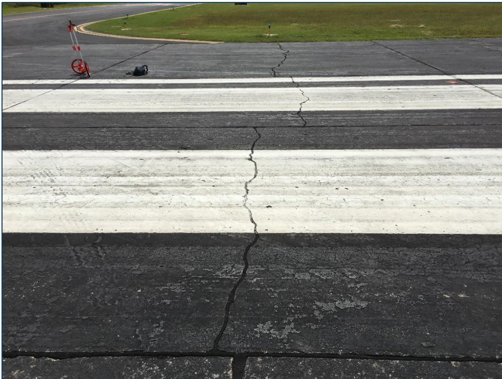
Runway 5-23, Section 6215, Sample Unit 198 – Low Severity (63) Longitudinal, Transverse, and Diagonal Cracking, Low Severity (65) Joint Seal Damage
