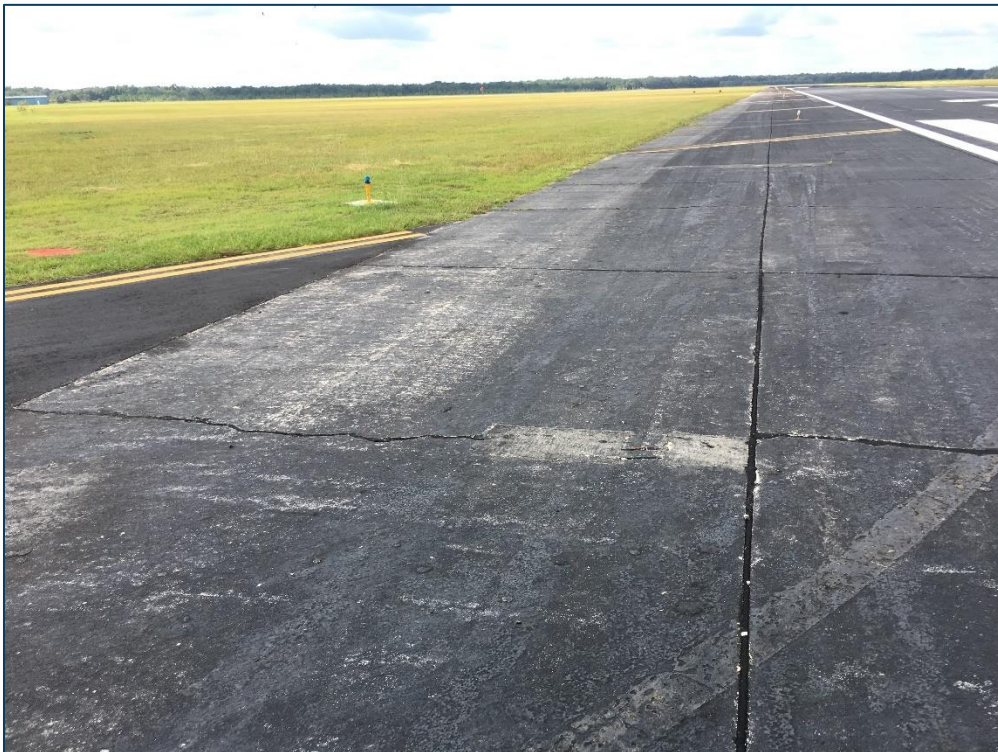
Taxiway A, Section 115, Sample Unit 135 – Low Severity (63) Longitudinal, Transverse, and Diagonal Cracking, Low Severity (65) Joint Seal Damage, Low Severity (66) Small Patching
