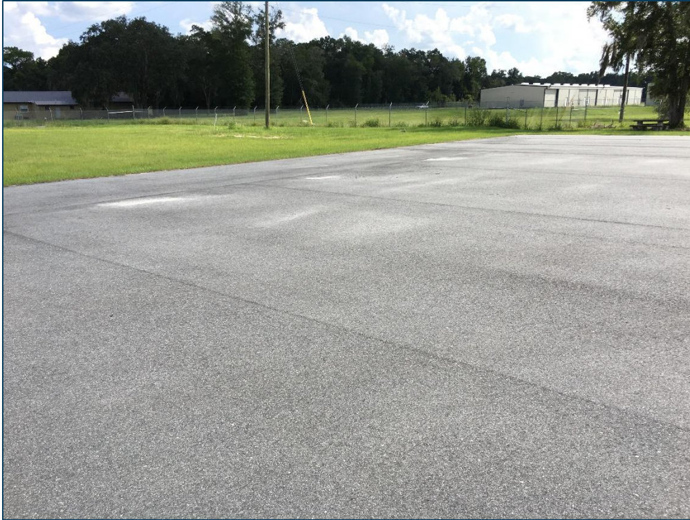
Terminal Apron, Section 4305, Sample Unit 203 – Low Severity (57) Weathering
