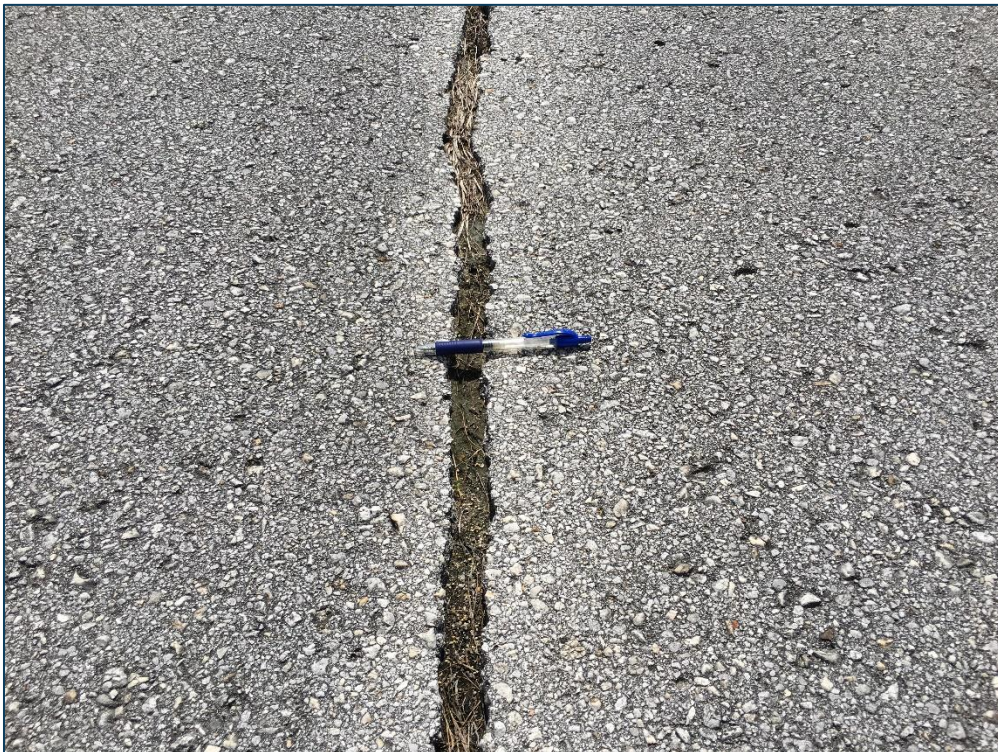
Hangar Apron, Section 4220, Sample Unit 300 – Low and Medium Severity (48) Longitudinal and Transverse Cracking, Low Severity (52) Raveling, Low Severity (57) Weathering
