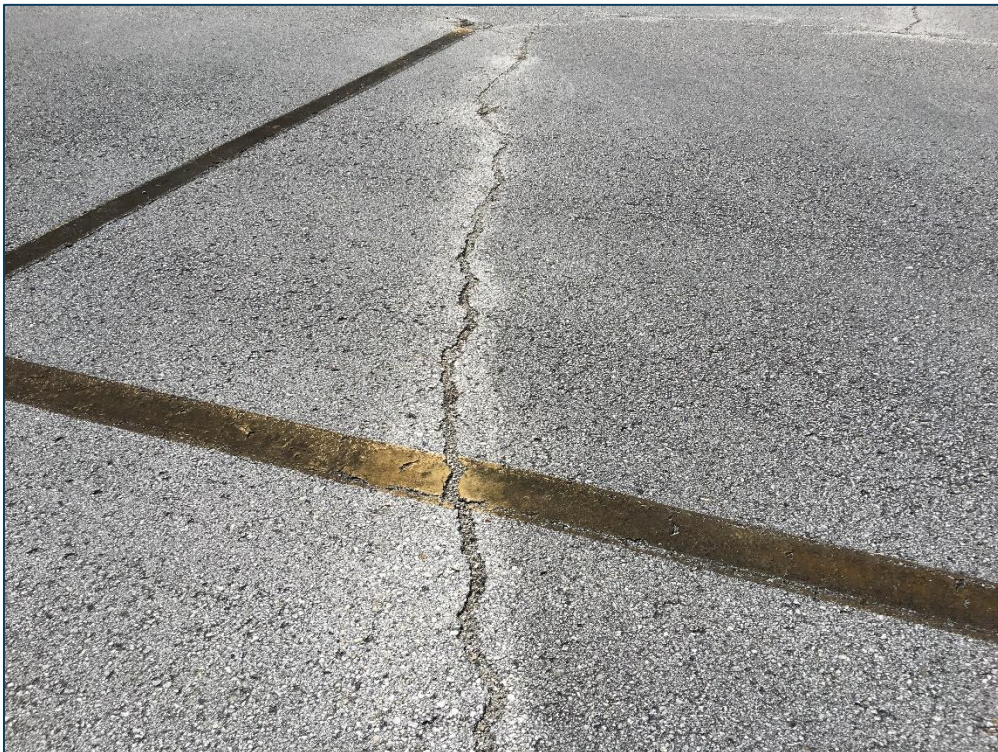
Apron AP, Section 4105, Sample Unit 204 – Medium Severity (48) Longitudinal and Transverse Cracking, Low Severity (52) Raveling
