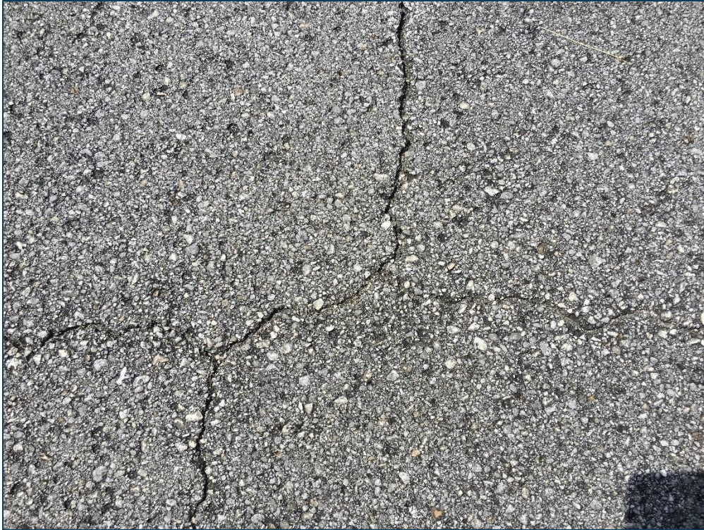
Apron, Section 4105, Sample Unit 307 – Low Severity (48) Longitudinal and Transverse Cracking, Medium Severity (48) Longitudinal and Transverse Cracking, Low Severity (52) Raveling
