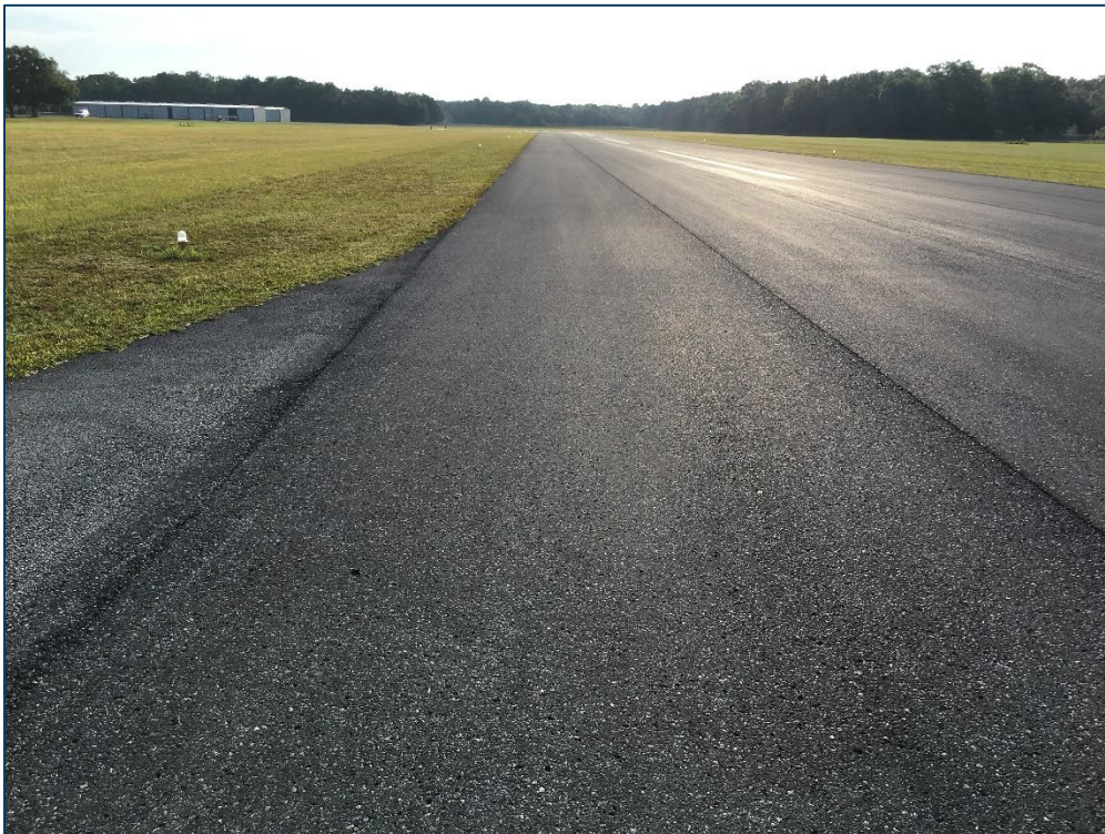
Runway 10-28, Section 6105, Sample Unit 118 – Low Severity (48) Longitudinal and Transverse Cracking, Low Severity (57) Weathering
