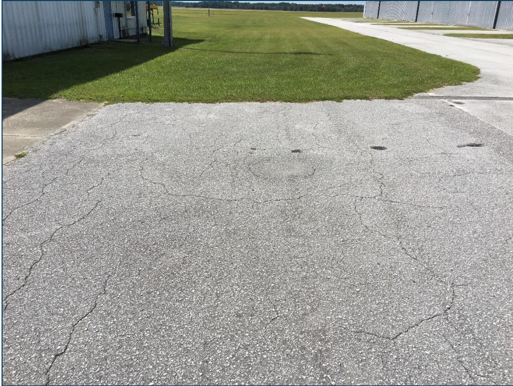
Hangar Apron, Section 4235, Sample Unit 400 – Low Severity (45) Depression, Low Severity (48) Longitudinal and Transverse Cracking, Low Severity (45) Depression, Low Severity (52) Raveling
