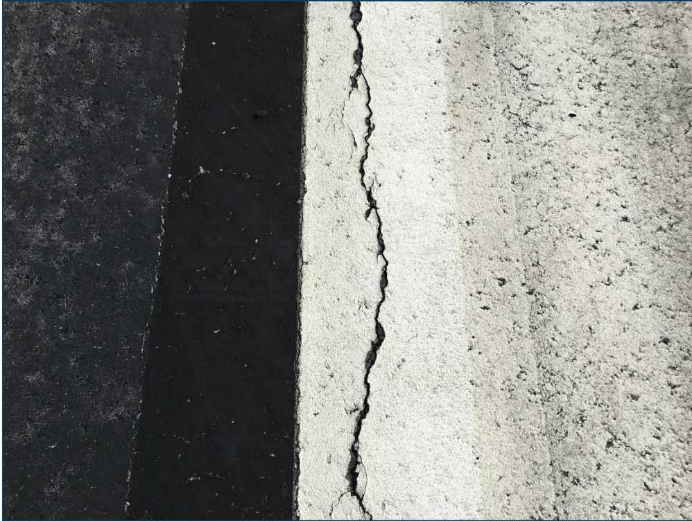
Runway 10-28, Section 6105, Sample Unit 101 – Low Severity (48) Longitudinal and Transverse Cracking, Low Severity (57) Weathering
