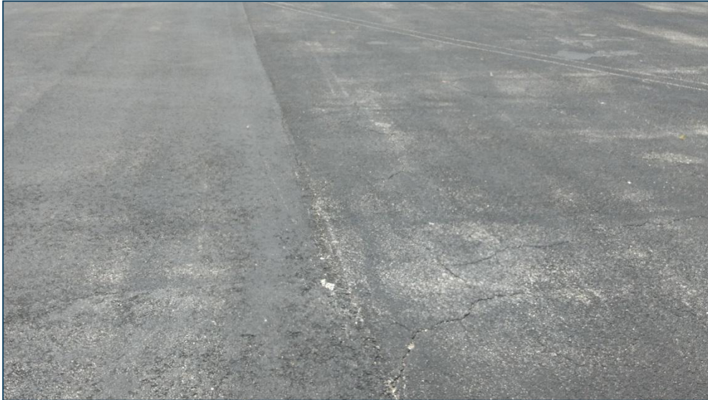
NW Apron, Section 4105, Sample Unit 454 – Low Severity (48) Longitudinal and Transverse Cracking, Low Severity (50) Patching, Low Severity (52) Raveling
