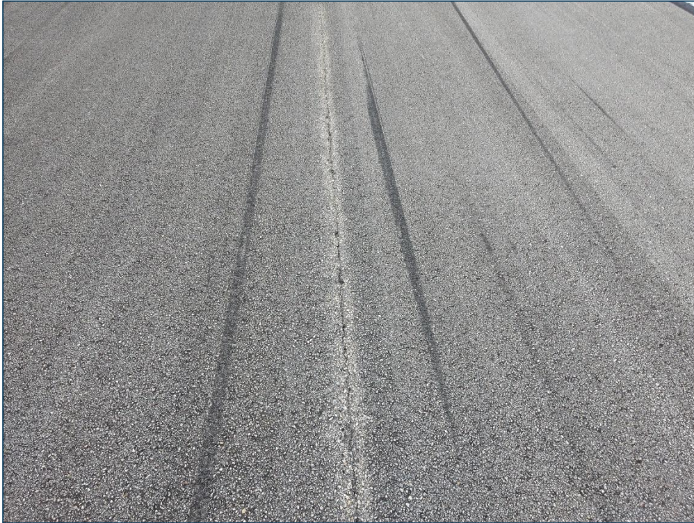
Runway 18-36, Section 6105, Sample Unit 305 – Low Severity (48) Longitudinal and Transverse Cracking, Low Severity (52) Raveling, Low Severity (57) Weathering
