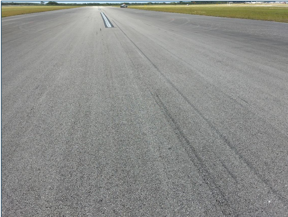
Runway 18-36, Section 6105, Sample Unit 329 – Low Severity (48) Longitudinal and Transverse Cracking, Low Severity (57) Weathering
