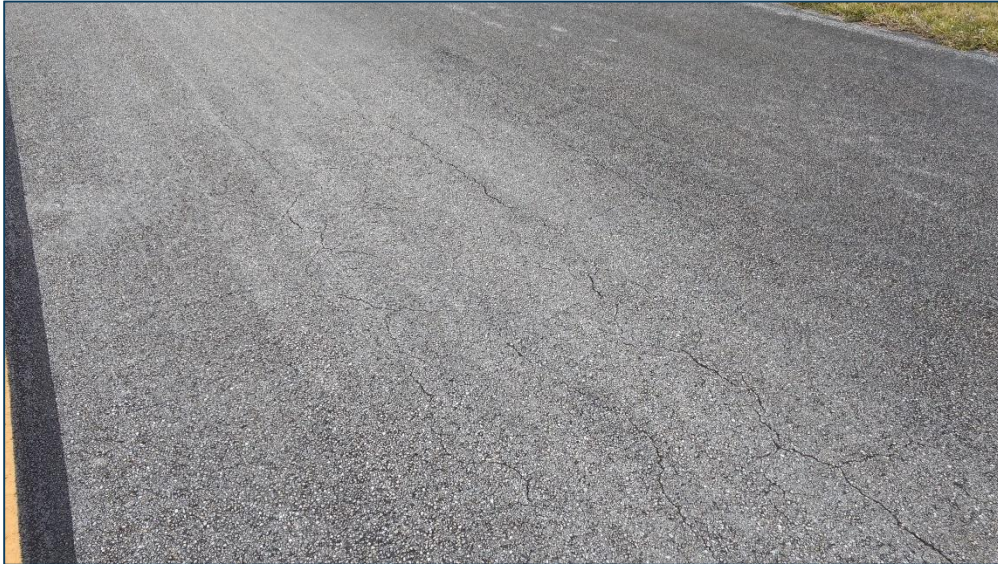
Taxiway A, Section 215, Sample Unit 117 – Low Severity (43) Block Cracking, Low Severity (48) Longitudinal and Transverse Cracking, Low Severity (52) Raveling
