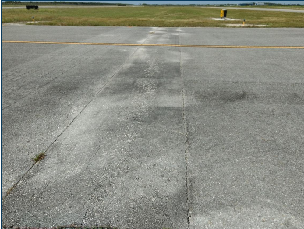
Taxiway B3, Section 130, Sample Unit 302 – Low Severity (48) Longitudinal and Transverse Cracking, Low Severity (50) Patching, Low Severity (52) Raveling, Medium Severity (52) Raveling
