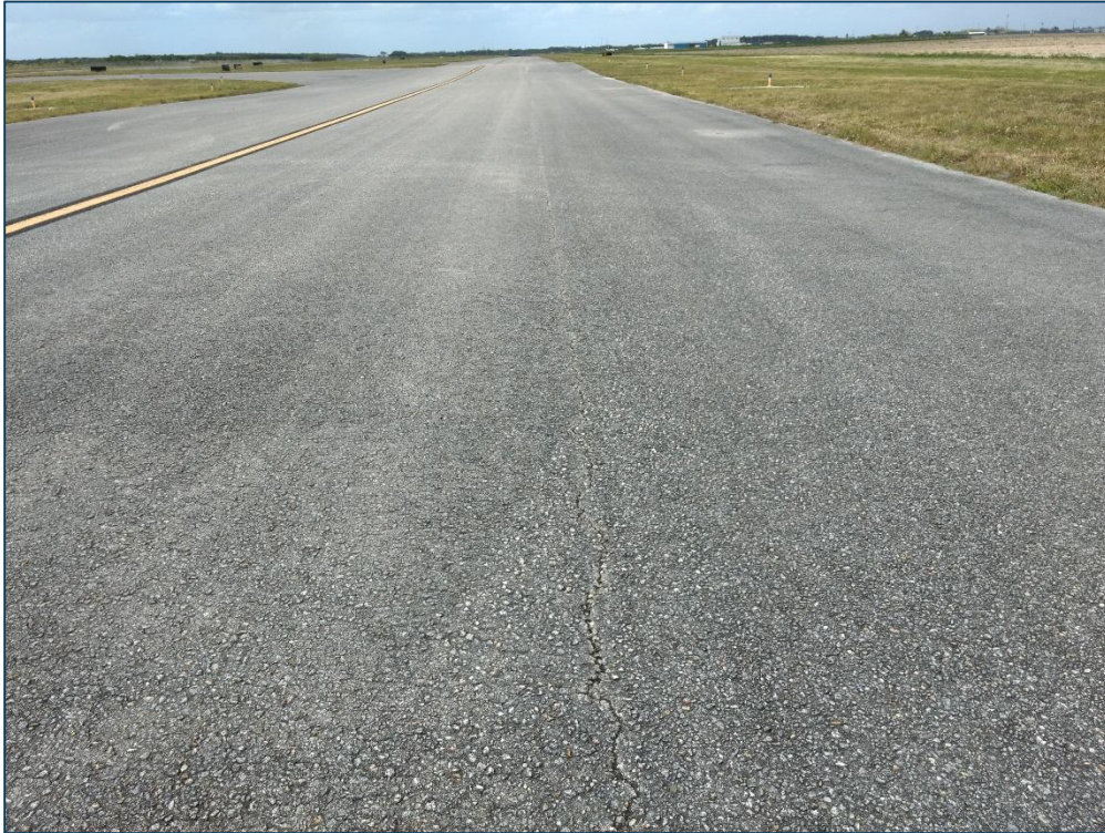
Taxiway B, Section 105, Sample Unit 103 – Low Severity (48) Longitudinal and Transverse Cracking, Low Severity (52) Raveling
