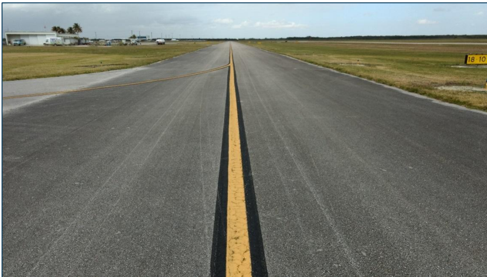
Taxiway A, Section 215, Sample Unit 123 – Low Severity (48) Longitudinal and Transverse Cracking, Low Severity (52) Raveling
