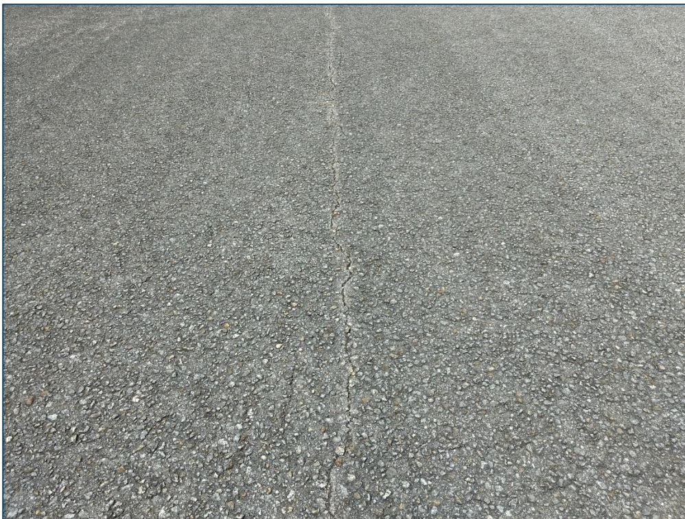
Taxiway B, Section 105, Sample Unit 132 – Low Severity (48) Longitudinal and Transverse Cracking, Low Severity (52) Raveling
