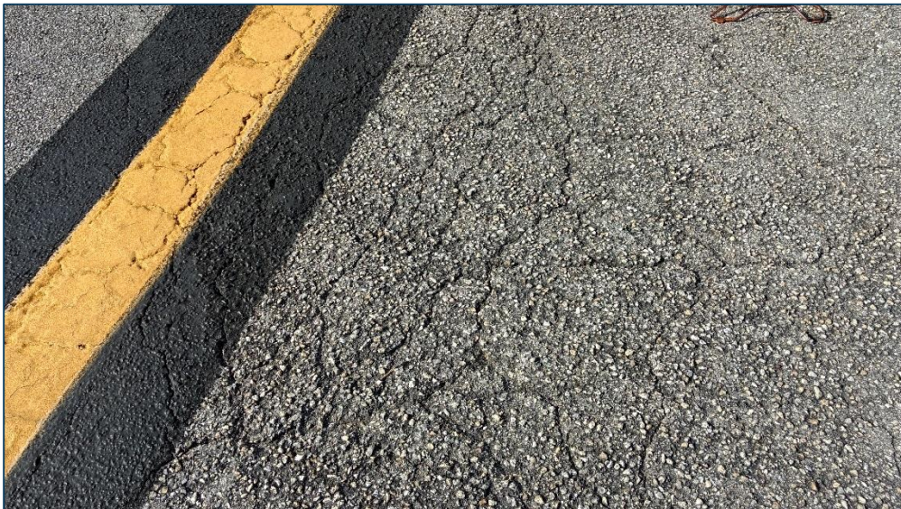
Taxiway A1, Section 230, Sample Unit 100 – Low Severity (41) Alligator Cracking, Medium Severity (52) Raveling
