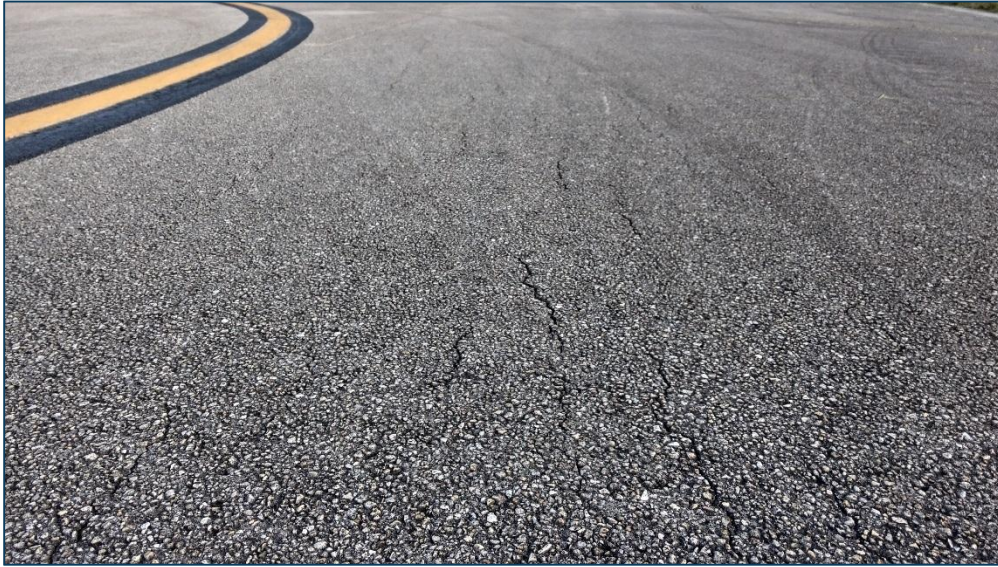
Taxiway A3, Section 250, Sample Unit 301 – Low Severity (41) Alligator Cracking, Low Severity (52) Raveling, Low Severity (57) Weathering
