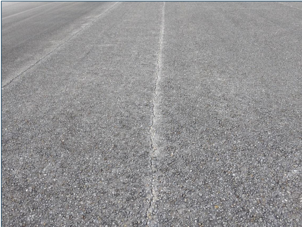
Runway 18-36, Section 6110, Sample Unit 572 – Low Severity (48) Longitudinal and Transverse Cracking, Low Severity (52) Raveling
