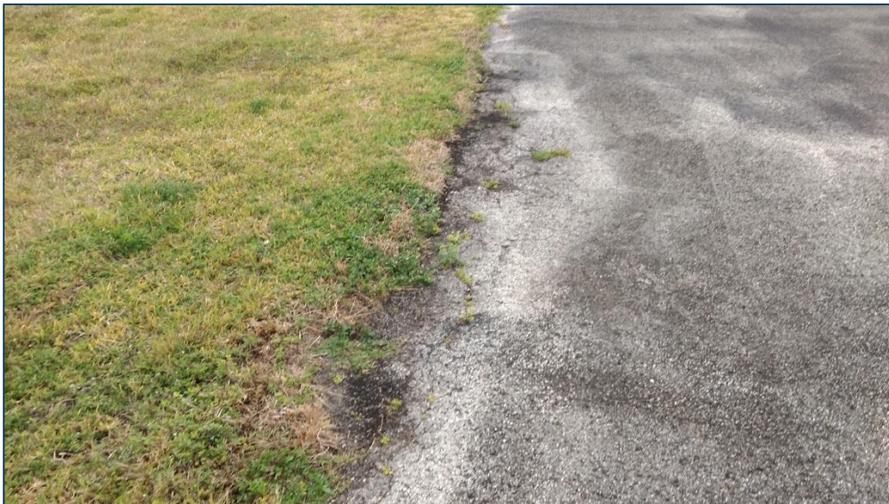
NW Apron, Section 4105, Sample Unit 100 – Low and Medium Severity (48) Longitudinal and Transverse Cracking, Low Severity (52) Raveling
