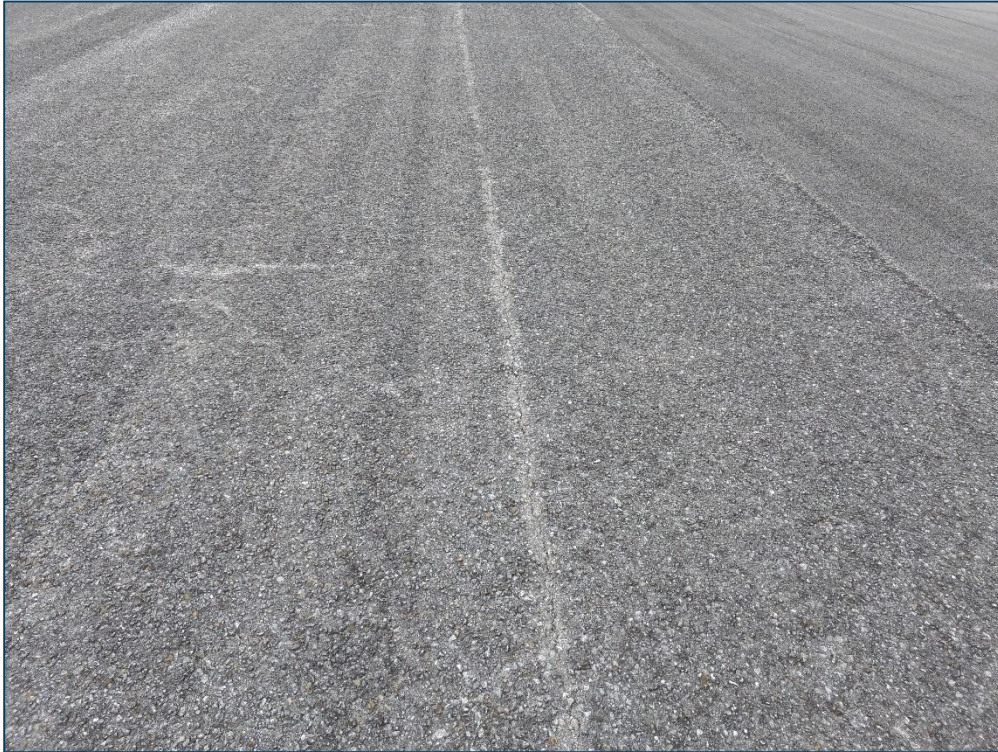
Runway 18-36, Section 6110, Sample Unit 128 – Low Severity (48) Longitudinal and Transverse Cracking, Low Severity (52) Raveling
