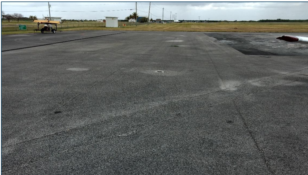
North Apron, Section 4205, Sample Unit 403 – Low Severity (48) Longitudinal and Transverse Cracking, Low Severity (50) Patching, Low Severity (52) Raveling
