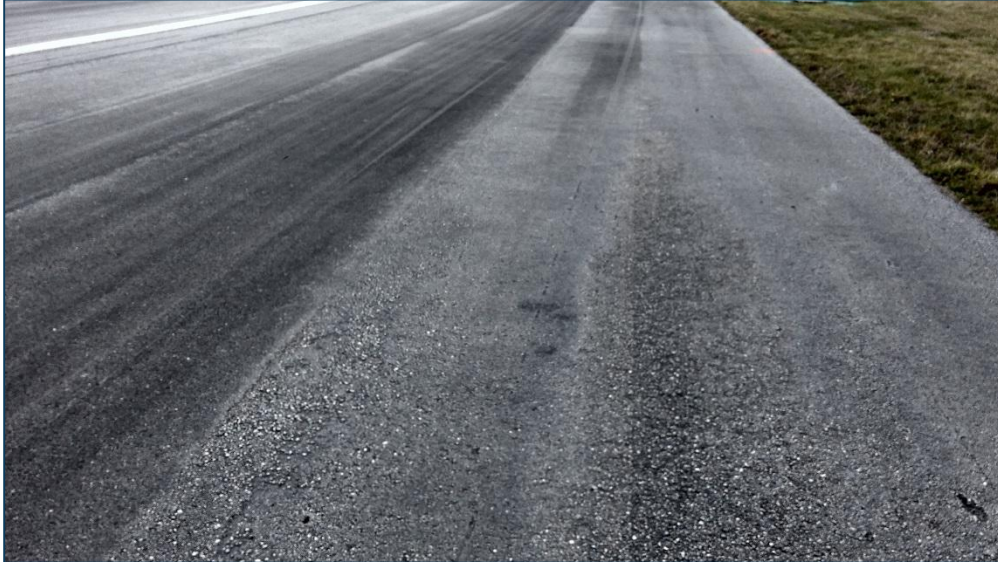
Runway 10-28, Section 6205, Sample Unit 143 – Low Severity (48) Longitudinal and Transverse Cracking, Low Severity (52) Raveling, Low Severity (57) Weathering
