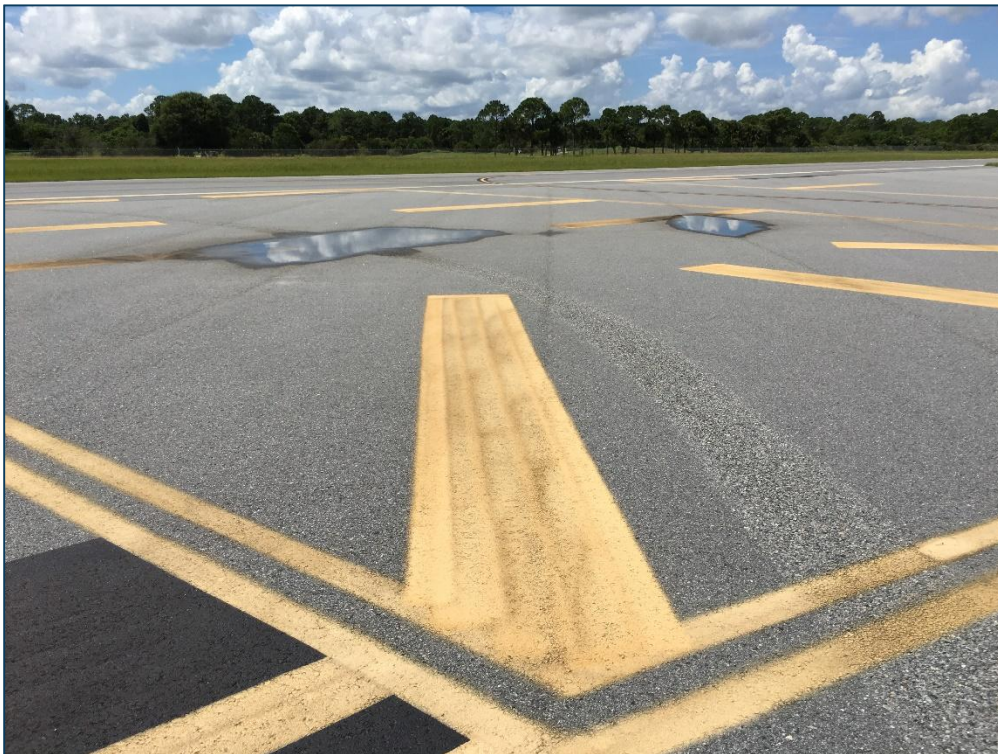
Taxiway C2, Section 705, Sample Unit 200 – Low Severity (45) Depression, Low Severity (57) Weathering
