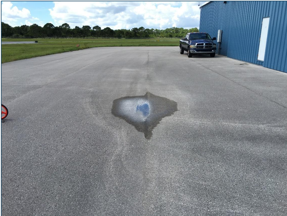
Apron AP, Section 4120, Sample Unit 301 – Low Severity (45) Depression, Low Severity (48) Longitudinal and Transverse Cracking, Low Severity (57) Weathering, Low Severity (52) Raveling
