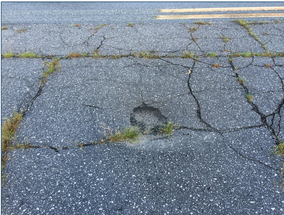
Apron AP, Section 4130, Sample Unit 306 – Medium Severity (41) Alligator Cracking, High Severity (43) Block Cracking, Medium Severity (45) Depression, Low Severity (52) Raveling
