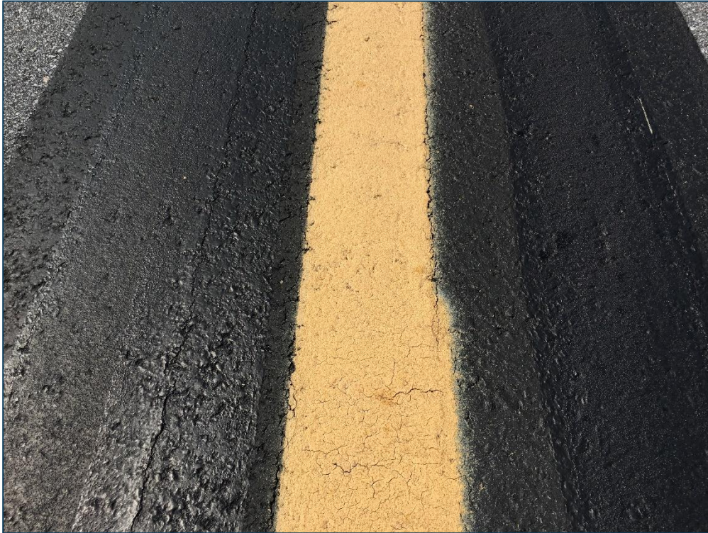
Taxiway A, Section 305, Sample Unit 106 – Low Severity (48) Longitudinal and Transverse Cracking, Low Severity (57) Weathering
