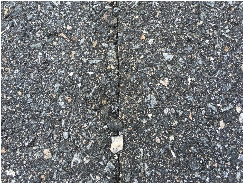
Runway 10-28, Section 6205, Sample Unit 141 – Low Severity (48) Longitudinal and Transverse Cracking, Low Severity (52) Raveling, Low Severity (57) Weathering
