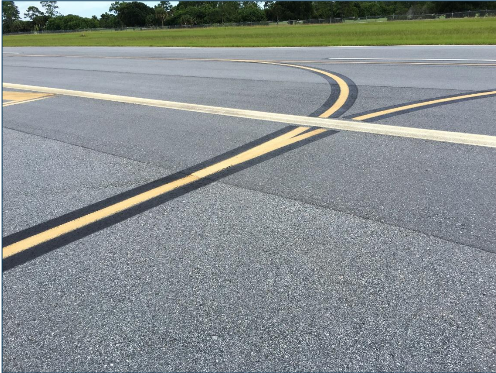
Taxiway C1, Section 605, Sample Unit 100 – Low Severity (57) Weathering
