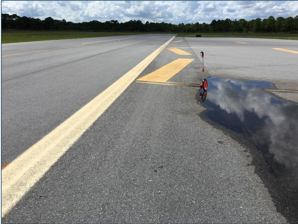
Runway 10-28, Section 6205, Sample Unit 106 – Low Severity (45) Depression, Low Severity (57) Weathering
