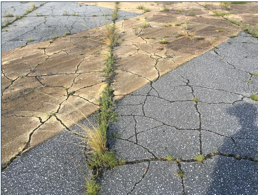
Apron AP, Section 4145, Sample Unit 400 – High Severity (43) Block Cracking, Medium Severity (41) Alligator Cracking, Low Severity (52) Raveling
