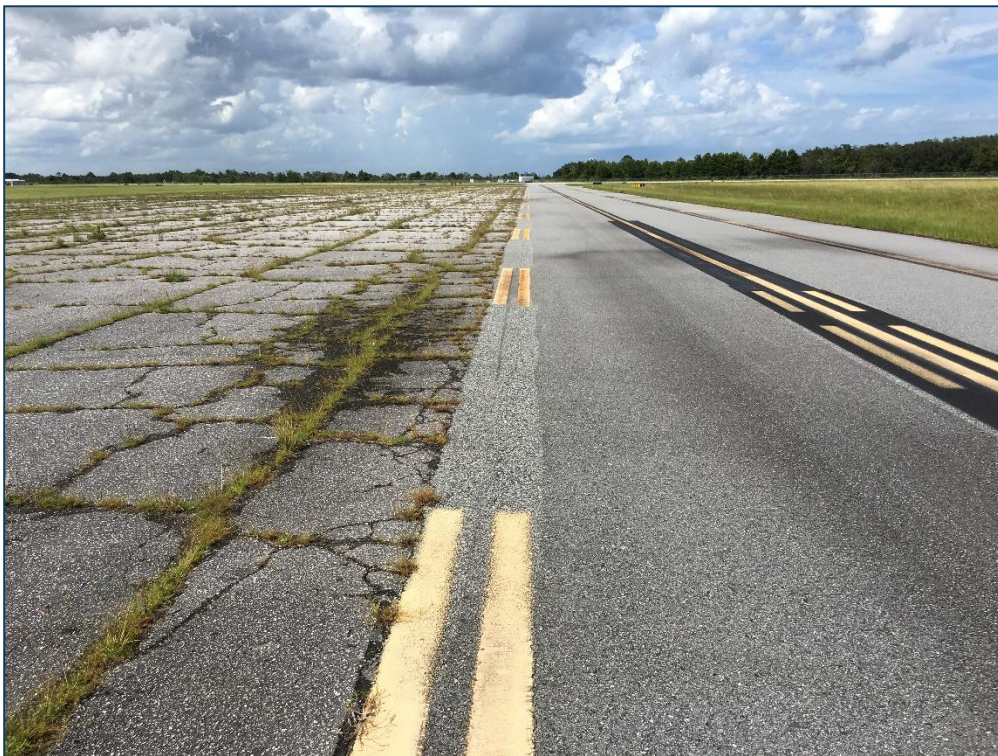
Taxiway B, Section 110, Sample Unit 101 – Low Severity (48) Longitudinal and Transverse Cracking, Low Severity (52) Raveling, Low Severity (57) Weathering
