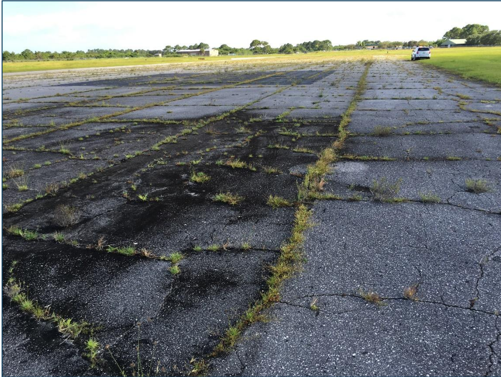
Apron AP, Section 4130, Sample Unit 104 – High Severity (43) Block Cracking, Low Severity (52) Raveling
