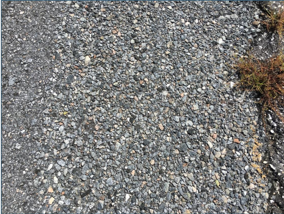
Taxiway B, Section 110, Sample Unit 101 – Low Severity (52) Raveling, Low Severity (57) Weathering
