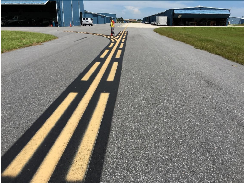
Taxiway D, Section 505, Sample Unit 101 – Low Severity (48) Longitudinal and Transverse Cracking, Low Severity (57) Weathering
