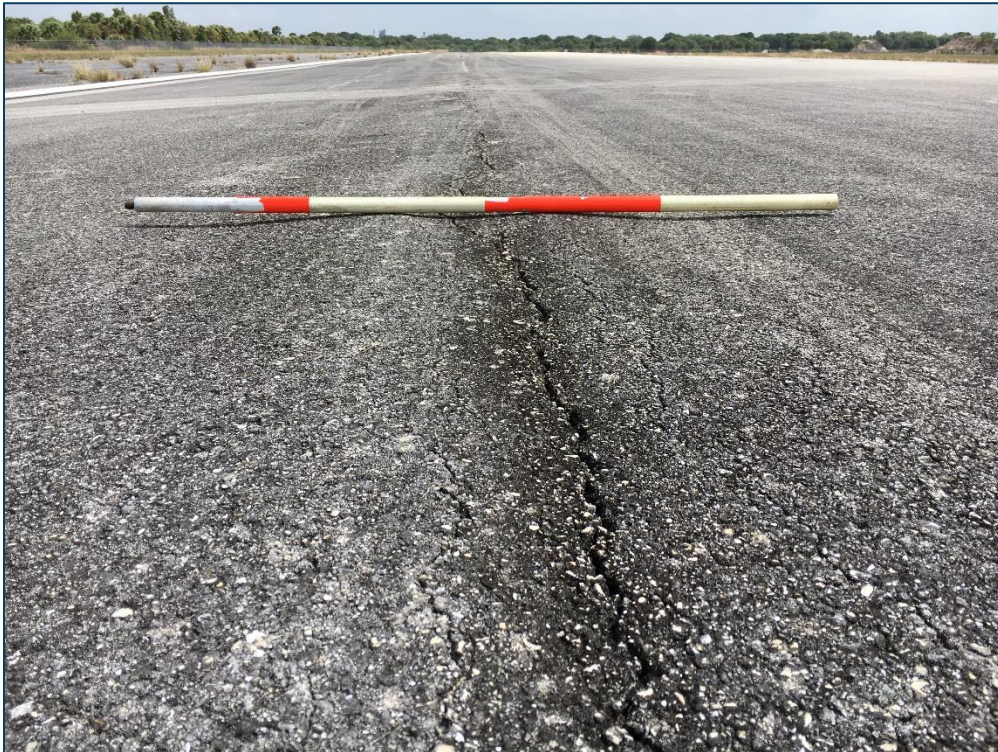
Runway 14-32, Section 6205, Sample Unit 333 – Low and Medium Severity (48) Longitudinal and Transverse Cracking, Low Severity (52) Raveling, Low Severity (56) Swelling, Low Severity (57) Weathering
