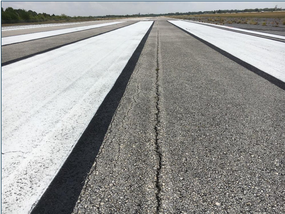
Runway 14-32, Section 6205, Sample Unit 378 – Low Severity (48) Longitudinal and Transverse Cracking, Low Severity (57) Weathering, Low Severity (56) Swelling, Low Severity (57) Weathering
