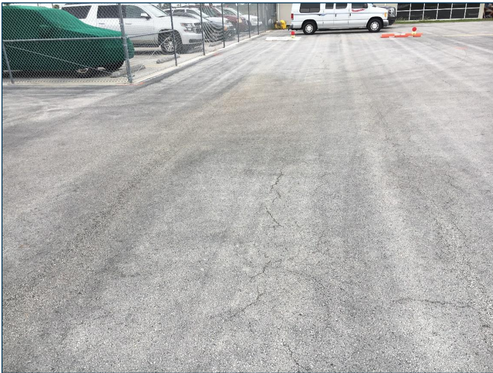
Apron, Section 4110, Sample Unit 70 – Low Severity (48) Longitudinal and Transverse Cracking, Low Severity (52) Raveling, Low Severity (57) Weathering
