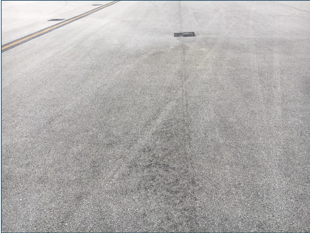
Apron, Section 4105, Sample Unit 500 – Low Severity (57) Weathering
