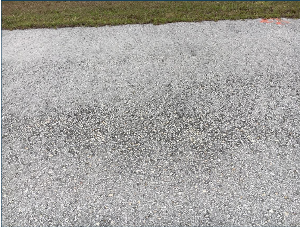
Taxiway A, Section 110, Sample Unit 212 – Low Severity (57) Weathering
