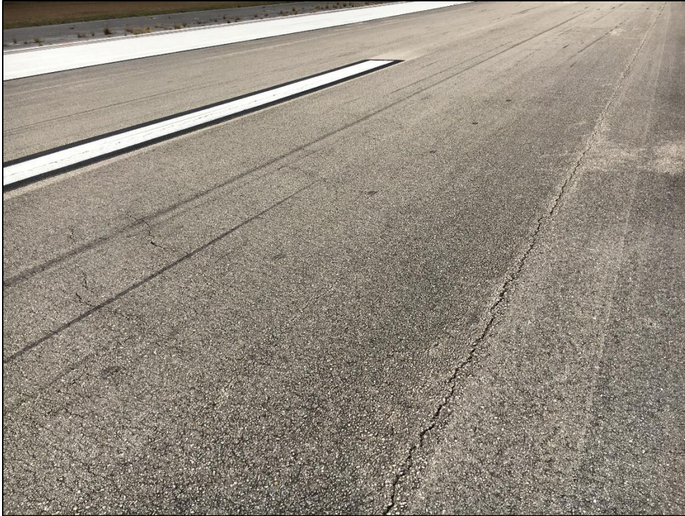
Runway 14-32, Section 6205, Sample Unit 357 – Low Severity (48) Longitudinal and Transverse Cracking, Low Severity (52) Raveling, Low Severity (57) Weathering
