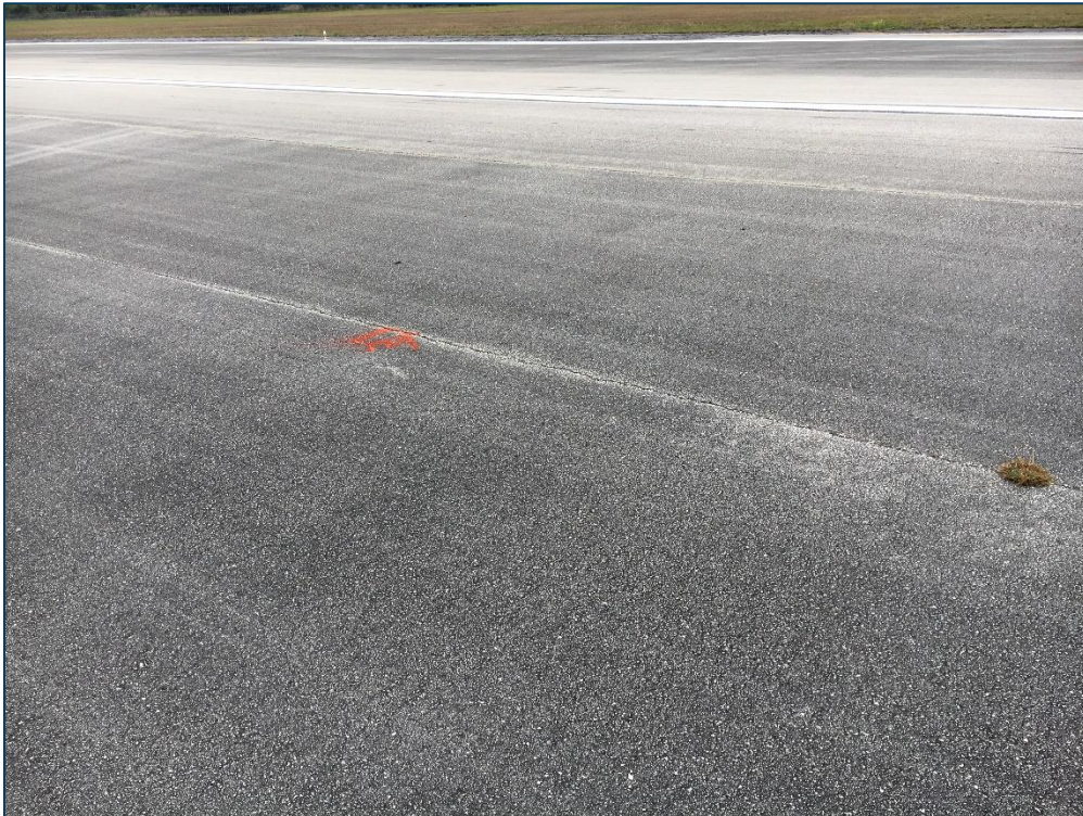
Runway 5-23, Section 6107, Sample Unit 124 – Low and Medium Severity (48) Longitudinal and Transverse Cracking, Low Severity (57) Weathering
