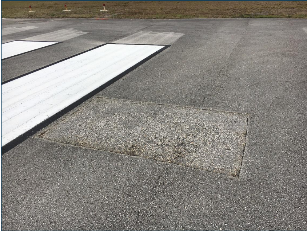
Runway 5-23, Section 6105, Sample Unit 300 – Low Severity (50) Patching, Medium Severity (50) Patching, Low Severity (52) Raveling, Low Severity (57) Weathering
