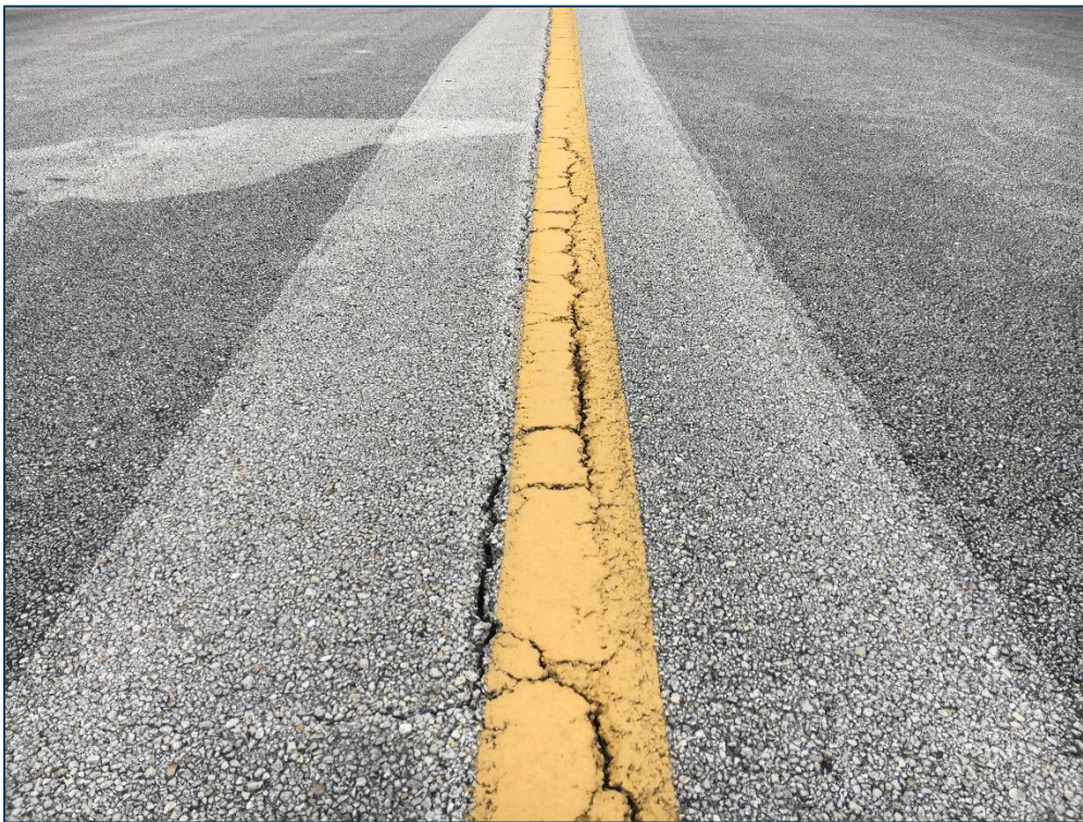
Taxiway B, Section 205, Sample Unit 142 – Low and Medium Severity (48) Longitudinal and Transverse Cracking, Low Severity (52) Raveling, Low Severity (56) Swelling, Low Severity (57) Weathering
