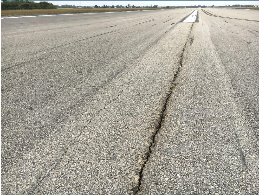
Runway 5-23, Section 6105, Sample Unit 335 – Low Severity (48) Longitudinal and Transverse Cracking, Low Severity (56) Swelling, Low Severity (57) Weathering
