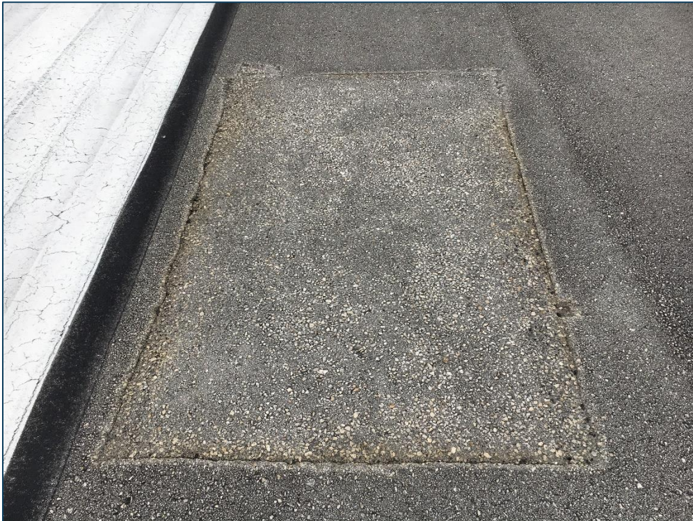
Runway 5-23, Section 6105, Sample Unit 349 – Medium Severity (50) Patching, Low Severity (52) Raveling, Low Severity (57) Weathering
