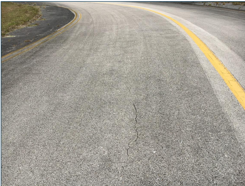
Taxiway B, Section 205, Sample Unit 105 – Low Severity (48) Longitudinal and Transverse Cracking, Low Severity (52) Raveling, Low Severity (57) Weathering
