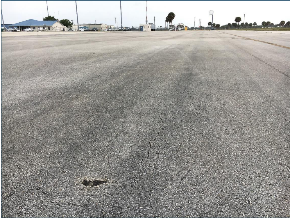
Apron, Section 4110, Sample Unit 604 – Low Severity (48) Longitudinal and Transverse Cracking, Low Severity (52) Raveling, Low Severity (57) Weathering
