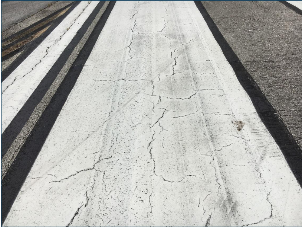
Runway 14-32, Section 6205, Sample Unit 301 – Low Severity (43) Block Cracking, Low Severity (48) Longitudinal and Transverse Cracking, Low Severity (52) Raveling, Medium Severity (52) Raveling
