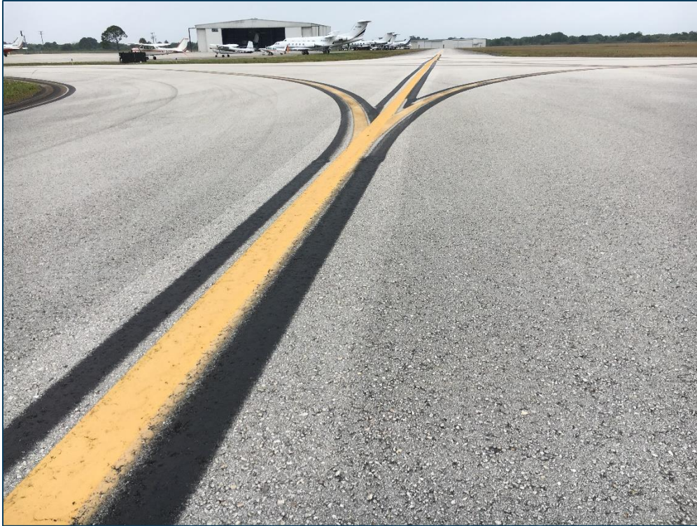
Taxiway B, Section 210, Sample Unit 126 – Low Severity (57) Weathering
