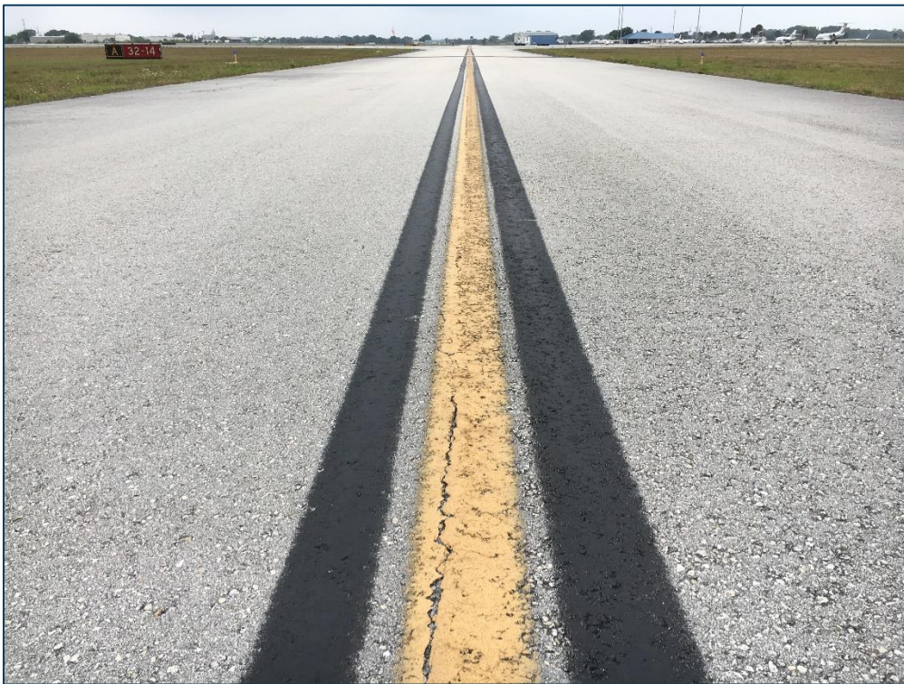
Taxiway A, Section 110, Sample Unit 231 – Low Severity (48) Longitudinal and Transverse Cracking, Low Severity (57) Weathering
