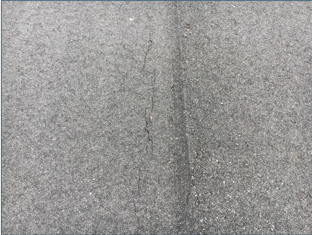
Runway 1-19, Section 6115, Sample Unit 182 – Low Severity (48) Longitudinal and Transverse Cracking, Low Severity (57) Weathering
