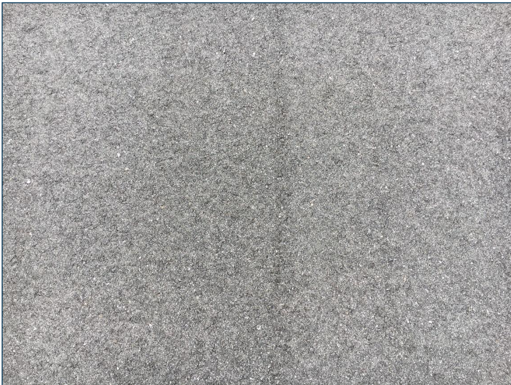
Runway 1-19, Section 6115, Sample Unit 194 – Low Severity (57) Weathering
