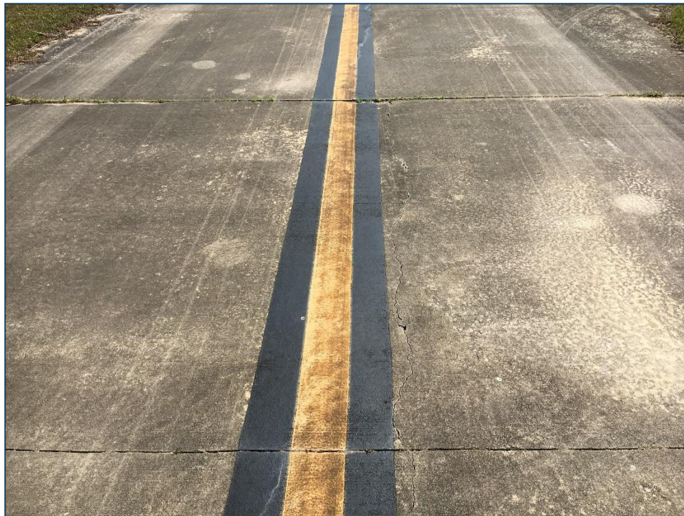
T-Hangar Taxilane, Section 4110, Sample Unit 300 – Low Severity (63) Longitudinal, Transverse, and Diagonal Cracking, High Severity (65) Joint Seal Damage.
