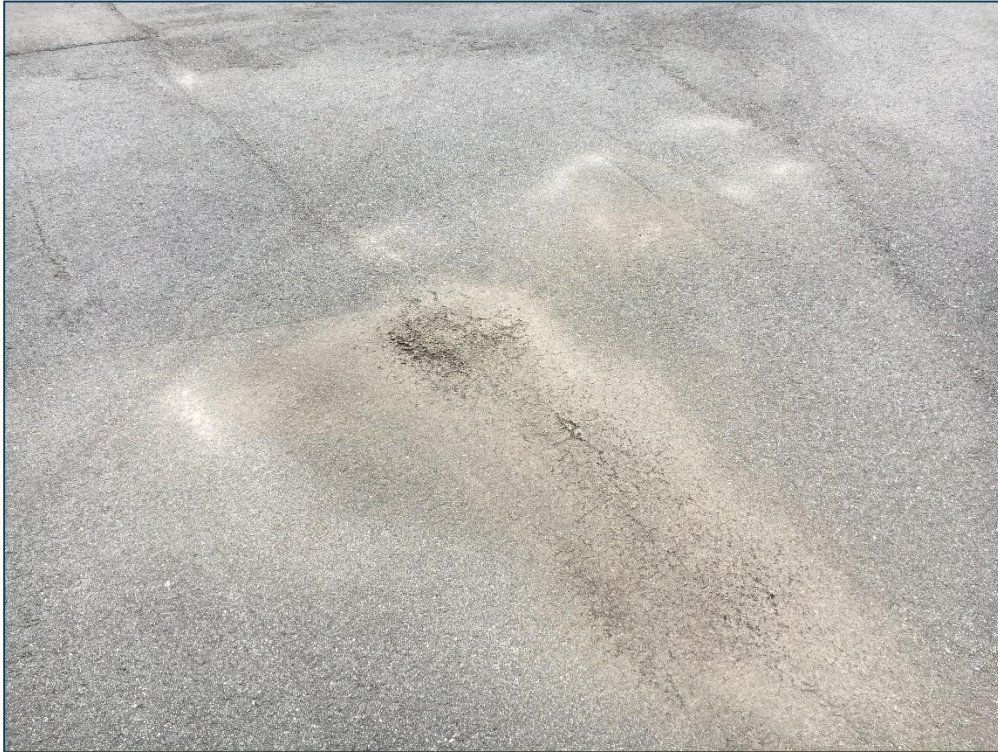
Taxiway A3, Section 305, Sample Unit 100 – Low Severity (45) Depression, Low Severity (57) Weathering,
