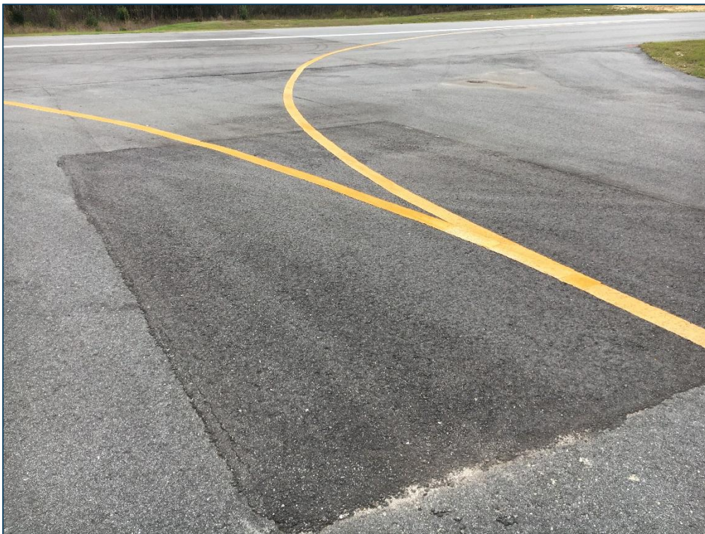
Taxiway A3, Section 305, Sample Unit 100 – Low Severity (50) Patching, Low Severity (57) Weathering
