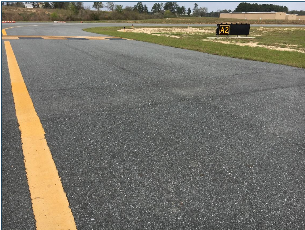
Taxiway A2, Section 205, Sample Unit 100 – Low Severity (50) Patching, Low Severity (57) Weathering
