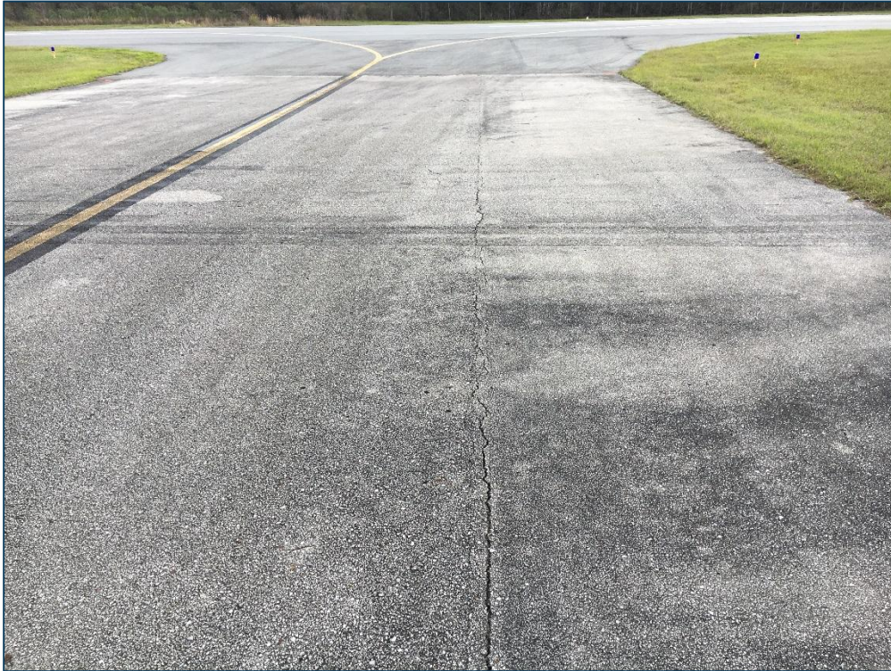
Taxiway A1, Section 105, Sample Unit 100 – Low Severity (48) Longitudinal and Transverse Cracking, Low Severity (52) Raveling, Low Severity (57) Weathering
