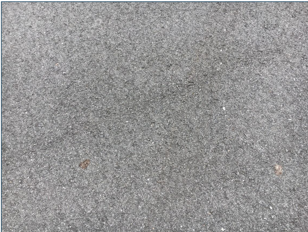
Taxiway A, Section 120, Sample Unit 106 – Low Severity (57) Weathering
