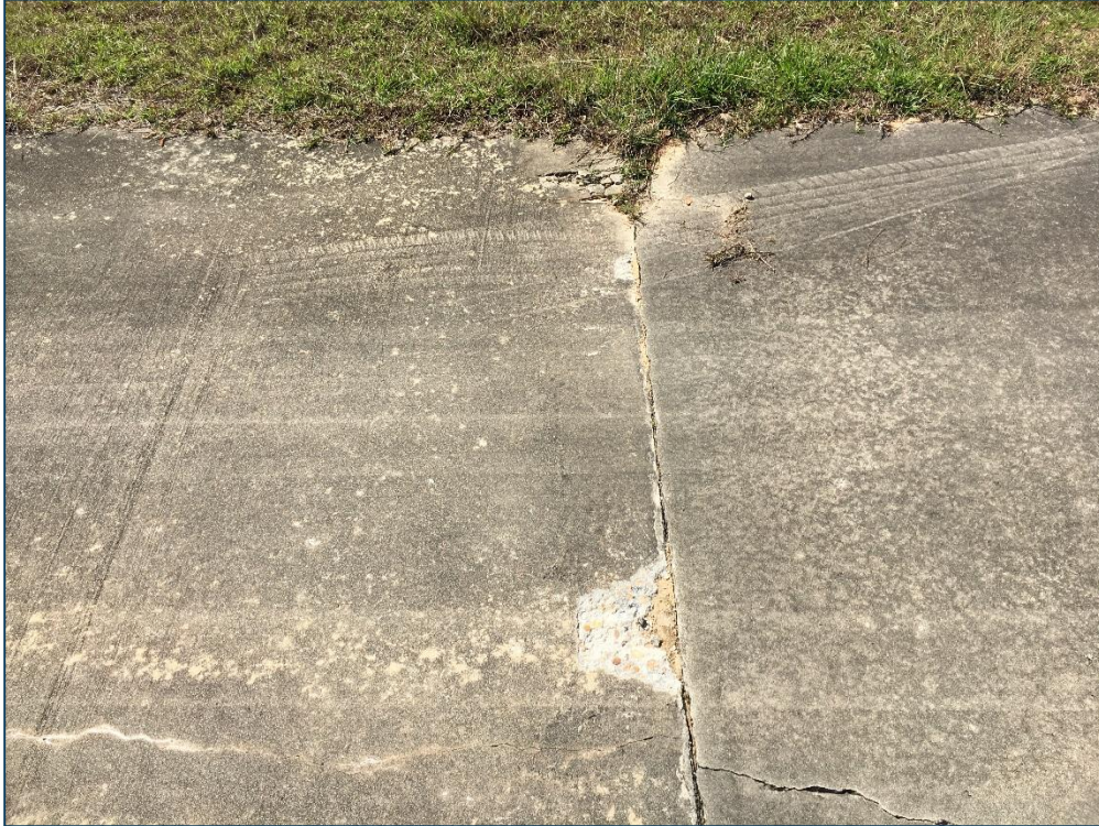
T-Hangar Taxilane, Section 4110, Sample Unit 300 – Low Severity (63) Longitudinal, Transverse, and Diagonal Cracking, Low Severity (74) Joint Spalling, High Severity (65) Joint Seal Damage.
