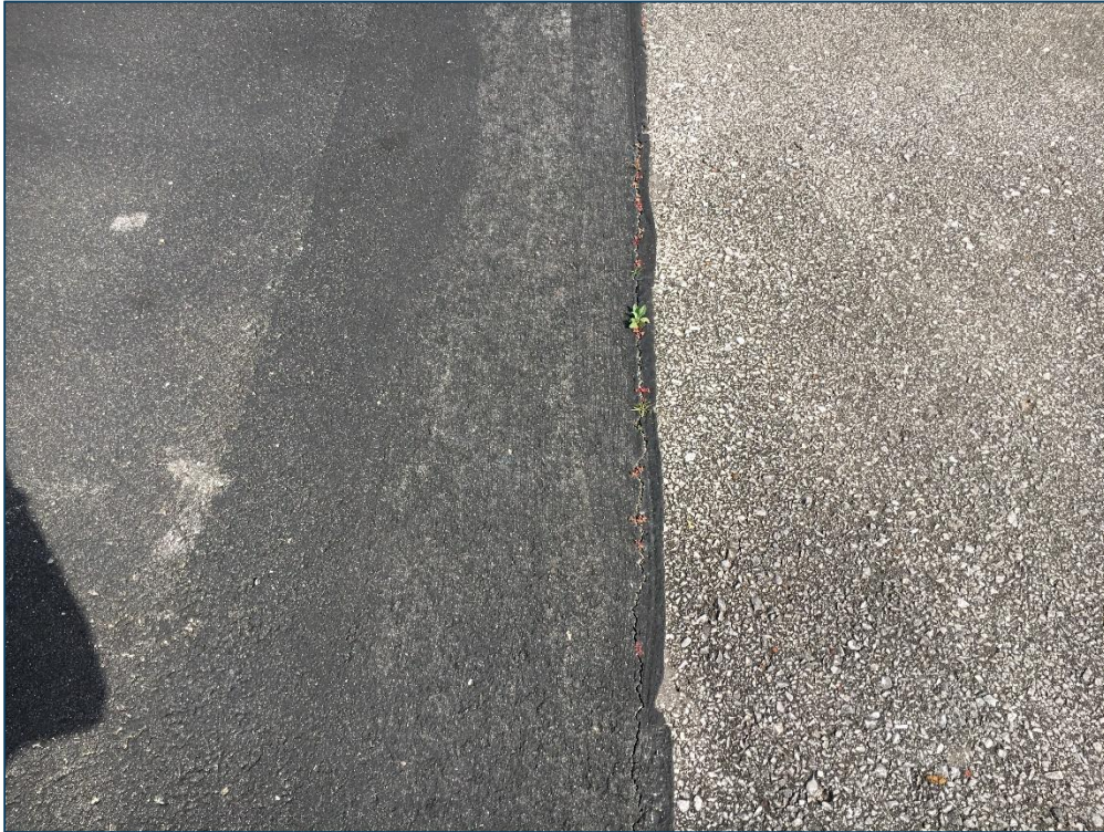
Apron, Section 4105, Sample Unit 100 - Low Severity (48) Longitudinal and Transverse Cracking, Low Severity (57) Weathering
