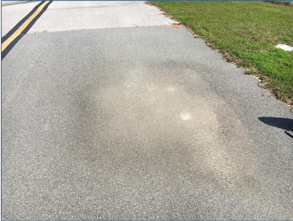
T-Hangar Taxilane, Section 4125, Sample Unit 106 – Low Severity (45) Depression, Low Severity (57) Weathering
