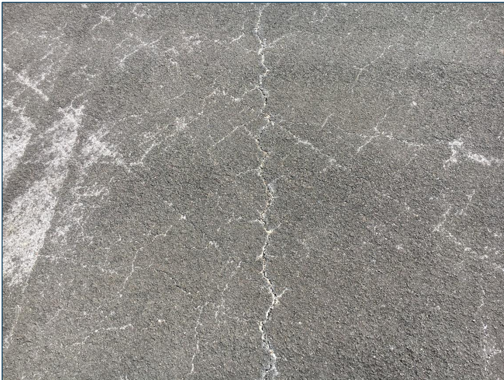
Apron, Section 4115, Sample Unit 303 - Low Severity (48) Longitudinal and Transverse Cracking, Low Severity (52) Raveling, Low Severity (57) Weathering
