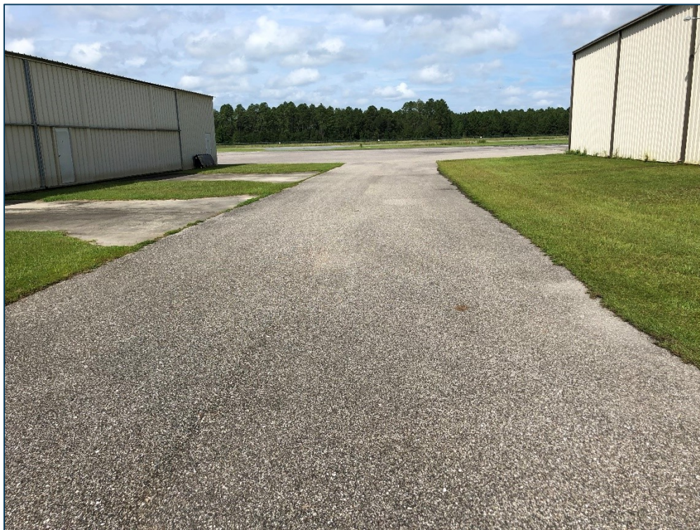
AP T-HANG, Section 805, Sample Unit 101 - Low Severity (52) Raveling and Low Severity (57) Weathering
