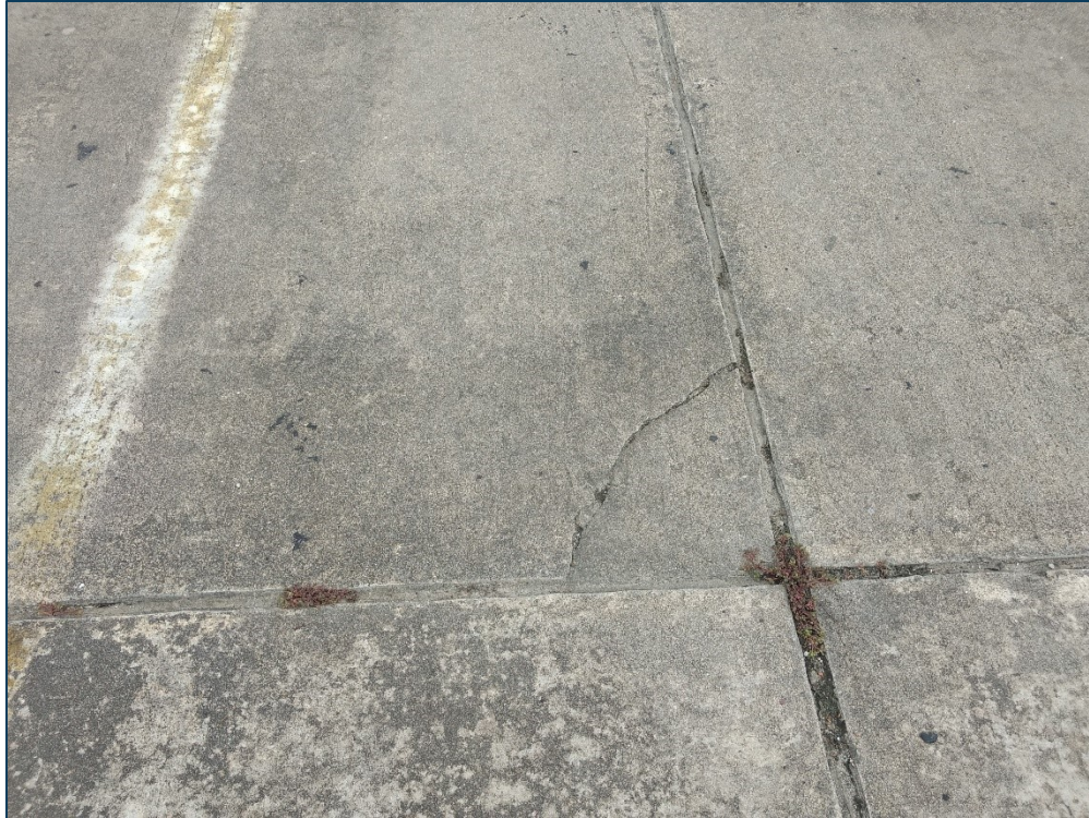
AP GA, Section 4105, Sample Unit 214 - Low Severity (65) Joint Seal Damage and Medium Severity (75) Corner Spall
