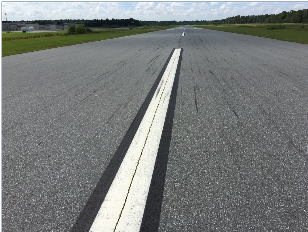
RW 18-36, Section 6105, Sample Unit 160 - Low Severity (48) Longitudinal & Transverse Cracking, Low Severity (52) Raveling, and Low Severity (57) Weathering
