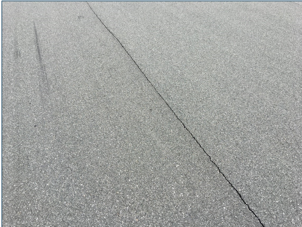
RW 18-36, Section 6105, Sample Unit 148 - Low Severity (48) Longitudinal & Transverse Cracking and Low Severity (57) Weathering
