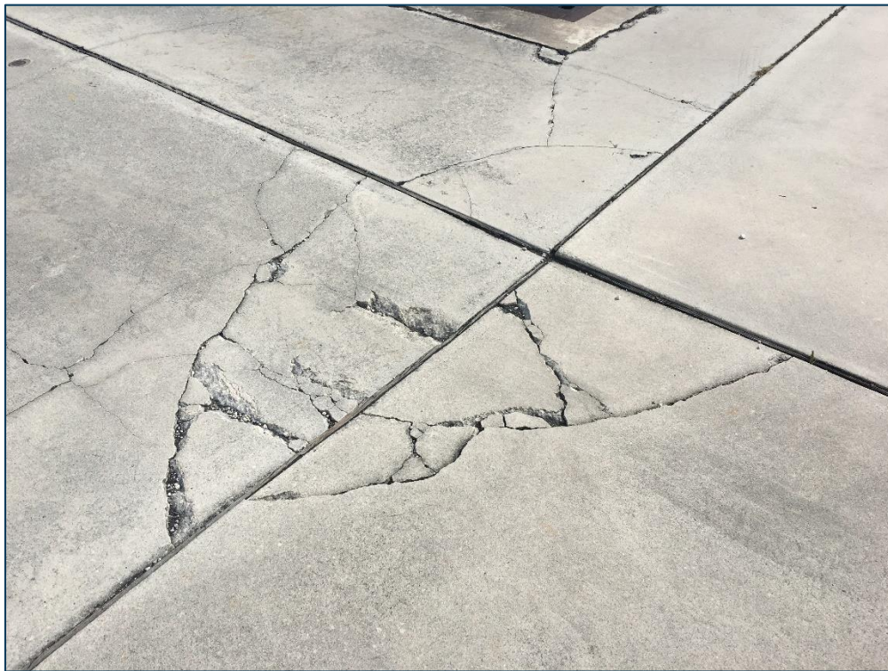
AP CENTER, Section 4235, Sample Unit 100 - High Severity (62) Corner Break and Medium Severity (65) Joint Seal Damage
