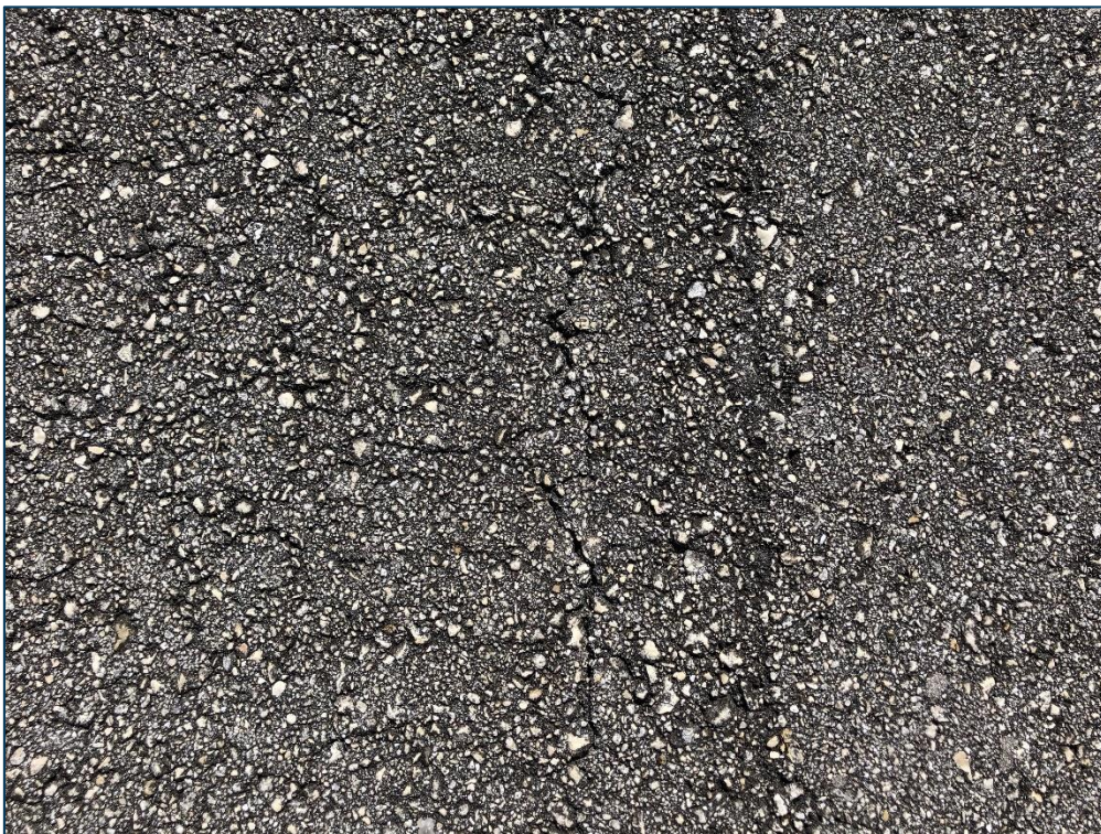
RW 12L-30R, Section 6220, Sample Unit 117 - Low Severity (48) Longitudinal & Transverse Cracking, Low Severity (52) Raveling, and Low Severity (57) Weathering
