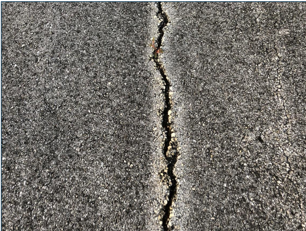
RW 4-22, Section 6310, Sample Unit 149 - Medium Severity (48) Longitudinal & Transverse Cracking and Low Severity (57) Weathering
