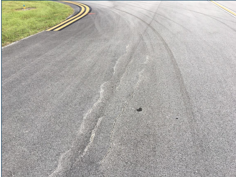
TWA, Section 125, Sample Unit 126 - Low Severity (41) Alligator Cracking, Low Severity (48) Longitudinal & Transverse Cracking, and Low Severity (57) Weathering
