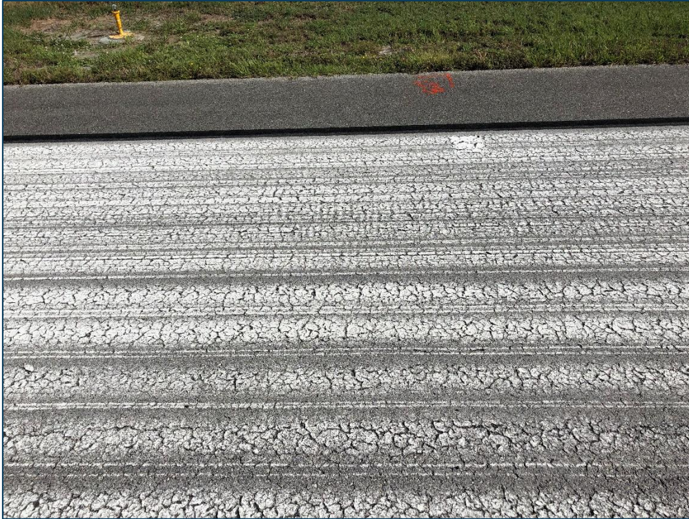
RW 12L-30R, Section 6215, Sample Unit 123 - Medium Severity (52) Raveling
