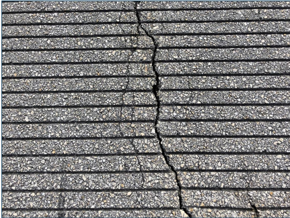
RW 12R-30L, Section 6110, Sample Unit 195 - Low Severity (41) Alligator Cracking and Medium Severity (57) Weathering
