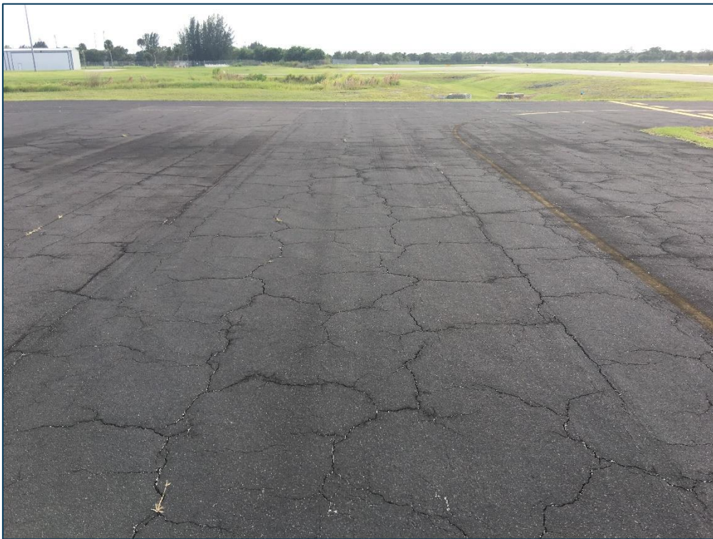
AP SW, Section 4105, Sample Unit 100 – Low and Medium Severity (43) Block Cracking and Medium Severity (52) Raveling
