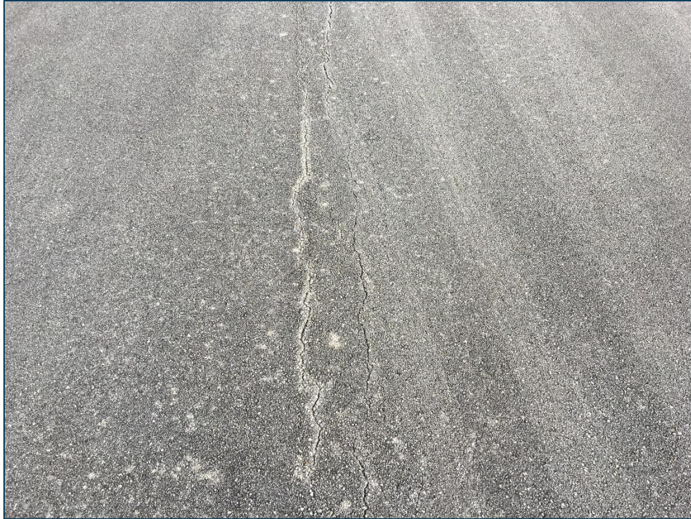
TWC3, Section 350, Sample Unit 201 - Low Severity (41) Alligator Cracking, Low Severity (52) Raveling, and Low Severity (57) Weathering
