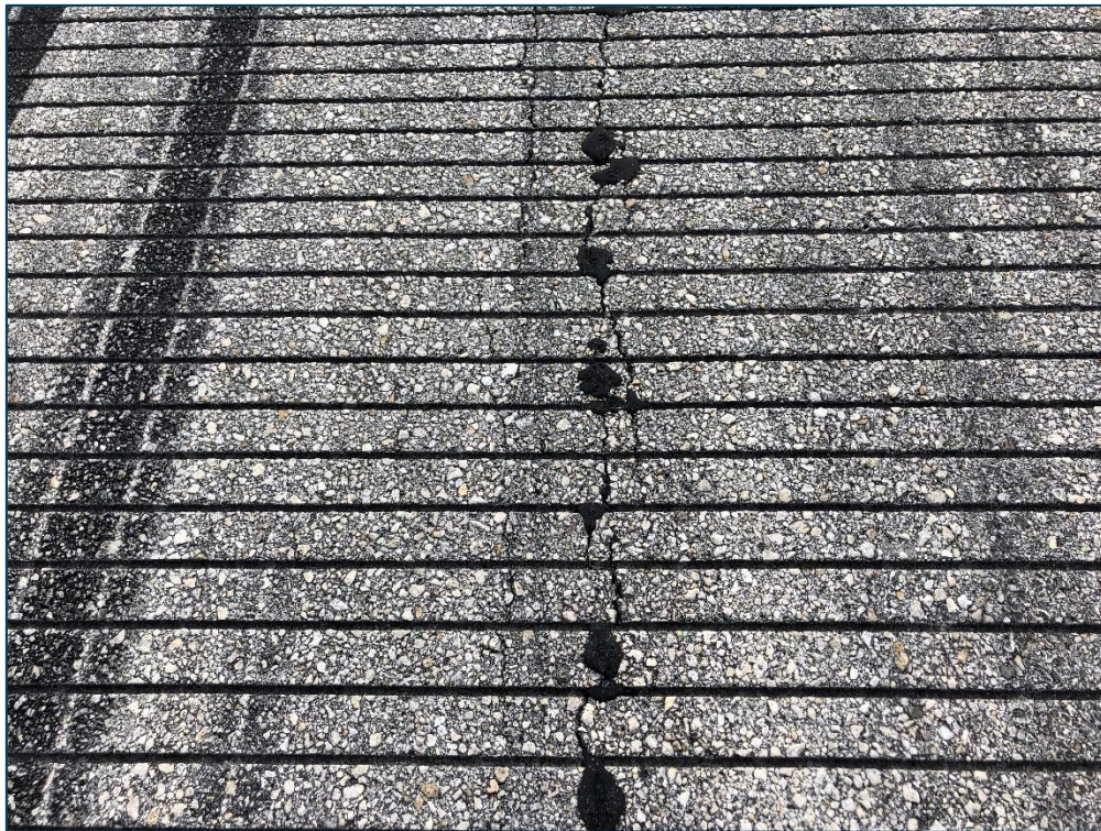
RW 12R-30L, Section 6110, Sample Unit 214 - Low Severity (41) Alligator Cracking, (42) Bleeding, Low Severity (52) Raveling, and Medium Severity (57) Weathering
