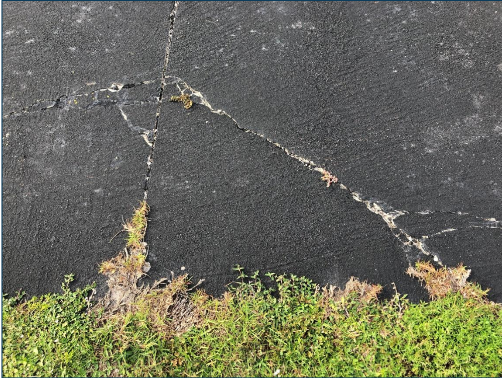
AP SW, Section 4115, Sample Unit 202 - Medium Severity (62) Corner Break and High Severity (65) Joint Seal Damage
