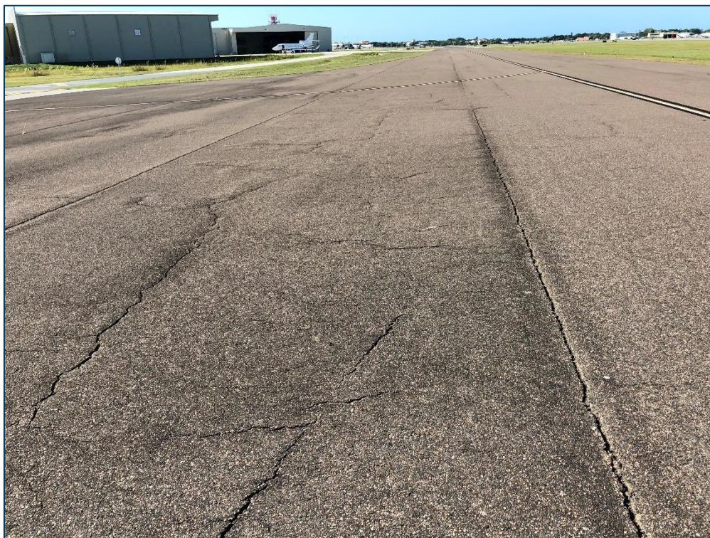
TWB, Section 210, Sample Unit 111 - Low Severity (43) Block Cracking, Low Severity (56) Swelling, and Low Severity (57) Weathering
