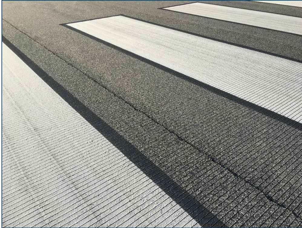
RW 14-32, Section 6105, Sample Unit 326 -Medium Severity (48) Longitudinal & Transverse Cracking and Low Severity (57) Weathering
