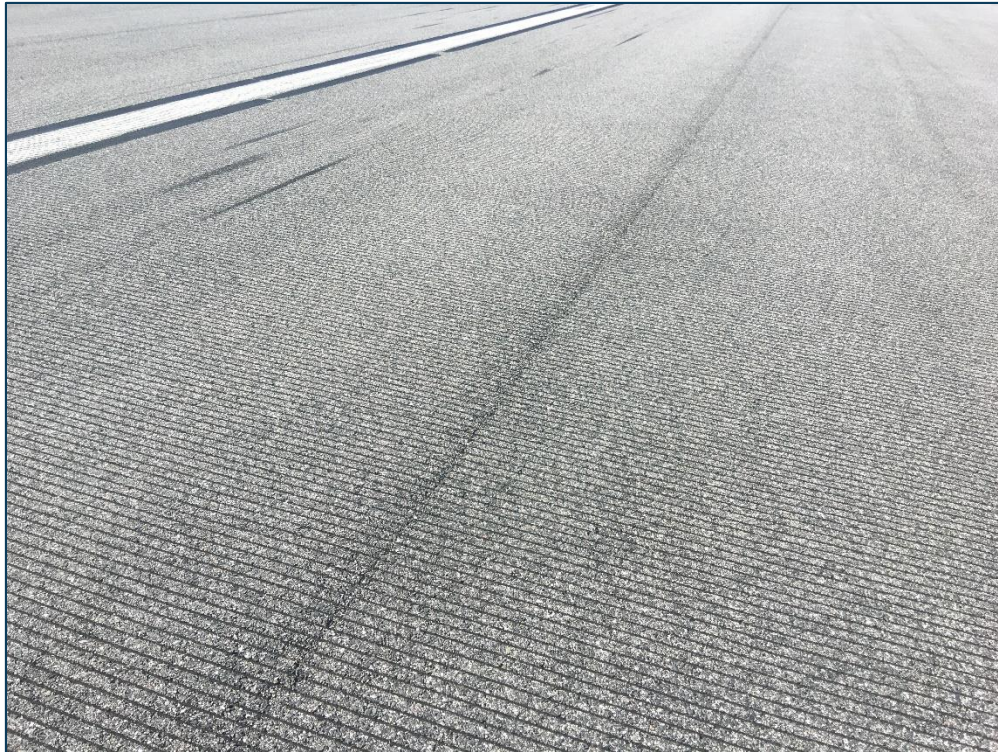
RW 4-22, Section 6205, Sample Unit 306 - Low Severity (48) Longitudinal & Transverse Cracking and Low Severity (57) Weathering
