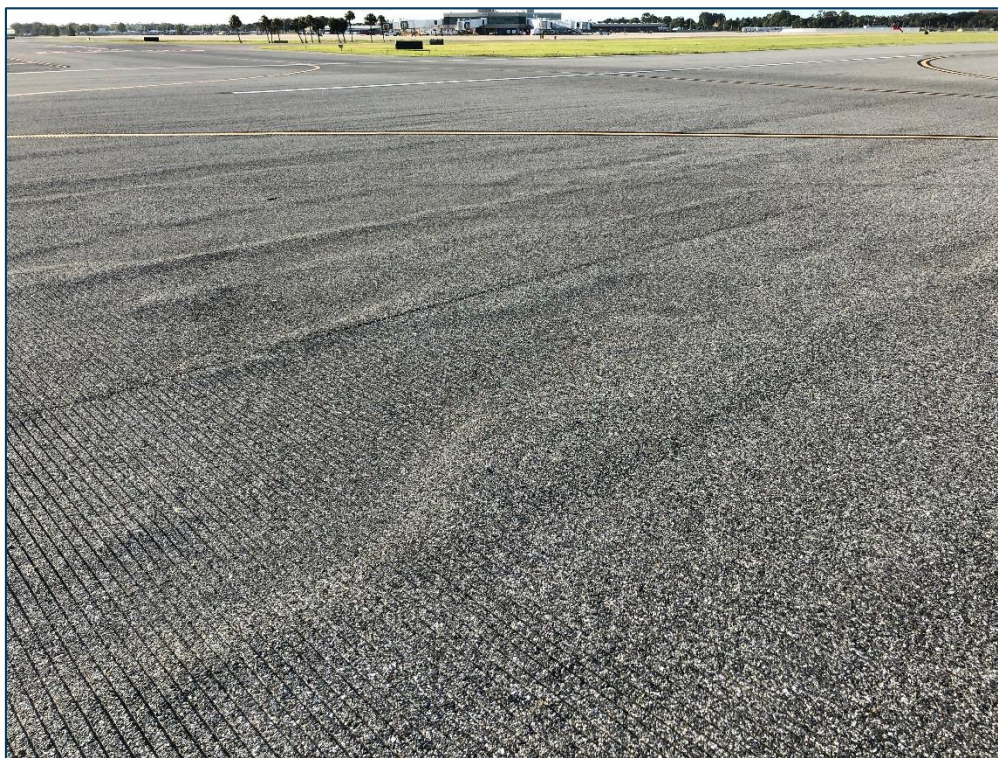
RW 4-22, Section 6210, Sample Unit 164 - Low Severity (48) Longitudinal & Transverse Cracking, Low Severity (56) Swelling, and Low Severity (57) Weathering
