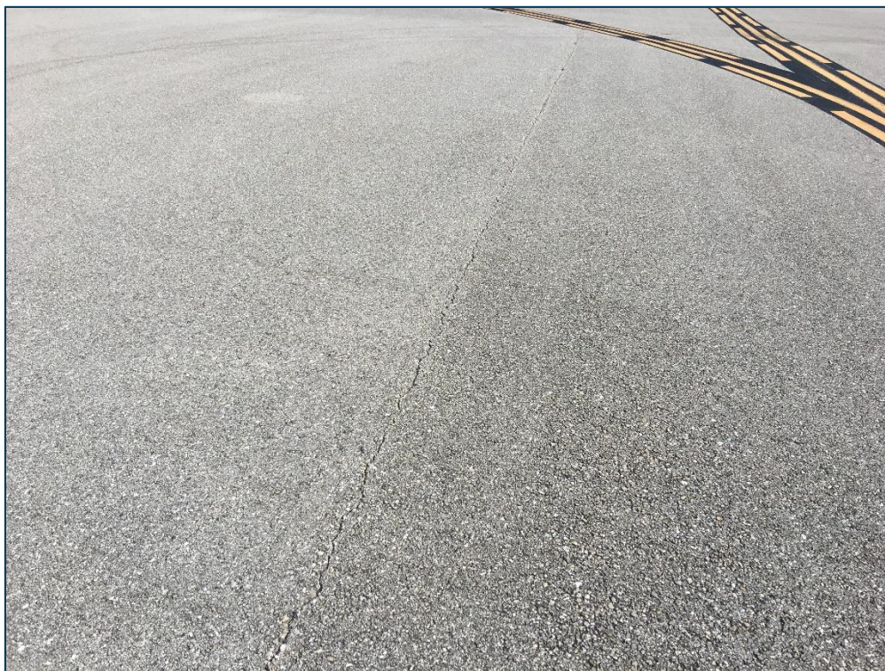
TWD, Section 430, Sample Unit 144 - Low Severity (48) Longitudinal & Transverse Cracking and Low Severity (57) Weathering
