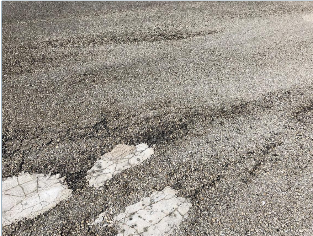
TWC, Section 305, Sample Unit 159 - Medium Severity (41) Alligator Cracking, Low Severity (48) Longitudinal & Transverse Cracking, High Severity (50) Patching, Low and Medium Severity (52) Raveling
