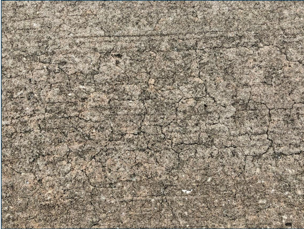
AP TERM, Section 4110, Sample Unit 161 - (73) Shrinkage Cracking
