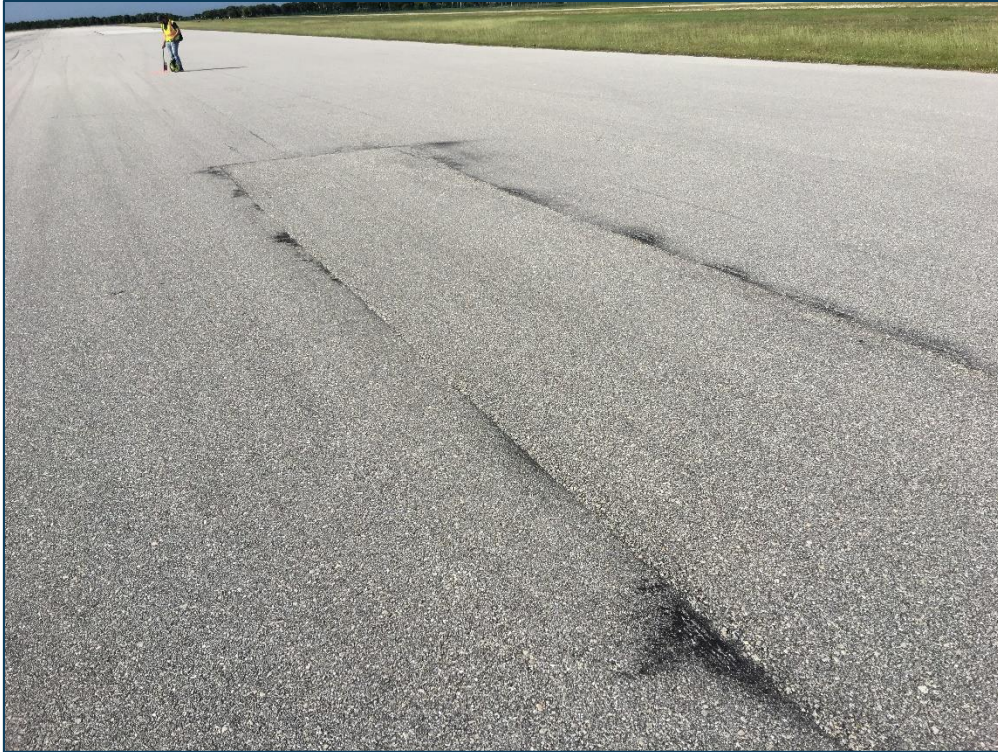
RW 5-23, Section 6205, Sample Unit 115 - Low Severity (50) Patching, Low Severity (52) Raveling, and Low Severity (57) Weathering
