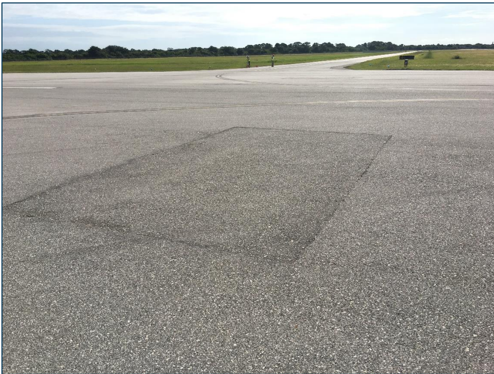
RW 5-23, Section 6240, Sample Unit 320 - Low Severity (50) Patching and Low Severity (57) Weathering
