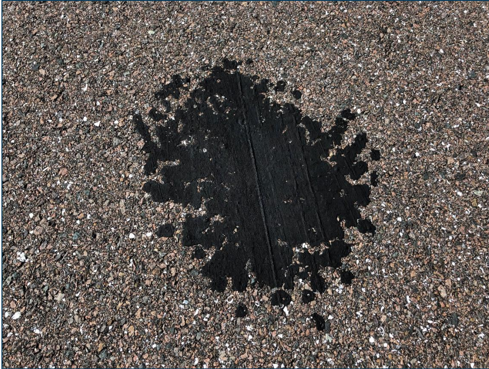
TWE, Section 515, Sample Unit 125 - (42) Bleeding and Low Severity (57) Weathering
