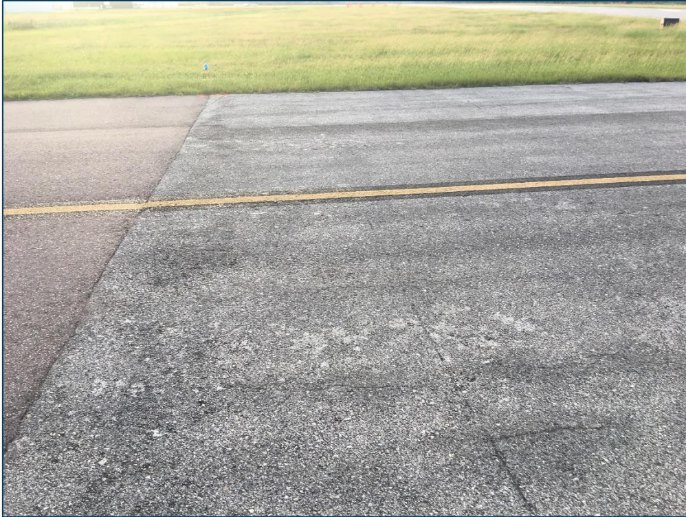
TW A, Section 125, Sample Unit 100 - Low Severity (48) Longitudinal & Transverse Cracking, Low Severity (52) Raveling, and Medium Severity (57) Weathering
