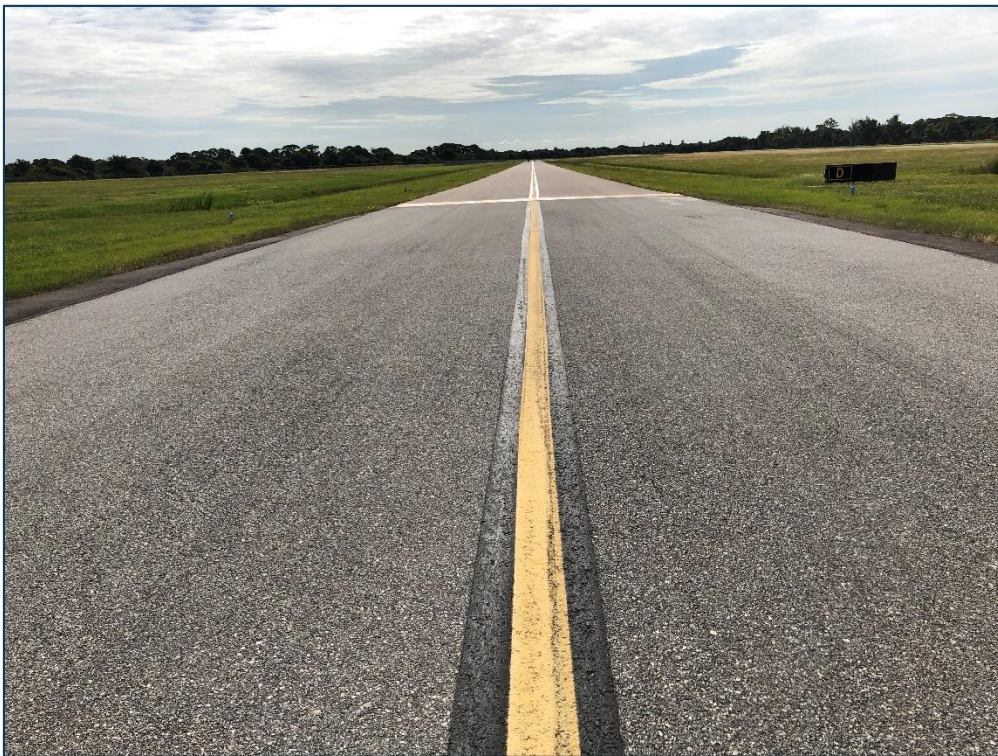
TW D, Section 410, Sample Unit 101 - Low Severity (57) Weathering
