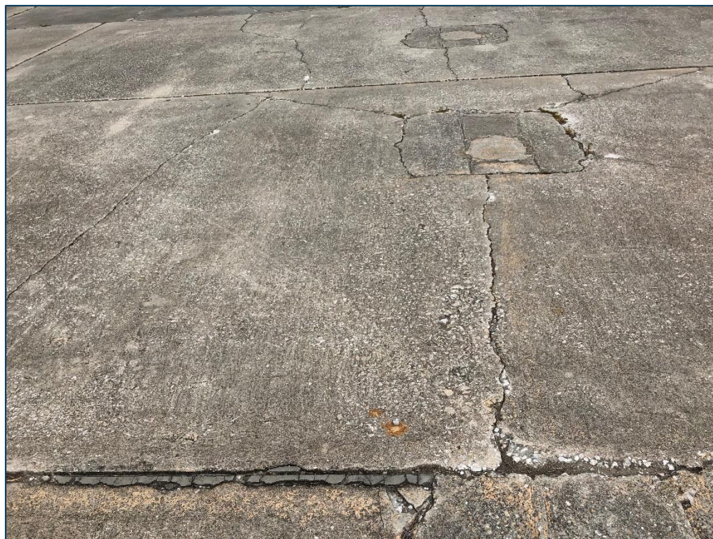
AP, Section 4115, Sample Unit300 - High Severity (65) Joint Seal Damage and Medium Severity (72) Shattered Slab
