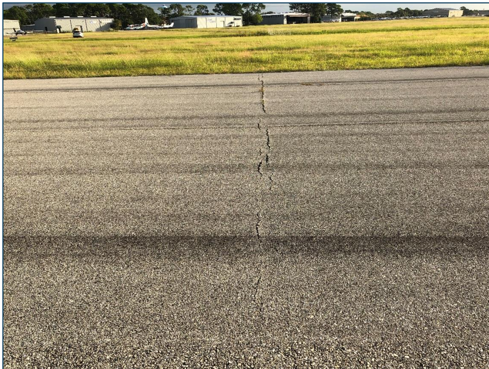
RW 13-31, Section 6125, Sample Unit 395 - Low and Medium Severity (47) Joint Reflection Cracking, Low Severity (48) Longitudinal & Transverse Cracking, Low Severity (52) Raveling, and Low Severity (57) Weathering
