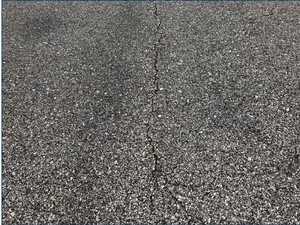
RW 13-31, Section 6110, Sample Unit 128 - Low Severity (48) Longitudinal & Transverse Cracking, Low Severity (56) Swelling, and Low Severity (57) Weathering
