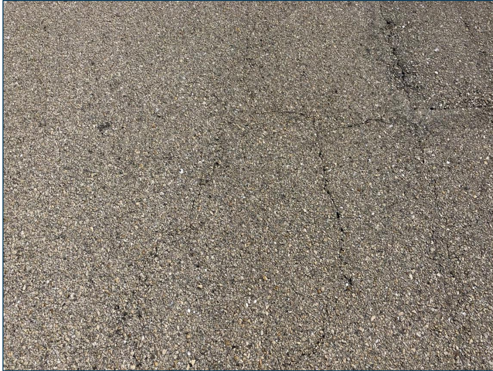
TW J, Section 535, Sample Unit 549 - Low Severity (48) Longitudinal & Transverse Cracking, Low Severity (52) Raveling, and Low Severity (57) Weathering
