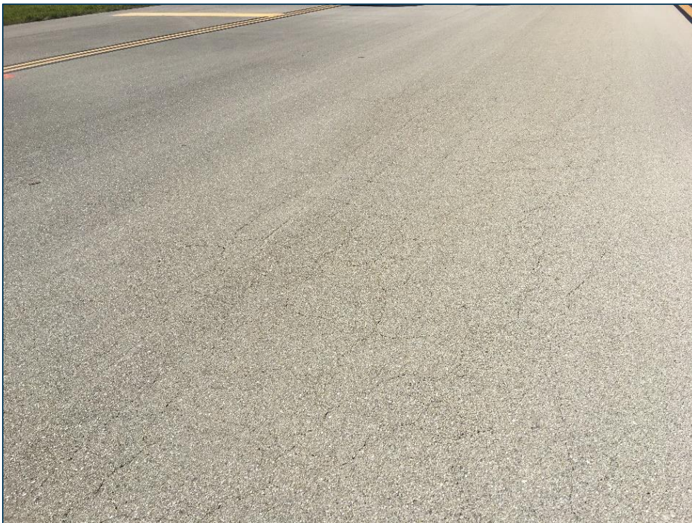
TW F, Section 250, Sample Unit 122 - Low Severity (41) Alligator Cracking, Low Severity (48) Longitudinal & Transverse Cracking, Low Severity (52) Raveling, and Low Severity (57) Weathering
