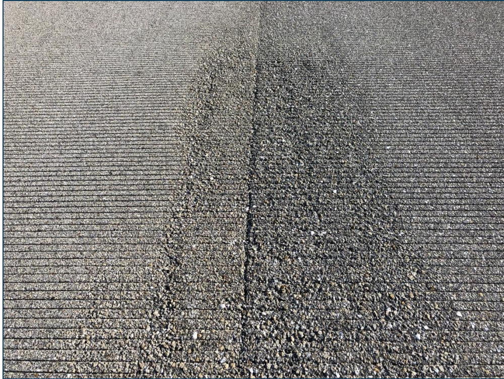
RW 6-24, Section 6104, Sample Unit 484 - Low Severity (48) Longitudinal & Transverse Cracking, Low Severity (52) Raveling, and Medium Severity (52) Raveling
