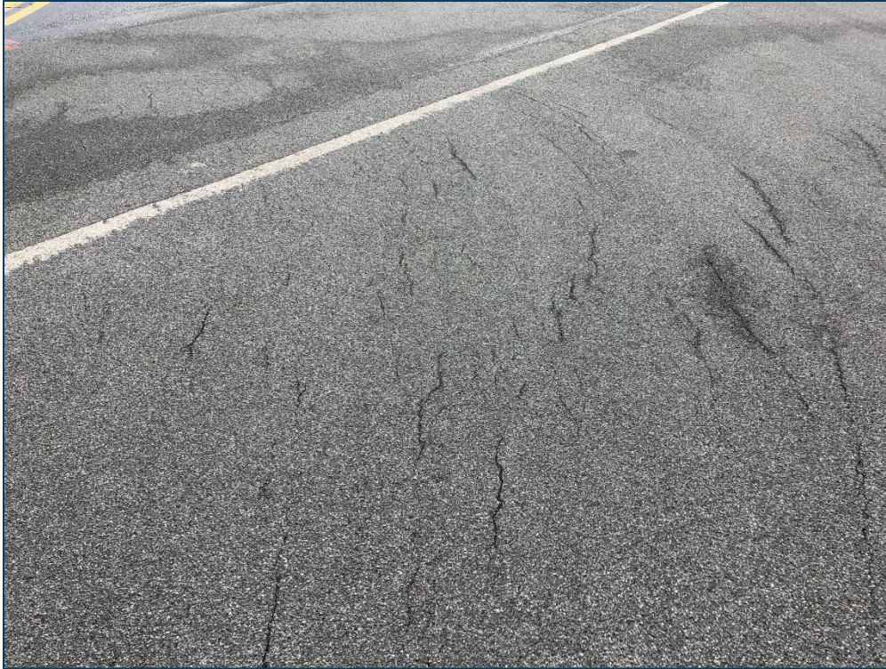
TW A, Section 109, Sample Unit 62 - Low Severity (48) Longitudinal & Transverse Cracking and Low Severity (57) Weathering
