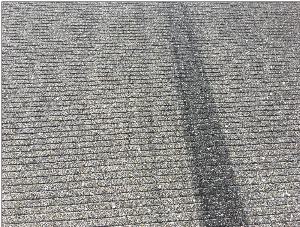
RW 6-24, Section 6105, Sample Unit 585 - Low Severity (48) Longitudinal & Transverse Cracking and Low Severity (57) Weathering
