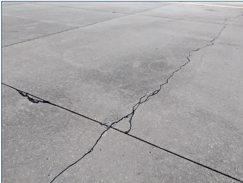
AP CARGO, Section 4110, Sample Unit 153 - Low Severity (63) Linear Cracking and Low Severity (74) Joint Spall
