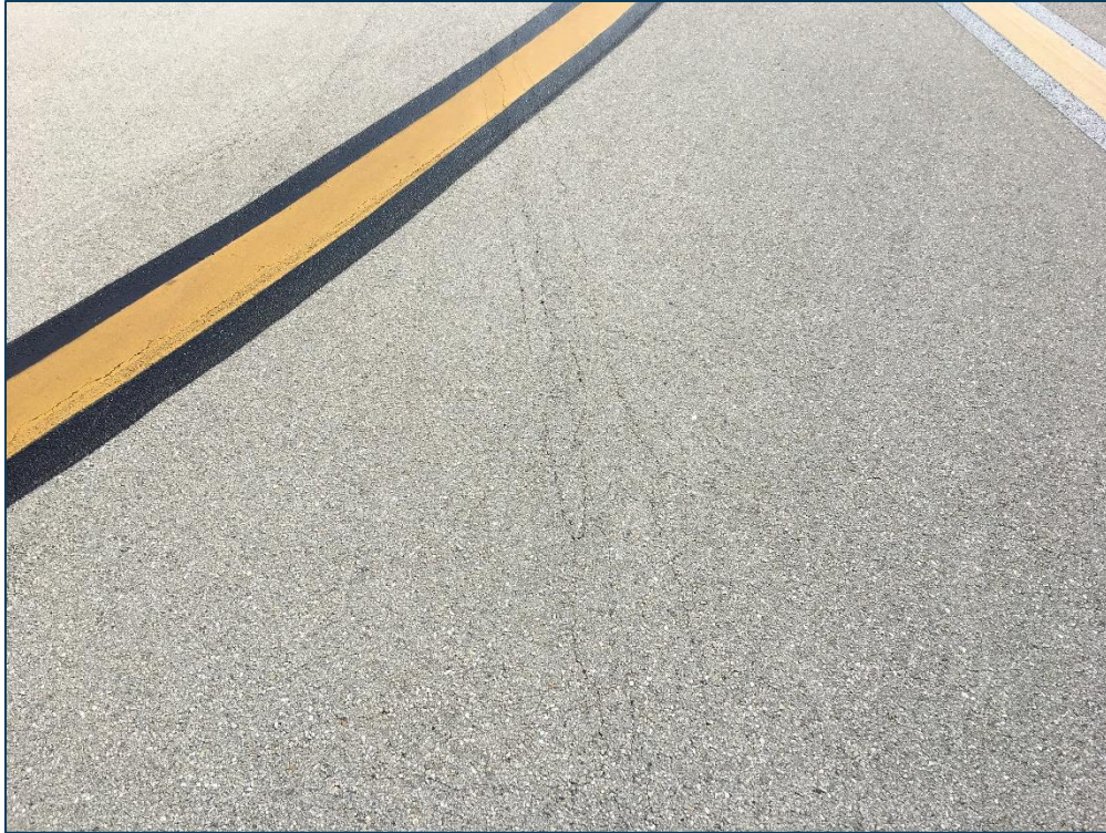
AP S, Section 4405, Sample Unit 119 - Low Severity (48) Longitudinal & Transverse Cracking and Low Severity (57) Weathering
