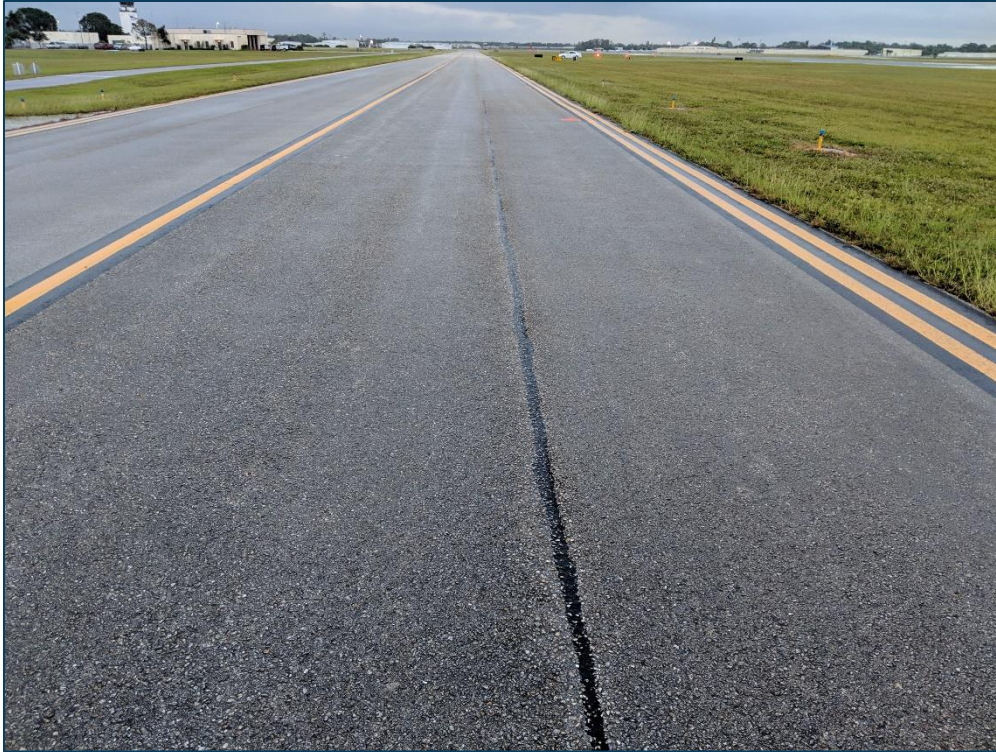
TW B, Section 205, Sample Unit 146 - Low Severity (48) Longitudinal & Transverse Cracking, Low Severity (52) Raveling, and Low Severity (57) Weathering
