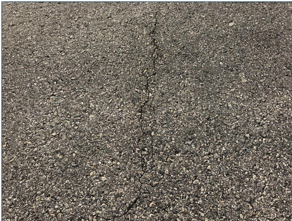
AP W, Section 4805, Sample Unit 302 - Low Severity (48) Longitudinal & Transverse Cracking, Low Severity (52) Raveling, and Low Severity (57) Weathering
