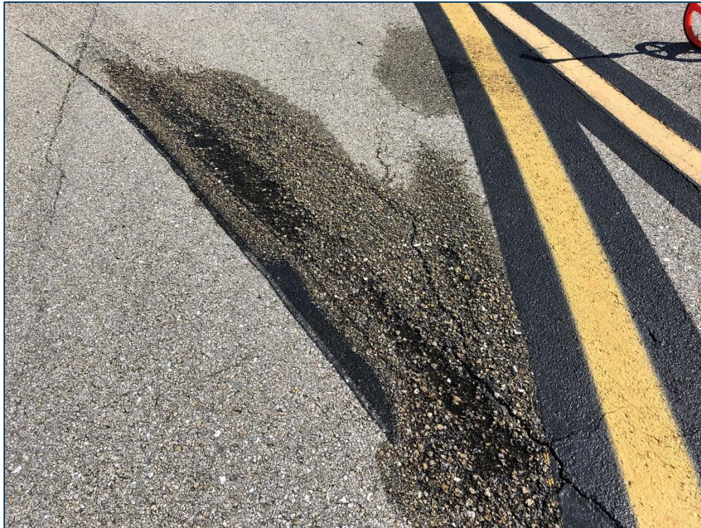
TW D, Section 136, Sample Unit 122 - Low and Medium Severity (48) Longitudinal & Transverse Cracking, Low and Medium Severity (52) Raveling
