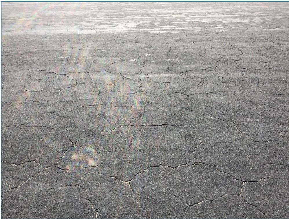
AP S, Section 4120, Sample Unit 103 - Medium Severity (43) Block Cracking and Low Severity (52) Raveling
