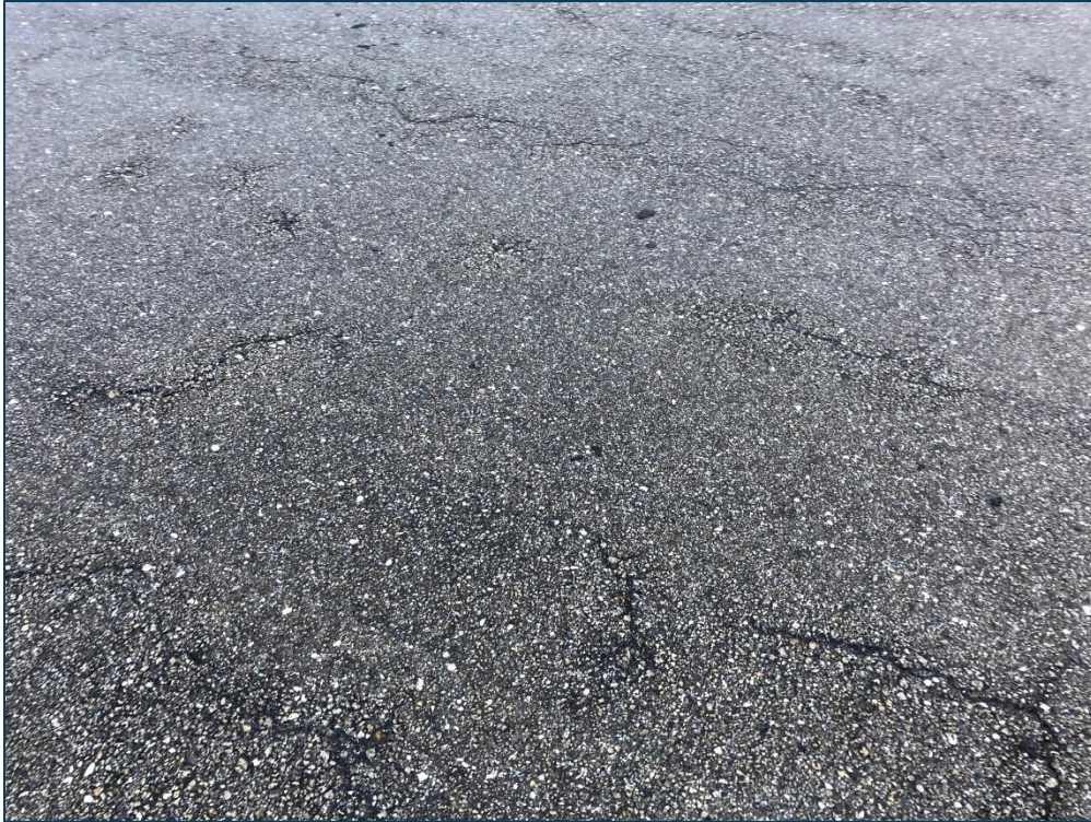
AP N, Section 4305, Sample Unit 502 - Low Severity (48) Longitudinal & Transverse Cracking, Low Severity (52) Raveling, and Low Severity (56) Swelling
