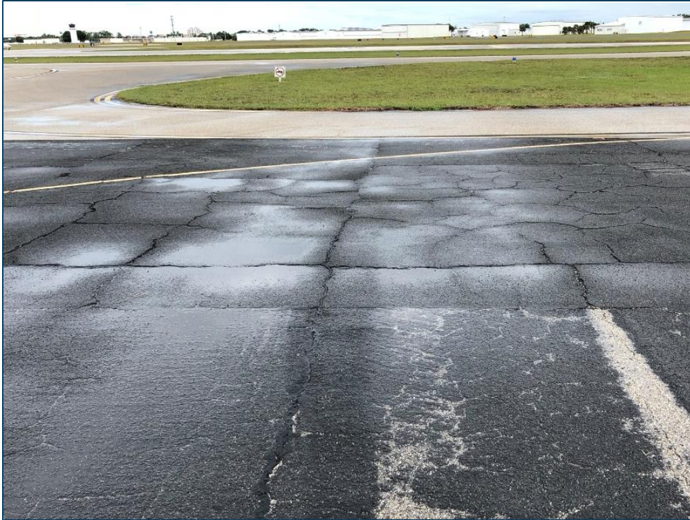
AP SE, Section 4415, Sample Unit 102 - Low and Medium Severity (43) Block Cracking and Low and Medium Severity (52) Raveling
