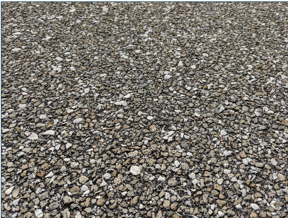
TW C, Section 305, Sample Unit 213 – Low and Medium Severity (57) Weathering
