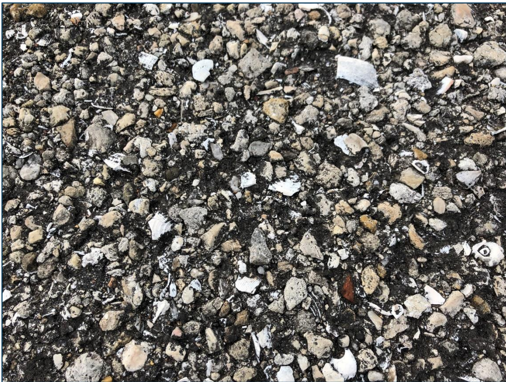
RW 9-27, Section 6305, Sample Unit 327 - Medium Severity (52) Raveling
