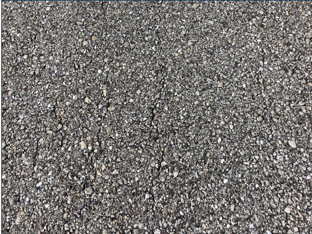
TWC, Section 310, Sample Unit 308 - Low Severity (41) Alligator Cracking, Low Severity (52) Raveling, and Low Severity (57) Weathering
