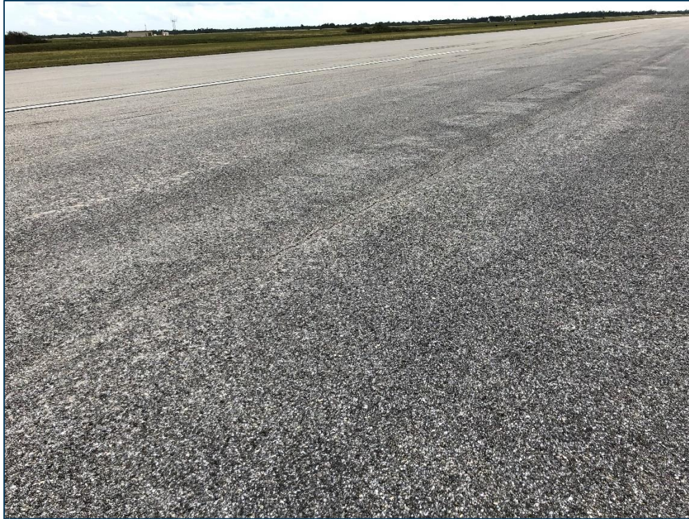
RW 15-33, Section 6210, Sample Unit 380 - Low Severity (48) Longitudinal & Transverse Cracking, Low Severity (52) Raveling, Low Severity (56) Swelling, and Medium Severity (57) Weathering
