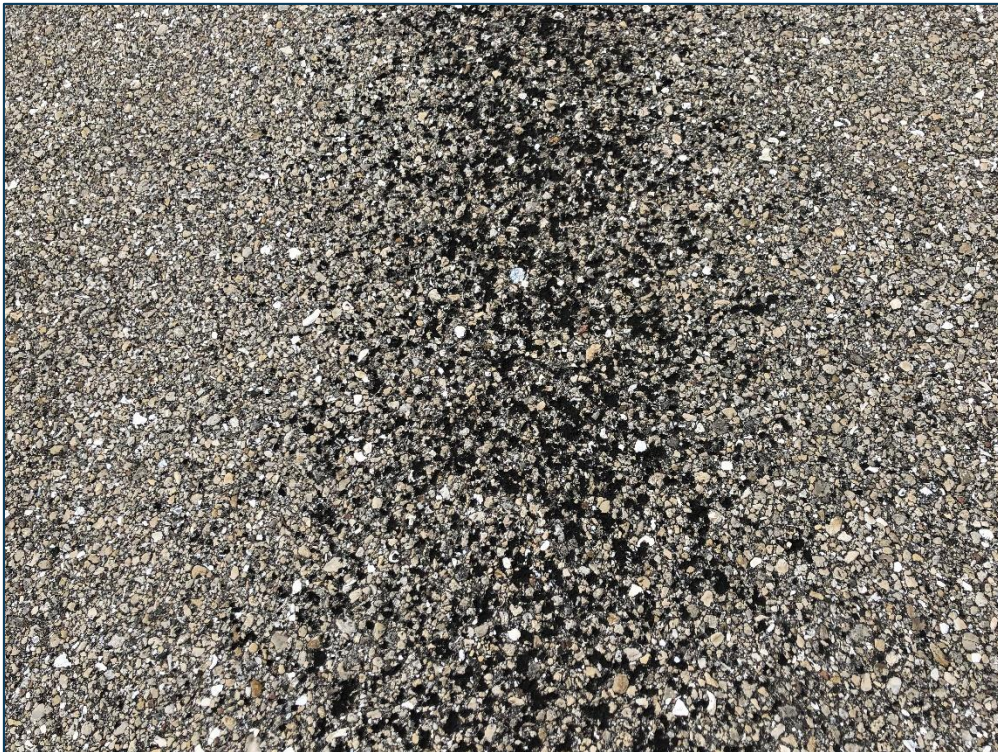
RW 4-22, Section 6125, Sample Unit291 - (42) Bleeding, Low Severity (52) Raveling, and Low Severity (57) Weathering
