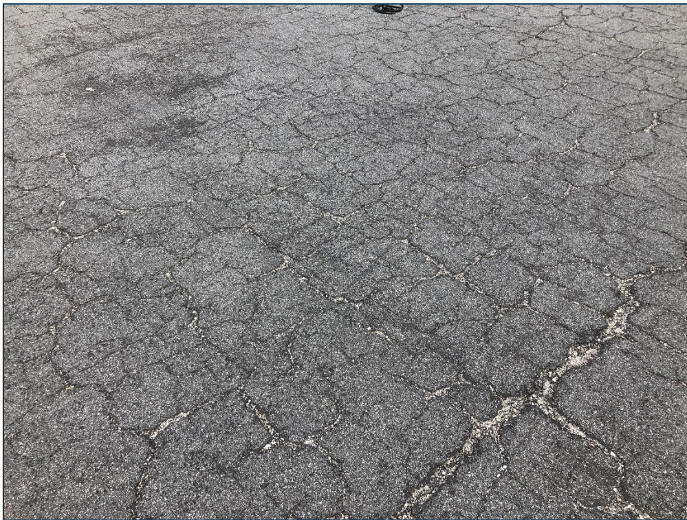
AP S, Section 4105, Sample Unit 405 - Low Severity (43) Block Cracking, Low and Medium Severity (52) Raveling
