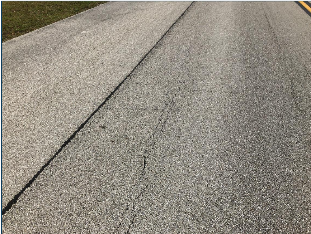
TWD, Section 115, Sample Unit 114 - Low Severity (41) Alligator Cracking, Low Severity (48) Longitudinal & Transverse Cracking, and Low Severity (57) Weathering
