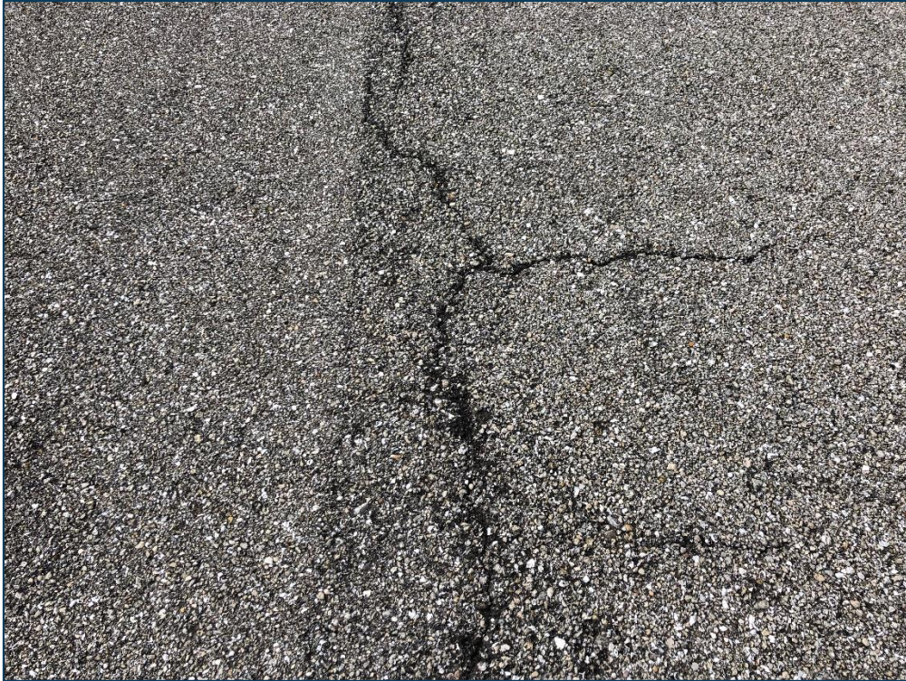
RW 9-27, Section 6305, Sample Unit 345 - Low Severity (48) Longitudinal & Transverse Cracking, Medium Severity (48) Longitudinal & Transverse Cracking, Low Severity (52) Raveling, and Medium Severity (52) Raveling
