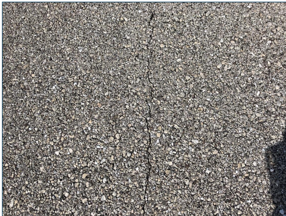
TWA, Section 330, Sample Unit 203 - Low Severity (48) Longitudinal & Transverse Cracking, Low Severity (52) Raveling, and Low Severity (57) Weathering
