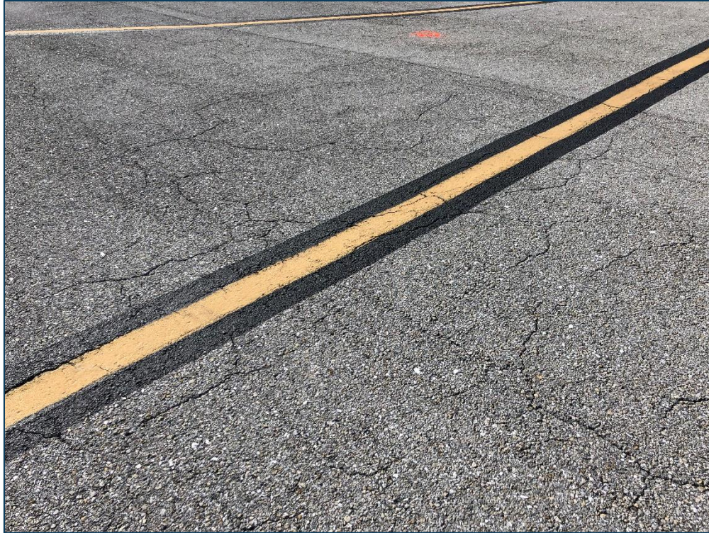
RW 15-33, Section 6210, Sample Unit 348 - Low Severity (43) Block Cracking, Low Severity (52) Raveling, and Medium Severity (57) Weathering
