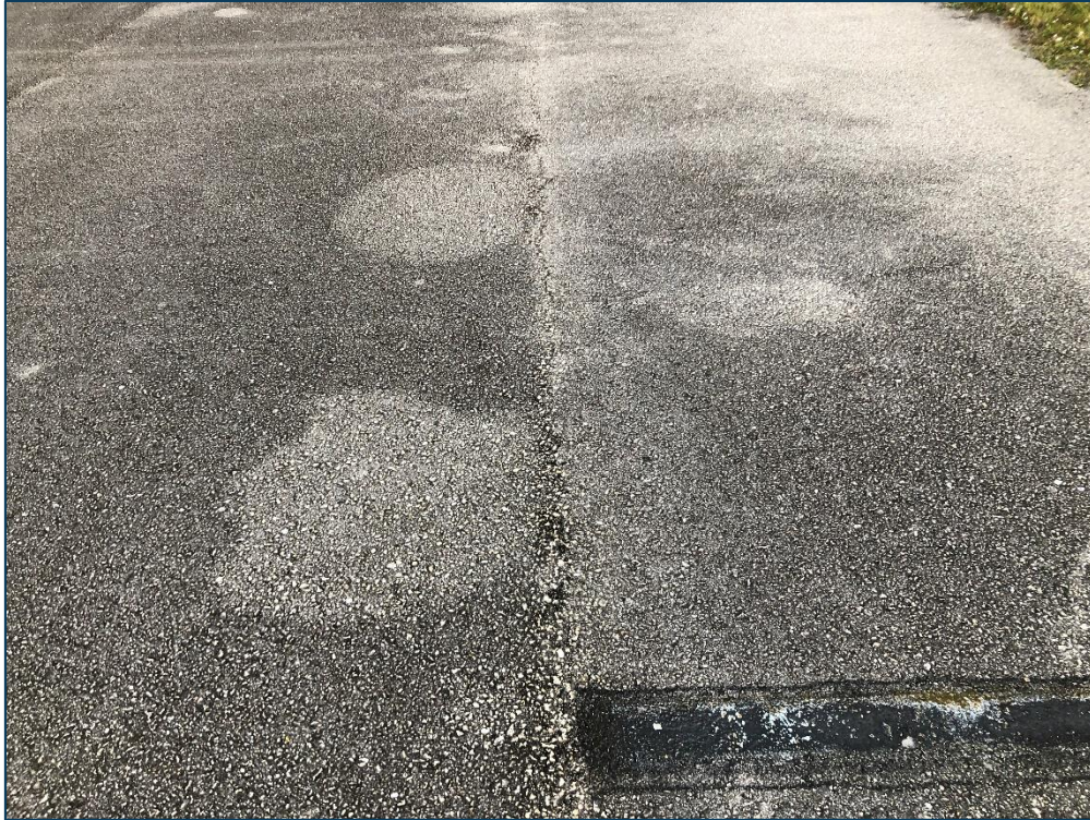
TWC, Section 315, Sample Unit 105 - Low Severity (48) Longitudinal & Transverse Cracking, Low and Medium Severity (52) Raveling
