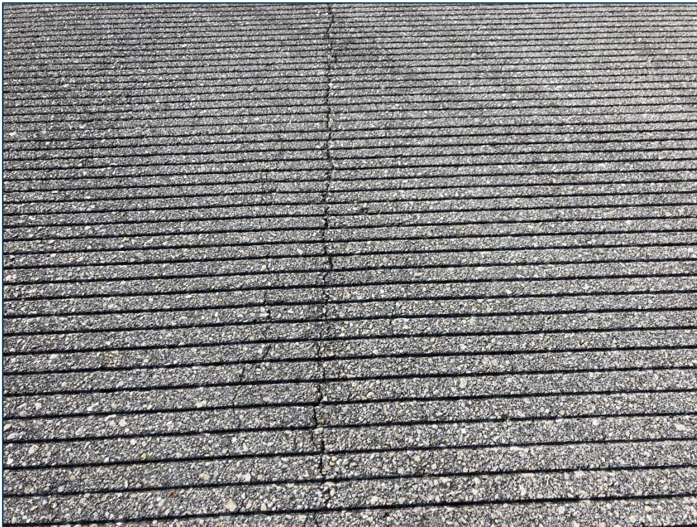
RW 5-23, Section 6105, Sample Unit354 - Low Severity (48) Longitudinal & Transverse Cracking and Low Severity (57) Weathering
