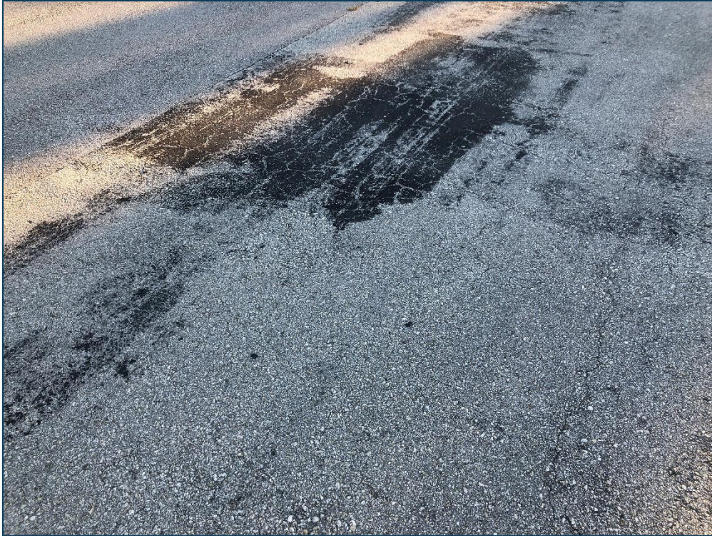
AP COMMERC, Section 4105, Sample Unit 400 - Low Severity (48) Longitudinal & Transverse Cracking and Low Severity (52) Raveling
