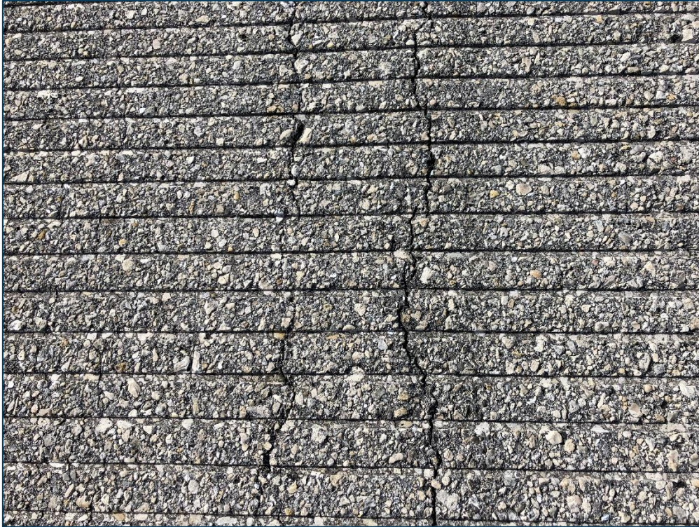
RW 5-23, Section 6105, Sample Unit339 - Low Severity (41) Alligator Cracking, Low and Medium Severity (57) Weathering
