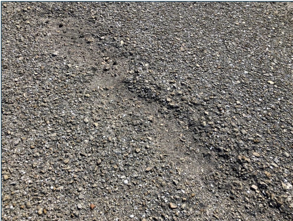
AP GA, Section 4295, Sample Unit 354 - Low and Medium Severity (52) Raveling.
