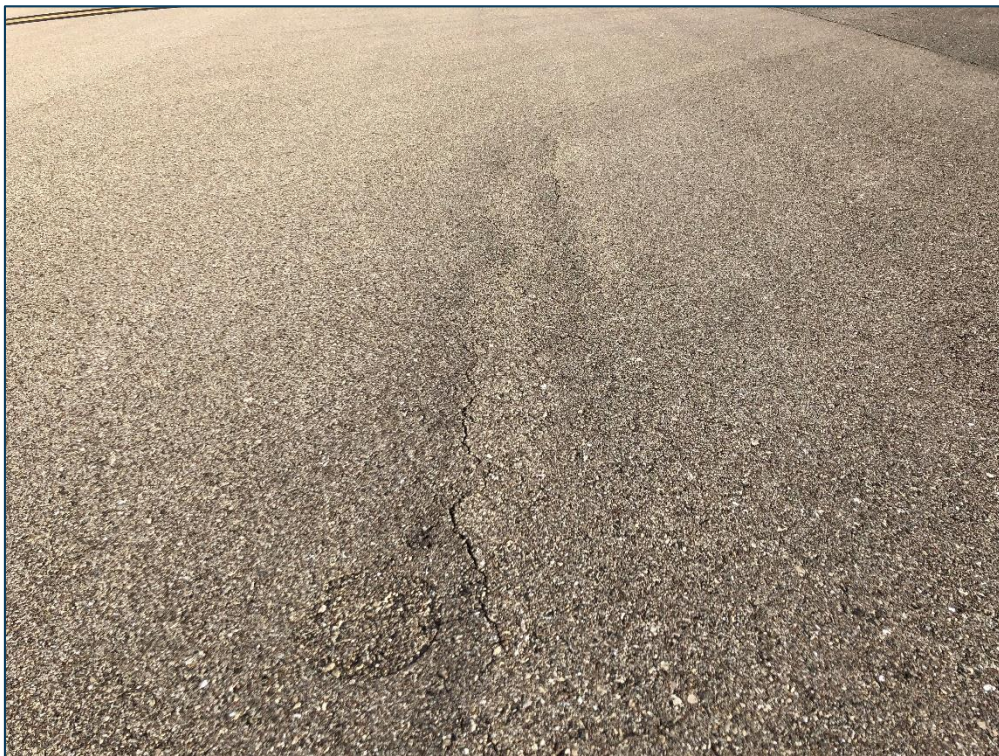
TWB, Section 205, Sample Unit 126 - Low Severity (48) Longitudinal & Transverse Cracking, Low Severity (56) Swelling, and Low Severity (57) Weathering
