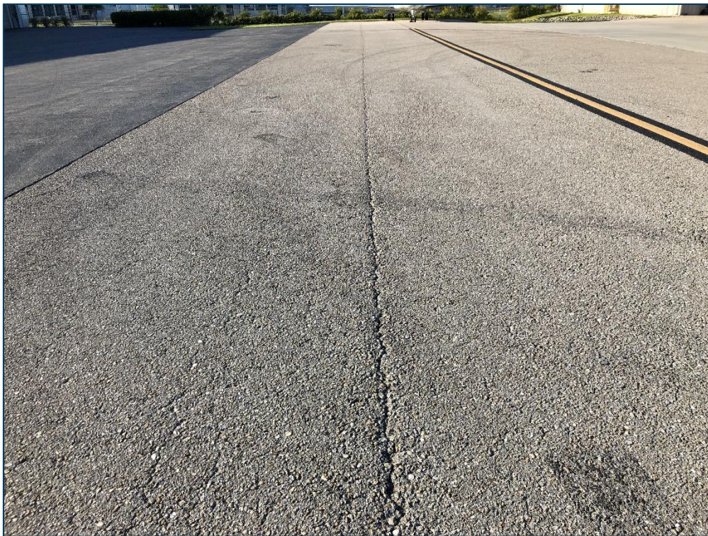
TWD3, Section 1110, Sample Unit 303 - Low and Medium Severity (48) Longitudinal & Transverse Cracking, Low and Medium Severity (52) Raveling
