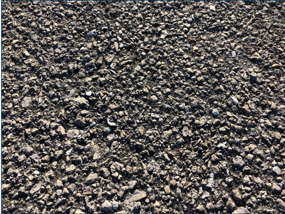
TWA, Section 165, Sample Unit 151 - Medium Severity (52) Raveling
