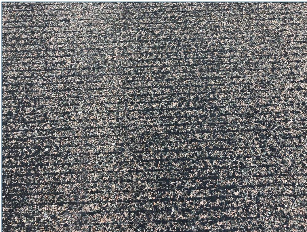
RW 18L-36R, Section 6197, Sample Unit 292 - (42) Bleeding and Low Severity (57) Weathering
