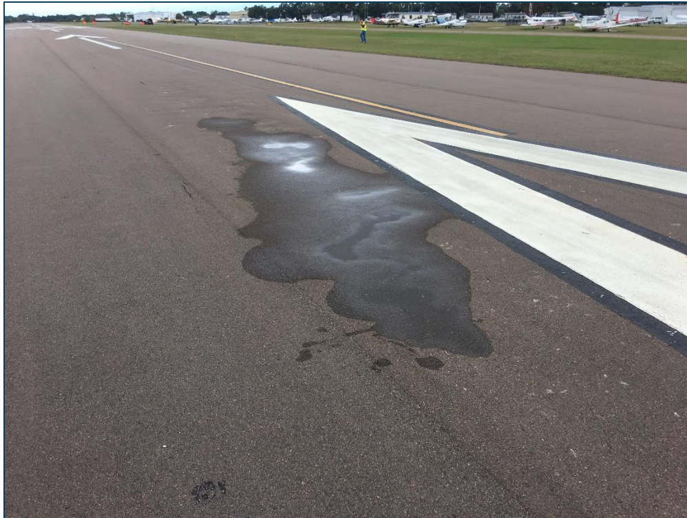
RW 16-34, Section 6110, Sample Unit 102 - Low Severity (45) Depression, Low Severity (48) Longitudinal & Transverse Cracking, Low Severity (56) Swelling, and Low Severity (57) Weathering
