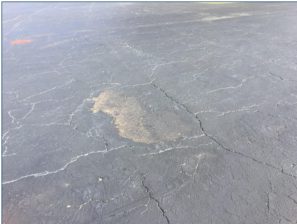
TW CONN 34, Section 5105, Sample Unit 102 - Low Severity (43) Block Cracking, Medium Severity (43) Block Cracking, Low Severity (48) Longitudinal & Transverse Cracking, and Low Severity (52) Raveling
