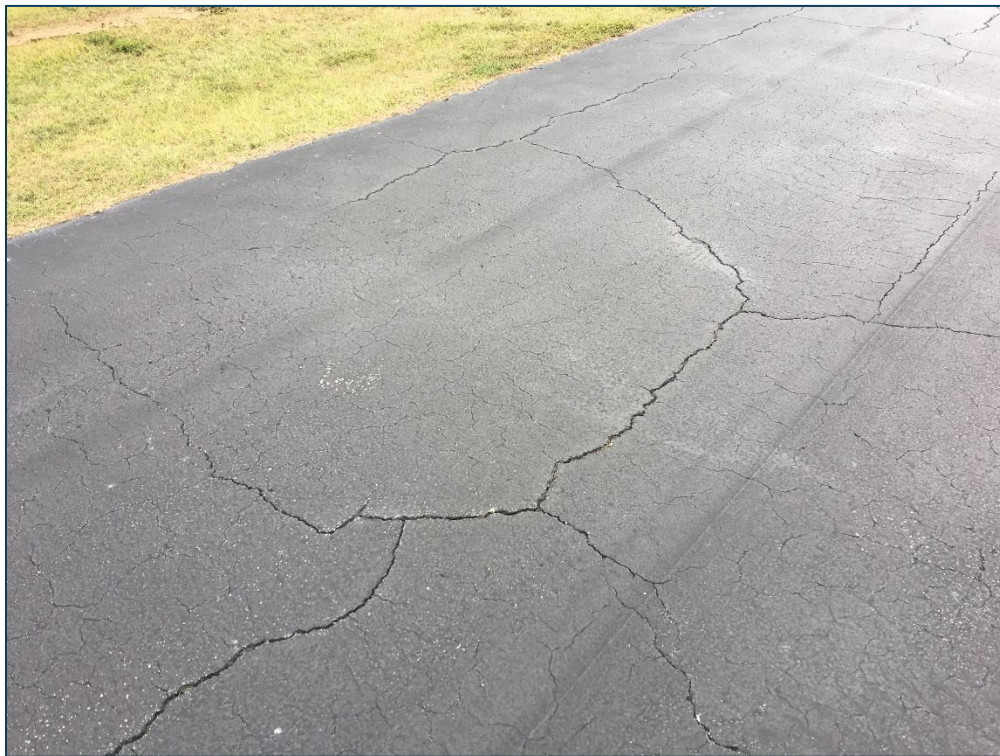
AP T-HANG, Section 4605, Sample Unit 105 - Severity (43) Block Cracking, Medium Severity (43) Block Cracking, and Low Severity (52) Raveling
