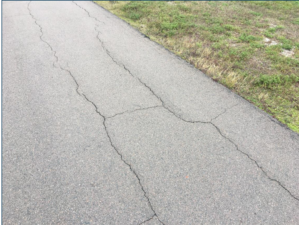
TW A, Section 135, Sample Unit 128 - Low Severity (48) Longitudinal & Transverse Cracking, Medium Severity (48) Longitudinal & Transverse Cracking, and Low Severity (57) Weathering
