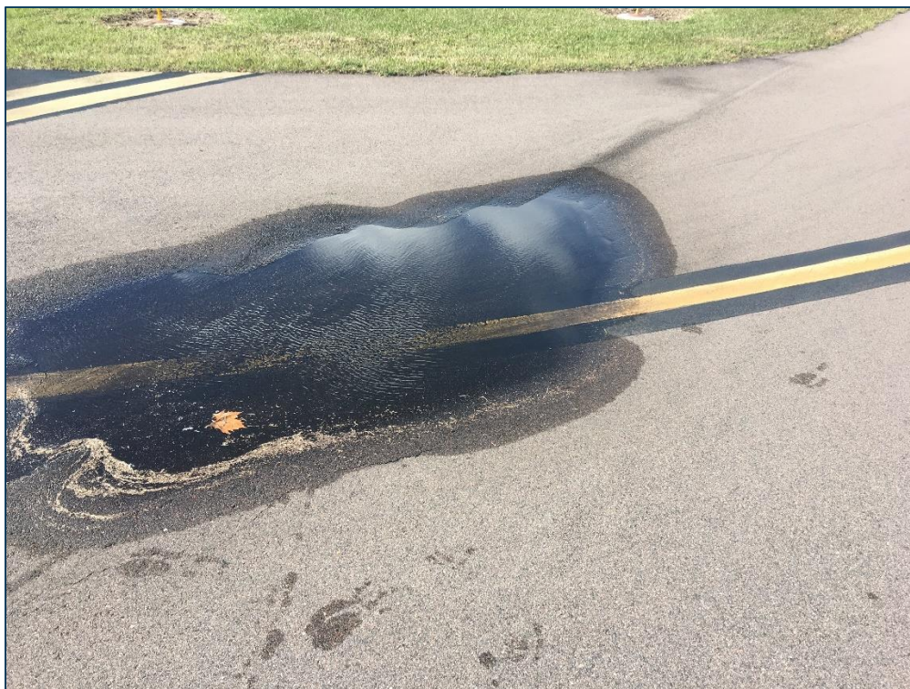
TW A, Section 105, Sample Unit 102 - Medium Severity (45) Depression, Low Severity (48) Longitudinal & Transverse Cracking, and Low Severity (57) Weathering
