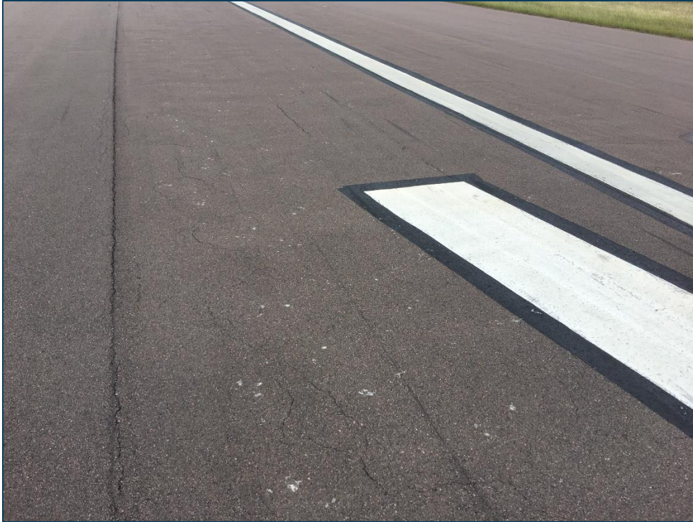
RW 16-34, Section 6110, Sample Unit 110 - Low Severity (48) Longitudinal & Transverse Cracking, Low Severity (56) Swelling, and Low Severity (57) Weathering
