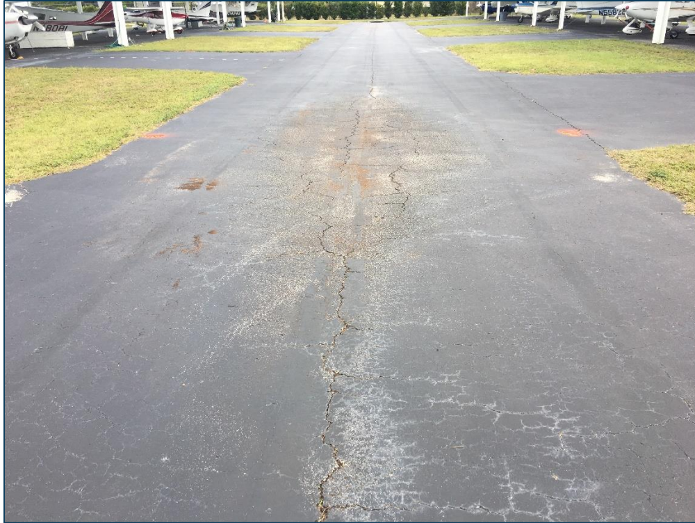
AP T-HAN 2, Section 4105, Sample Unit 400 - Low Severity (43) Block Cracking, Low Severity (45) Depression, Medium Severity (48) Longitudinal & Transverse Cracking, and Low Severity (52) Raveling
