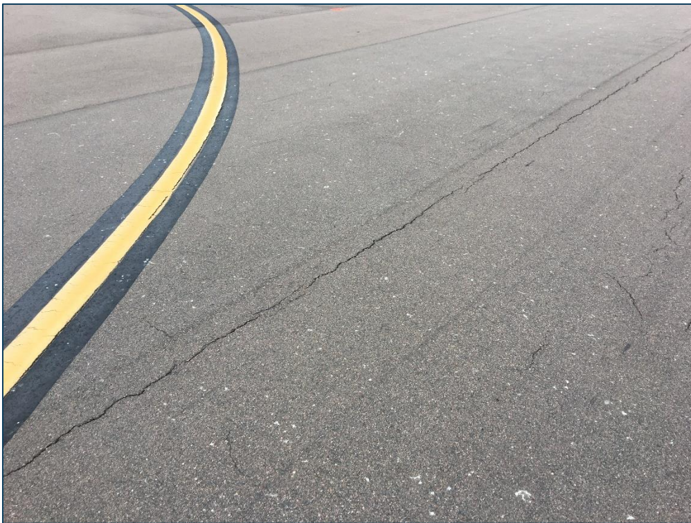
RW 16-34, Section 6110, Sample Unit 130 - Low Severity (48) Longitudinal & Transverse Cracking, Low Severity (56) Swelling, and Low Severity (57) Weathering
