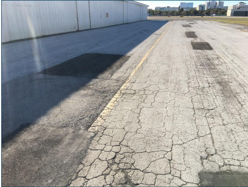
AP, Section 4120, Sample Unit 455 - Medium Severity (41) Alligator Cracking, Low Severity (50) Patching, and Medium Severity (52) Raveling
