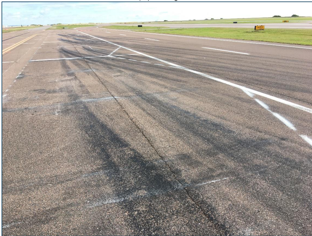
AP W, Section 4210, Sample Unit 103 - Low Severity (48) Longitudinal & Transverse Cracking and Low Severity (52) Raveling
