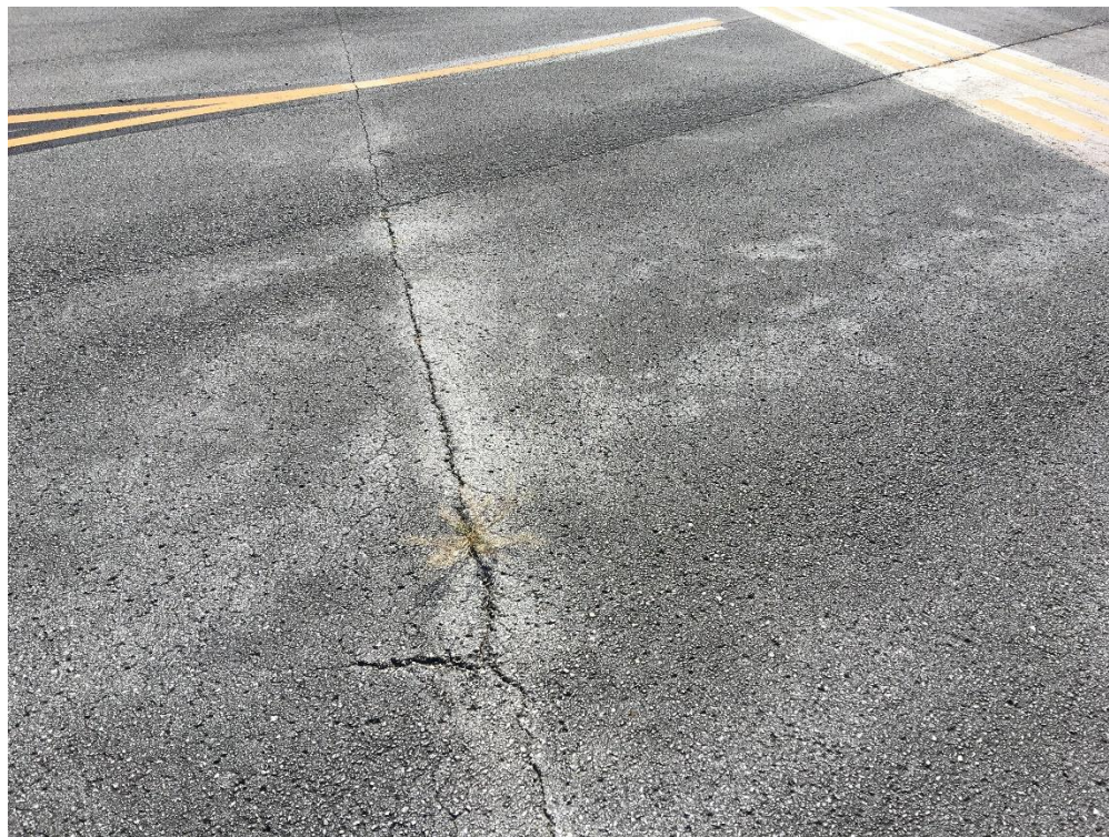
TW B, Section 253, Sample Unit 100 - Low Severity (48) Longitudinal & Transverse Cracking, Low Severity (52) Raveling, and Medium Severity (52) Raveling
