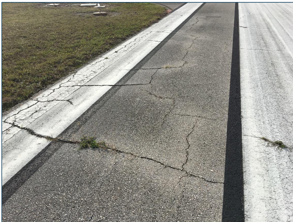
RW 18-36, Section 6110, Sample Unit 552 - Medium Severity (43) Block Cracking, Low Severity (48) Longitudinal & Transverse Cracking, and Low Severity (52) Raveling
