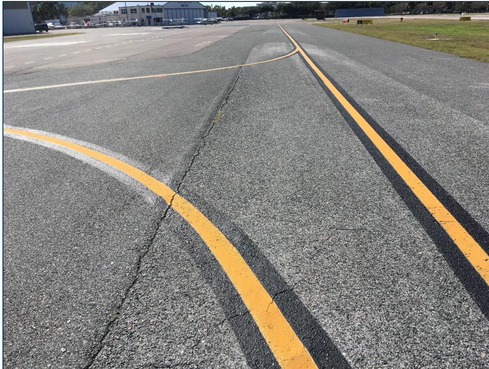
TW A, Section 105, Sample Unit 103 - Low Severity (48) Longitudinal & Transverse Cracking, Medium Severity (48) Longitudinal & Transverse Cracking, Low Severity (52) Raveling, and Medium Severity (52) Raveling
