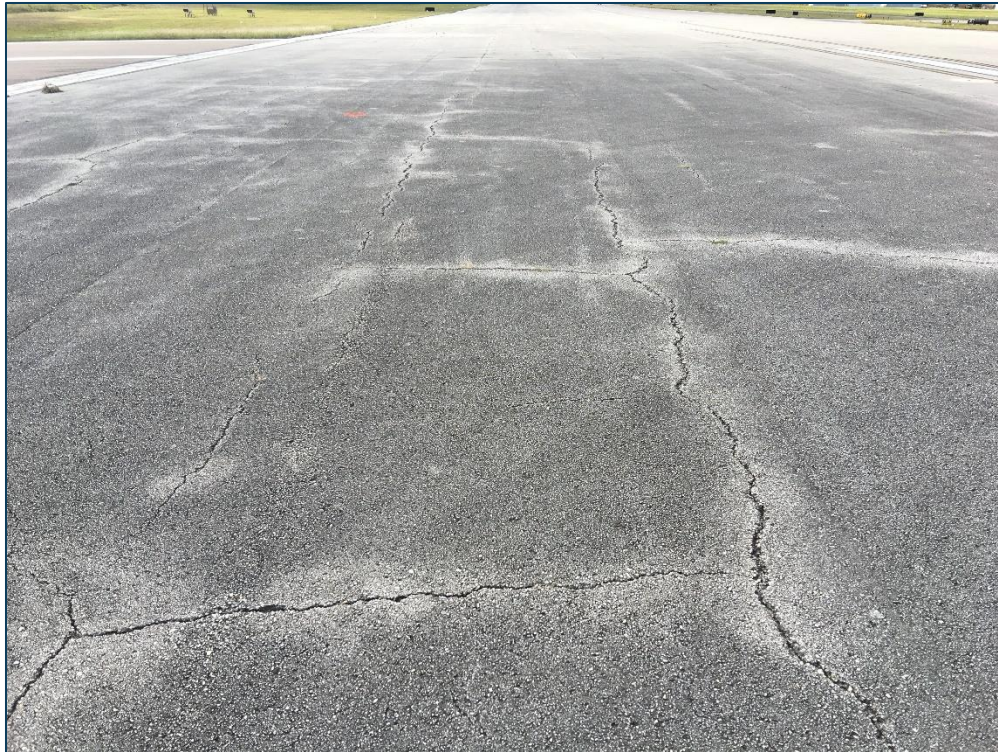
RW 18-36, Section 6105, Sample Unit 350 - Medium Severity (43) Block Cracking, Low Severity (48) Longitudinal & Transverse Cracking, Low Severity (52) Raveling, and Medium Severity (52) Raveling
