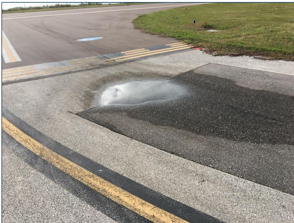
TAXIWAY D, Section 155, Sample Unit 101 - High Severity (45) Depression, Low Severity (48) Longitudinal & Transverse Cracking, Medium Severity (50) Patching, and Low Severity (52) Raveling
