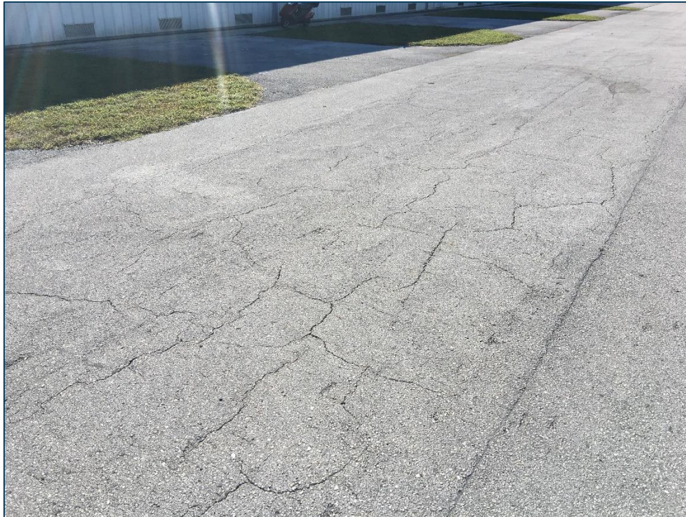
TW C, Section 307, Sample Unit 209 - Low Severity (43) Block Cracking, Low Severity (48) Longitudinal & Transverse Cracking, Low Severity (52) Raveling, and Low Severity (56) Swelling
