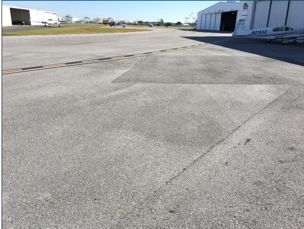
AP, Section 4110, Sample Unit 603 - Low Severity (45) Depression, Low Severity (48) Longitudinal & Transverse Cracking, Low Severity (50) Patching, Low Severity (52) Raveling, and Low Severity (57) Weathering
