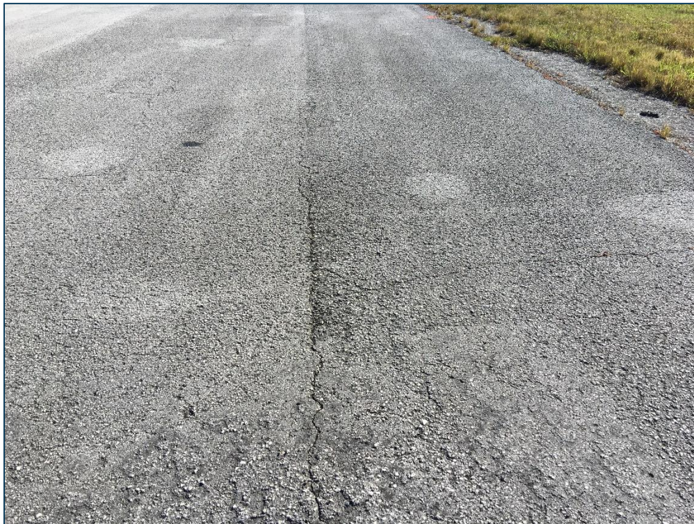
AP, Section 4140, Sample Unit 102 - Low Severity (48) Longitudinal & Transverse Cracking, Low Severity (52) Raveling, and Medium Severity (52) Raveling
