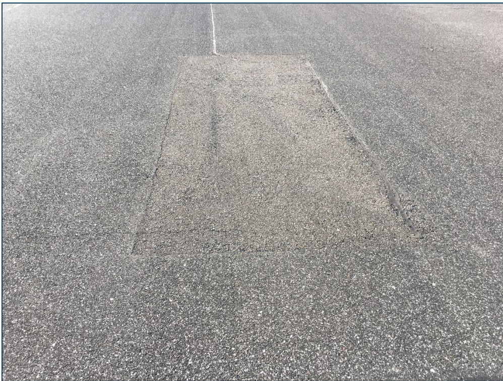
RW 18-36, Section 6205, Sample Unit 108 - Low Severity (48) Longitudinal & Transverse Cracking, Low Severity (50) Patching, Low Severity (52) Raveling, and Low Severity (57) Weathering
