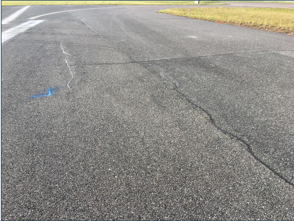
RW 18-36, Section 6205, Sample Unit 102 - Low Severity (48) Longitudinal & Transverse Cracking, Low Severity (52) Raveling, and Low Severity (57) Weathering
