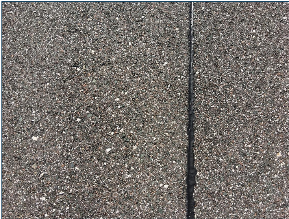
TW F, Section 605, Sample Unit 114 - Low Severity (48) Longitudinal & Transverse Cracking, Low Severity (52) Raveling, and Low Severity (57) Weathering
