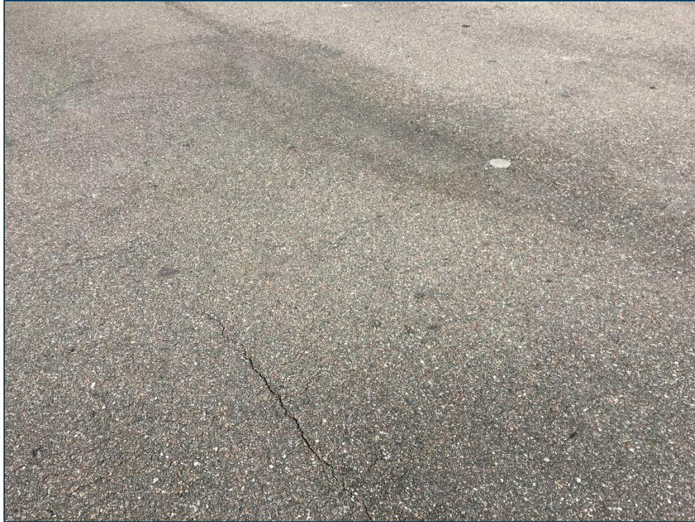
TL T-HANG, Section 710, Sample Unit 152 - Low Severity (45) Depression, Low Severity (48) Longitudinal & Transverse Cracking, Low Severity (52) Raveling, and Low Severity (57) Weathering
