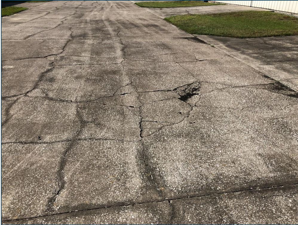
AP NW, Section 4615, Sample Unit 502 - High Severity (65) Joint Seal Damage
