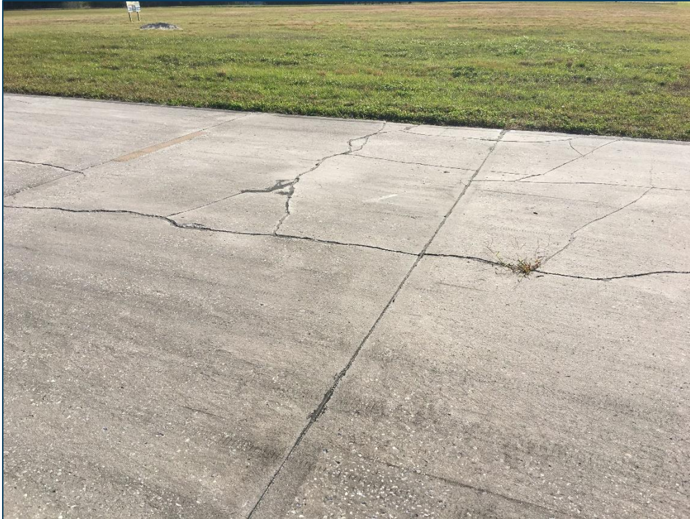
TW E, Section 520, Sample Unit 451 - Low Severity (66) Small Patch and Low Severity (72) Shattered Slab
