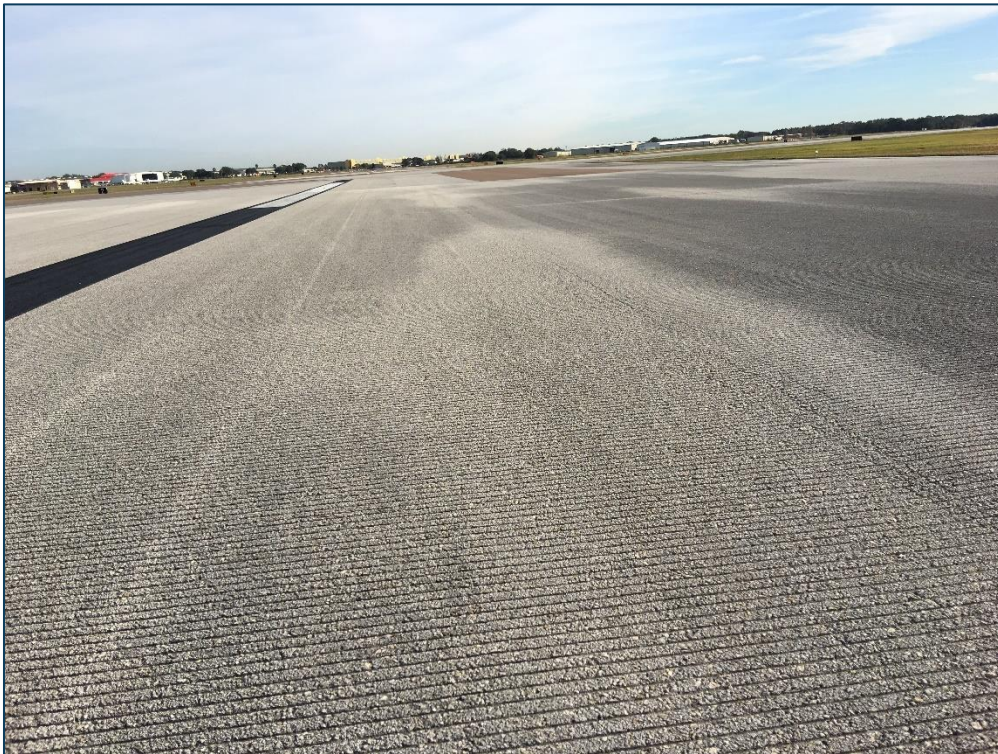
RW 5-23, Section 6255, Sample Unit 353 - Low Severity (48) Longitudinal & Transverse Cracking, Low Severity (52) Raveling, and Medium Severity (57) Weathering
