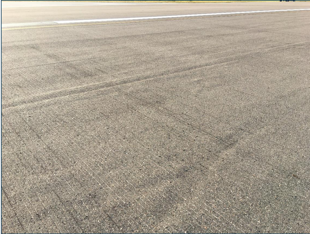
RW 5-23, Section 6245, Sample Unit 374 - Low Severity (52) Raveling and Low Severity (56) Swelling
