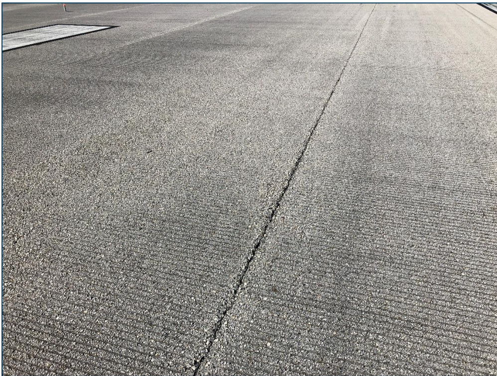
RW 9-27, Section 6115, Sample Unit 360 - Medium Severity (48) Longitudinal & Transverse Cracking, Low Severity (52) Raveling, and Low Severity (57) Weathering
