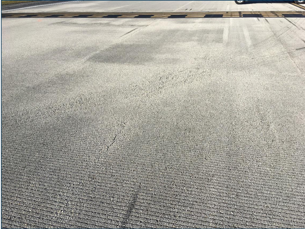
RW 9-27, Section 6150, Sample Unit 421 - Low Severity (48) Longitudinal & Transverse Cracking, Low Severity (52) Raveling, and Medium Severity (52) Raveling
