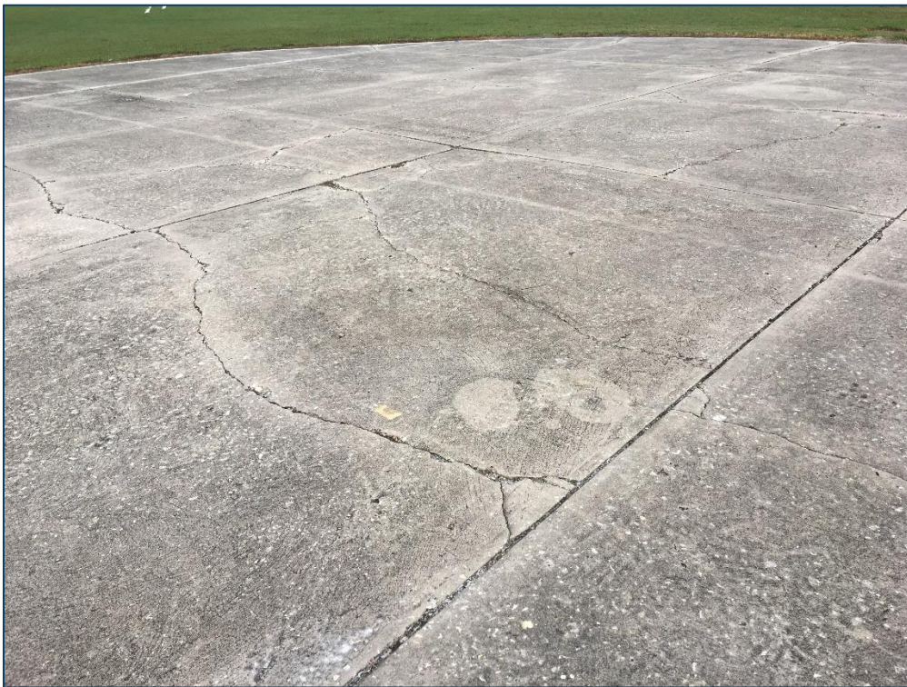
AP SW, Section 917, Sample Unit 202 - Medium Severity (63) Linear Cracking, High Severity (65) Joint Seal Damage, and Low Severity (74) Joint Spall
