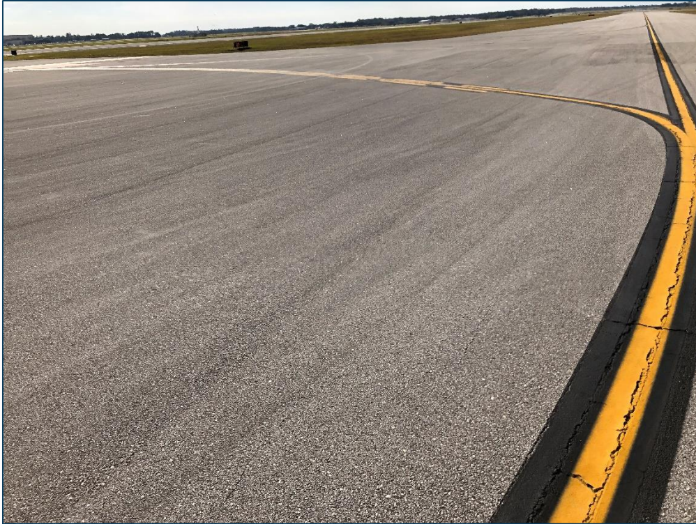
TW A, Section 150, Sample Unit 227 - Low Severity (48) Longitudinal & Transverse Cracking, Low Severity (52) Raveling, and Medium Severity (57) Weathering
