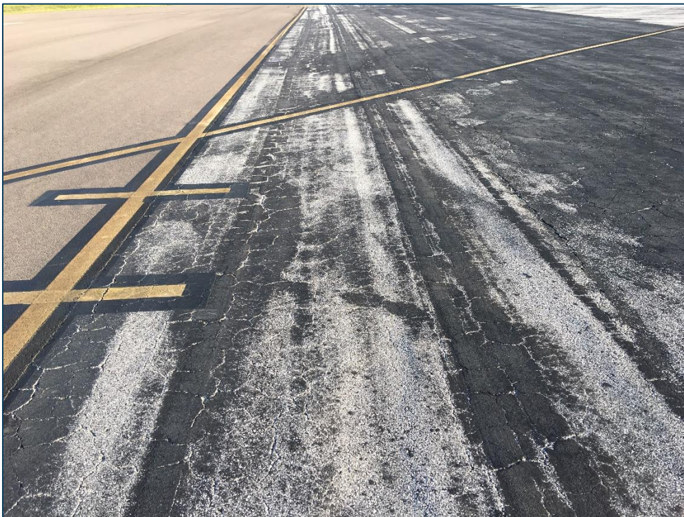
AP N, Section 4140, Sample Unit 203 - Low Severity (43) Block Cracking, Low Severity (48) Longitudinal & Transverse Cracking, and Low Severity (52) Raveling
