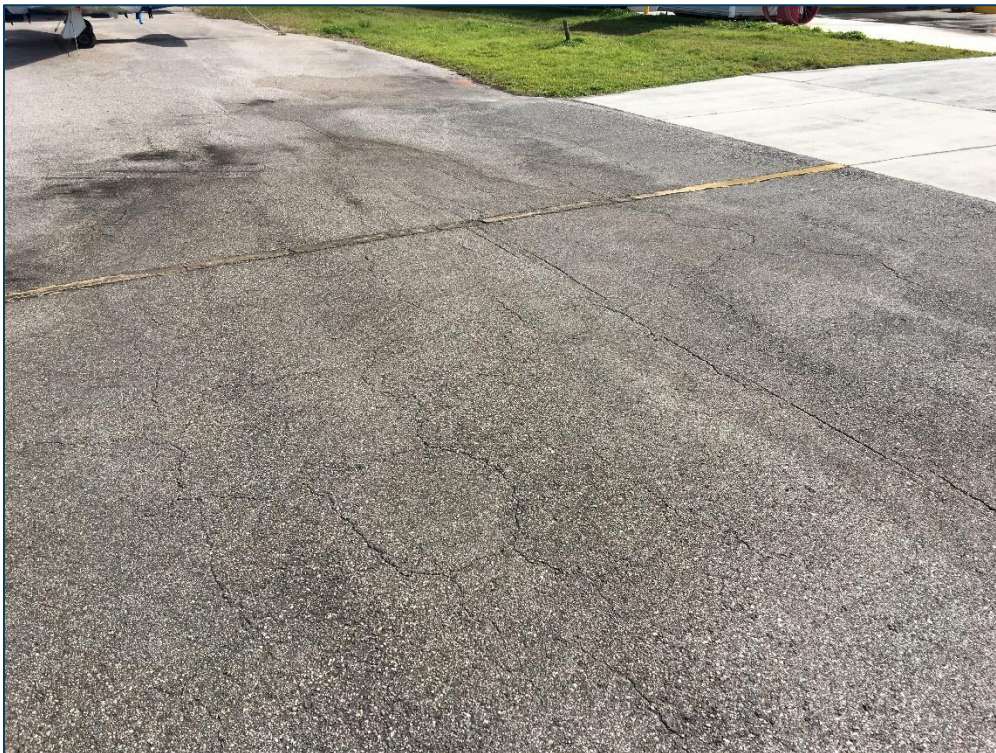
AP S, Section 4105, Sample Unit 200 - Low Severity (43) Block Cracking, Low Severity (45) Depression, Low Severity (48) Longitudinal & Transverse Cracking, Low Severity (56) Swelling, and Medium Severity (57) Weathering
