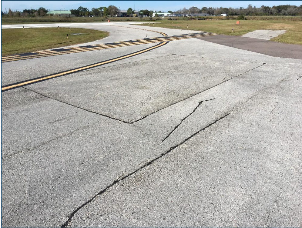
TW A, Section 105, Sample Unit 130 - Low Severity (48) Longitudinal & Transverse Cracking, Low Severity (50) Patching, Medium Severity (50) Patching, Low Severity (52) Raveling, Medium Severity (52) Raveling, and Low Severity (56) Swelling
