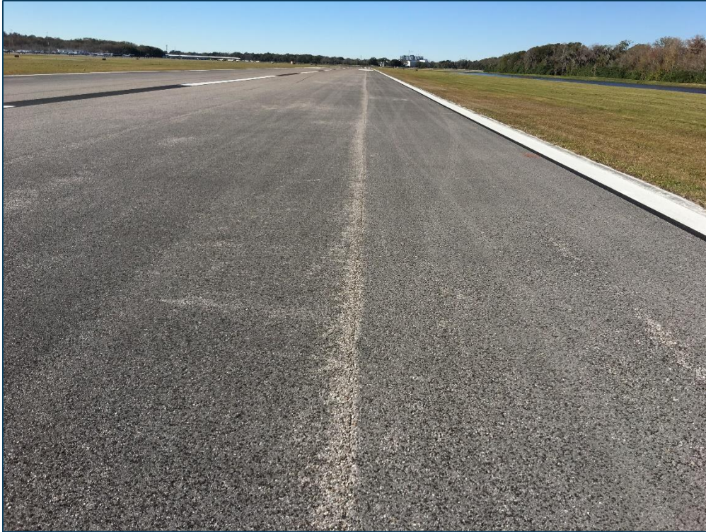
RW 5-23, Section 6205, Sample Unit 138 - Low Severity (48) Longitudinal & Transverse Cracking, Medium Severity (48) Longitudinal & Transverse Cracking, Low Severity (52) Raveling, and Medium Severity (57) Weathering
