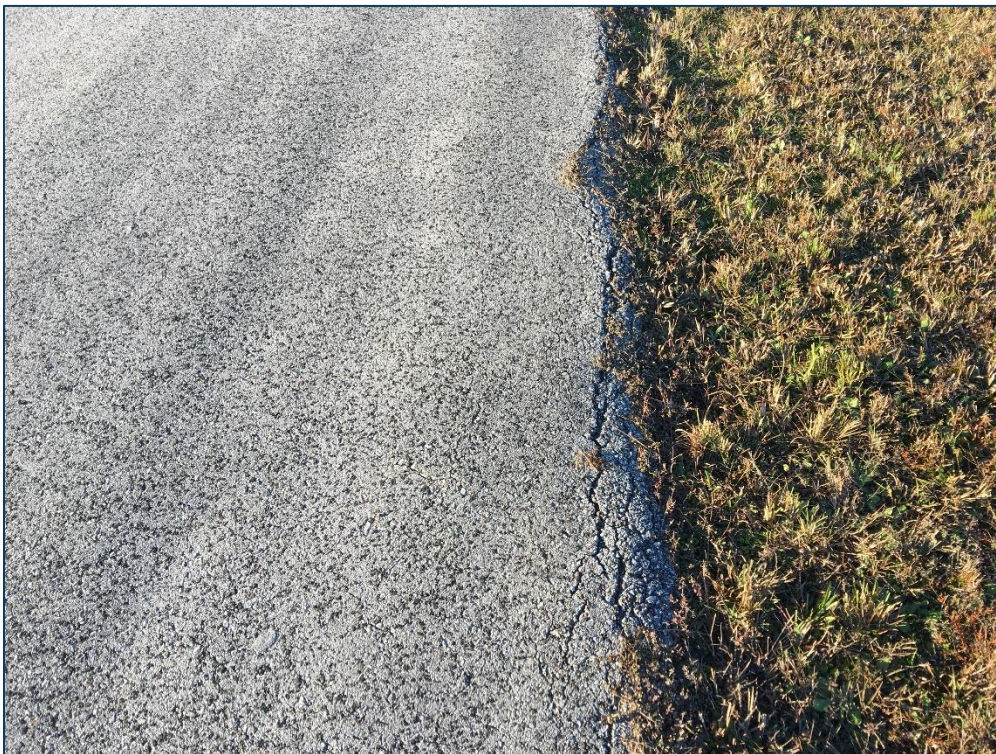
TW E, Section 505, Sample Unit 134 - Medium Severity (48) Longitudinal & Transverse Cracking, Low Severity (52) Raveling, and Medium Severity (57) Weathering
