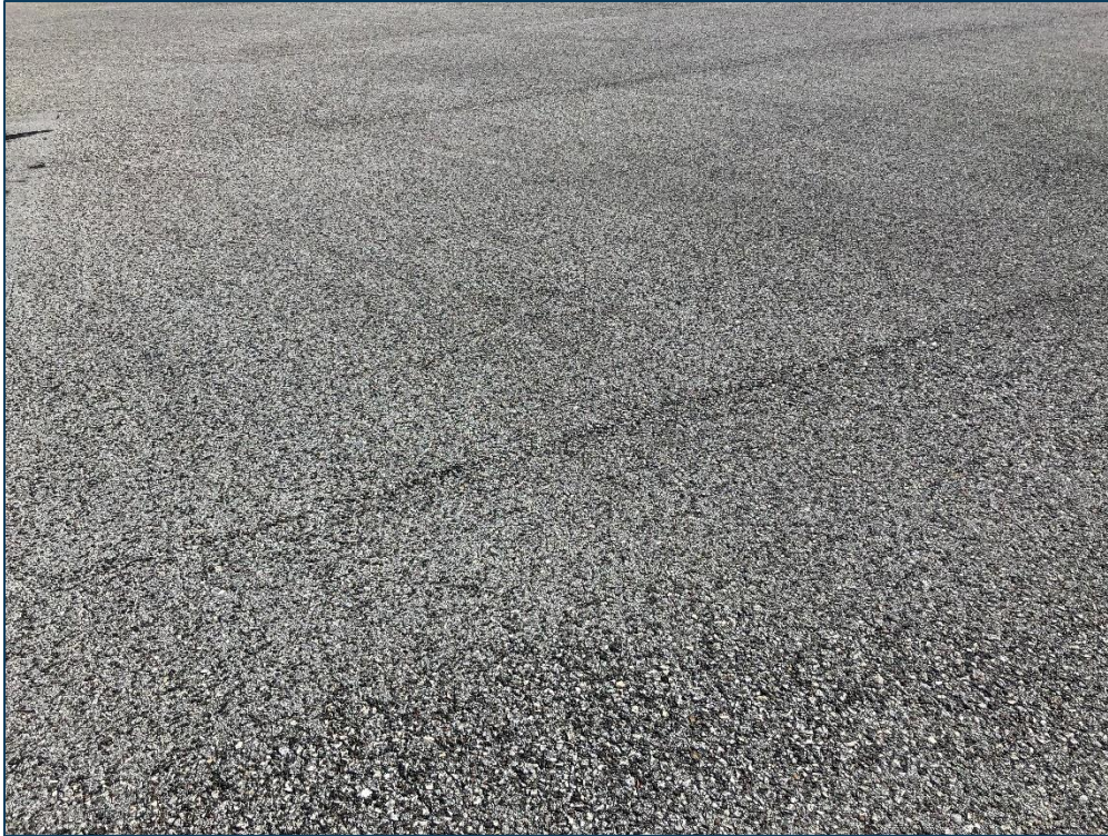
AP MAIN, Section 4410, Sample Unit 900 - Low Severity (48) Longitudinal & Transverse Cracking, Low Severity (52) Raveling, and Medium Severity (57) Weathering
