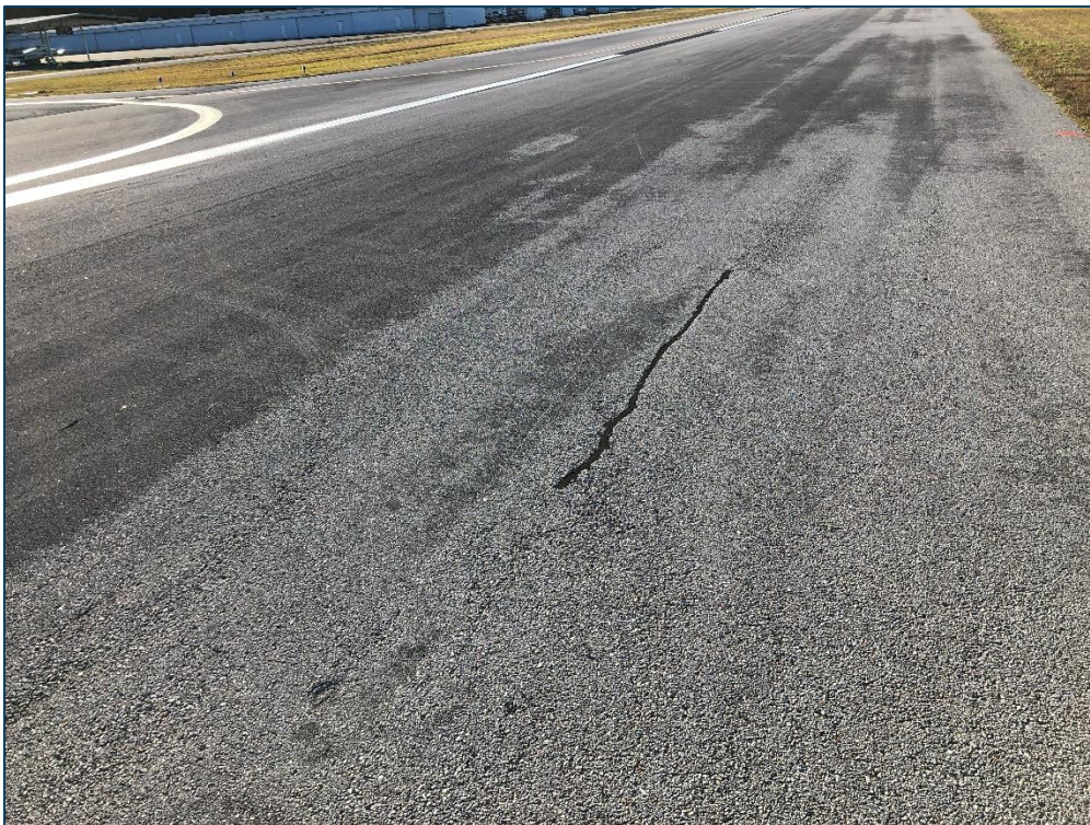
RW 18-36, Section 6105, Sample Unit 131 - Low Severity (48) Longitudinal & Transverse Cracking, Low Severity (52) Raveling, and Medium Severity (57) Weathering
