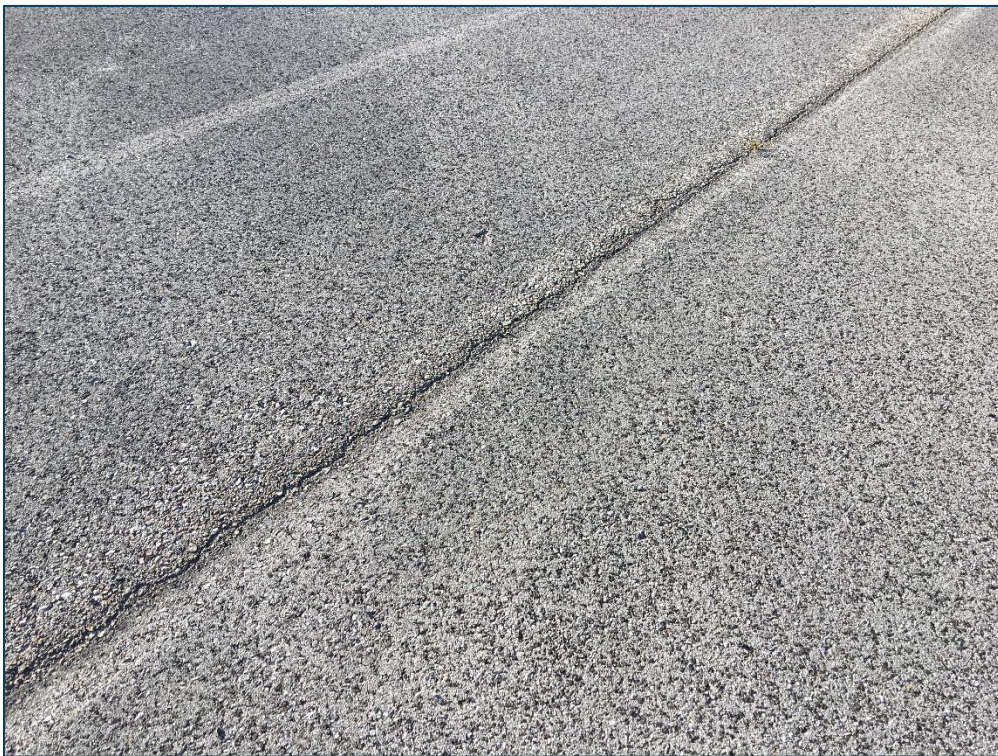
RW 5-23, Section 6205, Sample Unit 196 - Medium Severity (48) Longitudinal & Transverse Cracking, Low Severity (52) Raveling, and Medium Severity (57) Weathering
