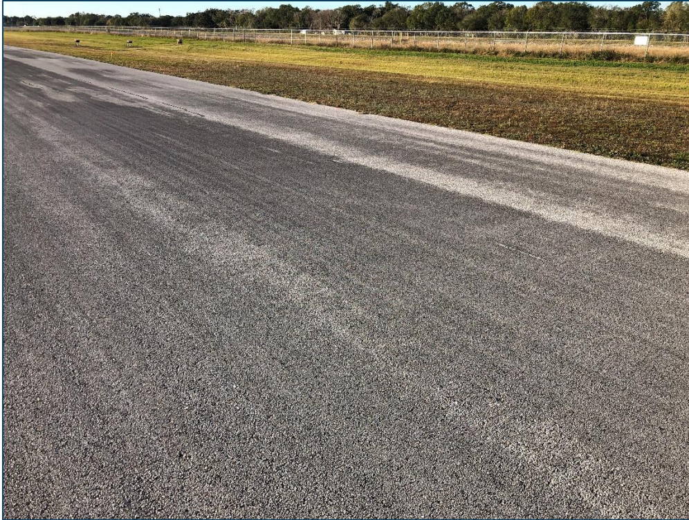
RW 18-36, Section 6105, Sample Unit 119 - Low Severity (48) Longitudinal & Transverse Cracking, Low Severity (52) Raveling, and Medium Severity (57) Weathering
