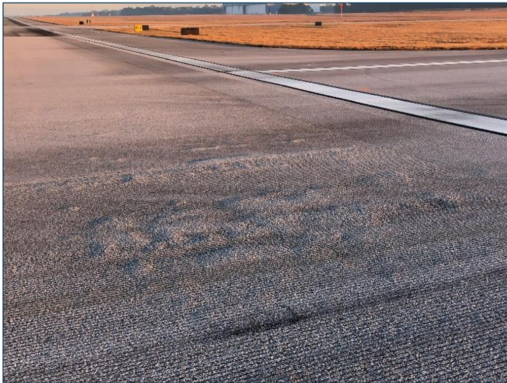
RW 17-35, Section 6120, Sample Unit 554 - Low Severity (56) Swelling and Low Severity (57) Weathering
