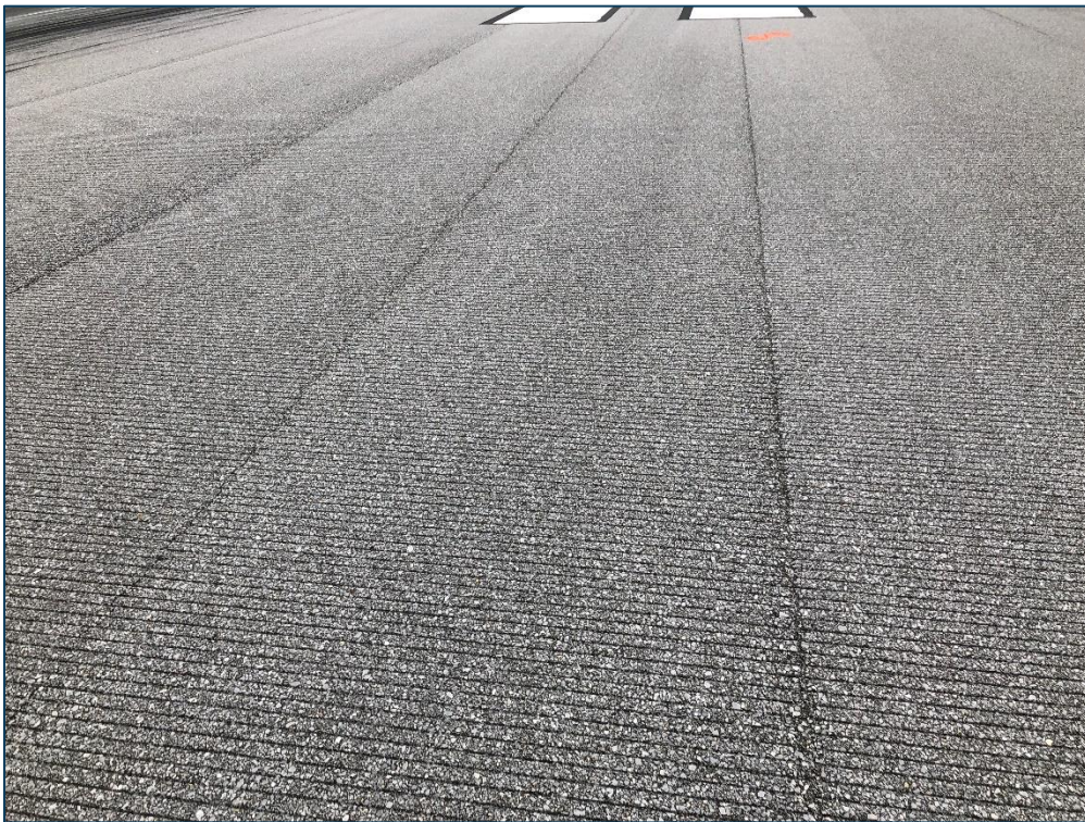
RW 8-26, Section 6245, Sample Unit 407 - Low Severity (48) Longitudinal & Transverse Cracking and Low Severity (57) Weathering
