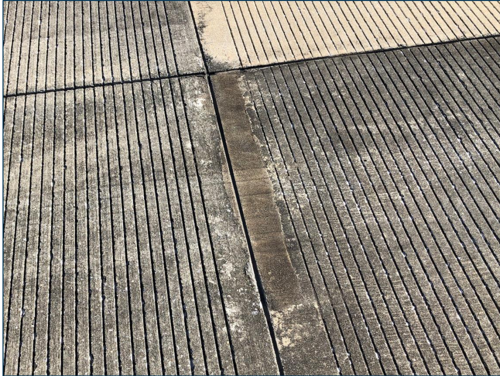
RW 17-35, Section 6125, Sample Unit 374 - Low Severity (66) Small Patch
