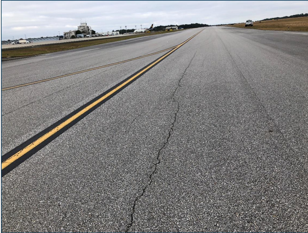
TW A, Section 115, Sample Unit 113 - Low and Medium Severity (48) Longitudinal & Transverse Cracking and Low Severity (57) Weathering
