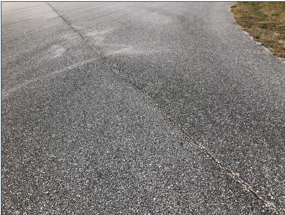
TW B, Section 210, Sample Unit 105 - Low and Medium Severity (48) Longitudinal & Transverse Cracking and Low Severity (57) Weathering
