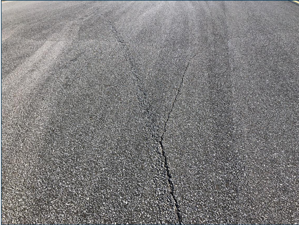
TW D, Section 140, Sample Unit 306 - Low and Medium Severity (48) Longitudinal & Transverse Cracking, Low Severity (52) Raveling, and Low Severity (57) Weathering
