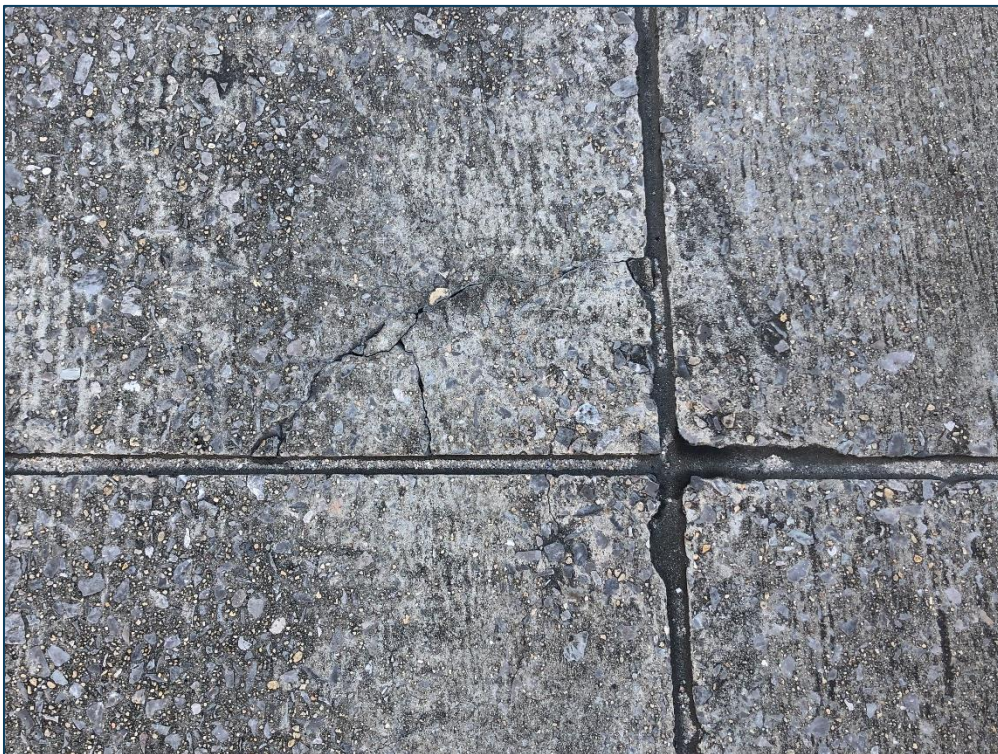
AP TERM, Section 4205, Sample Unit 211 - Low Severity (75) Corner Spall
