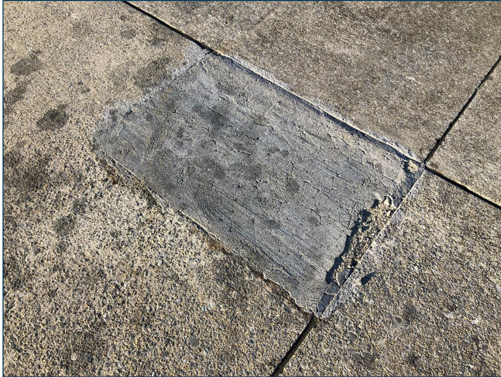
AP TERM, Section 4210, Sample Unit 906 - Medium Severity (67) Large Patch/Utility Cut
