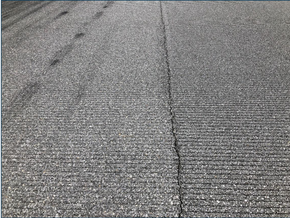
RW 8-26, Section 6225, Sample Unit 336 - Low Severity (48) Longitudinal & Transverse Cracking and Low Severity (57) Weathering
