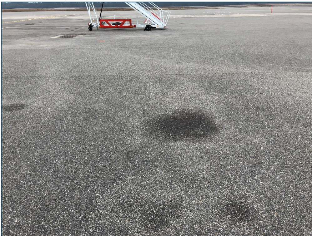
AP CARGO, Section 4210, Sample Unit 319 - Low Severity (45) Depression, (49) Oil Spillage, Low Severity (52) Raveling, and Low Severity (57) Weathering
