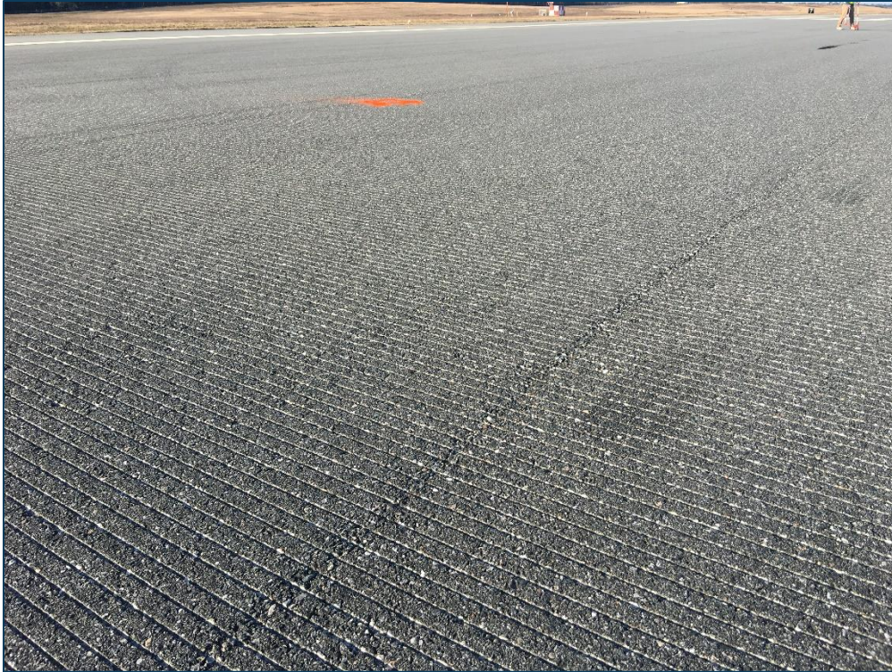
RW 9-27, Section 6205, Sample Unit 377 - Low Severity (48) Longitudinal & Transverse Cracking and Low Severity (57) Weathering
