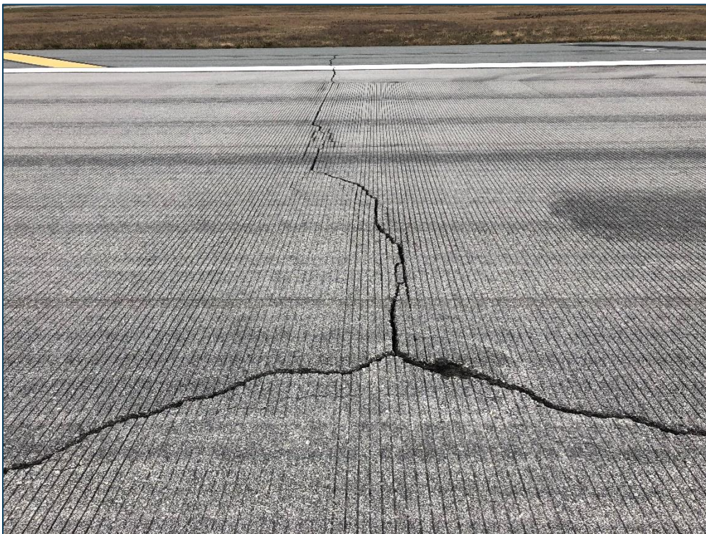
RW 18-36, Section 6105, Sample Unit 411 - Medium Severity (48) Longitudinal & Transverse Cracking and Medium Severity (57) Weathering
