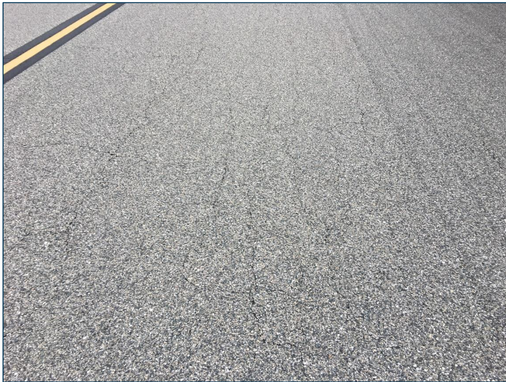
TW B, Section 205, Sample Unit 186 - Low Severity (41) Alligator Cracking and Low Severity (57) Weathering
