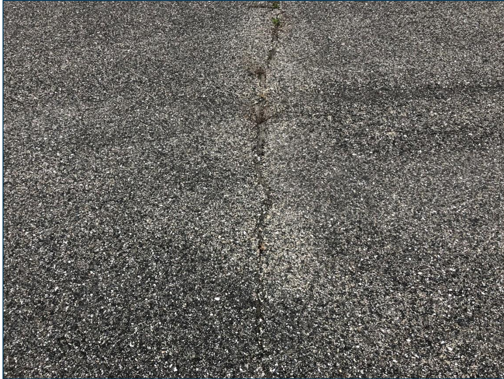
TW A, Section 105, Sample Unit 212 - Medium Severity (48) Longitudinal & Transverse Cracking, Low Severity (52) Raveling, and Medium Severity (57) Weathering
