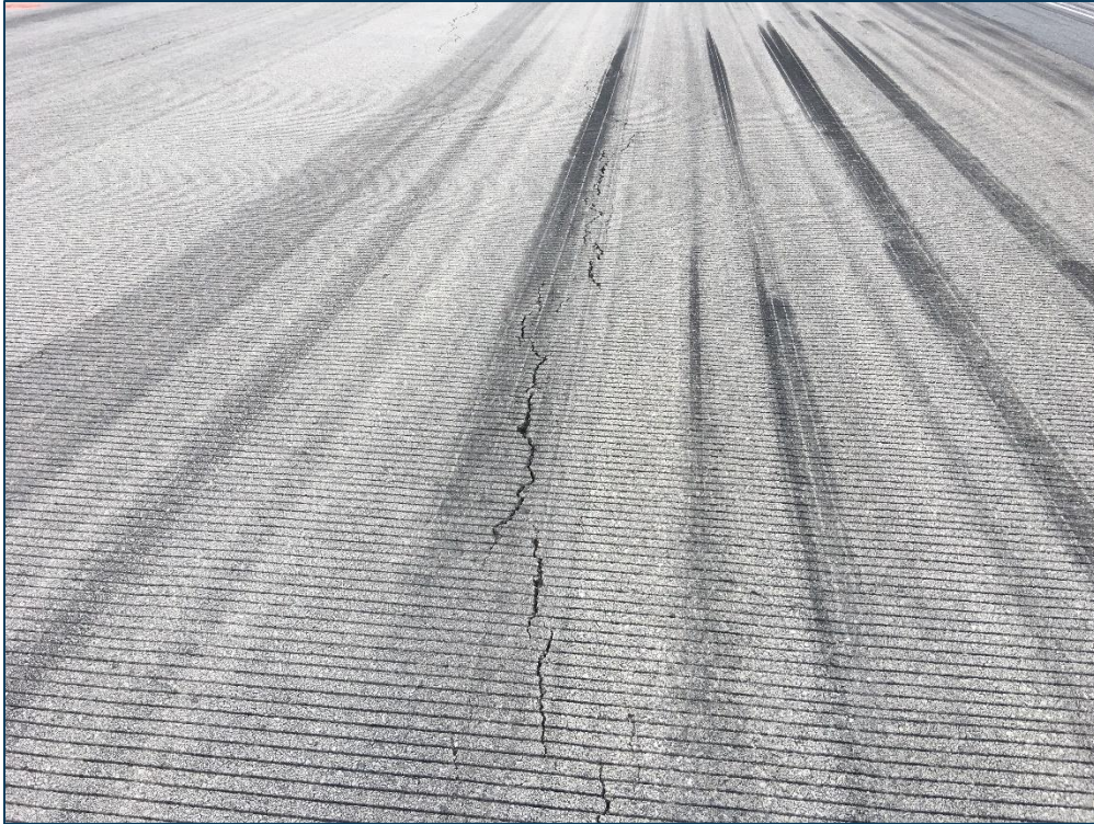
RW 18-36, Section 6105, Sample Unit 324 - Medium Severity (48) Longitudinal & Transverse Cracking and Medium Severity (57) Weathering
