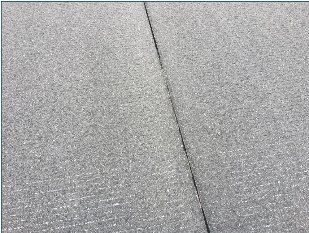
RW 9-27, Section 6210, Sample Unit 113 - Low Severity (48) Longitudinal & Transverse Cracking and Low Severity (57) Weathering
