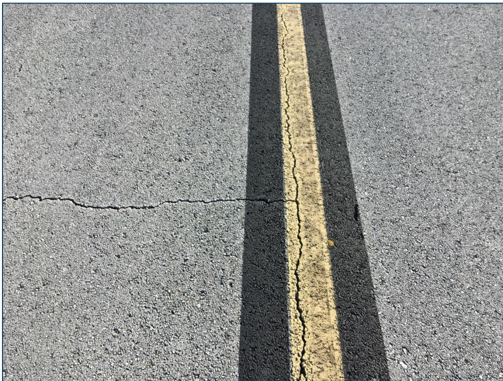
RW 8-26, Section 6205, Sample Unit 128 - Low Severity (48) Longitudinal & Transverse Cracking and Low Severity (57) Weathering
