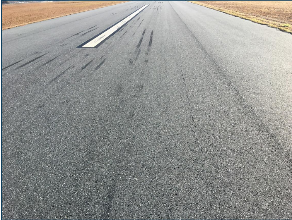
RW 8-26, Section 6205, Sample Unit 104 - Low Severity (48) Longitudinal & Transverse Cracking and Low Severity (57) Weathering
