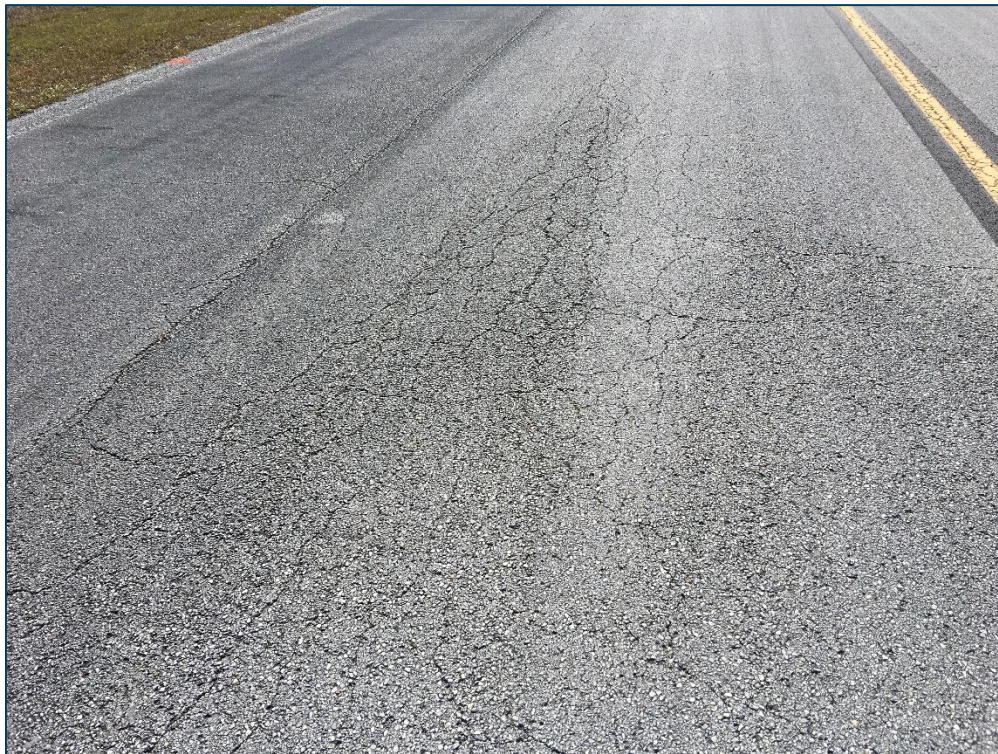
TW A, Section 540, Sample Unit 114 - Low Severity (41) Alligator Cracking, Medium Severity (41) Alligator Cracking, Low Severity (48) Longitudinal & Transverse Cracking, Medium Severity (48) Longitudinal & Transverse Cracking, Low Severity (52) Raveling, Medium Severity (52) Raveling, and Low Severity (53) Rutting
