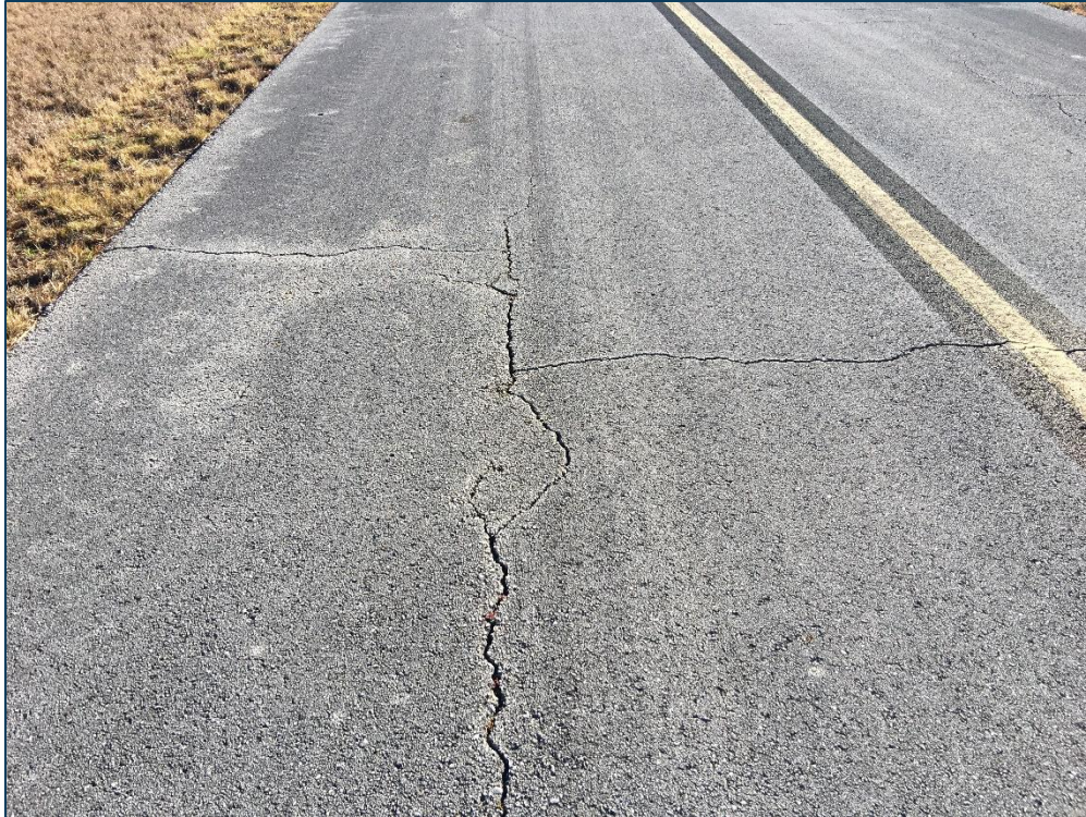
TW B, Section 105, Sample Unit 107 - Low Severity (48) Longitudinal & Transverse Cracking, Medium Severity (48) Longitudinal & Transverse Cracking, and Low Severity (52) Raveling
