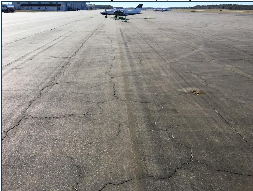
AP CENTER, Section 4120, Sample Unit 515 - Low Severity (43) Block Cracking, Low Severity (48) Longitudinal & Transverse Cracking, and Low Severity (57) Weathering
