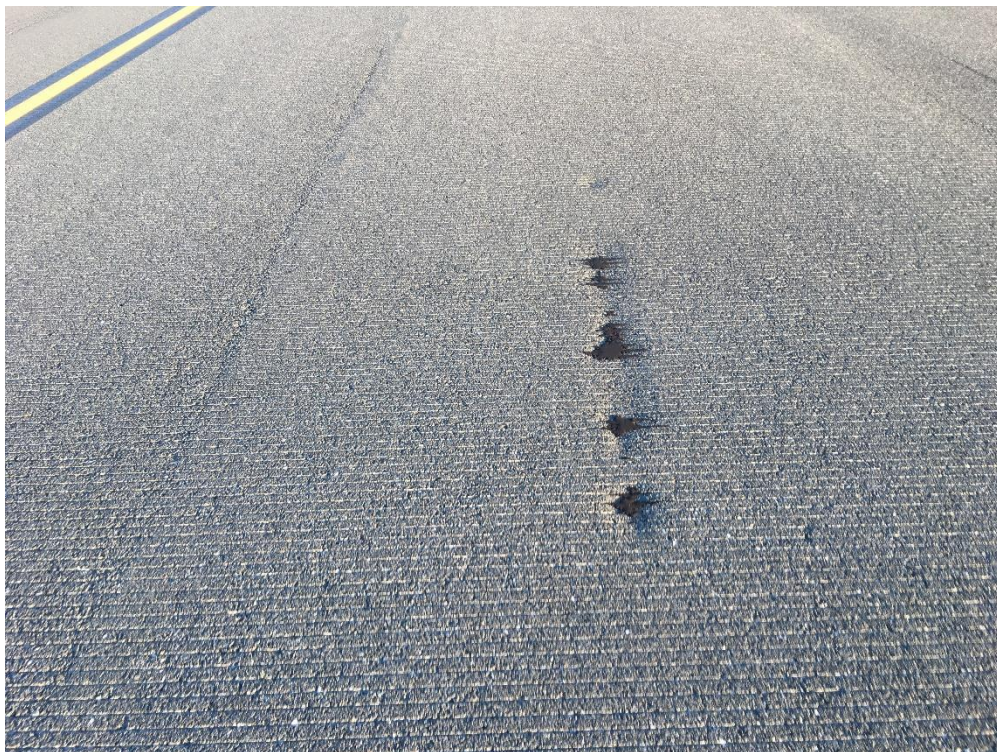
RW 18-36, Section 6105, Sample Unit 362 - (42) Bleeding, Low Severity (48) Longitudinal & Transverse Cracking, and Low Severity (57) Weathering
