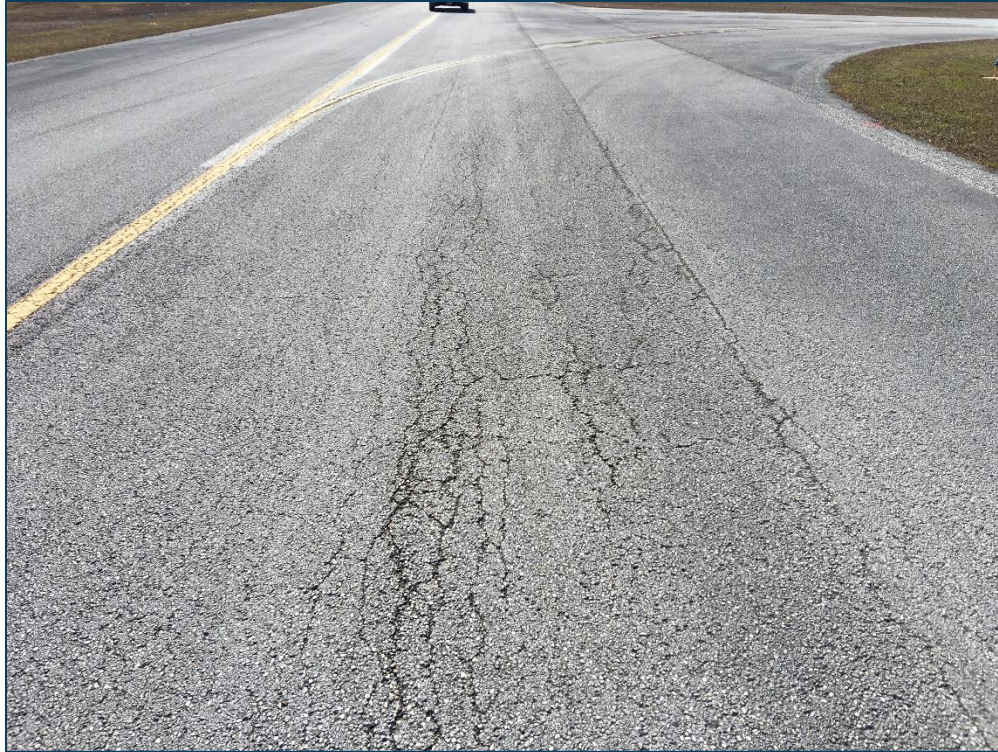
TW A, Section 540, Sample Unit 122 - Low Severity (41) Alligator Cracking, Medium Severity (41) Alligator Cracking, Low Severity (48) Longitudinal & Transverse Cracking, Medium Severity (48) Longitudinal & Transverse Cracking, Low Severity (52) Raveling, and Medium Severity (52) Raveling
