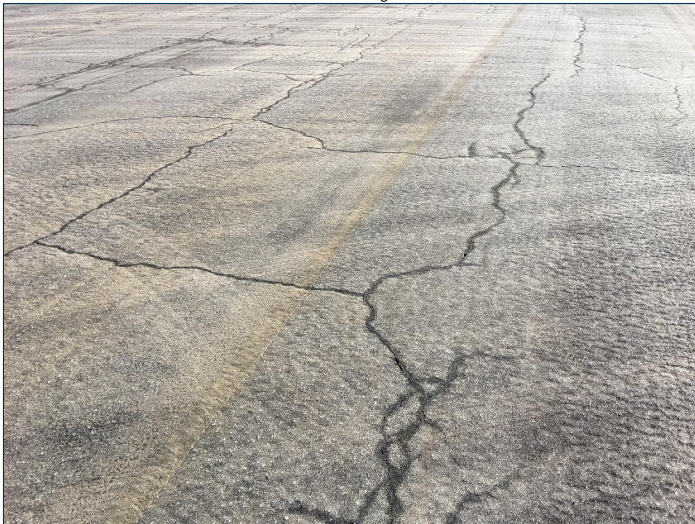
AP N, Section 4210, Sample Unit 700 - Low Severity (43) Block Cracking, Medium Severity (43) Block Cracking, and Low Severity (57) Weathering
