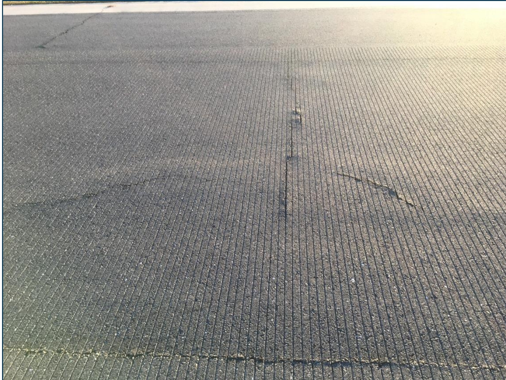
RW 18-36, Section 6110, Sample Unit 564 - Low Severity (48) Longitudinal & Transverse Cracking, Low Severity (56) Swelling, and Low Severity (57) Weathering
