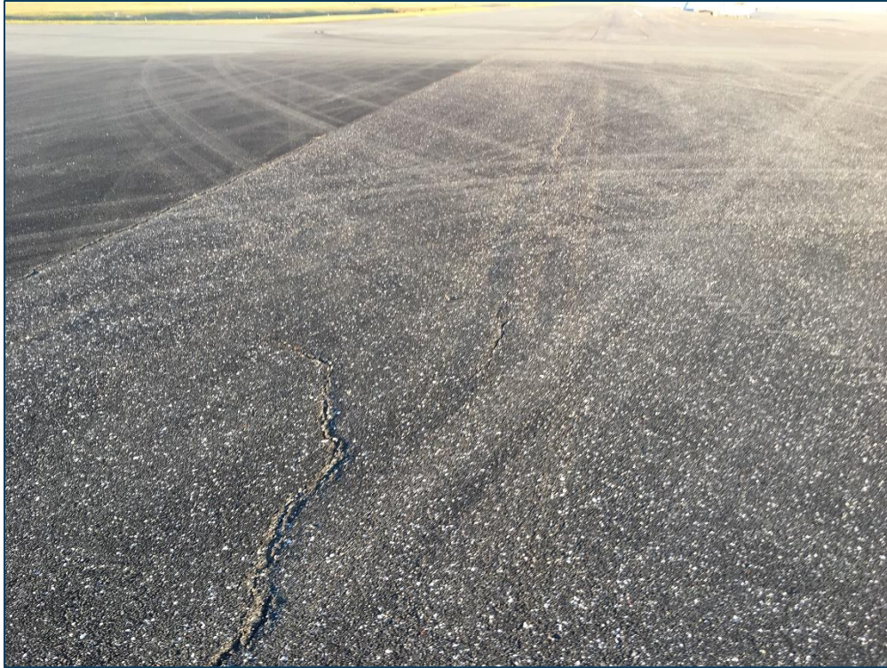
AP CENTER, Section 4105, Sample Unit 104 - Low Severity (48) Longitudinal & Transverse Cracking, Medium Severity (48) Longitudinal & Transverse Cracking, Low Severity (56) Swelling, Low Severity (57) Weathering, and Medium Severity (57) Weathering
