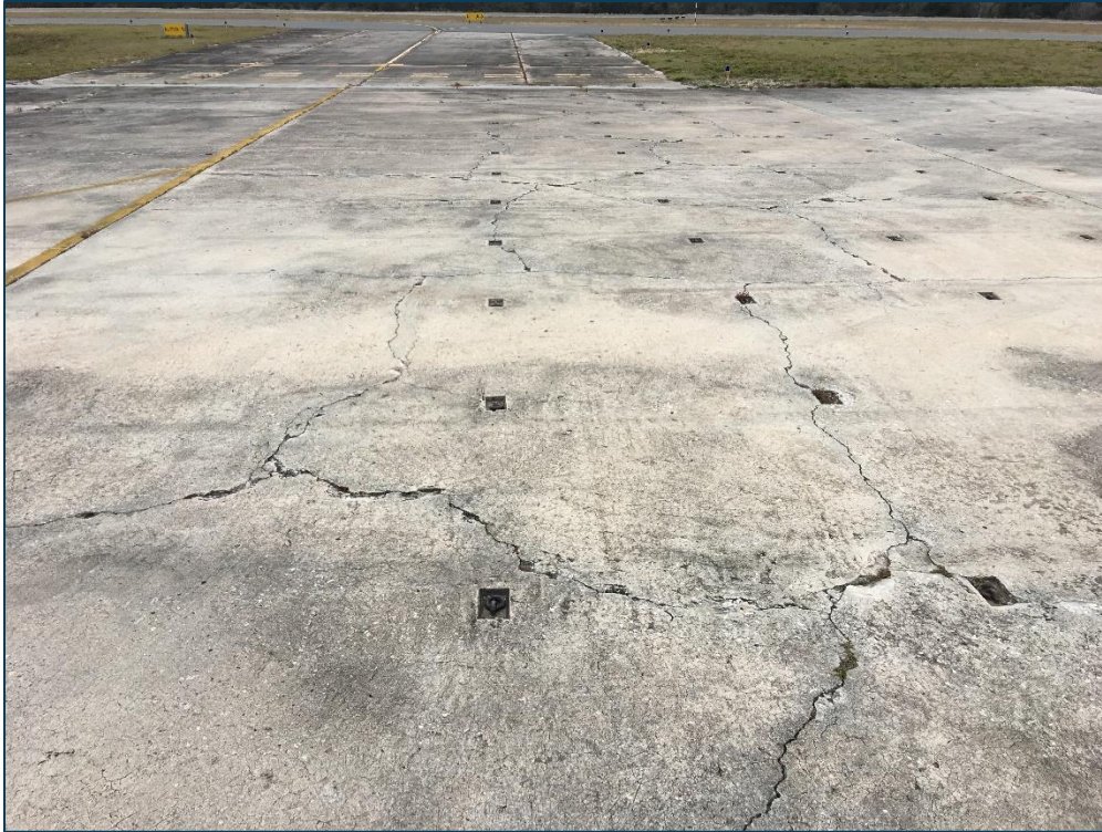
AP N, Section 4140, Sample Unit 602 - Medium Severity (72) Shattered Slab
