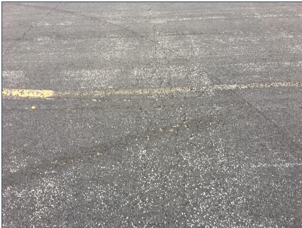
AP N, Section 4105, Sample Unit 158 - Medium Severity (41) Alligator Cracking, Low Severity (48) Longitudinal & Transverse Cracking, Low Severity (52) Raveling, and Low Severity (57) Weathering
