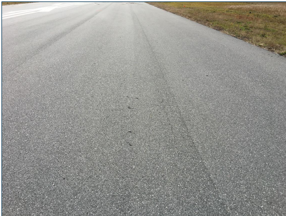
RW 3-21, Section 6210, Sample Unit 500 - (42) Bleeding, Low Severity (48) Longitudinal & Transverse Cracking, and Low Severity (57) Weathering
