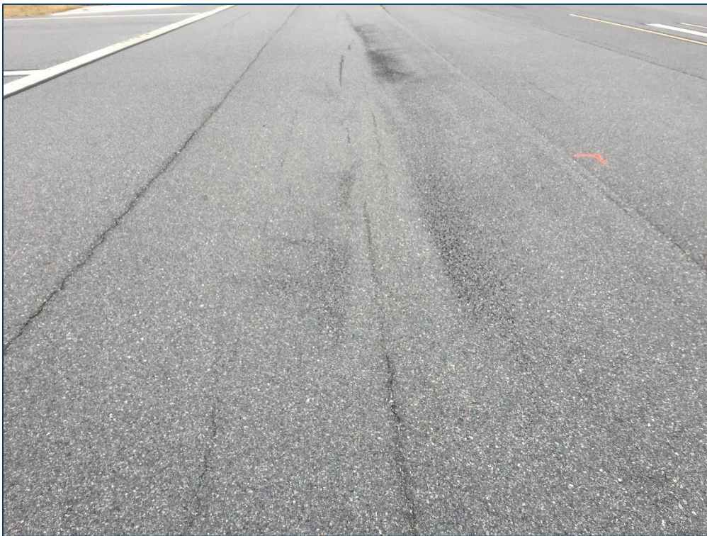
RW 13-31, Section 6110, Sample Unit 120 - (42) Bleeding, Low Severity (48) Longitudinal & Transverse Cracking, Medium Severity (48) Longitudinal & Transverse Cracking, and Medium Severity (52) Raveling
