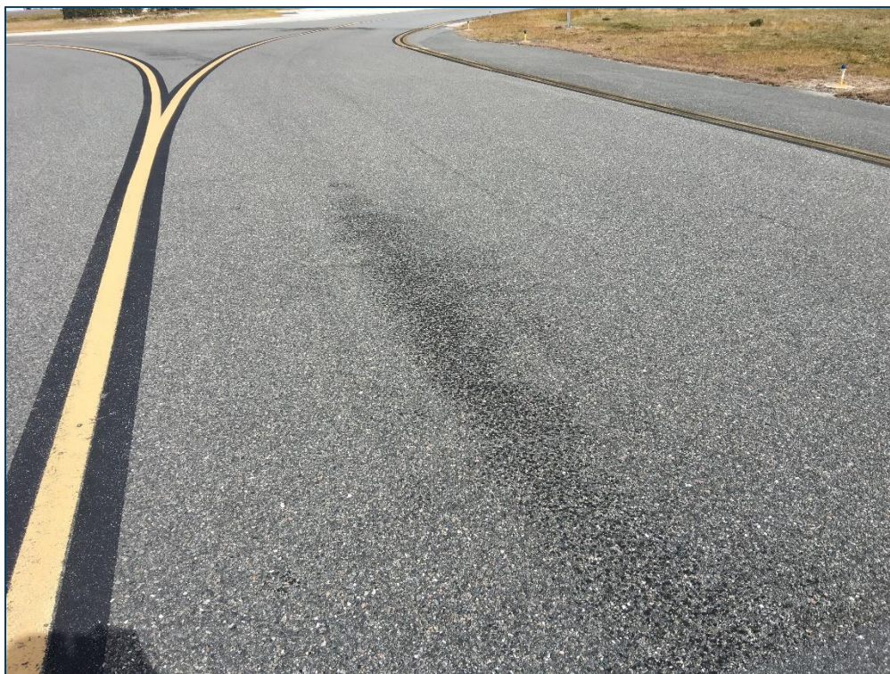
TW B, Section 205, Sample Unit 106 - (42) Bleeding, Low Severity (48) Longitudinal & Transverse Cracking, and Low Severity (52) Raveling
