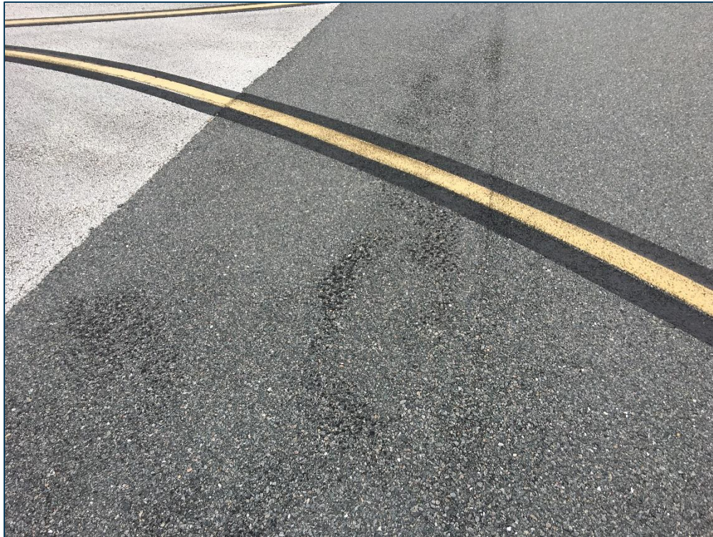
TW A, Section 110, Sample Unit 228 - (42) Bleeding, Low Severity (48) Longitudinal & Transverse Cracking, Low Severity (52) Raveling, and Low Severity (57) Weathering
