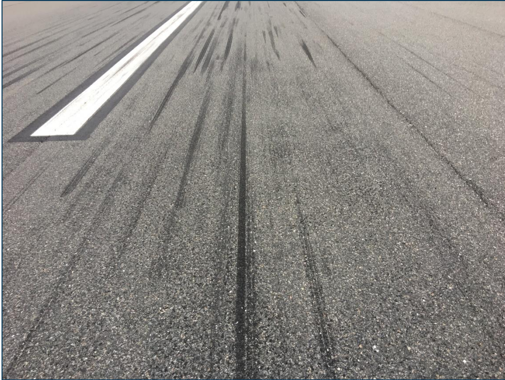
RW 13-31, Section 6105, Sample Unit 354 - (42) Bleeding, Low Severity (48) Longitudinal & Transverse Cracking, and Low Severity (57) Weathering
