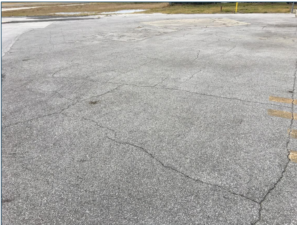
AP RFUEL, Section 4505, Sample Unit 301 - Low Severity (43) Block Cracking, Low Severity (45) Depression, Medium Severity (50) Patching, High Severity (50) Patching, Low Severity (52) Raveling, and Medium Severity (52) Raveling
