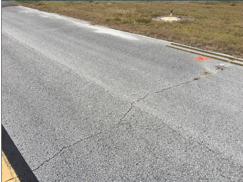
TW K, Section 715, Sample Unit 122 - Low Severity (48) Longitudinal & Transverse Cracking, Medium Severity (48) Longitudinal & Transverse Cracking, Low Severity (52) Raveling, and Low Severity (57) Weathering
