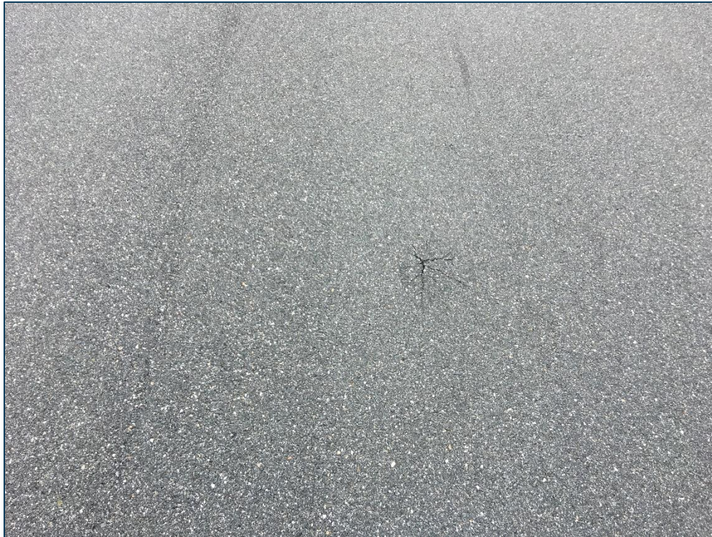
RW 3-21, Section 6205, Sample Unit 331 - Low Severity (48) Longitudinal & Transverse Cracking, Low Severity (56) Swelling, and Low Severity (57) Weathering
