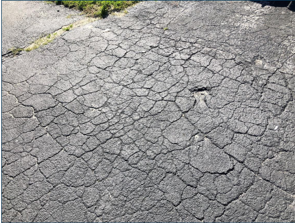
AP E, Section 4305, Sample Unit 101 - Medium Severity (41) Alligator Cracking, High Severity (41) Alligator Cracking, and Low Severity (52) Raveling
