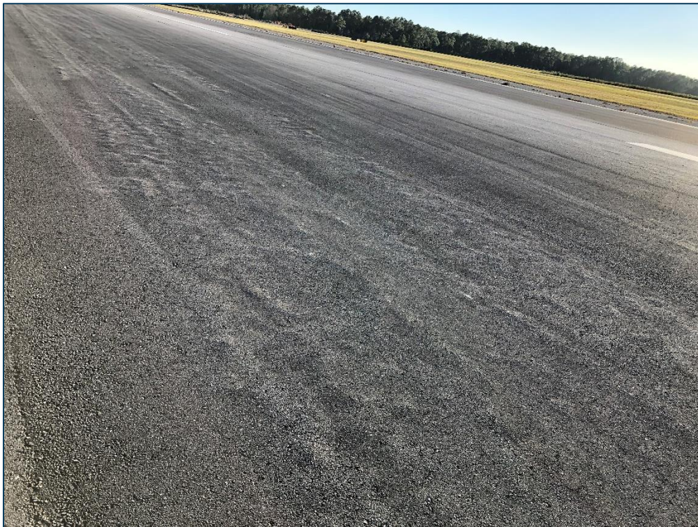
RW 17-35, Section 6205, Sample Unit 165 - Low Severity (52) Raveling, Low Severity (56) Swelling, and Low Severity (57) Weathering
