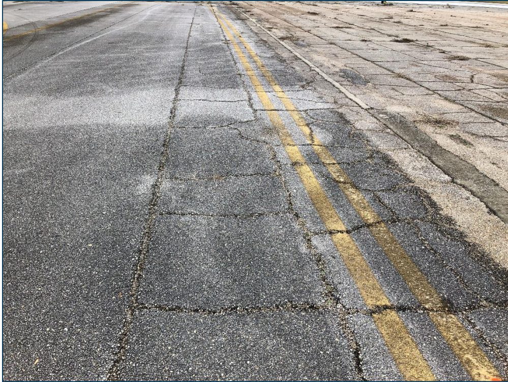
TW D, Section 405, Sample Unit 101 - Medium Severity (43) Block Cracking and Low Severity (52) Raveling
