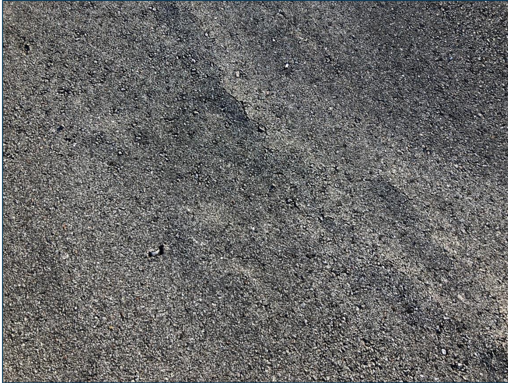
RW 17-35, Section 6205, Sample Unit 159 - Low Severity (48) Longitudinal & Transverse Cracking, Low Severity (52) Raveling, Low Severity (56) Swelling, and Low Severity (57) Weathering
