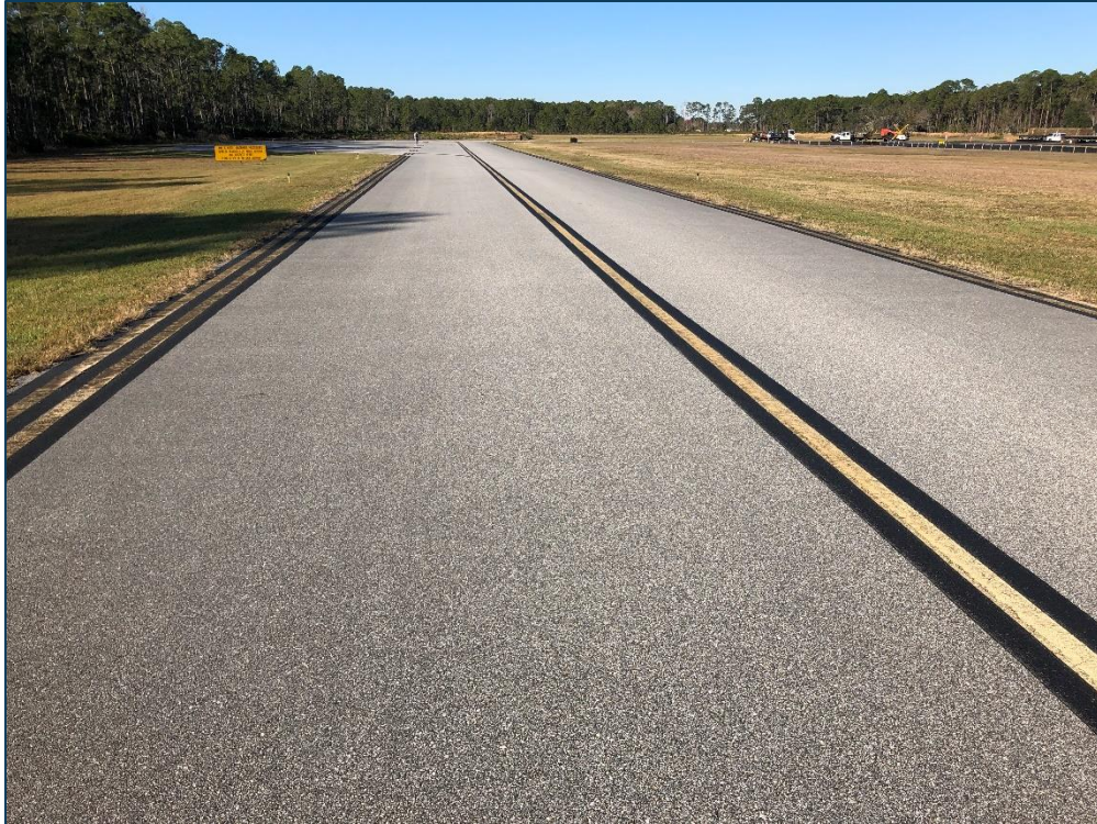
TW A, Section 100, Sample Unit 107 - Low Severity (57) Weathering
