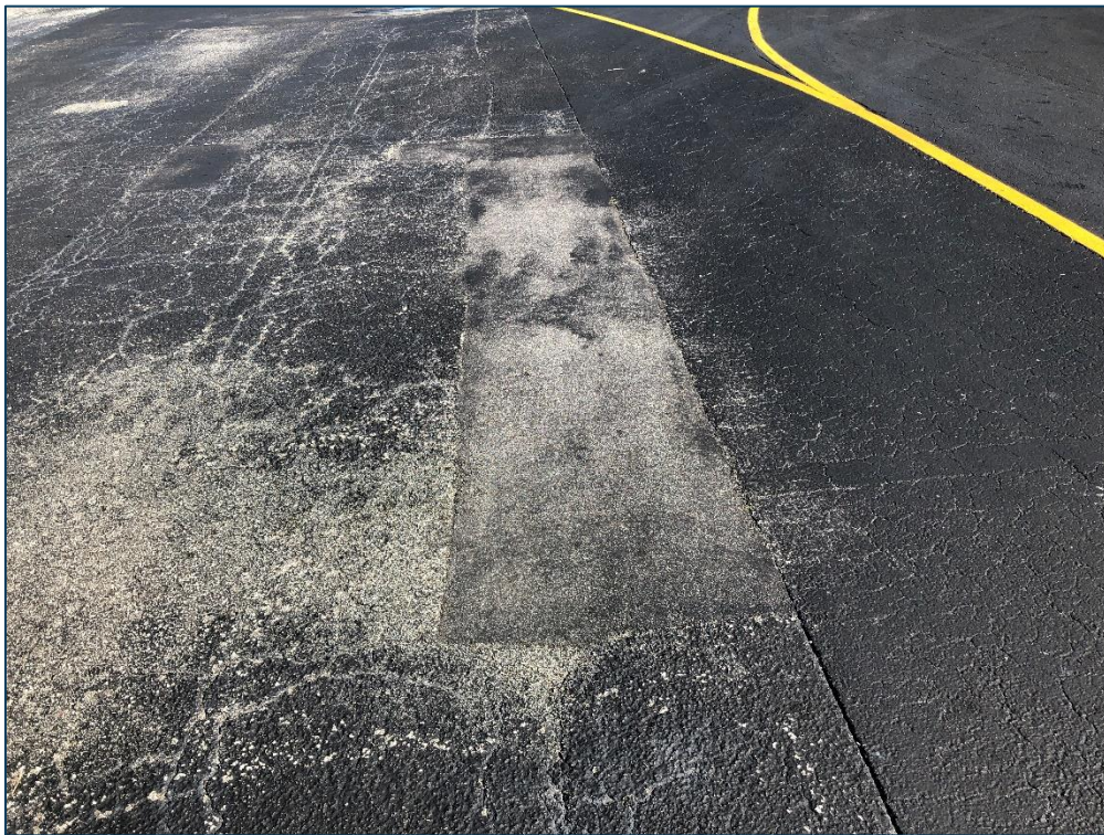
AP CENTER, Section 4205, Sample Unit 111 - Low Severity (48) Longitudinal & Transverse Cracking, Low Severity (50) Patching, Low Severity (52) Raveling, and Medium Severity (52) Raveling
