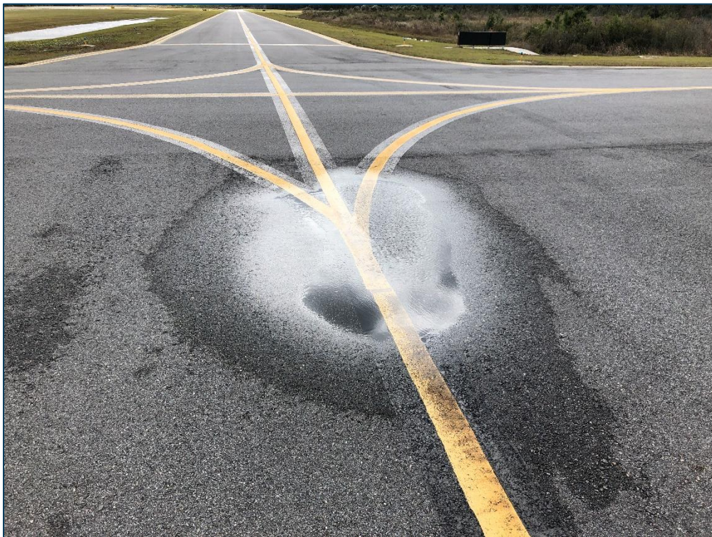
TW G, Section 700, Sample Unit 115 - Low Severity (45) Depression and Low Severity (57) Weathering
