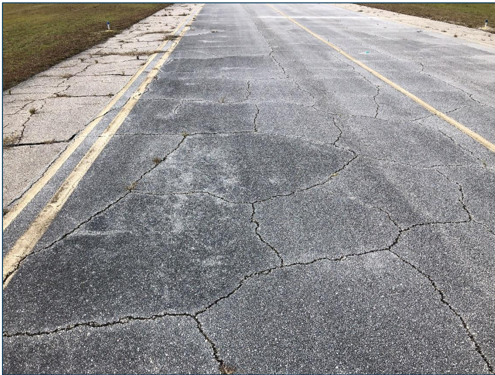
TW E, Section 505, Sample Unit 107 - Medium Severity (43) Block Cracking and Low Severity (52) Raveling
