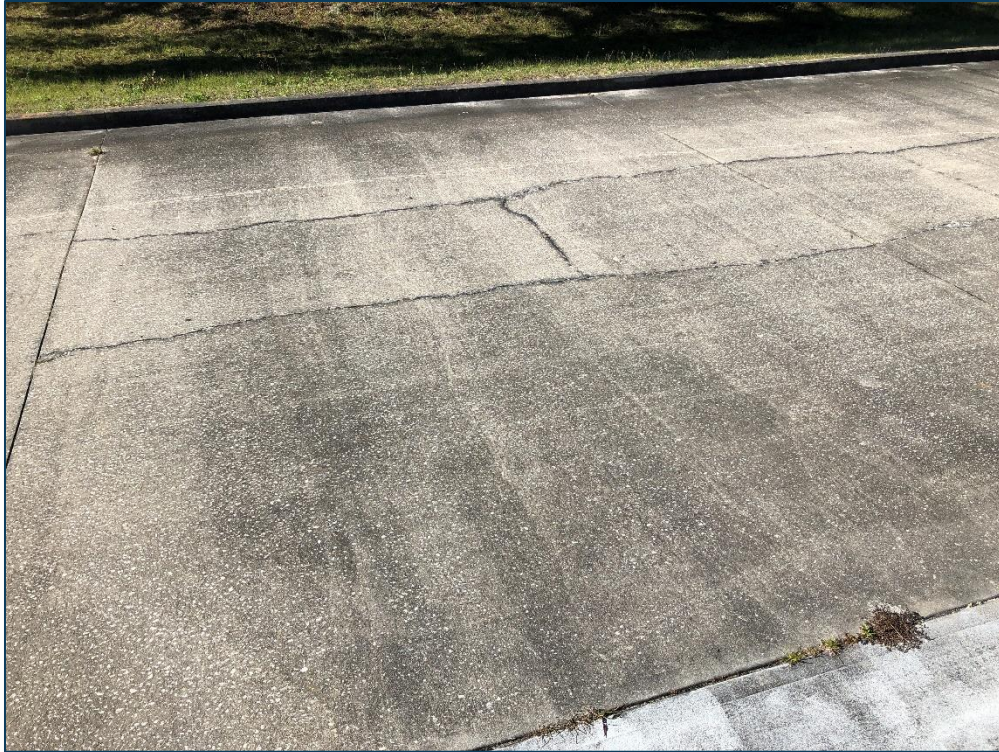
TW T-HANG, Section 2004, Sample Unit 602 - High Severity (65) Joint Seal Damage and Low Severity (72) Shattered Slab
