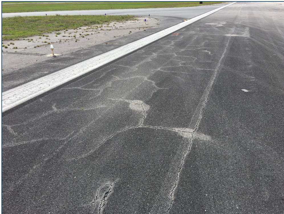
RUNWAY 9-27, Section 6210, Sample Unit 148 - Low Severity (43) Block Cracking, Low Severity (48) Longitudinal & Transverse Cracking, and Low Severity (57) Weathering
