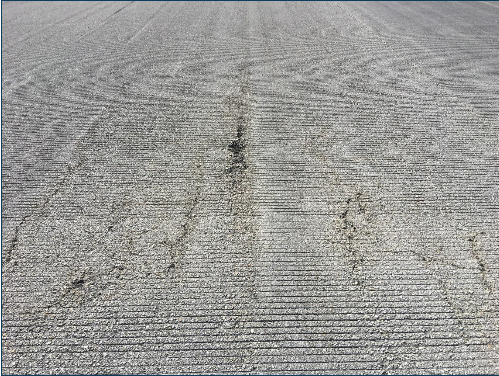
RW 18-36, Section 6105, Sample Unit 386 - Severity (48) Longitudinal & Transverse Cracking, High Severity (48) Longitudinal & Transverse Cracking, Low Severity (52) Raveling, and Medium Severity (52) Raveling
