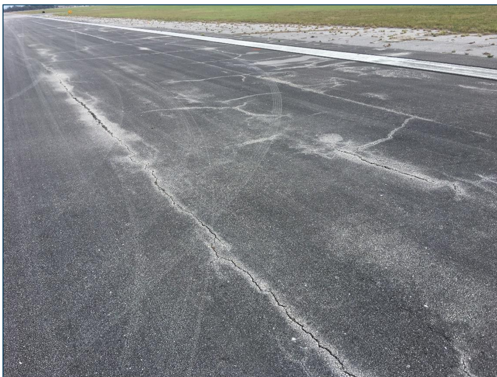
RW 9-27, Section 6210, Sample Unit 162 - Low Severity (43) Block Cracking, Low Severity (48) Longitudinal & Transverse Cracking, Medium Severity (48) Longitudinal & Transverse Cracking, Low Severity (57) Weathering, and Medium Severity (57) Weathering
