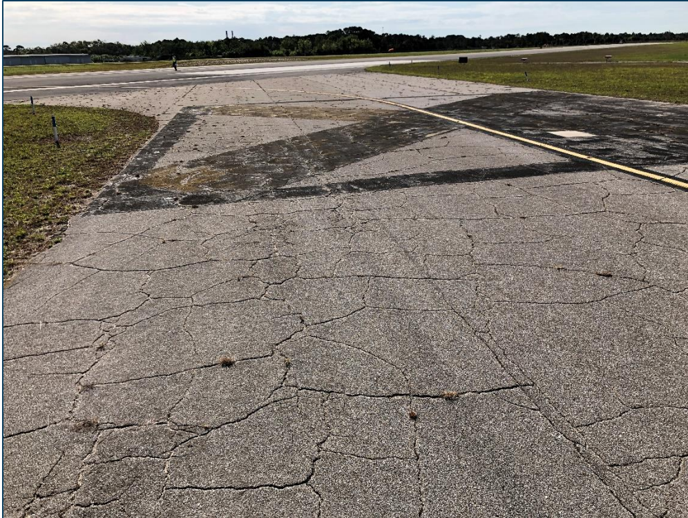
TW F, Section 605, Sample Unit 301 - Medium Severity (43) Block Cracking, Low Severity (50) Patching, and Medium Severity (52) Raveling
