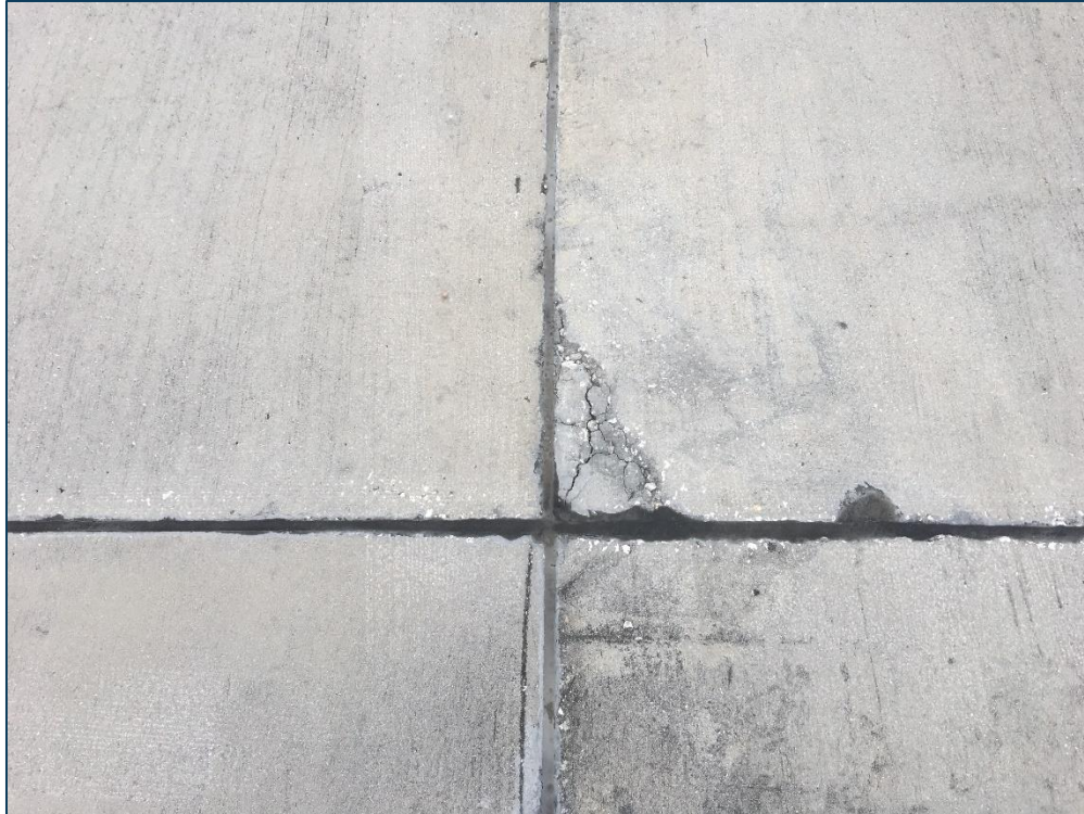
AP HELI, Section 4260, Sample Unit 643 – Low Severity (75) Corner Spall
