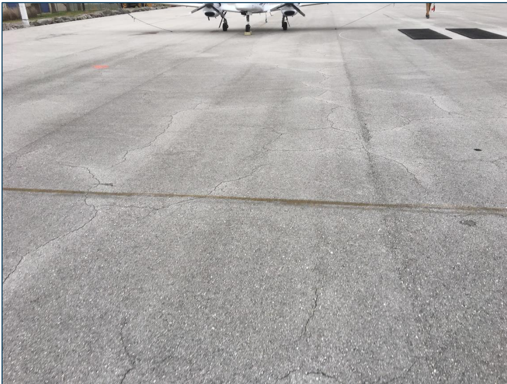
AP E, Section 4205, Sample Unit 250 - Low Severity (43) Block Cracking, Low Severity (48) Longitudinal & Transverse Cracking, and Low Severity (57) Weathering
