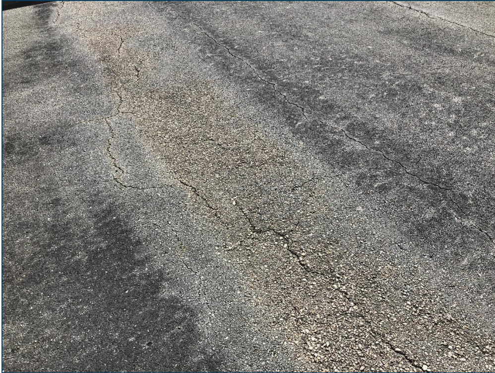
TW A, Section 120, Sample Unit 162 - Low Severity (48) Longitudinal & Transverse Cracking, Medium Severity (48) Longitudinal & Transverse Cracking, Low Severity (52) Raveling, and Medium Severity (57) Weathering
