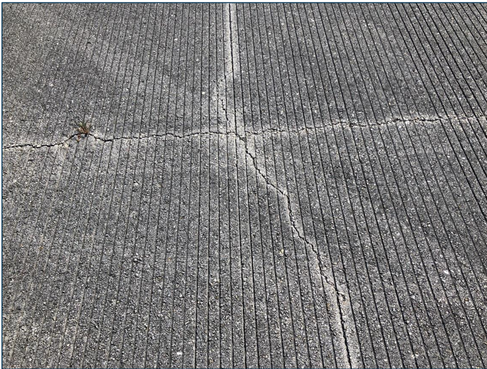
RW 18-36, Section 6110, Sample Unit 176 - Low Severity (48) Longitudinal & Transverse Cracking, Low Severity (52) Raveling, and Low Severity (57) Weathering
