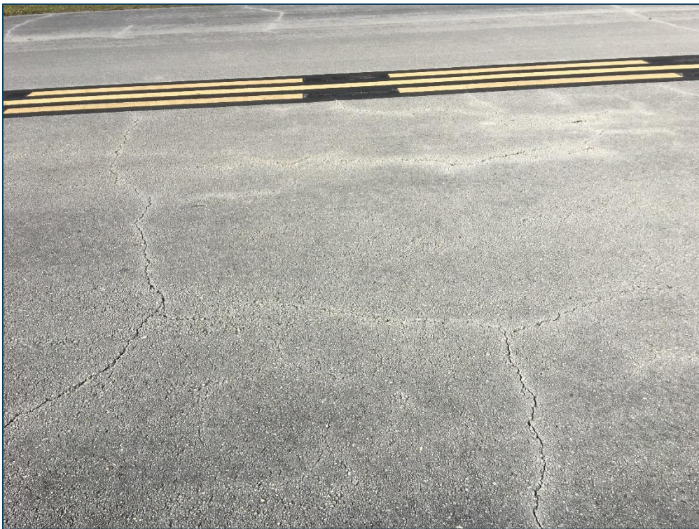
TW B, Section 205, Sample Unit 502 - Low Severity (43) Block Cracking, Low Severity (48) Longitudinal & Transverse Cracking, Low Severity (52) Raveling, and Medium Severity (57) Weathering
