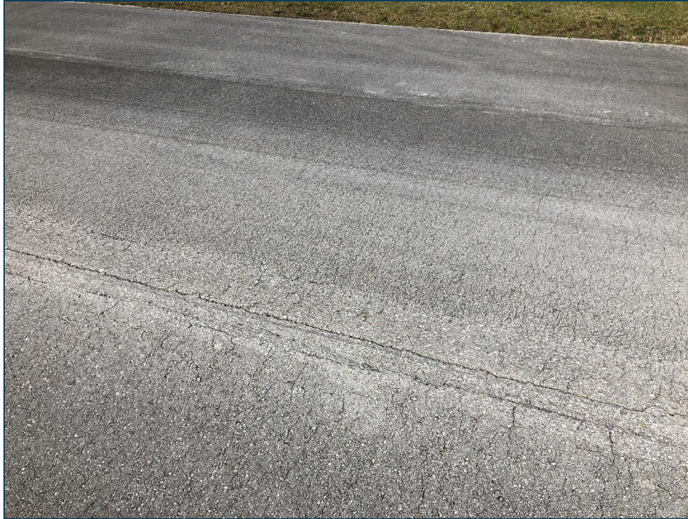
TW K, Section 1135, Sample Unit 187 - Low Severity (48) Longitudinal & Transverse Cracking, Low Severity (52) Raveling, and Low Severity (57) Weathering
