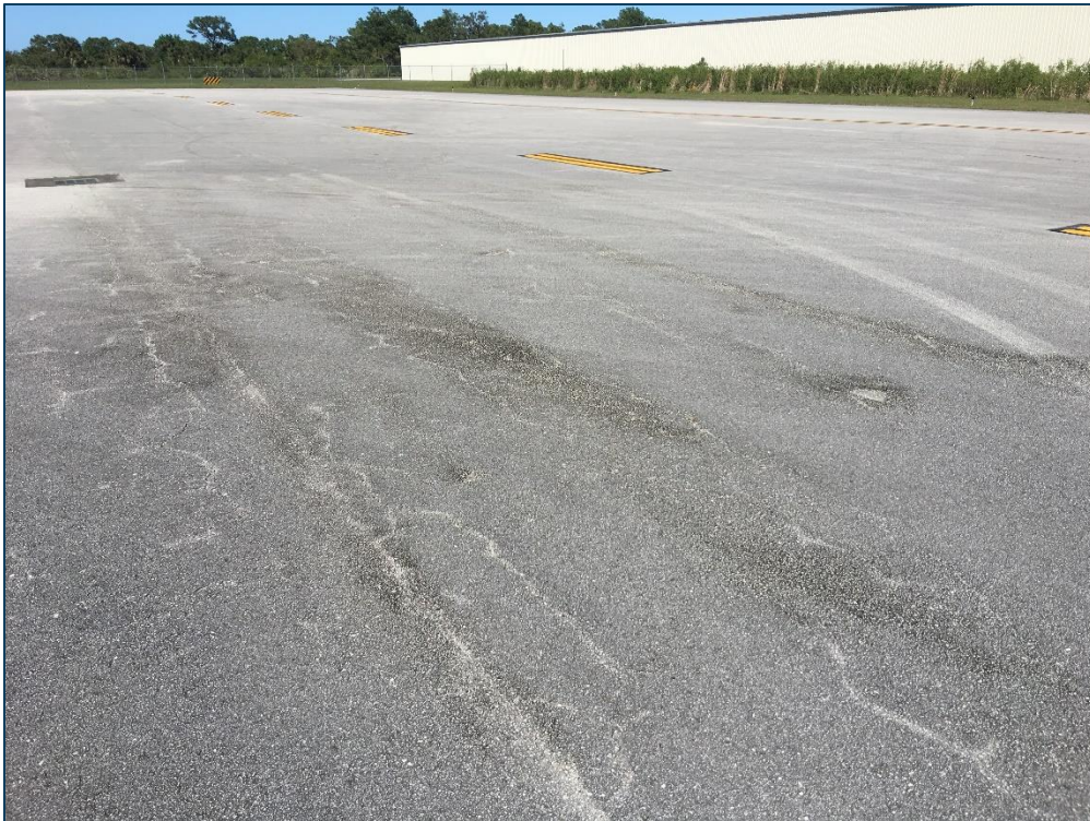
AP N GA, Section 4120, Sample Unit 402 - Low Severity (48) Longitudinal & Transverse Cracking, Medium Severity (48) Longitudinal & Transverse Cracking, Low Severity (52) Raveling, and Medium Severity (52) Raveling
