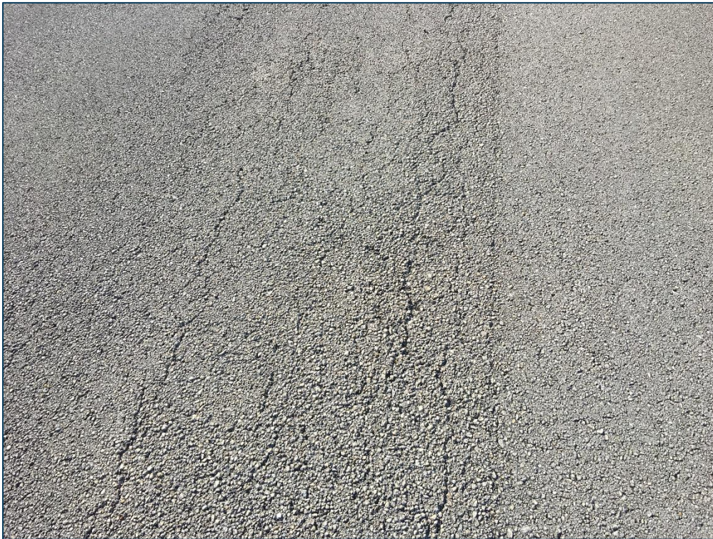
TW C, Section 330, Sample Unit 113 - Low Severity (41) Alligator Cracking, Low Severity (52) Raveling, Low Severity (56) Swelling, and Low Severity (57) Weathering
