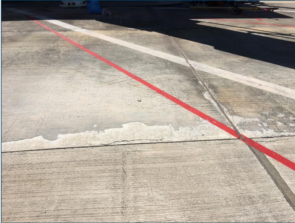
AP TERM, Section 4205, Sample Unit 202 - Low Severity (70) Scaling, (73) Shrinkage Cracking, and Low Severity (74) Joint Spall
