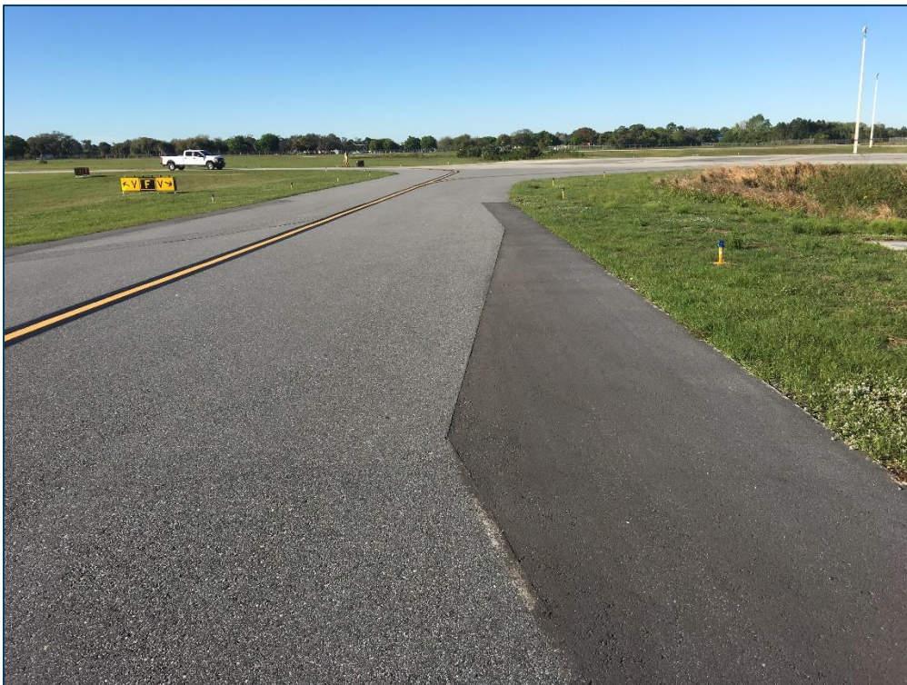
TW F, Section 810, Sample Unit 101 - Low Severity (50) Patching and Low Severity (57) Weathering
