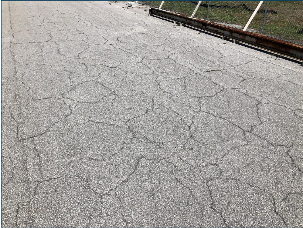
AP E, Section 4406, Sample Unit 810 - Low Severity (43) Block Cracking, Low Severity (52) Raveling, and Low Severity (57) Weathering
