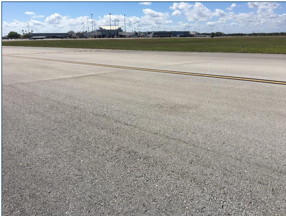
AP E, Section 4407, Sample Unit 103 - Low Severity (48) Longitudinal & Transverse Cracking, Low Severity (53) Rutting, Low Severity (56) Swelling, and Low Severity (57) Weathering
