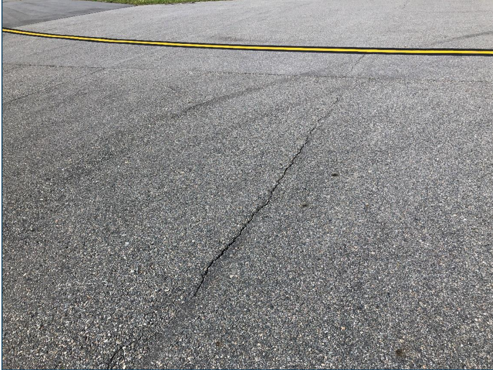
TW A, Section 120, Sample Unit 101 - Low Severity (48) Longitudinal & Transverse Cracking, Medium Severity (48) Longitudinal & Transverse Cracking, Low Severity (52) Raveling, Low Severity (56) Swelling, and Low Severity (57) Weathering
