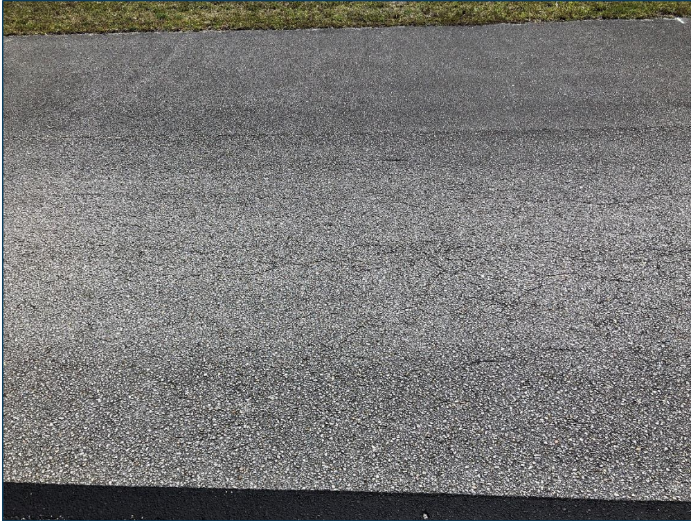
TW D, Section 410, Sample Unit 123 - Low Severity (41) Alligator Cracking, Low Severity (48) Longitudinal & Transverse Cracking, Low Severity (52) Raveling, and Low Severity (57) Weathering
