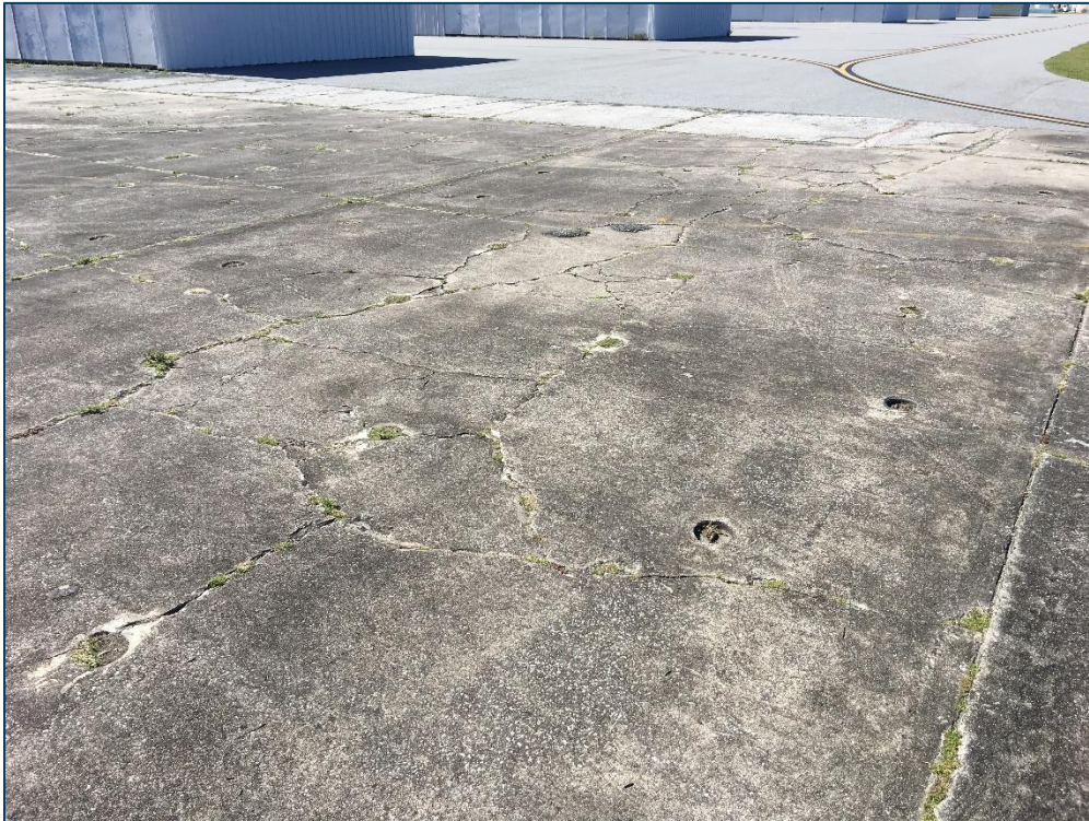
AP W, Section 4325, Sample Unit 200 - High Severity (65) Joint Seal Damage, Medium Severity (72) Shattered Slab, and High Severity (72) Shattered Slab
