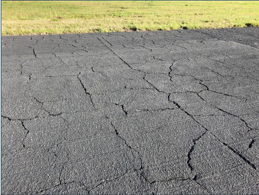
AP GA, Section 4205, Sample Unit 109 - Medium Severity (43) Block Cracking, Low Severity (52) Raveling, and Low Severity (56) Swelling
