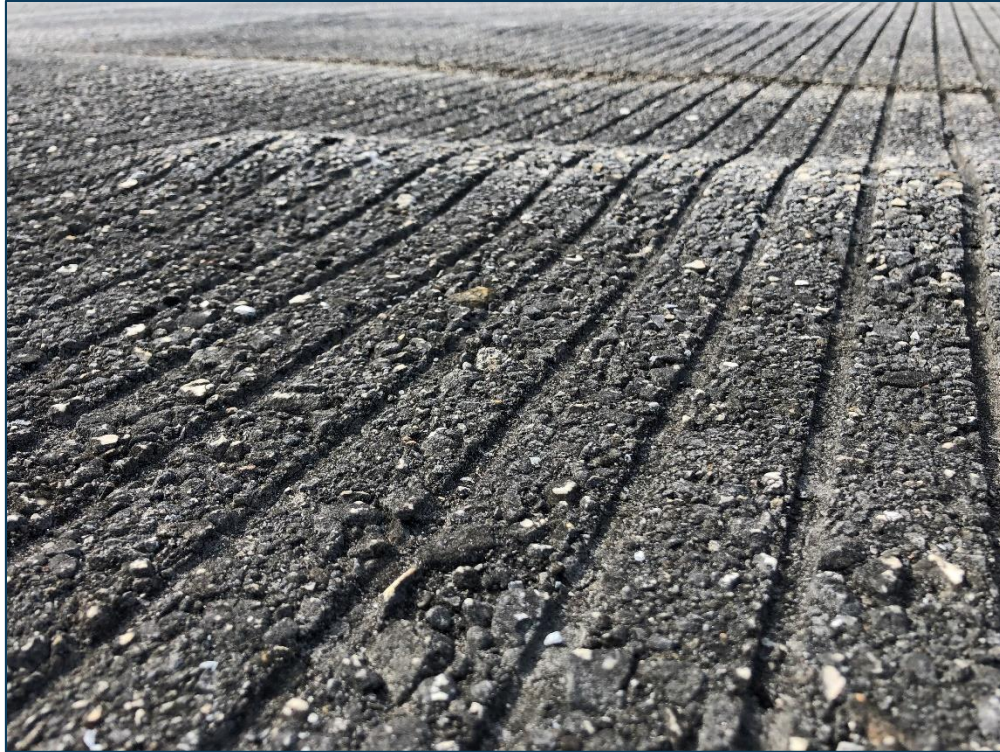
RW 13-31, Section 6205, Sample Unit 156 – Low Severity (52) Raveling, Medium Severity (56) Swelling, and Low Severity (57) Weathering
