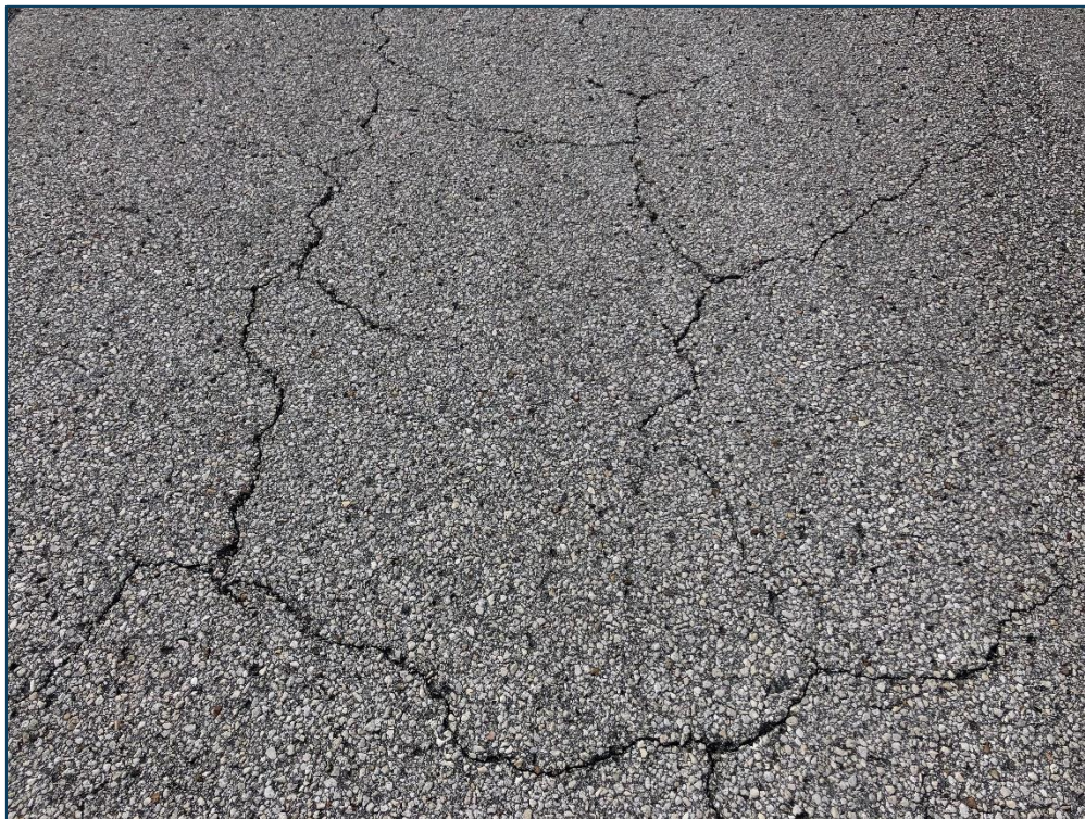
TWF, Section 605, Sample Unit 611 - Low Severity (43) Block Cracking, and Low Severity (52) Raveling.
