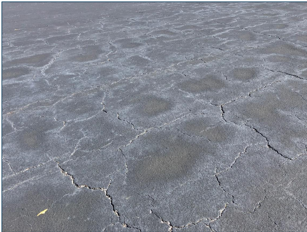
AP W, Section 4610, Sample Unit 531 - Medium Severity (43) Block Cracking, Low Severity (52) Raveling, and Low Severity (56) Swelling
