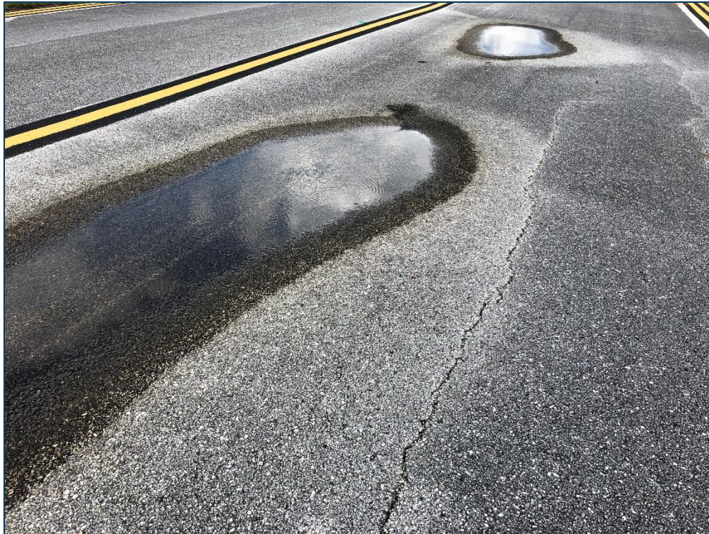
TWE3, Section 420, Sample Unit 405 - Medium Severity (45) Depression, Medium Severity (48) Longitudinal & Transverse Cracking, and Low Severity (52) Raveling
