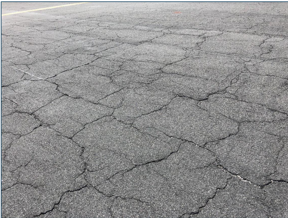
AP N, Section 4125, Sample Unit 513 - Medium Severity (43) Block Cracking and Medium Severity (52) Raveling
