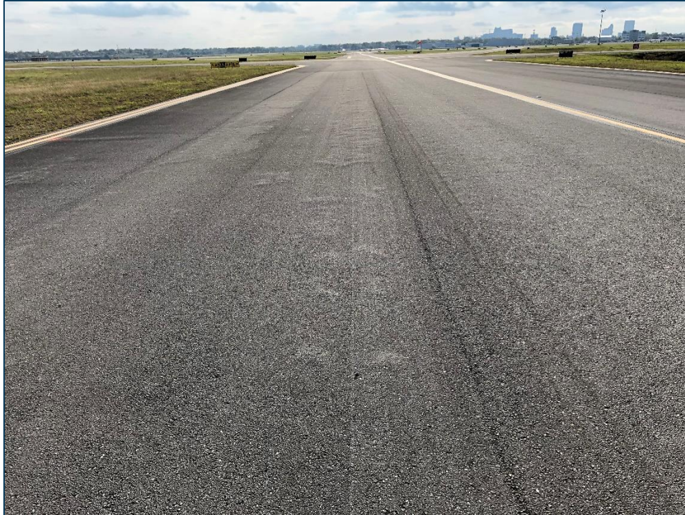
TWA, Section 125, Sample Unit 166 - Low Severity (48) Longitudinal & Transverse Cracking, Low Severity (52) Raveling, Low Severity (56) Swelling, and Low Severity (57) Weathering
