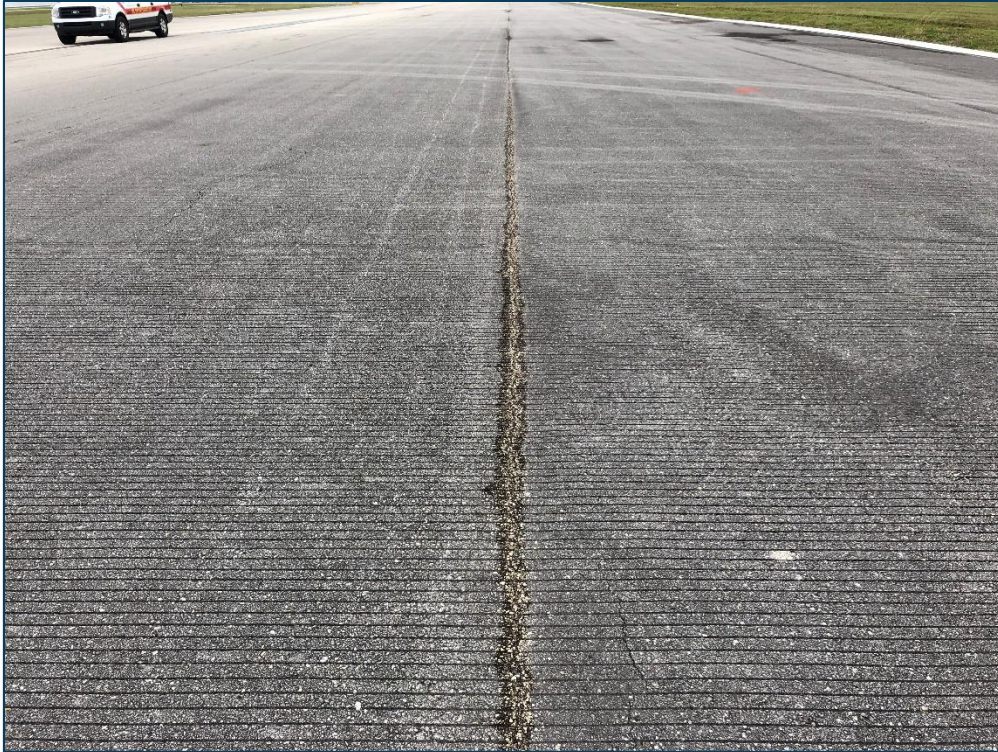
RW 7-25, Section 6105, Sample Unit 361 - Medium Severity (48) Longitudinal & Transverse Cracking, Low Severity (52) Raveling, Low Severity (56) Swelling, and Low Severity (57) Weathering
