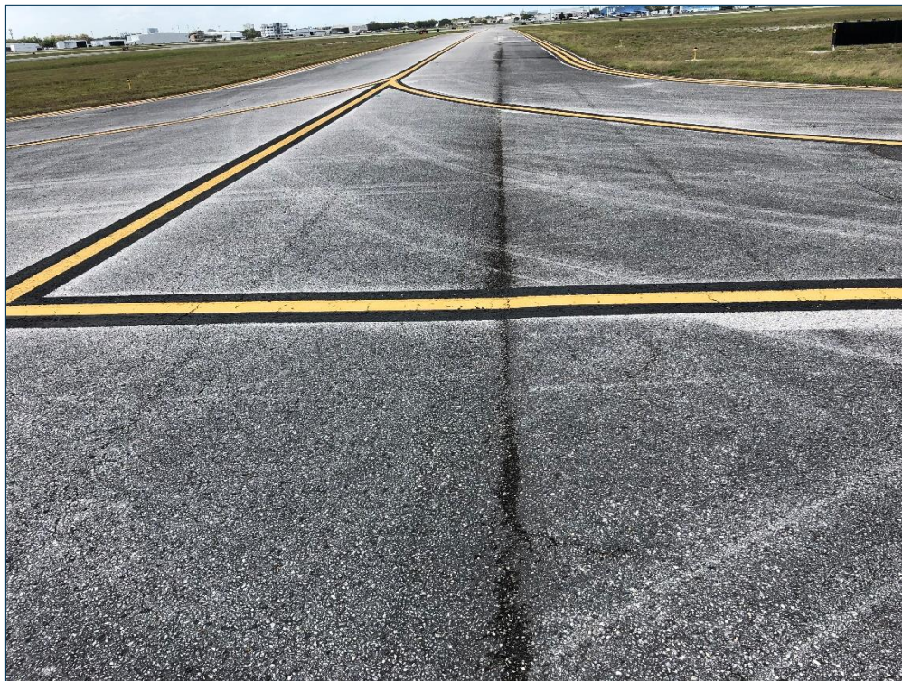
TWE, Section 505, Sample Unit 112 - Medium Severity (48) Longitudinal & Transverse Cracking, and Low Severity (52) Raveling
