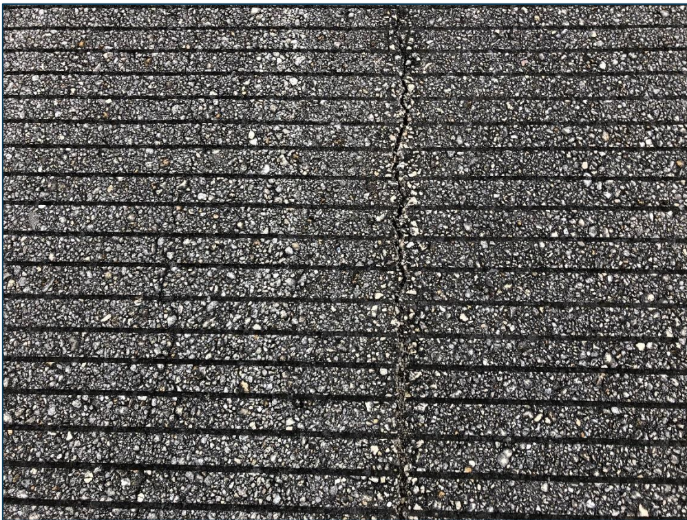
RW 7-25, Section 6105, Sample Unit 403 - Low Severity (48) Longitudinal & Transverse Cracking, Medium Severity (48) Longitudinal & Transverse Cracking, Low Severity (52) Raveling, and Low Severity (57) Weathering
