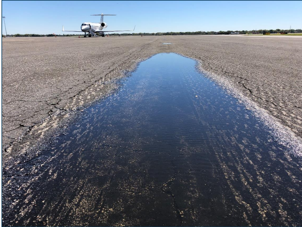
AP N, Section 4125, Sample Unit 210 - Medium Severity (41) Alligator Cracking, Medium Severity (52) Raveling, and Medium Severity (53) Rutting
