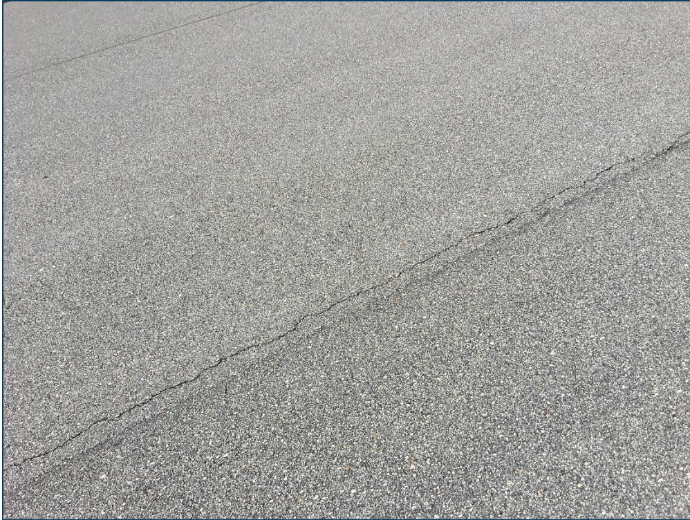
RW 11-29, Section 6105, Sample Unit 125 - Low Severity (48) Longitudinal & Transverse Cracking and Low Severity (57) Weathering
