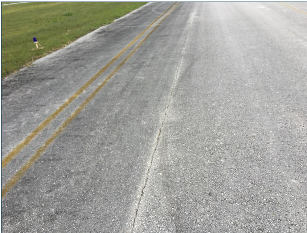
TW B, Section 215, Sample Unit 123 - Low Severity (48) Longitudinal & Transverse Cracking, Low Severity (52) Raveling, and Low Severity (57) Weathering
