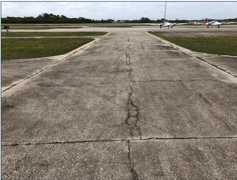
AP, Section 4115, Sample Unit 101 - Low Severity (63) Linear Cracking, Medium Severity (63) Linear Cracking, High Severity (65) Joint Seal Damage, and Low Severity (72) Shattered Slab
