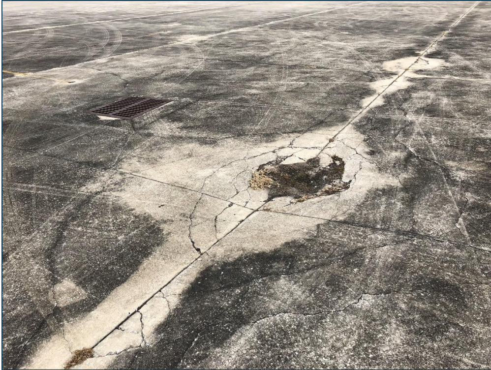
AP, Section 4102, Sample Unit 101 - Low Severity (62) Corner Break, Medium Severity (62) Corner Break, High Severity (62) Corner Break, High Severity (65) Joint Seal Damage, and Medium Severity (74) Joint Spall
