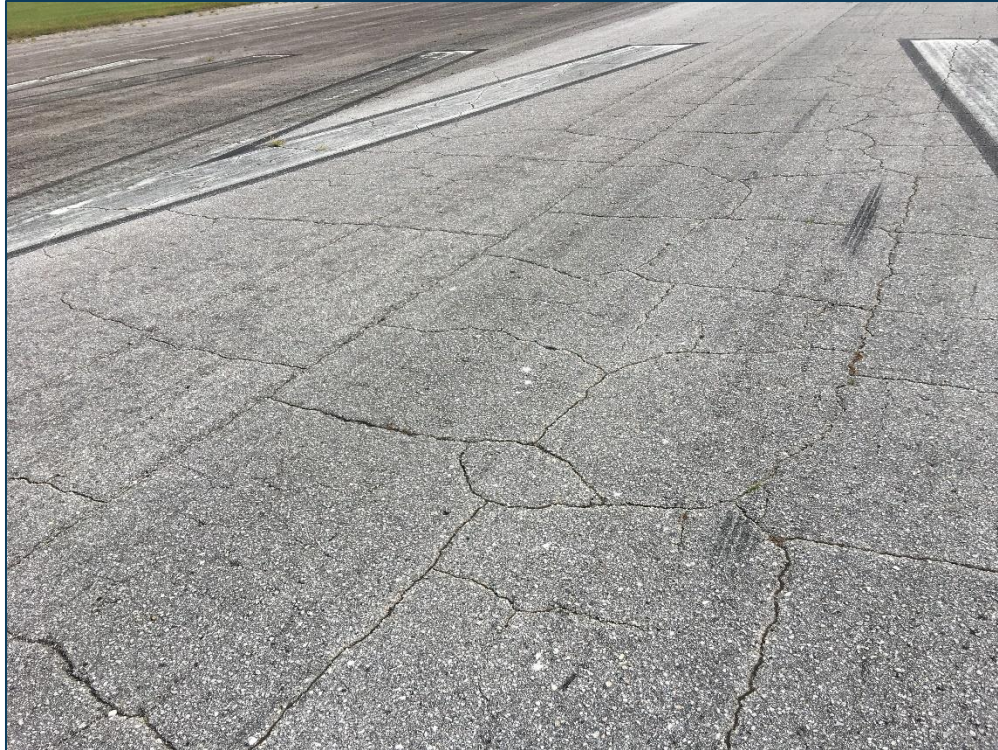
RW 2-20, Section 6405, Sample Unit 114 - Medium Severity (43) Block Cracking, Low Severity (52) Raveling, and Medium Severity (52) Raveling
