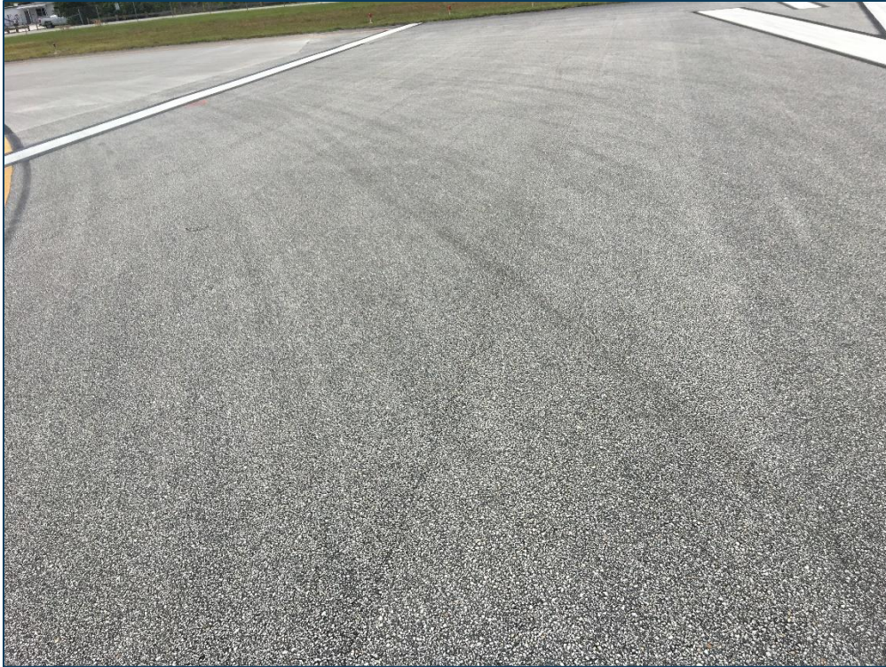
RW 7-25, Section 6202, Sample Unit 101 - Low Severity (48) Longitudinal & Transverse Cracking, Low Severity (52) Raveling, and Low Severity (57) Weathering
