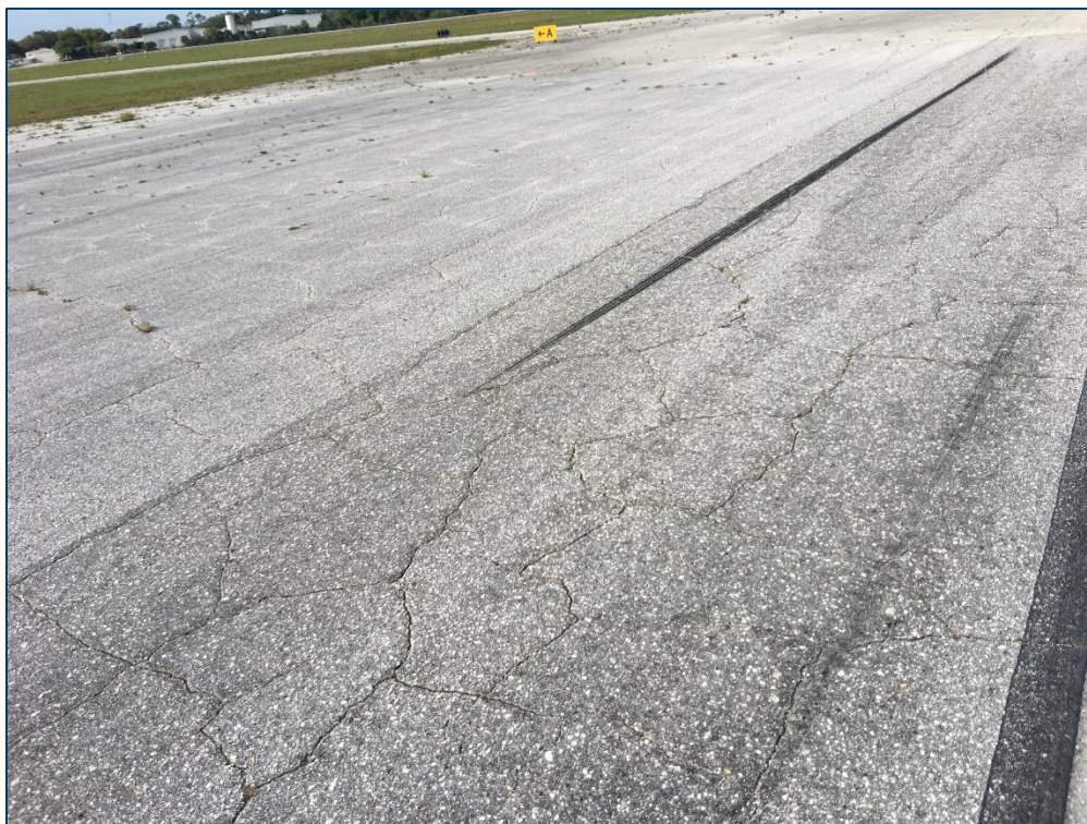
RW 2-20, Section 6425, Sample Unit 146 - Low Severity (43) Block Cracking, Medium Severity (43) Block Cracking, Low Severity (52) Raveling, and Medium Severity (52) Raveling
