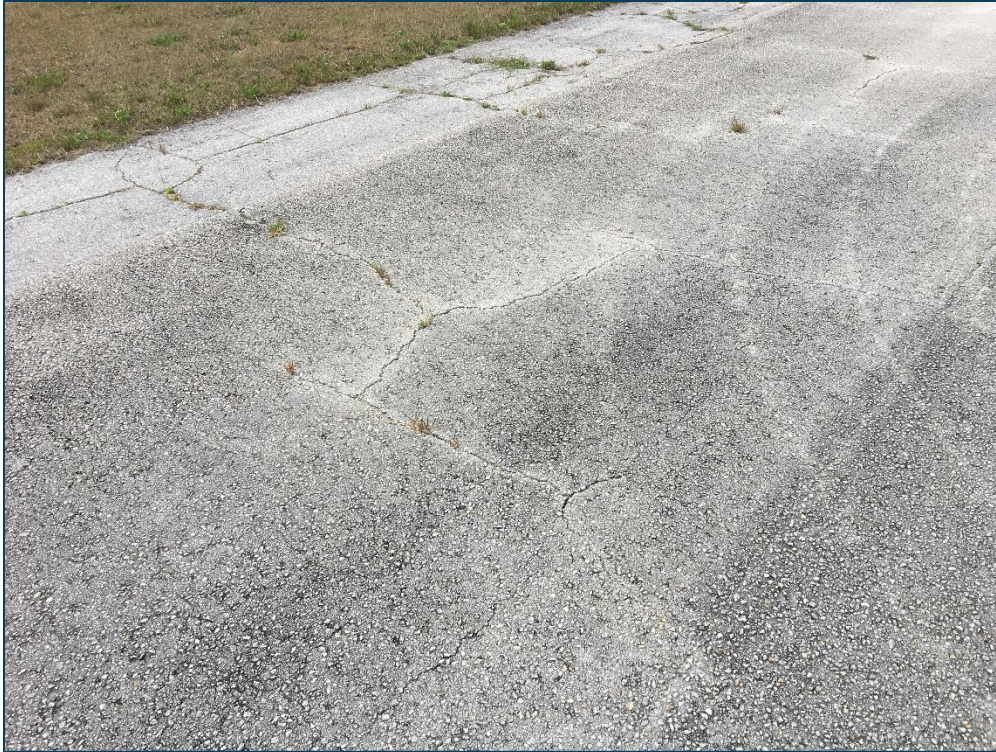
TW A, Section 105, Sample Unit 133 - Low Severity (43) Block Cracking, Low Severity (48) Longitudinal & Transverse Cracking, and Low Severity (52) Raveling
