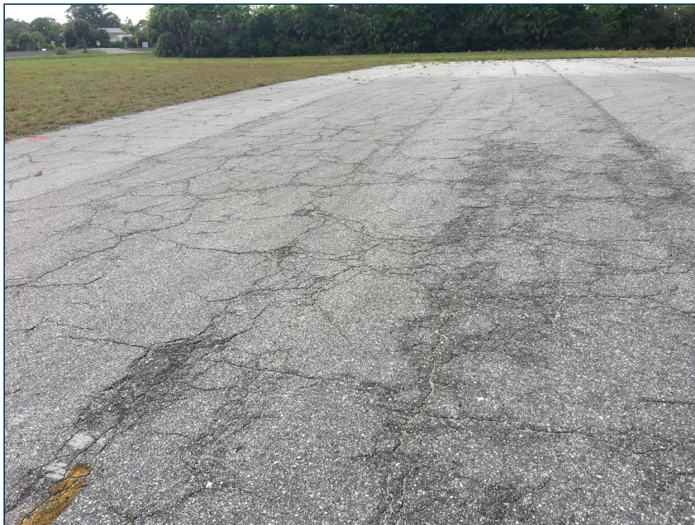
TW D, Section 415, Sample Unit 98 - Medium Severity (43) Block Cracking, High Severity (43) Block Cracking, Low Severity (52) Raveling, and Medium Severity (52) Raveling
