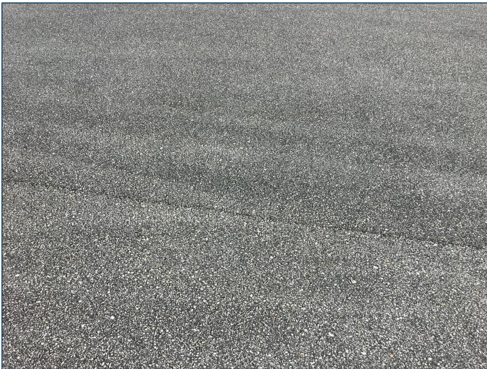
RW 7-25, Section 6210, Sample Unit 197 - Low Severity (48) Longitudinal & Transverse Cracking, Low Severity (52) Raveling, and Low Severity (57) Weathering
