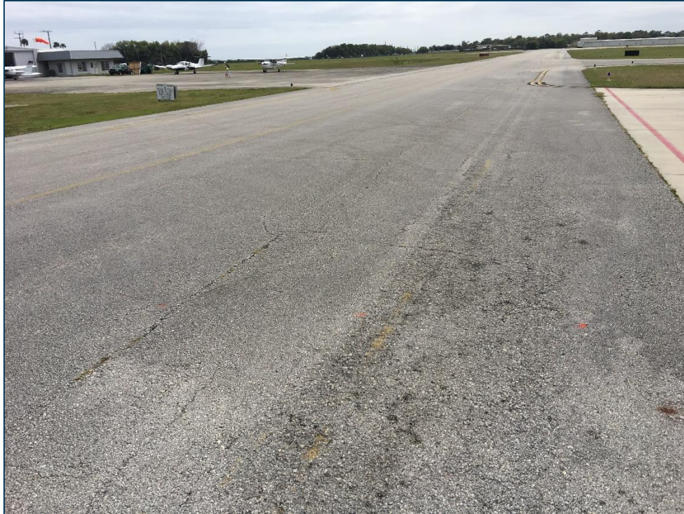
TW C, Section 310, Sample Unit 135 - Low Severity (48) Longitudinal & Transverse Cracking, Medium Severity (48) Longitudinal & Transverse Cracking, Low Severity (52) Raveling, and Medium Severity (52) Raveling
