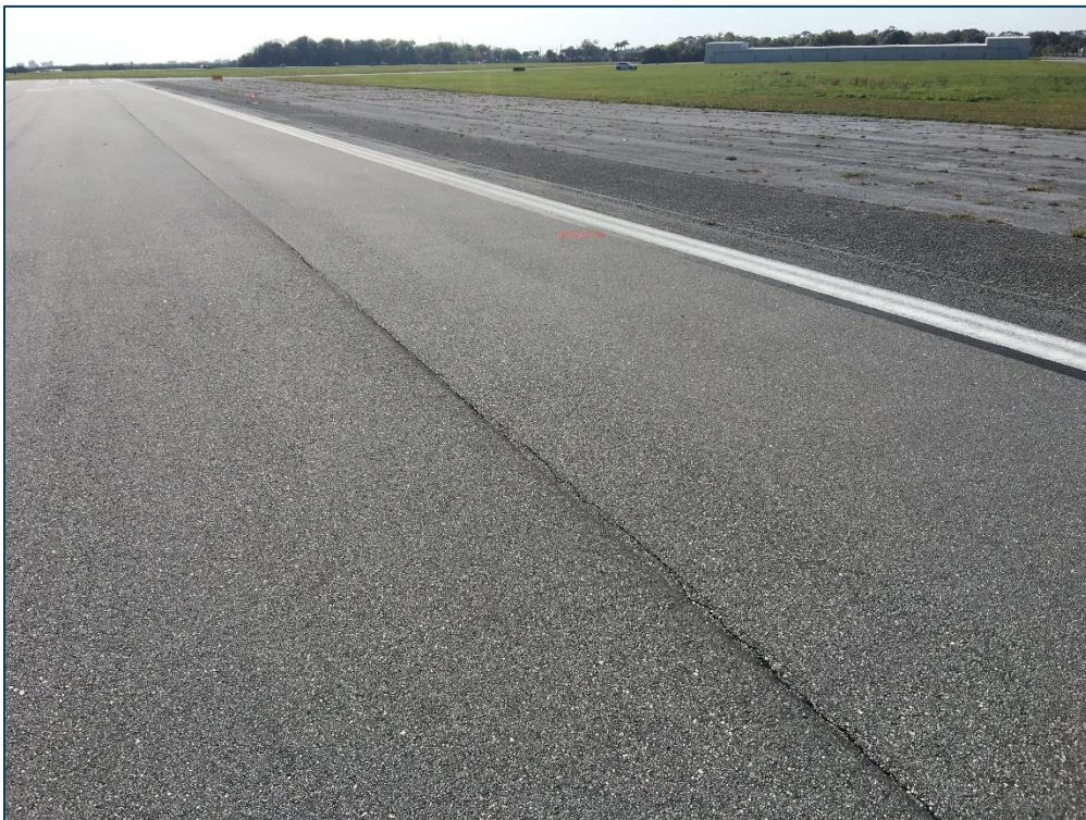
RW 11-29, Section 6105, Sample Unit 175 - Low Severity (48) Longitudinal & Transverse Cracking and Low Severity (57) Weathering
