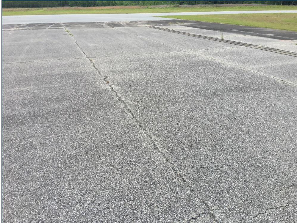
RW 5-23, Section 6112, Sample Unit 304 - Low Severity (47) Joint Reflection Cracking, Medium Severity (47) Joint Reflection Cracking, Low Severity (48) Longitudinal & Transverse Cracking, Low Severity (52) Raveling, and Low Severity (57) Weathering
