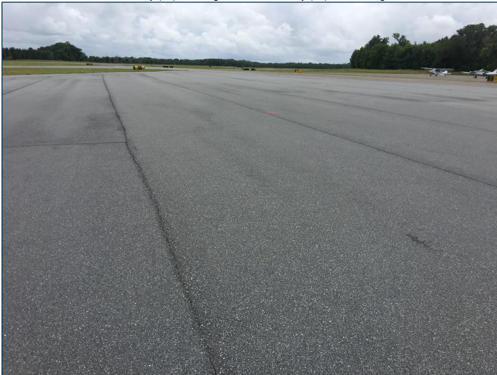
AP, Section 4110, Sample Unit 502 - Low Severity (48) Longitudinal & Transverse Cracking and Low Severity (57) Weathering
