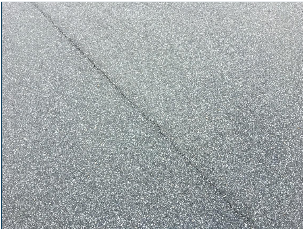
TW A, Section 205, Sample Unit 164 - Low Severity (48) Longitudinal & Transverse Cracking and Low Severity (57) Weathering
