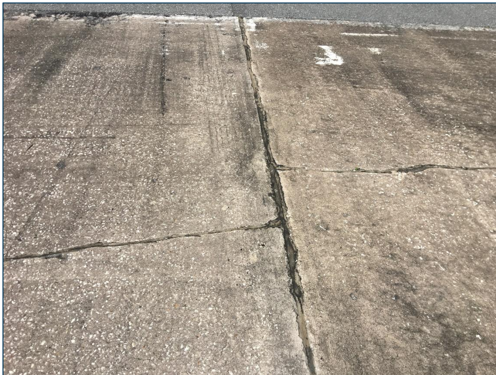
RW 14-32, Section 6205, Sample Unit 303 - Low Severity (63) Linear Cracking, Low Severity (65) Joint Seal Damage, and (73) Shrinkage Cracking
