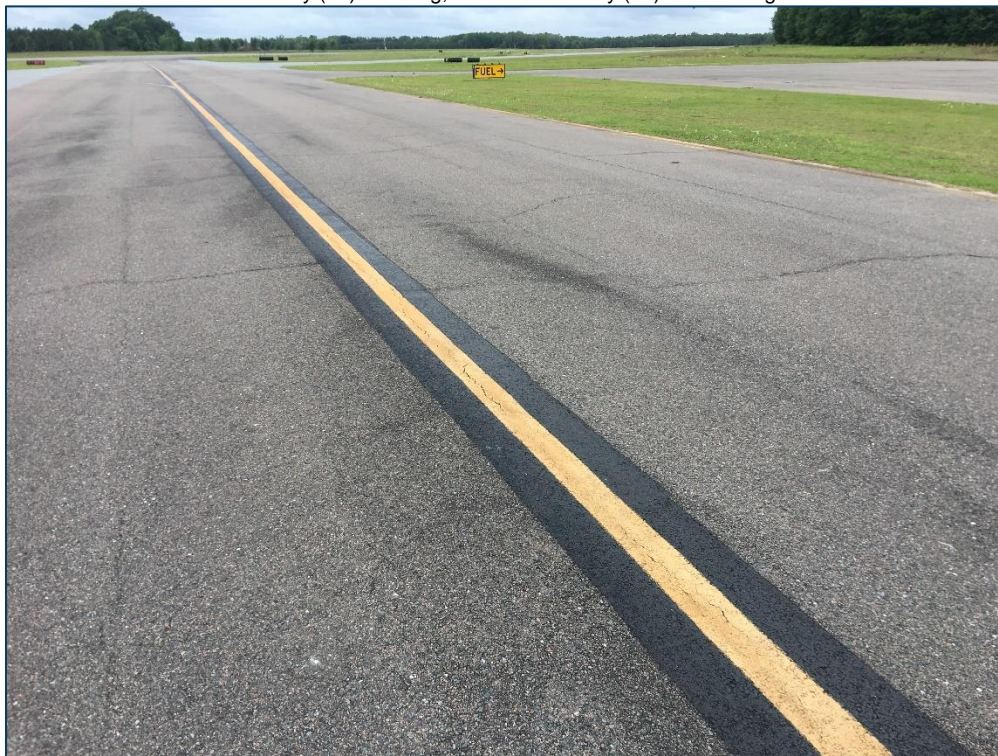
TW C, Section 105, Sample Unit 107 - Low Severity (45) Depression, Low Severity (48) Longitudinal & Transverse Cracking, Medium Severity (48) Longitudinal & Transverse Cracking, Low Severity (52) Raveling, Low Severity (56) Swelling, and Low Severity (57) Weathering
