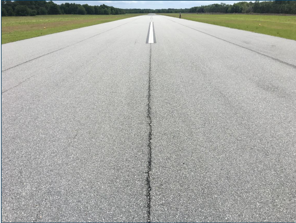
RW 14-32, Section 6215, Sample Unit 322 - Low Severity (48) Longitudinal & Transverse Cracking and Low Severity (57) Weathering
