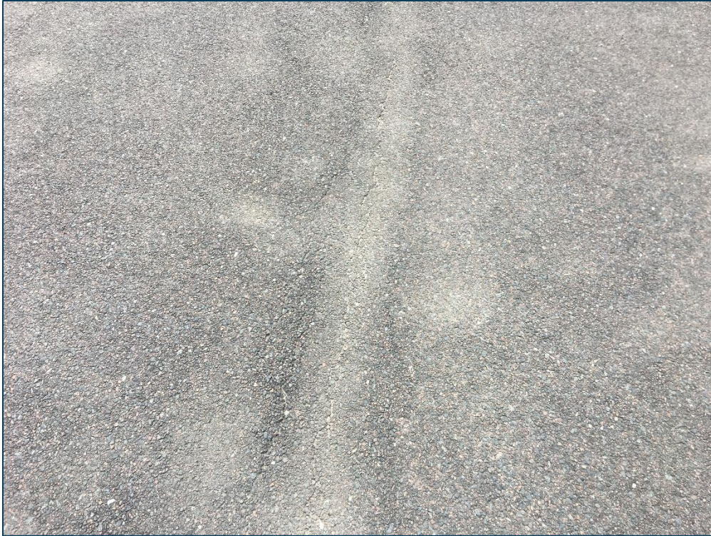
AP, Section 4105, Sample Unit 200 - Low Severity (48) Longitudinal & Transverse Cracking, Low Severity (52) Raveling, Low Severity (56) Swelling, and Low Severity (57) Weathering
