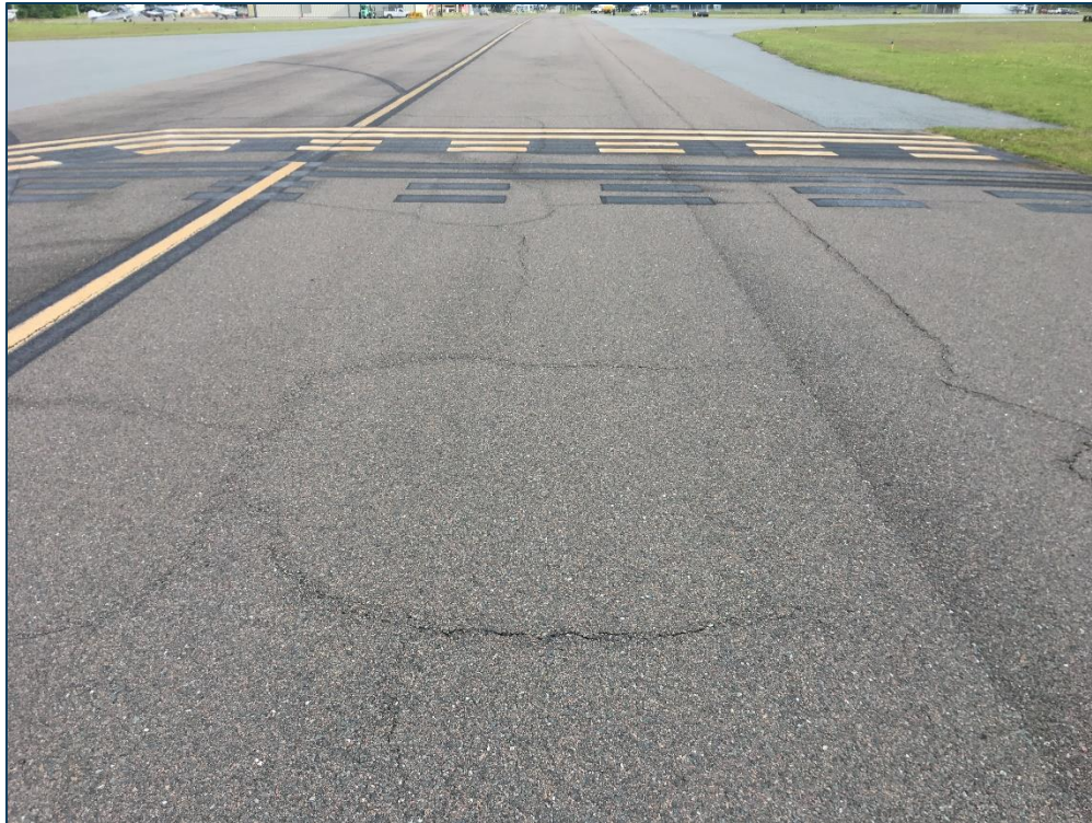
TW C, Section 105, Sample Unit 101 - Low Severity (48) Longitudinal & Transverse Cracking, Low Severity (52) Raveling, Low Severity (56) Swelling, and Low Severity (57) Weathering
