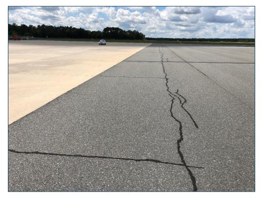
AP S, Section 4105, Sample Unit 151 - Low Severity (47) Joint Reflection Cracking, Low Severity (48) Longitudinal & Transverse Cracking, and Low Severity (57) Weathering
