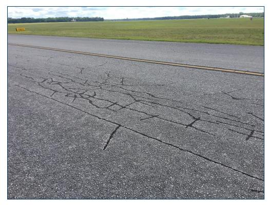
TW A, Section 105, Sample Unit 109 - Low Severity (41) Alligator Cracking, Low Severity (48) Longitudinal & Transverse Cracking, and Medium Severity (52) Raveling
