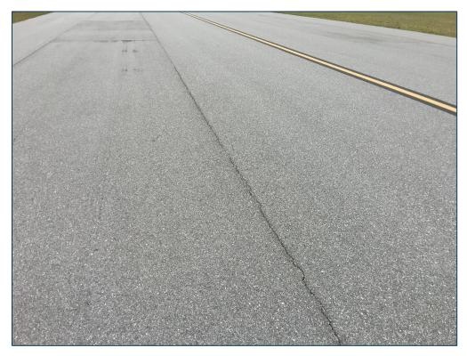
TW E, Section 505, Sample Unit 559 - Low Severity (48) Longitudinal & Transverse Cracking, Low Severity (56) Swelling, and Low Severity (57) Weathering
