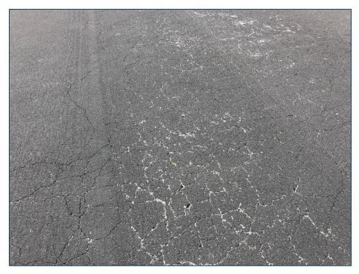
AP N, Section 4220, Sample Unit 109 - Medium Severity (41) Alligator Cracking, Low Severity (48) Longitudinal & Transverse Cracking, Low Severity (52) Raveling, and Low Severity (57) Weathering
