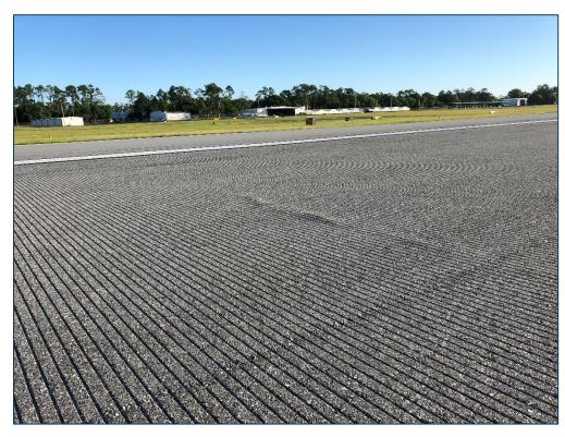
RW 7-25, Section 6105, Sample Unit 574 - Low Severity (48) Longitudinal & Transverse Cracking, Low Severity (56) Swelling, and Low Severity (57) Weathering
