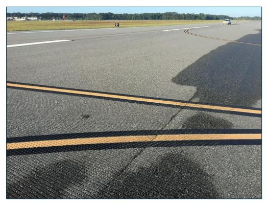
RW 7-25, Section 6105, Sample Unit 543 - Low Severity (48) Longitudinal & Transverse Cracking and Low Severity (57) Weathering
