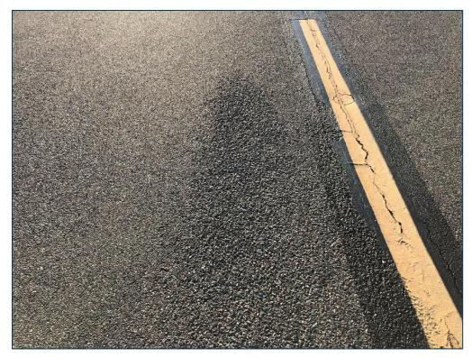
RW 11-29, Section 6202, Sample Unit 298 - (46) Jet Blast Erosion, Low Severity (48) Longitudinal & Transverse Cracking, Low Severity (52) Raveling, and Low Severity (57) Weathering
