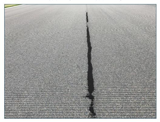
RW 11-29, Section 6225, Sample Unit 440 - Low Severity (48) Longitudinal & Transverse Cracking, Low Severity (52) Raveling, Low Severity (57) Weathering
