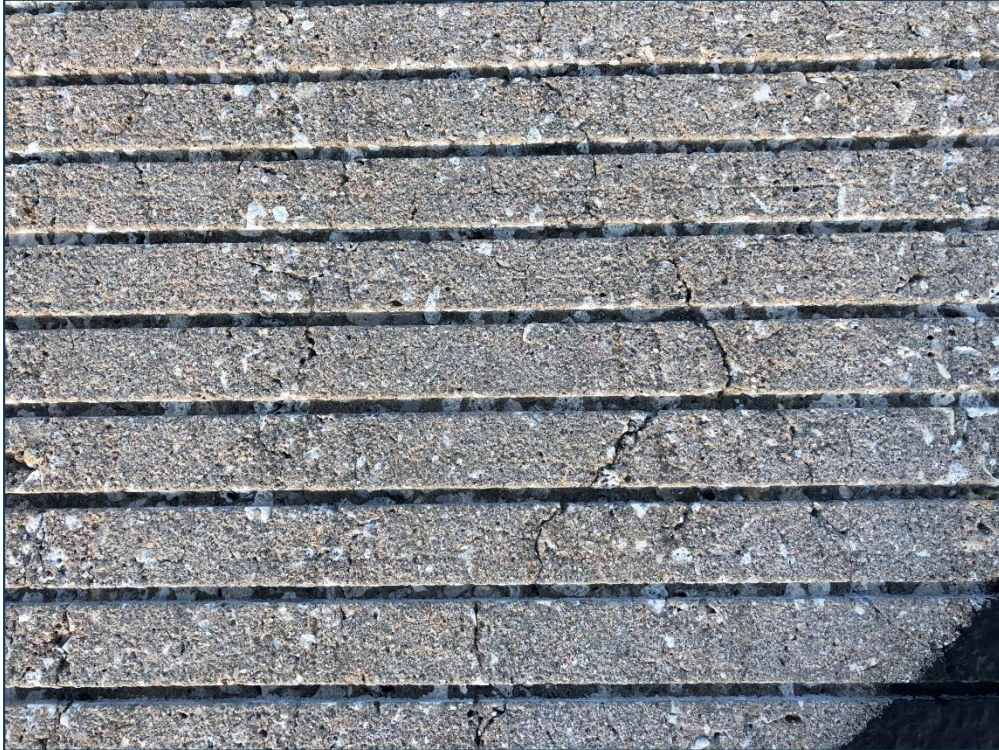
RW 8-26, Section 6105, Sample Unit377 - (73) Shrinkage Cracking
