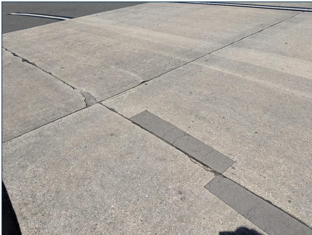
AP TERM, Section 4430, Sample Unit 405 - Low Severity (65) Joint Seal Damage, Medium Severity (66) Small Patch, Medium Severity (67) Large Patch/Utility Cut, and Low Severity (74) Joint Spall.
