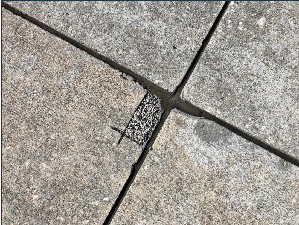
TWN, Section 305, Sample Unit 134 - Low Severity (66) Small Patch
