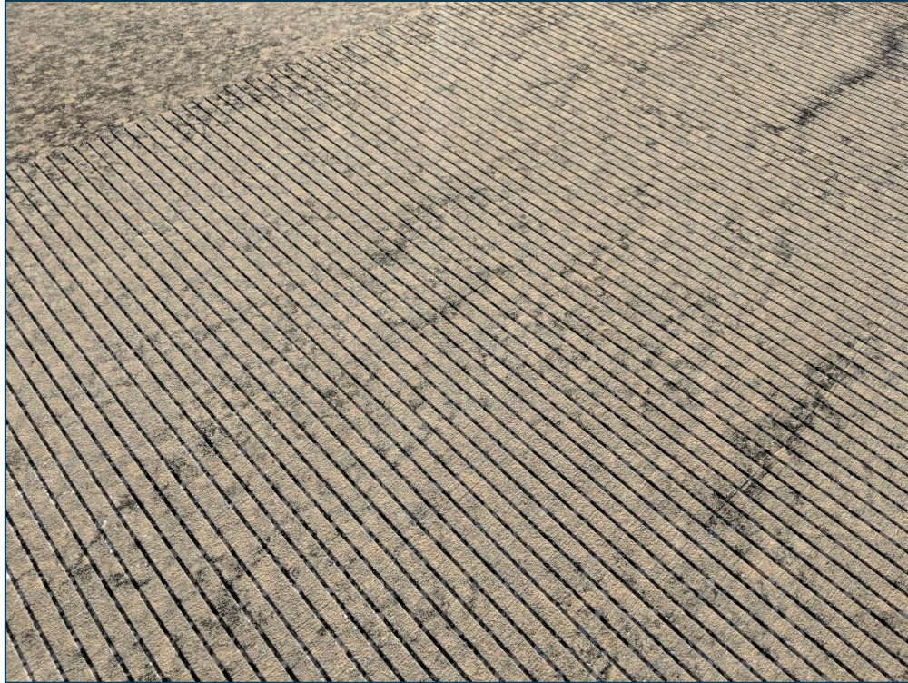
RW 14-32, Section 6207, Sample Unit 500 - (73) Shrinkage Cracking
