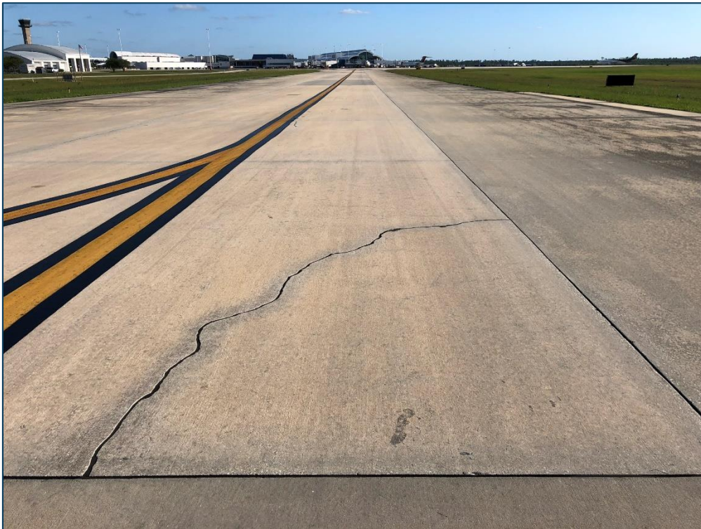
TW H, Section 555, Sample Unit 101 - Low Severity (62) Corner Break
