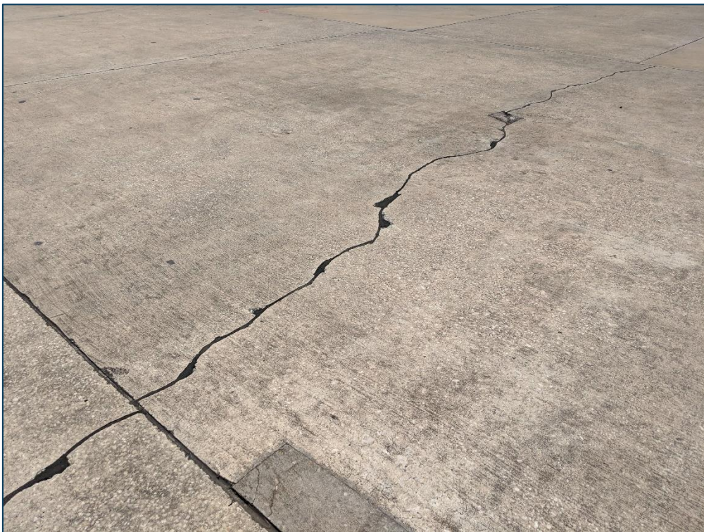
AP CARGO, Section 4125, Sample Unit 201 - Low Severity (63) Linear Cracking, Low Severity (65) Joint Seal Damage, and Low Severity (66) Small Patch.
