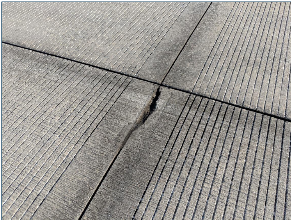
RW 14-32, Section 6215, Sample Unit 102 – Low Severity (74) Joint Spall
