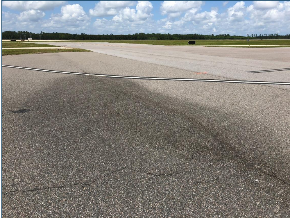
AP GA, Section 5105, Sample Unit 89 - Medium Severity (45) Depression, Low Severity (48) Longitudinal & Transverse Cracking, and Low Severity (57) Weathering
