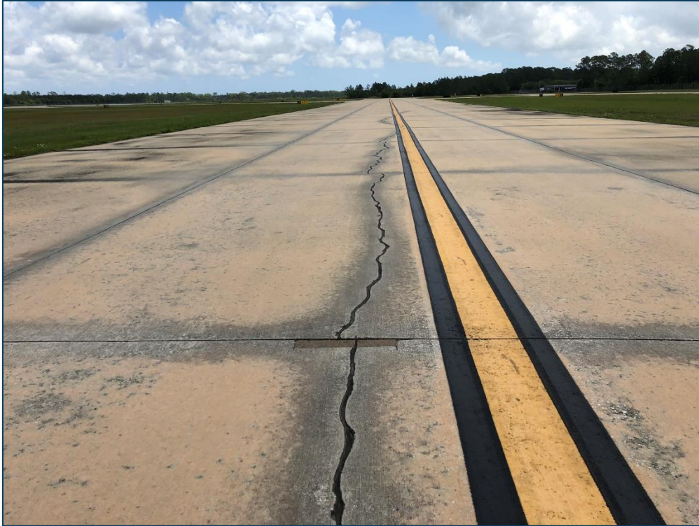
TW A, Section 125, Sample Unit 149 - Low Severity (63) Linear Cracking and Low Severity (66) Small Patch
