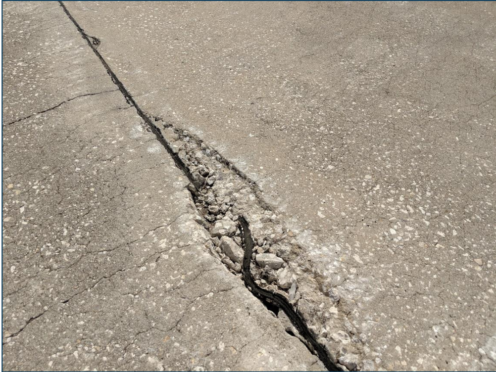
TW NE AP, Section 1105, Sample Unit 500 - High Severity (74) Joint Spall
