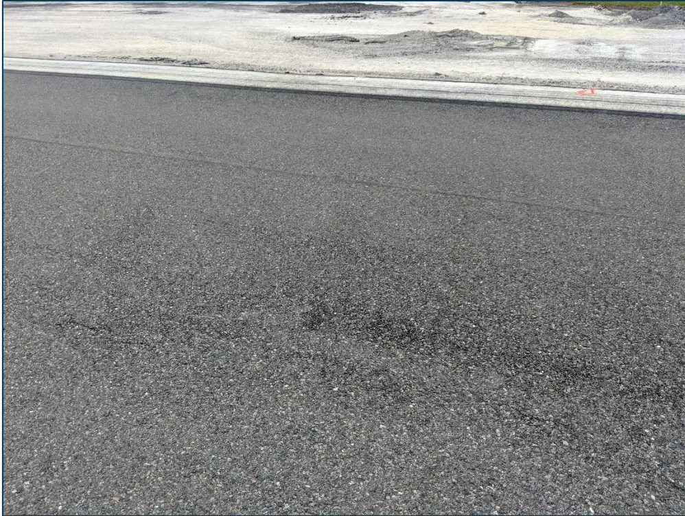
RW 7-25, Section 6105, Sample Unit 161 - Low Severity (48) Longitudinal & Transverse Cracking, Low Severity (52) Raveling, and Low Severity (57) Weathering
