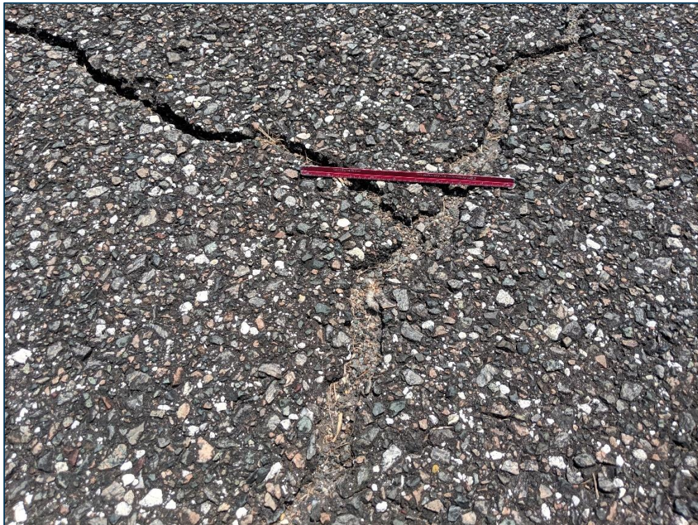
TW T-HANG, Section 925, Sample Unit 200 - Medium Severity (48) Longitudinal & Transverse Cracking, Low Severity (52) Raveling, and Medium Severity (57) Weathering
