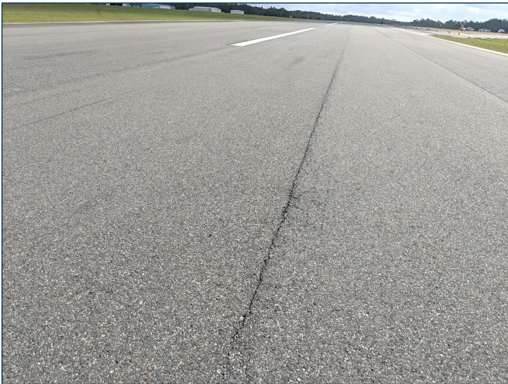
RW 7-25, Section 6110, Sample Unit 133 - Low Severity (48) Longitudinal & Transverse Cracking, Low Severity (52) Raveling, and Low Severity (57) Weathering
