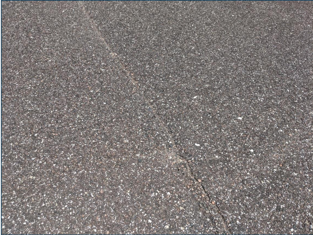
AP NW, Section 4115, Sample Unit 502 - Low Severity (48) Longitudinal & Transverse Cracking, Low Severity (52) Raveling, and Low Severity (57) Weathering
