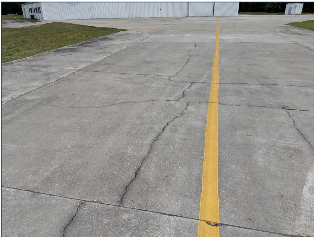
TWNE AP, Section 1105, Sample Unit500 - Low Severity (65) Joint Seal Damage and Medium Severity (72) Shattered Slab
