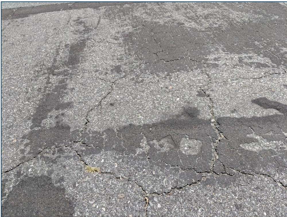
TWT-HANG, Section 905, Sample Unit 100 - Medium Severity (43) Block Cracking and Low Severity (52) Raveling
