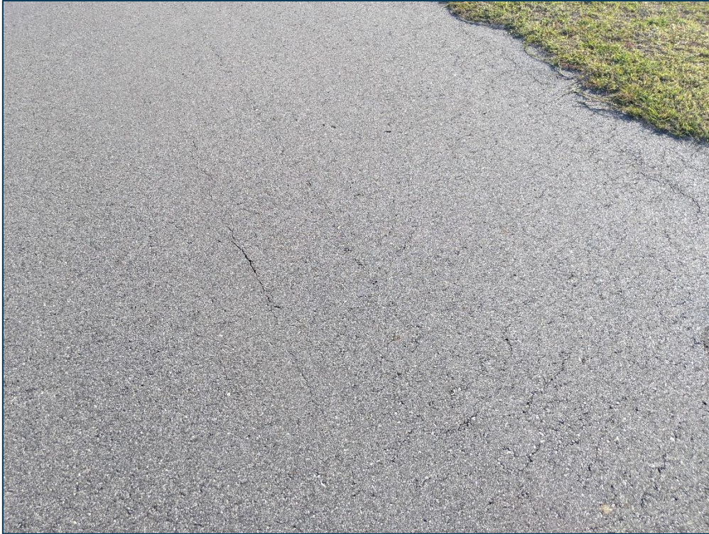
TWA, Section 105, Sample Unit102 - Low Severity (48) Longitudinal & Transverse Cracking and Low Severity (57) Weathering
