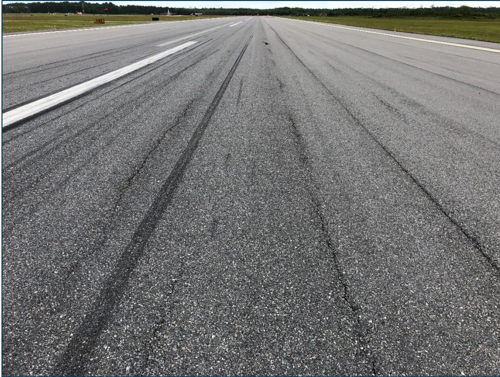
RW 5-23, Section 6105, Sample Unit 135 - Low Severity (48) Longitudinal & Transverse Cracking, Low Severity (57) Weathering, and Medium Severity (57) Weathering
