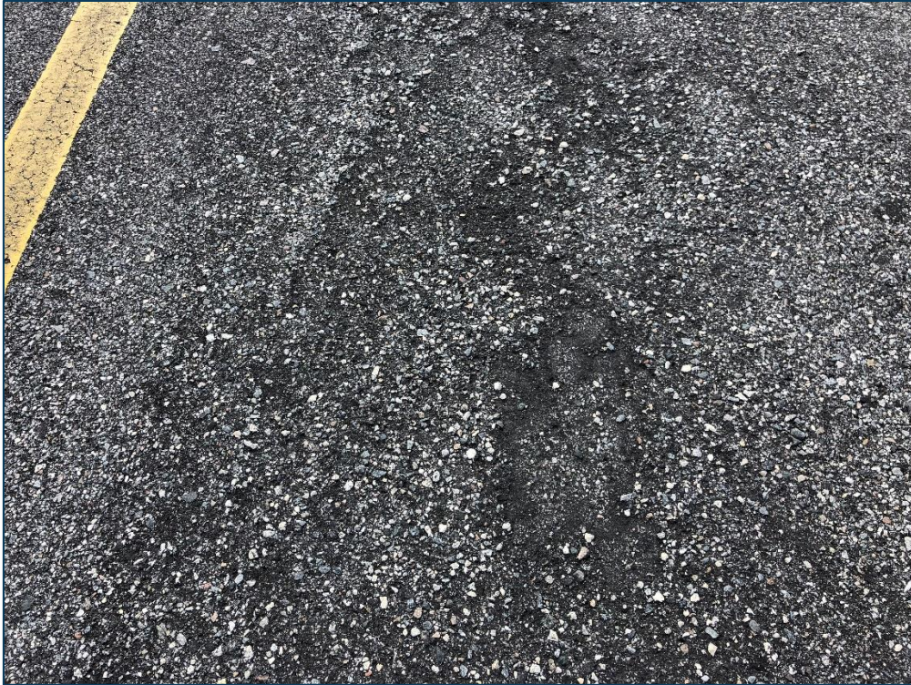
AP N, Section 4220, Sample Unit 600 - Medium Severity (52) Raveling
