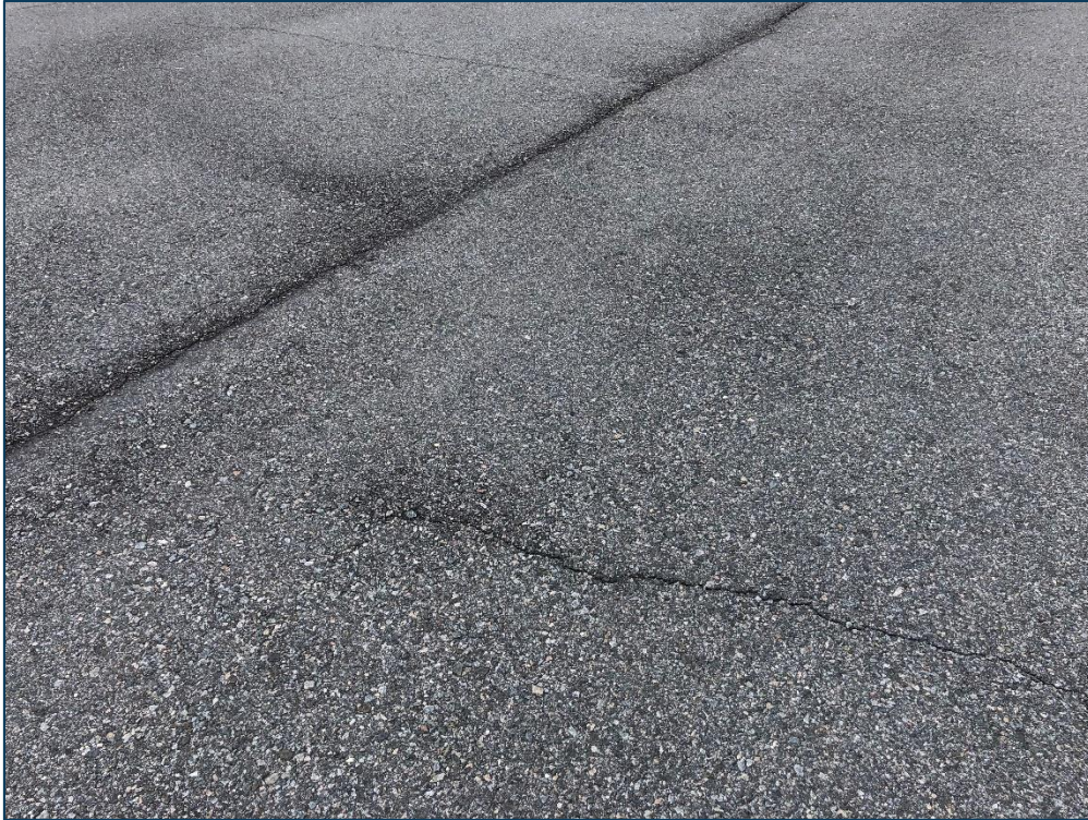
TWA, Section 105, Sample Unit 158 - Low Severity (48) Longitudinal & Transverse Cracking, Low Severity (52) Raveling, and Low Severity (57) Weathering
