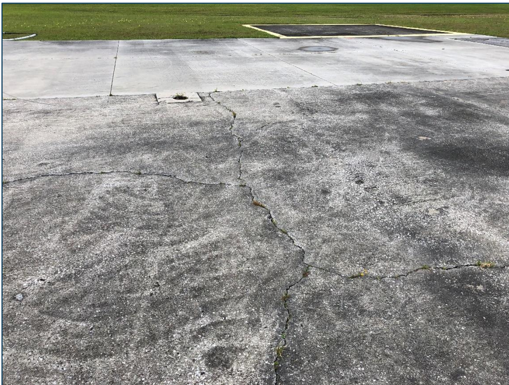
AP SW, Section 4405, Sample Unit 101 - Medium Severity (72) Shattered Slab
