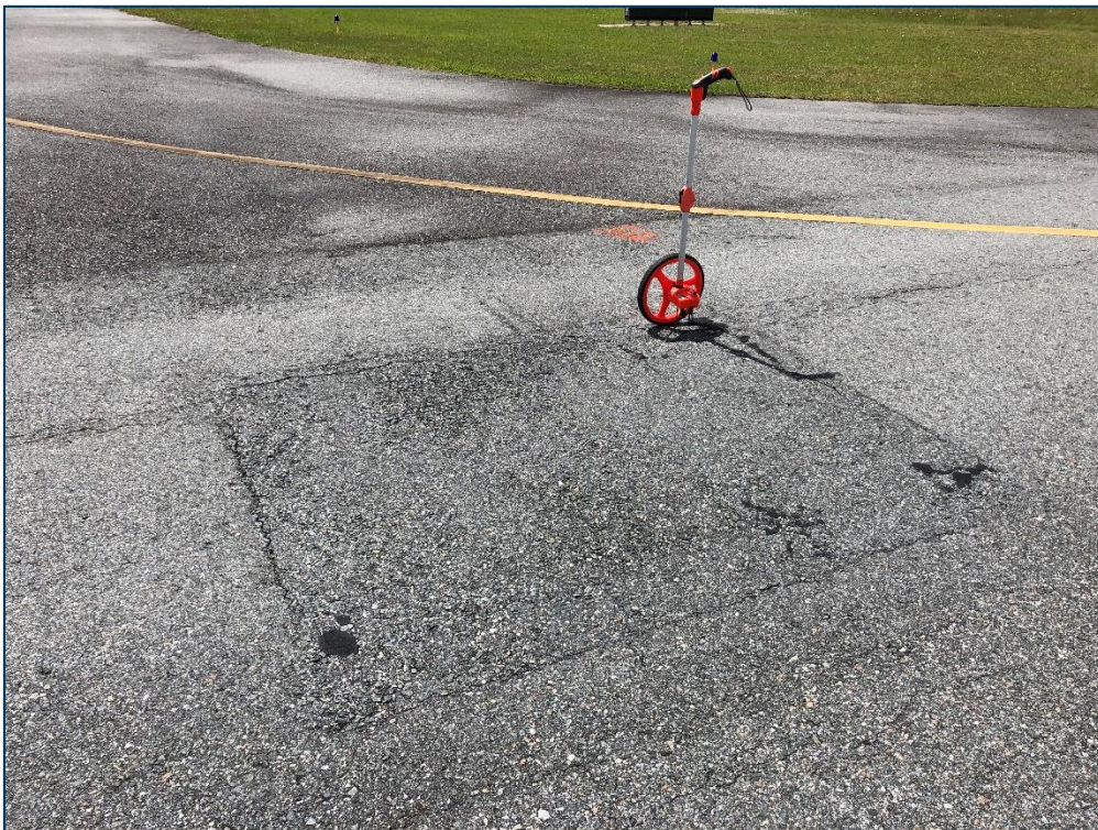
TWB, Section 225, Sample Unit 120 - Low Severity (50) Patching, Low Severity (52) Raveling, and Low Severity (57) Weathering
