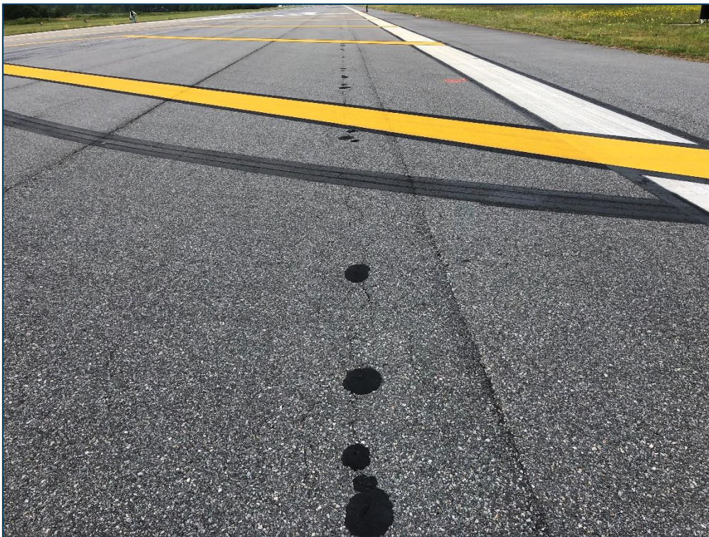
RW 5-23, Section 6105, Sample Unit 168 - (42) Bleeding, Low Severity (48) Longitudinal & Transverse Cracking, and Low Severity (57) Weathering
