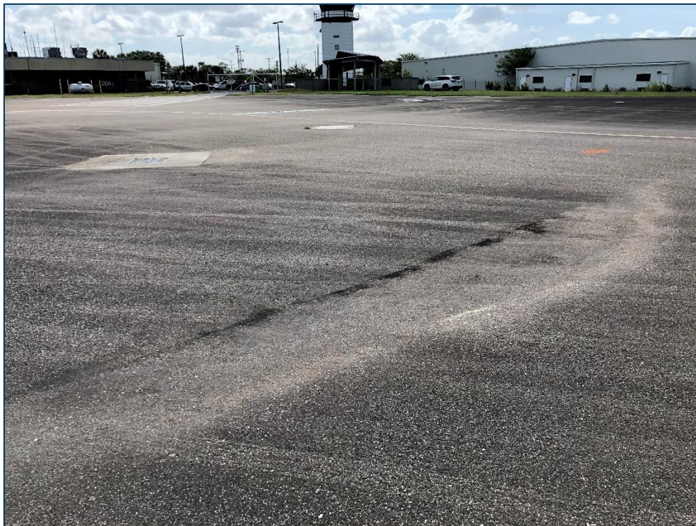
AP FAA, Section 4505, Sample Unit 603 - Low Severity (45) Depression, Low Severity (52) Raveling, and Low Severity (57) Weathering
