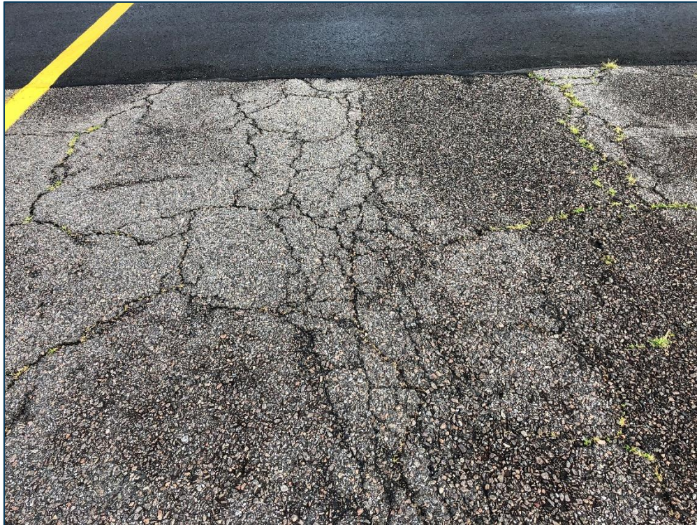
TW B4, Section 245, Sample Unit 407 - Low Severity (41) Alligator Cracking, Medium Severity (43) Block Cracking, Low Severity (52) Raveling, and Medium Severity (57) Weathering
