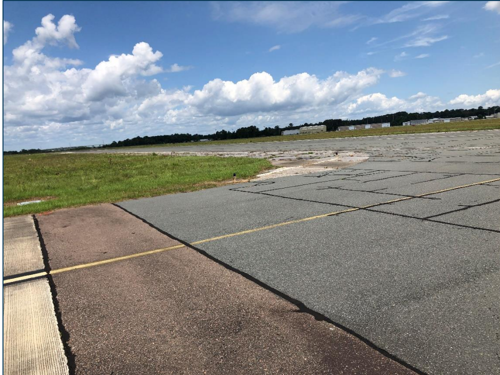
TW C, Section 120, Sample Unit 116 - Low Severity (48) Longitudinal & Transverse Cracking, Low Severity (50) Patching, and Low Severity (57) Weathering
