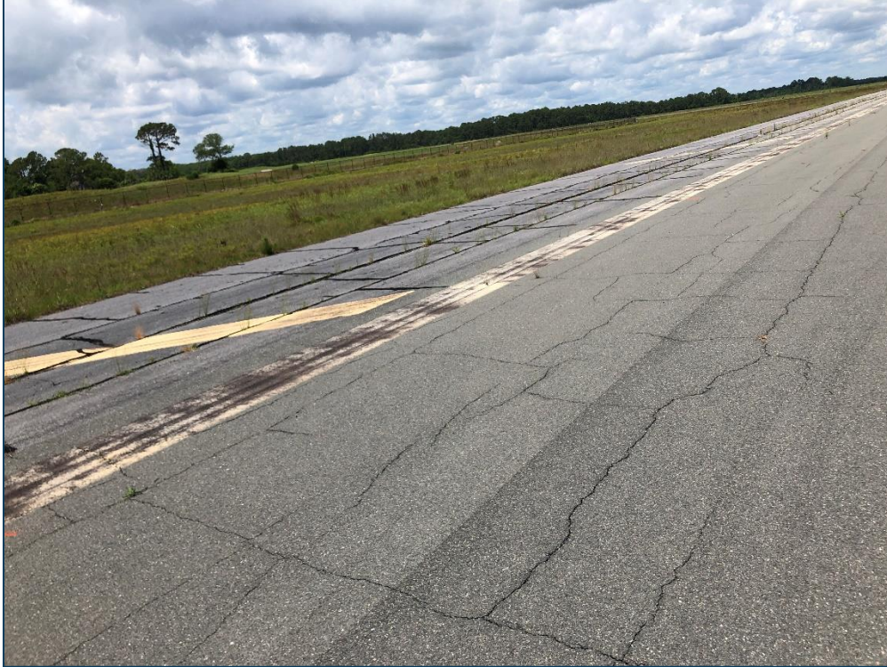
RW 13-31, Section 6215, Sample Unit 329 - Low Severity (43) Block Cracking, Low Severity (48) Longitudinal & Transverse Cracking, and Low Severity (57) Weathering
