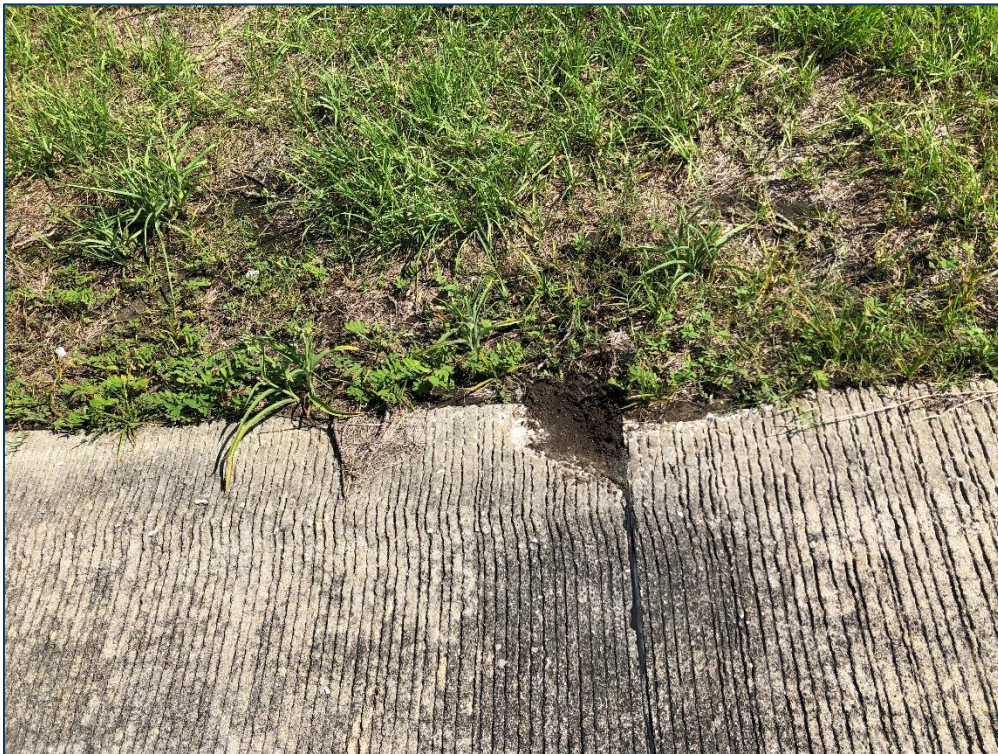
RW 9-27, Section 6335, Sample Unit 406 - High Severity (65) Joint Seal Damage and Medium Severity (75) Corner Spall
