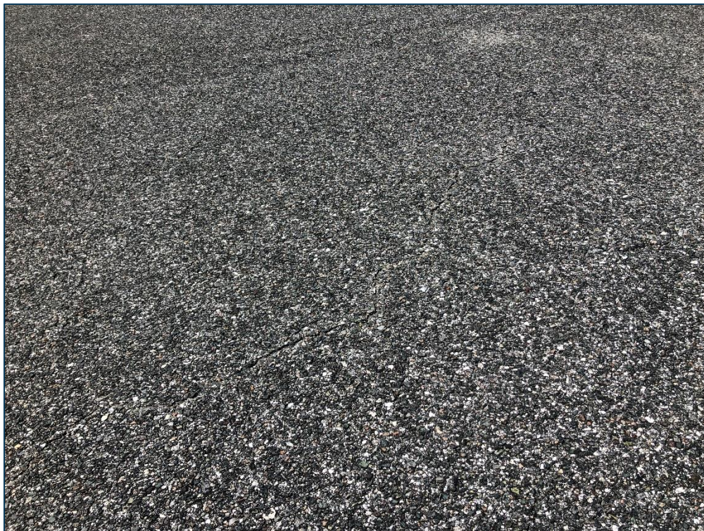
AP N, Section 4215, Sample Unit 208 - Low Severity (48) Longitudinal & Transverse Cracking, Low and Medium Severity (57) Weathering
