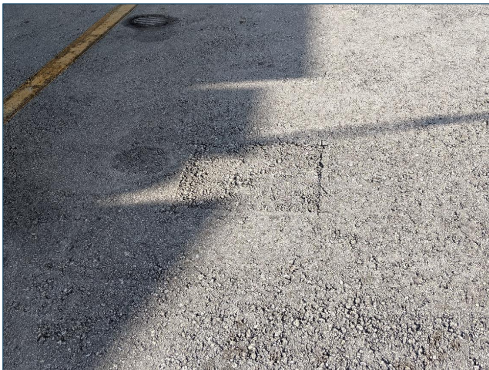
AP GA, Section 4105, Sample Unit 360 - Low Severity (50) Patching, Low Severity (52) Raveling, and Low Severity (57) Weathering
