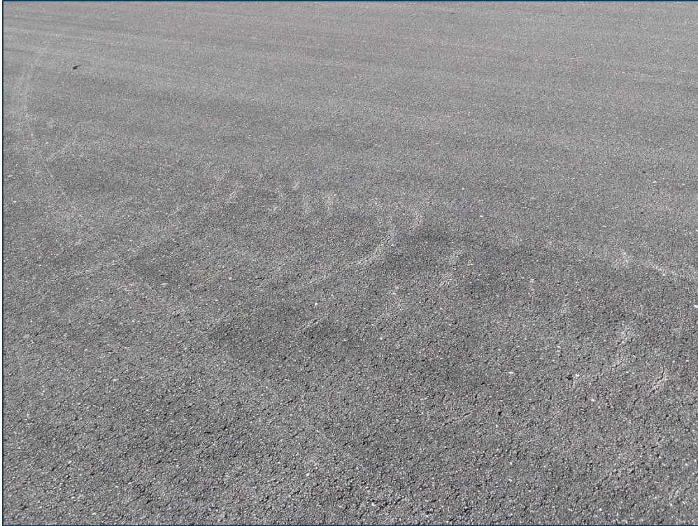
RW 10-28, Section 6105, Sample Unit 364 - Low Severity (48) Longitudinal & Transverse Cracking, Low Severity (52) Raveling, and Low Severity (57) Weathering
