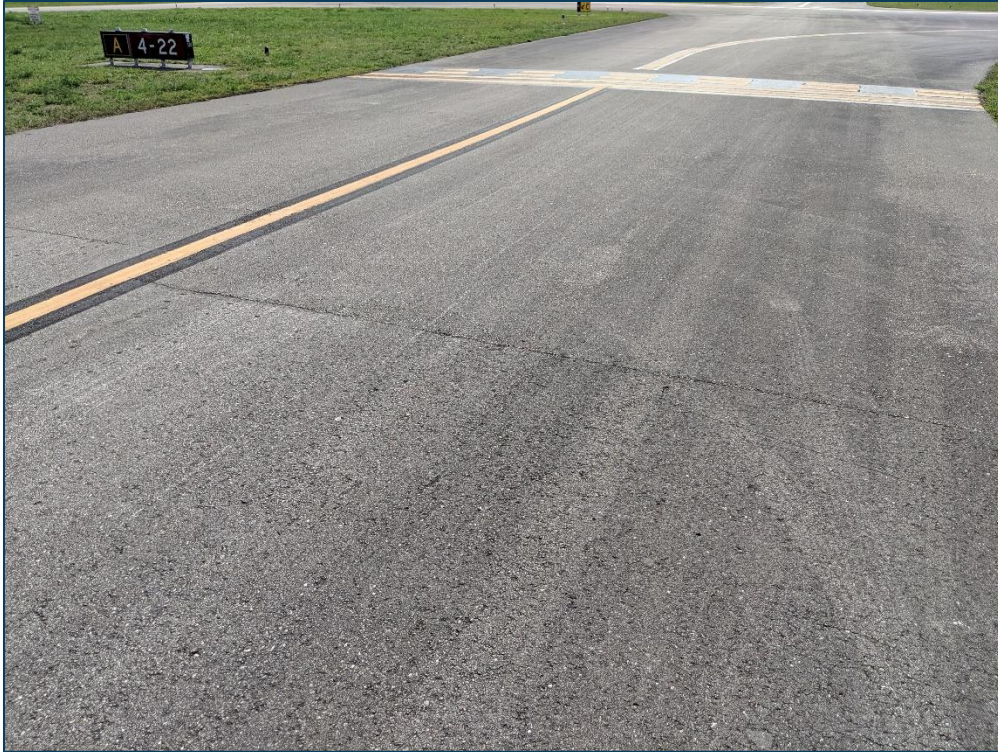
TW A, Section 310, Sample Unit 307 - Low Severity (48) Longitudinal & Transverse Cracking and Low Severity (52) Raveling
