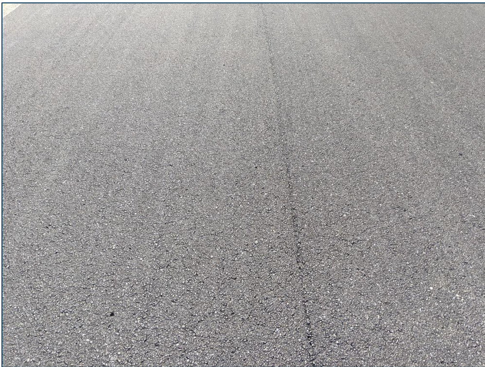
RW 10-28, Section 6105, Sample Unit 337 - Low Severity (52) Raveling and Low Severity (57) Weathering
