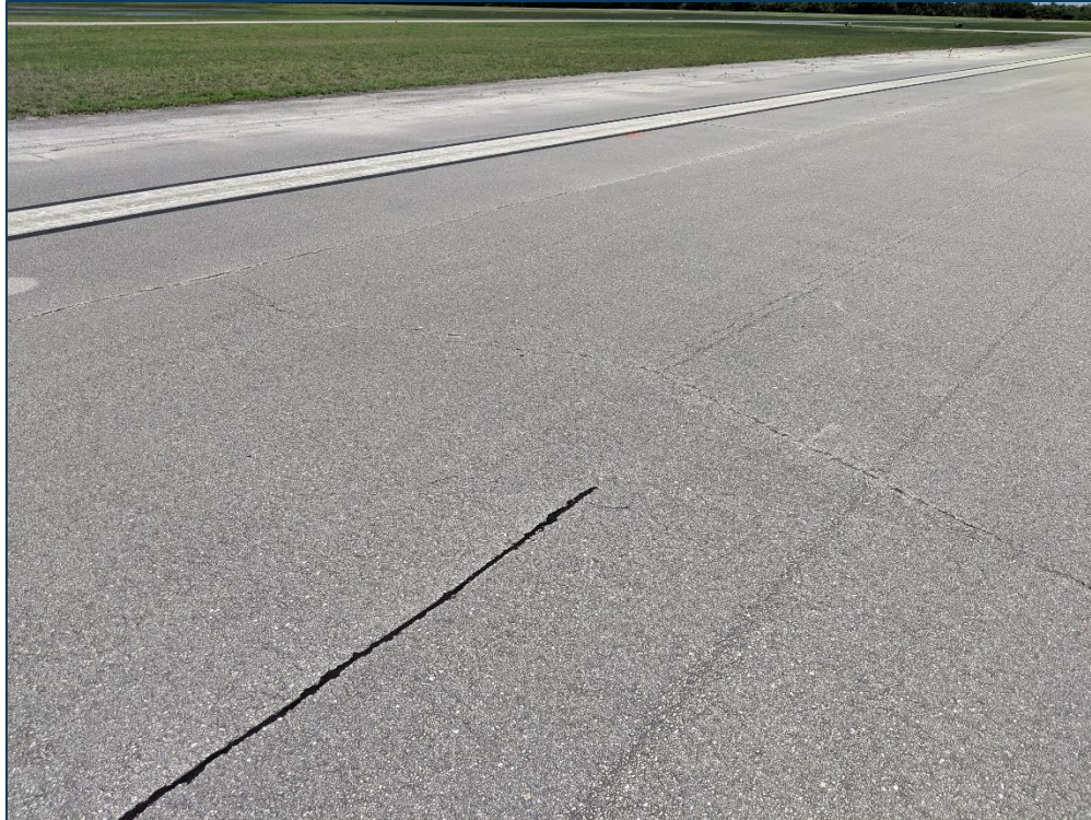
RW 16-34, Section 6215, Sample Unit 124 - Low Severity (48) Longitudinal & Transverse Cracking and Low Severity (52) Raveling
