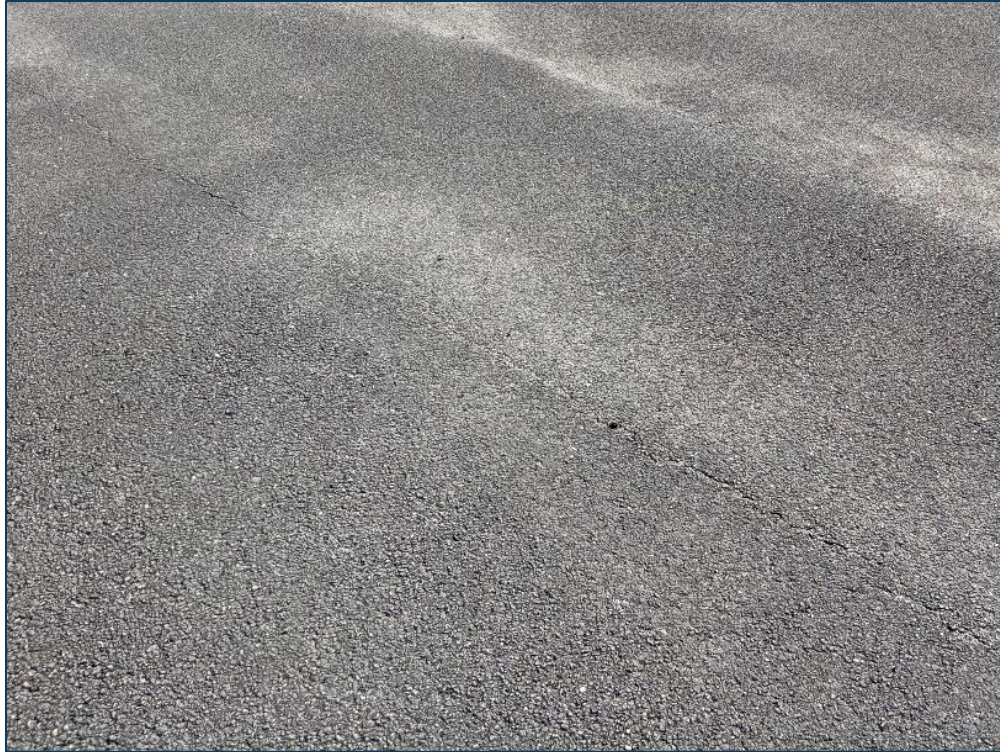
AP GA, Section 4110, Sample Unit 553 - Low Severity (48) Longitudinal & Transverse Cracking and Low Severity (52) Raveling
