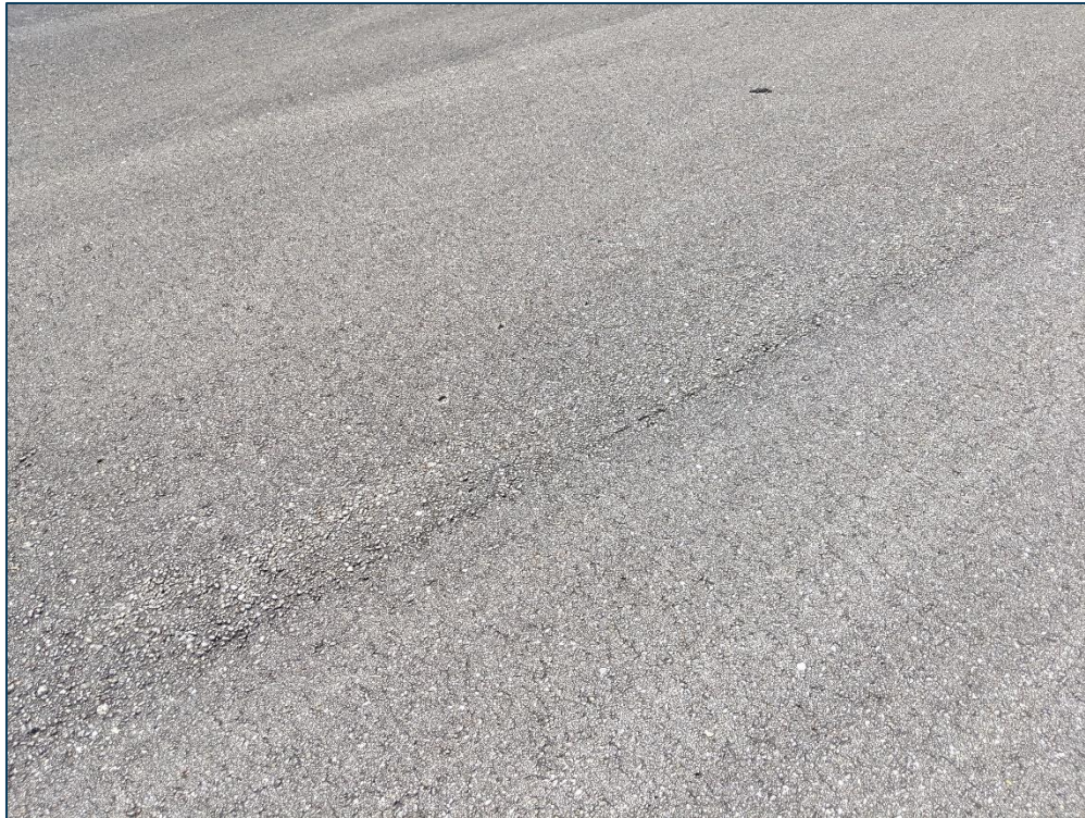
TW C, Section 103, Sample Unit 101 - Low Severity (48) Longitudinal & Transverse Cracking, Low Severity (52) Raveling, and Low Severity (57) Weathering
