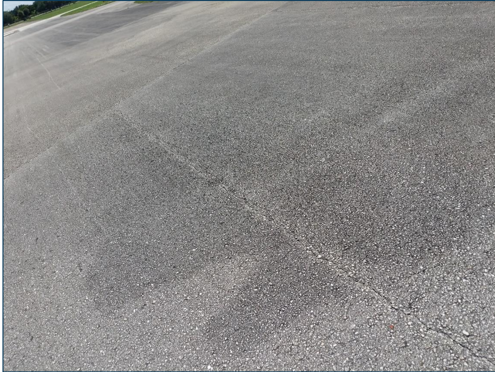
RW 4-22, Section 6305, Sample Unit 106 - Low Severity (48) Longitudinal & Transverse Cracking, Low Severity (52) Raveling, and Low Severity (57) Weathering
