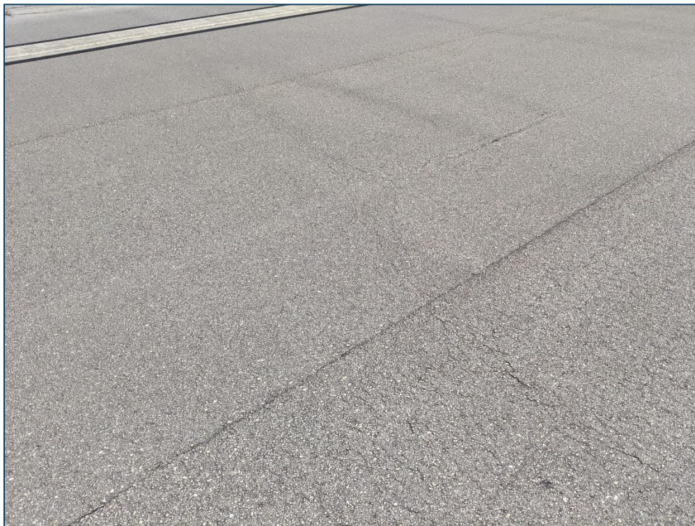
RW 16-34, Section 6215, Sample Unit 134 - Low Severity (48) Longitudinal & Transverse Cracking, Low Severity (52) Raveling, and Low Severity (57) Weathering
