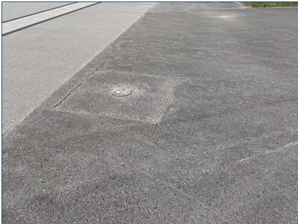
RW 4-22, Section 6305, Sample Unit 159 - Low Severity (48) Longitudinal & Transverse Cracking, Medium Severity (50) Patching, Low Severity (52) Raveling, and Low Severity (57) Weathering
