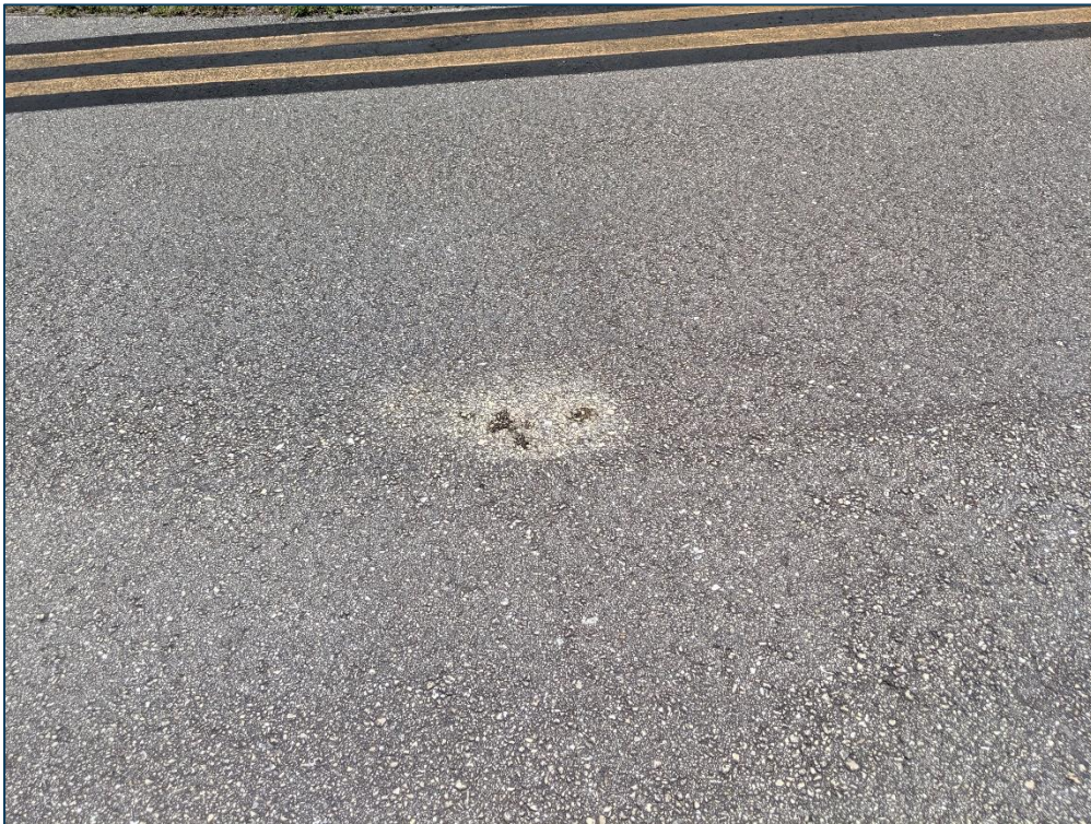
TW B, Section 217, Sample Unit 100 – Low and Medium Severity (57) Weathering
