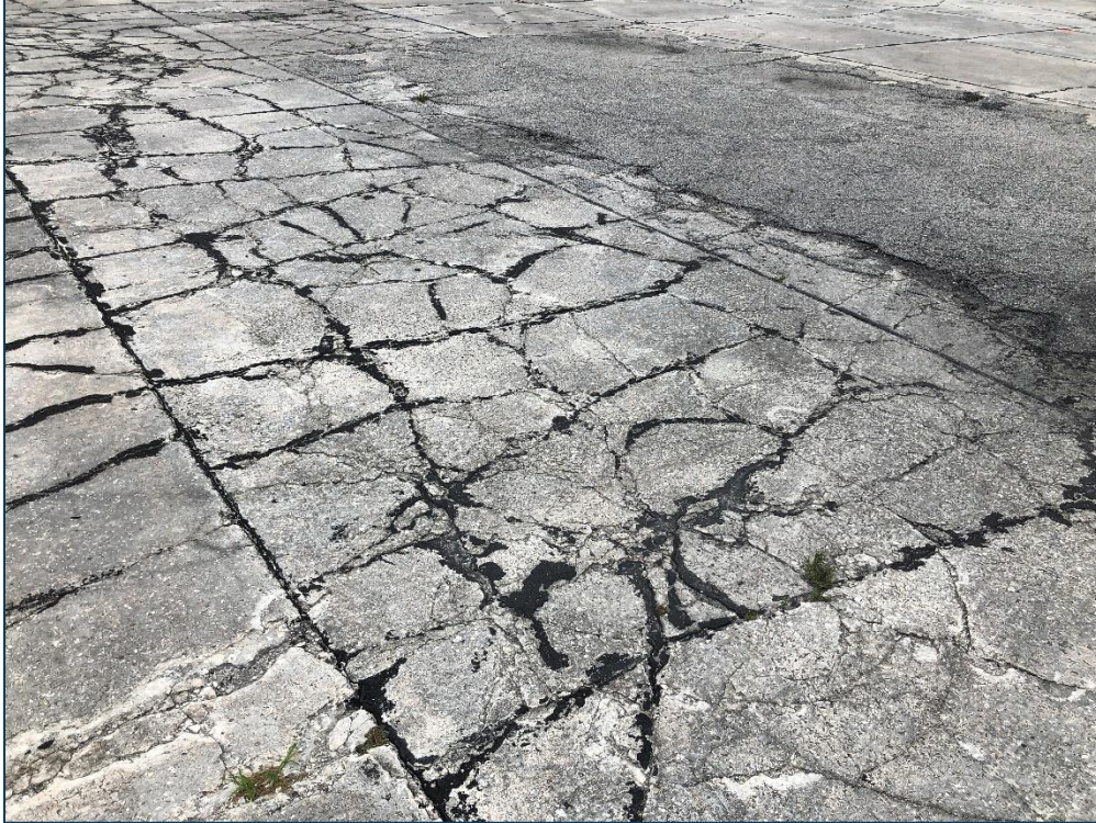
AP SW GA, Section 4307, Sample Unit 449 - High Severity (65) Joint Seal Damage and High Severity (72) Shattered Slab
