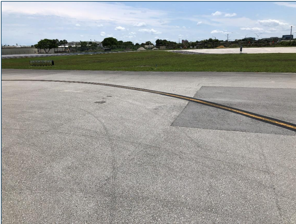
AP RU 5, Section 5115, Sample Unit 201 - Low Severity (48) Longitudinal & Transverse Cracking, Low Severity (50) Patching, and Low Severity (57) Weathering
