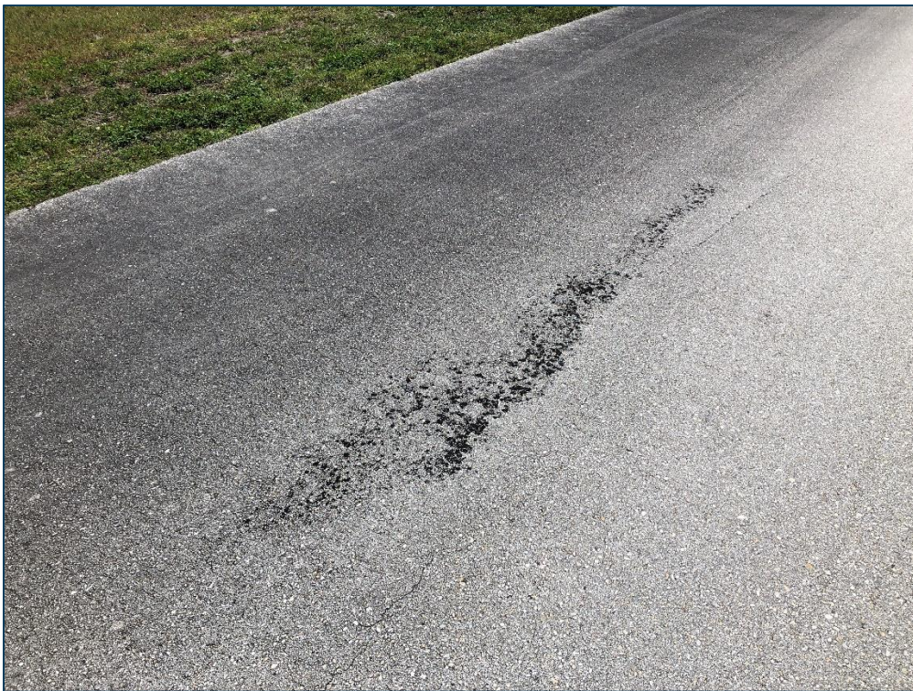
TW P, Section 105, Sample Unit 105 - (42) Bleeding, Low Severity (48) Longitudinal & Transverse Cracking, and Low Severity (57) Weathering
