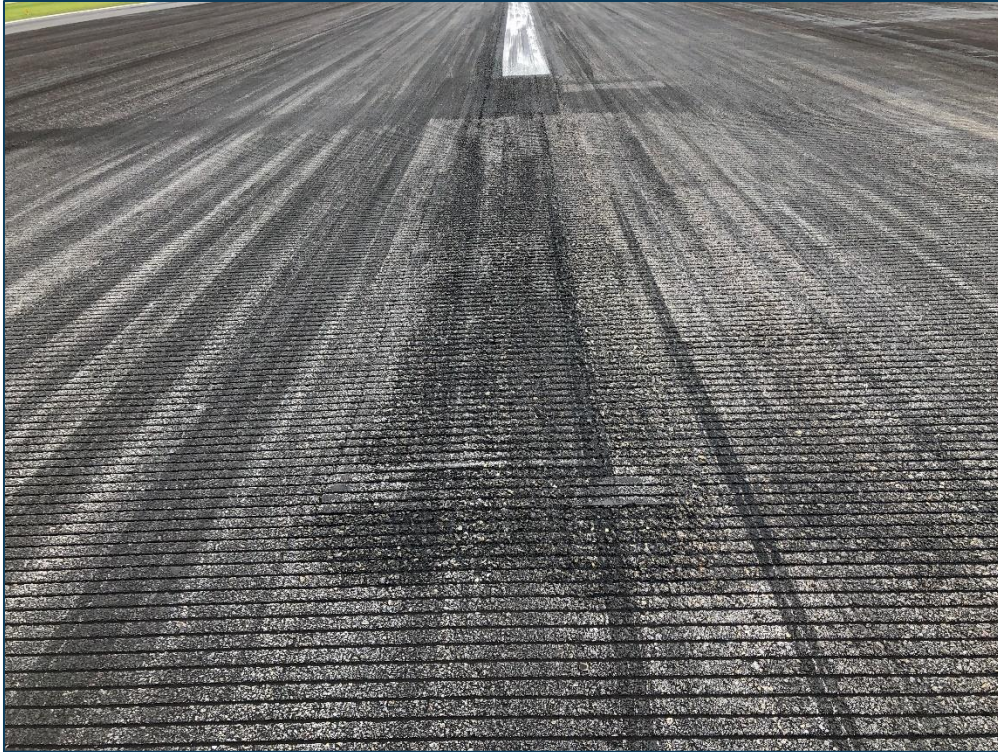
RW 5-23, Section 6105, Sample Unit 382 - Low Severity (48) Longitudinal & Transverse Cracking, Low Severity (52) Raveling, and Low Severity (57) Weathering
