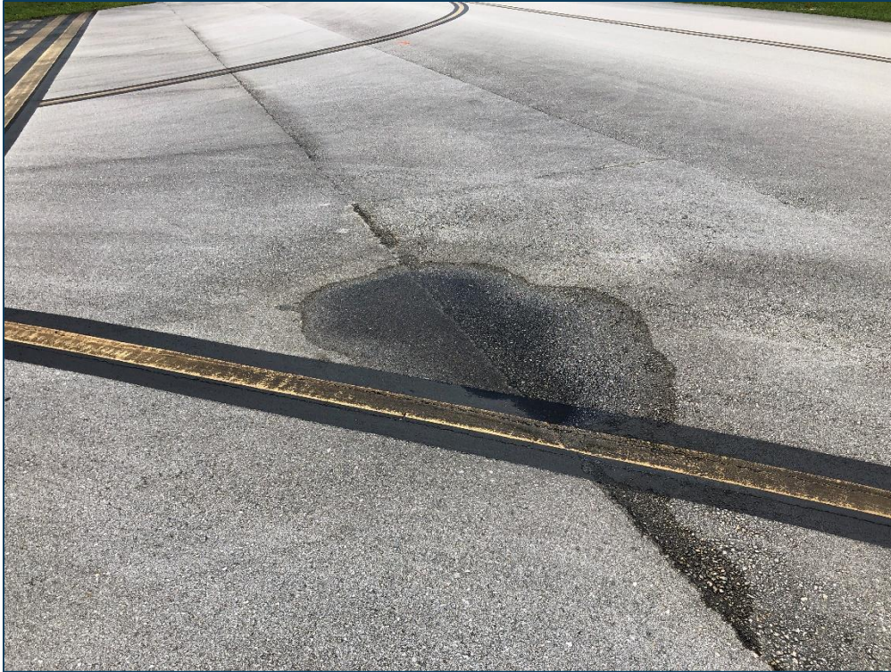
TW E, Section 116, Sample Unit 251 - Low Severity (45) Depression, Low Severity (48) Longitudinal & Transverse Cracking, and Low Severity (57) Weathering
