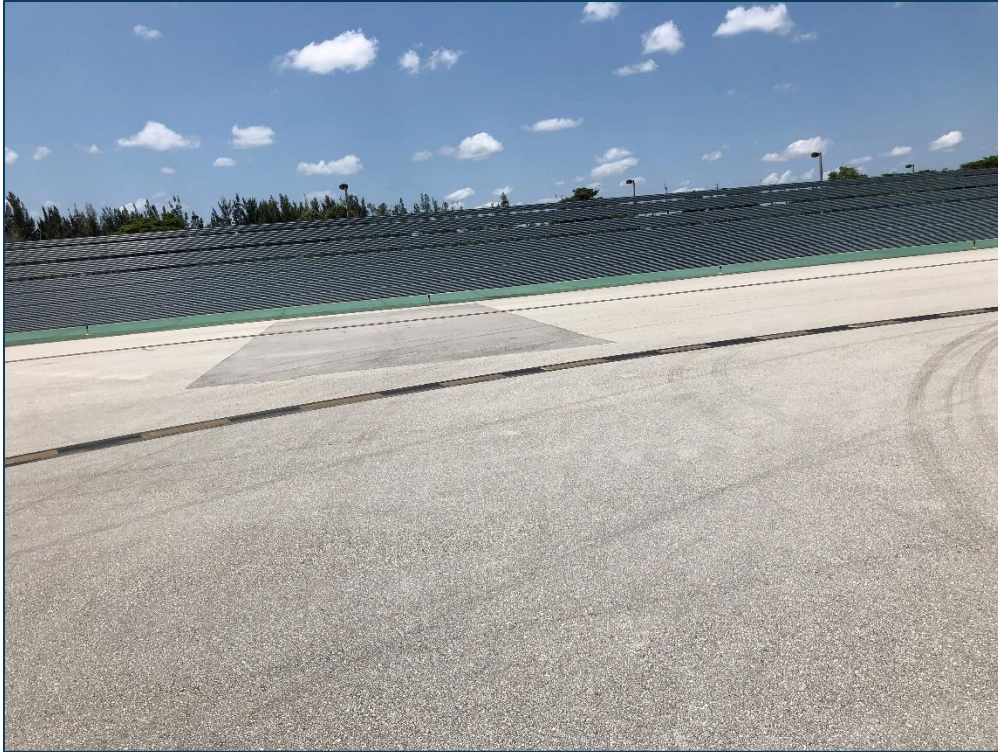
AP RU 5, Section 5105, Sample Unit 100 - Low Severity (50) Patching and Low Severity (57) Weathering
