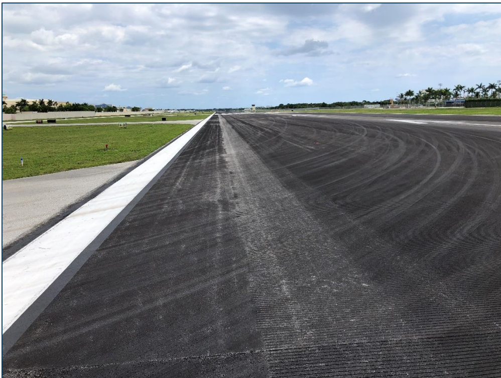
RW 5-23, Section 6111, Sample Unit 84 - Low Severity (48) Longitudinal & Transverse Cracking and Low Severity (57) Weathering
