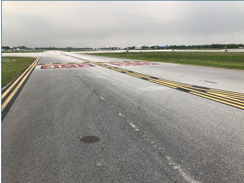
TW A, Section 110, Sample Unit 127 - Low Severity (48) Longitudinal & Transverse Cracking, Low Severity (52) Raveling, and Low Severity (57) Weathering
