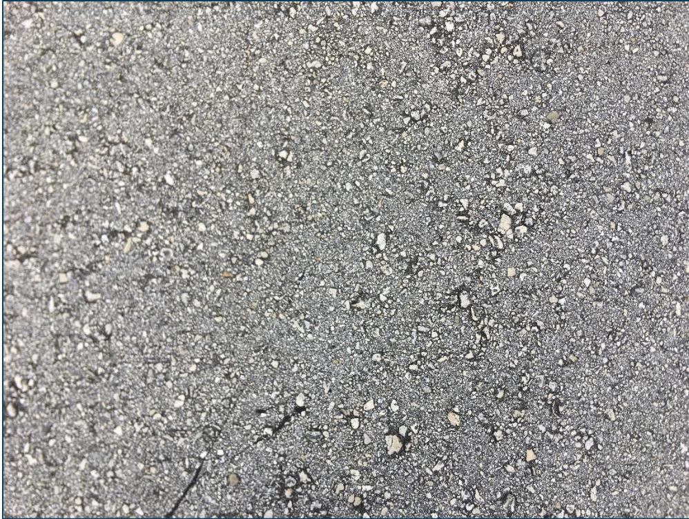
AP CUSTOMS, Section 5605, Sample Unit 252 - Low Severity (57) Weathering and Medium Severity (57) Weathering
