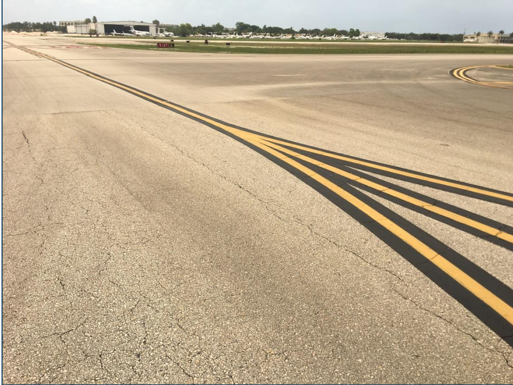
TW D, Section 414, Sample Unit 112 - Low Severity (43) Block Cracking, Low Severity (48) Longitudinal & Transverse Cracking, Low Severity (52) Raveling, Medium Severity (52) Raveling, Low Severity (53) Rutting, and Medium Severity (53) Rutting
