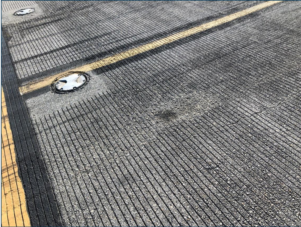
RW 13-31, Section 6205, Sample Unit 165 - Low Severity (48) Longitudinal & Transverse Cracking, Low Severity (52) Raveling, and Medium Severity (52) Raveling
