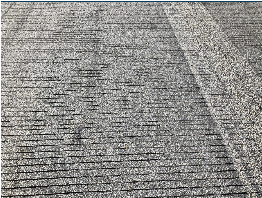
RW 13-31, Section 6210, Sample Unit 145 - Low Severity (48) Longitudinal & Transverse Cracking, Low Severity (52) Raveling, and Low Severity (57) Weathering
