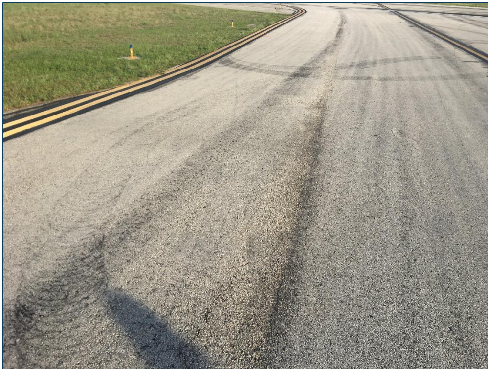
TW B, Section 210, Sample Unit 140 - Low Severity (48) Longitudinal & Transverse Cracking, Low Severity (52) Raveling, Low Severity (56) Swelling, and Low Severity (57) Weathering
