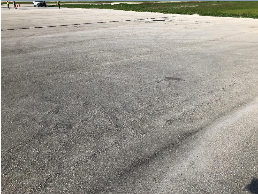
AP MAINT, Section 5405, Sample Unit 104 - Low Severity (48) Longitudinal & Transverse Cracking, Low Severity (56) Swelling, and Low Severity (57) Weathering
