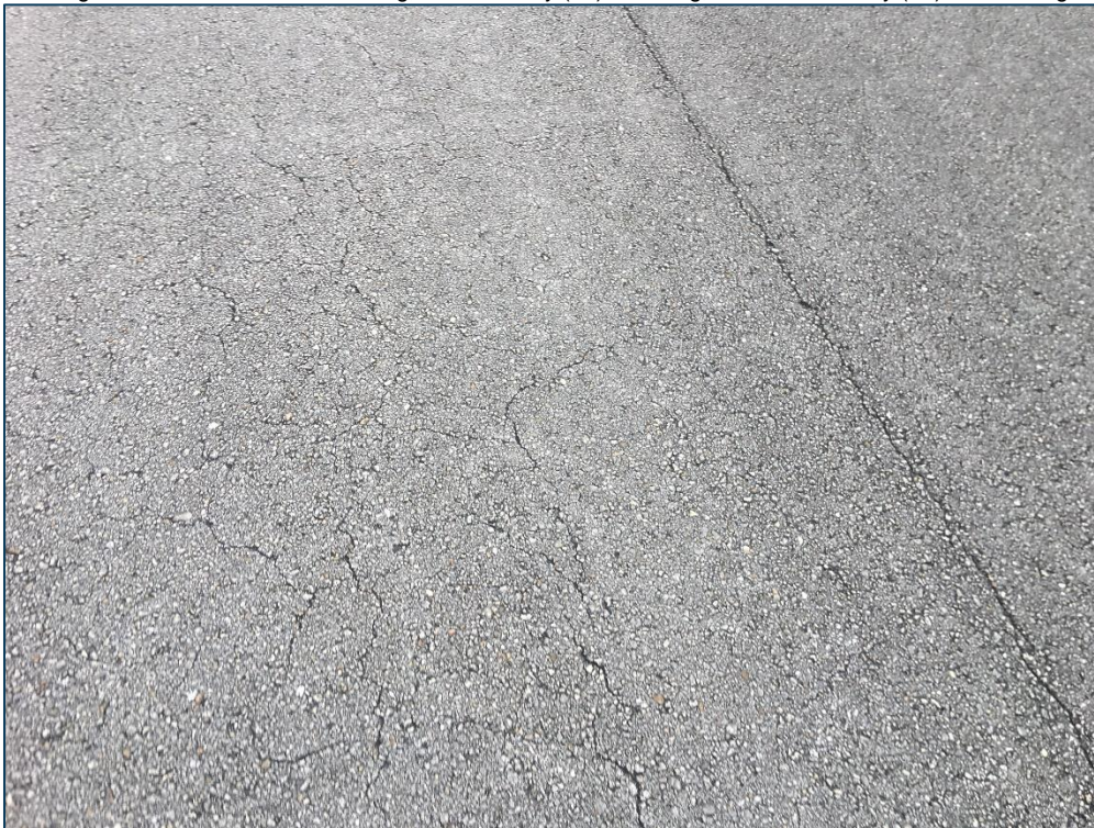
TW G, Section 723, Sample Unit 119 - Low Severity (43) Block Cracking, Low Severity (48) Longitudinal & Transverse Cracking, Low Severity (52) Raveling, and Low Severity (57) Weathering
