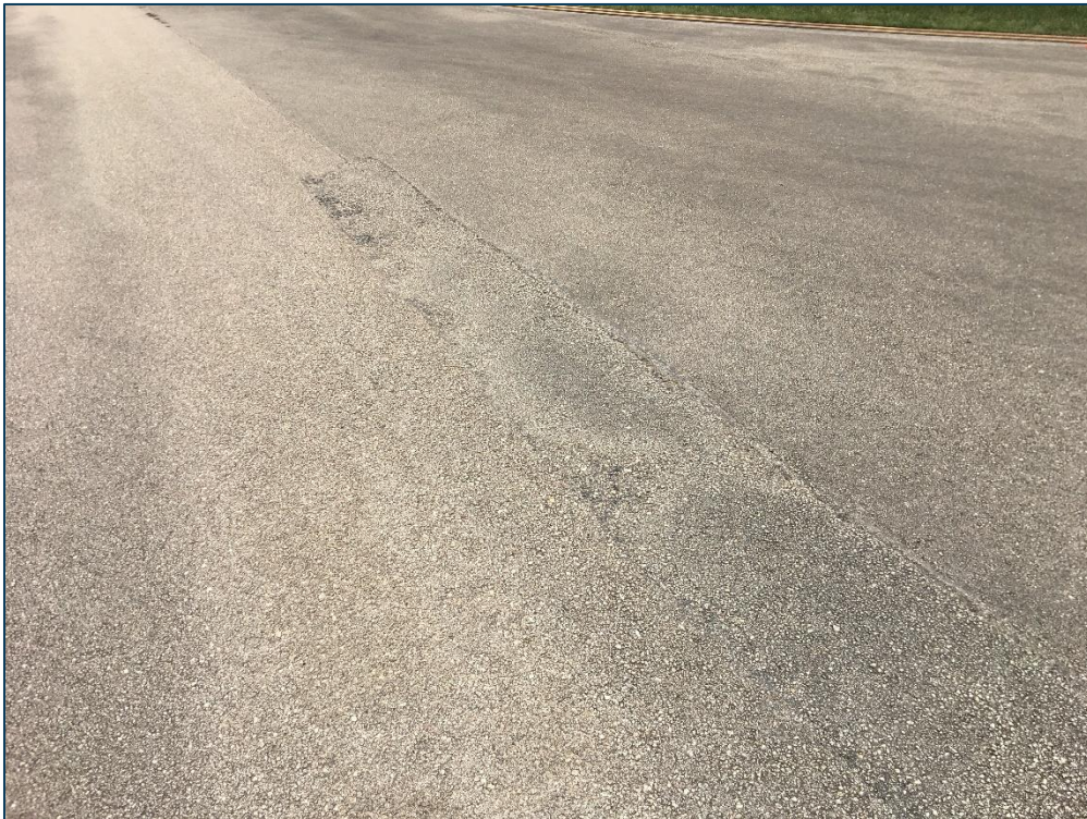
TW E, Section 520, Sample Unit 110 - Low Severity (50) Patching, Low Severity (52) Raveling, and Low Severity (57) Weathering
