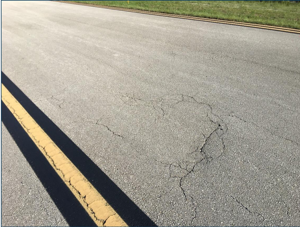
TW F, Section 607, Sample Unit 144 - Medium Severity (41) Alligator Cracking, Low Severity (45) Depression, Low Severity (48) Longitudinal & Transverse Cracking, Low Severity (52) Raveling, and Low Severity (57) Weathering
