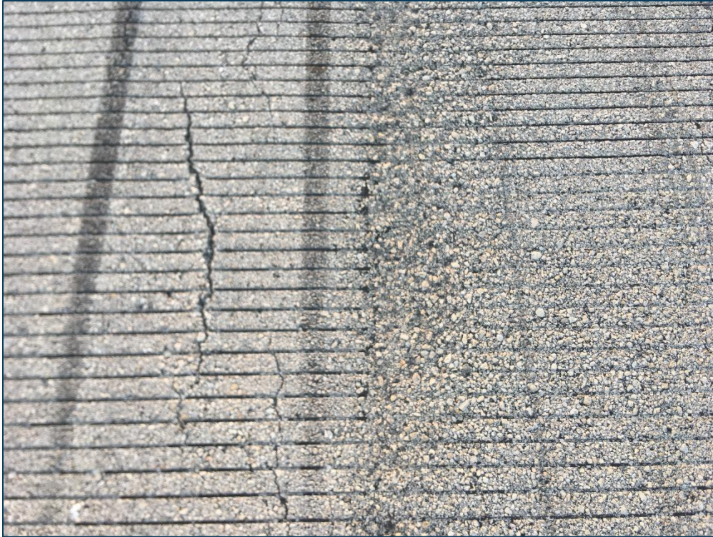
RW 9-27, Section 6105, Sample Unit 347 - Severity (48) Longitudinal & Transverse Cracking, Medium Severity (48) Longitudinal & Transverse Cracking, Low Severity (52) Raveling, and Low Severity (57) Weathering
